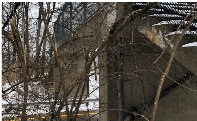
Photograph 1: Overall Bridge Condition
