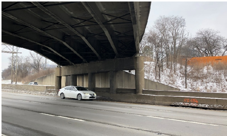
Photograph 1: Bridge HAM-75-0125 existing forward abutment/retaining wall
