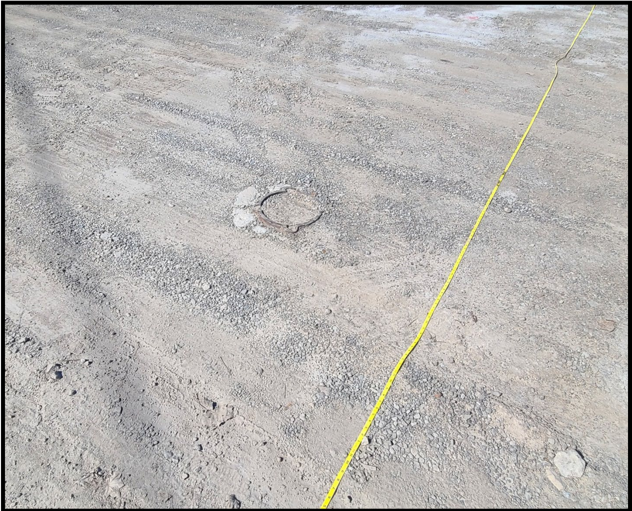
Photograph 1. Buried Hydraulic Lift Outer Casing.
