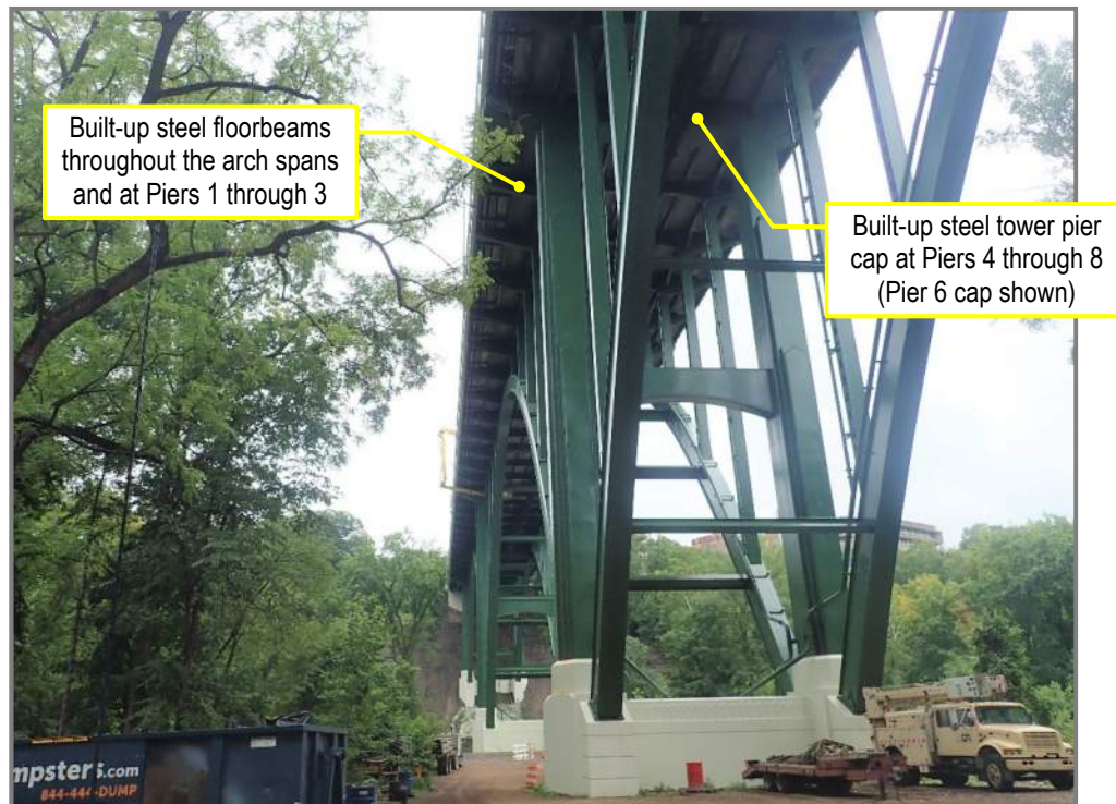
Figure 2 – CUY-10-0869 (SFN 1801325) overall view of Spans 6 through 9 looking east.
