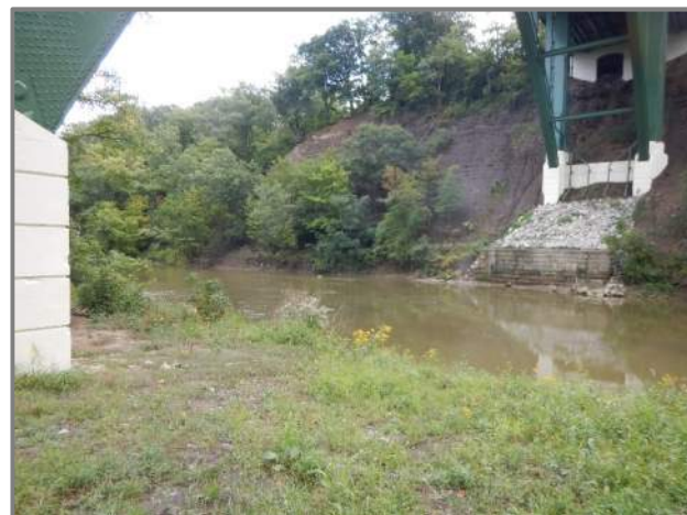
Photo 44 – View of the channel below Span 8 (looking northeast).
