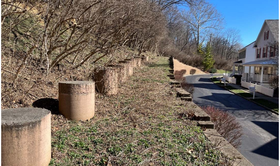
Photograph 2: Existing retaining walls downslope of US-50
