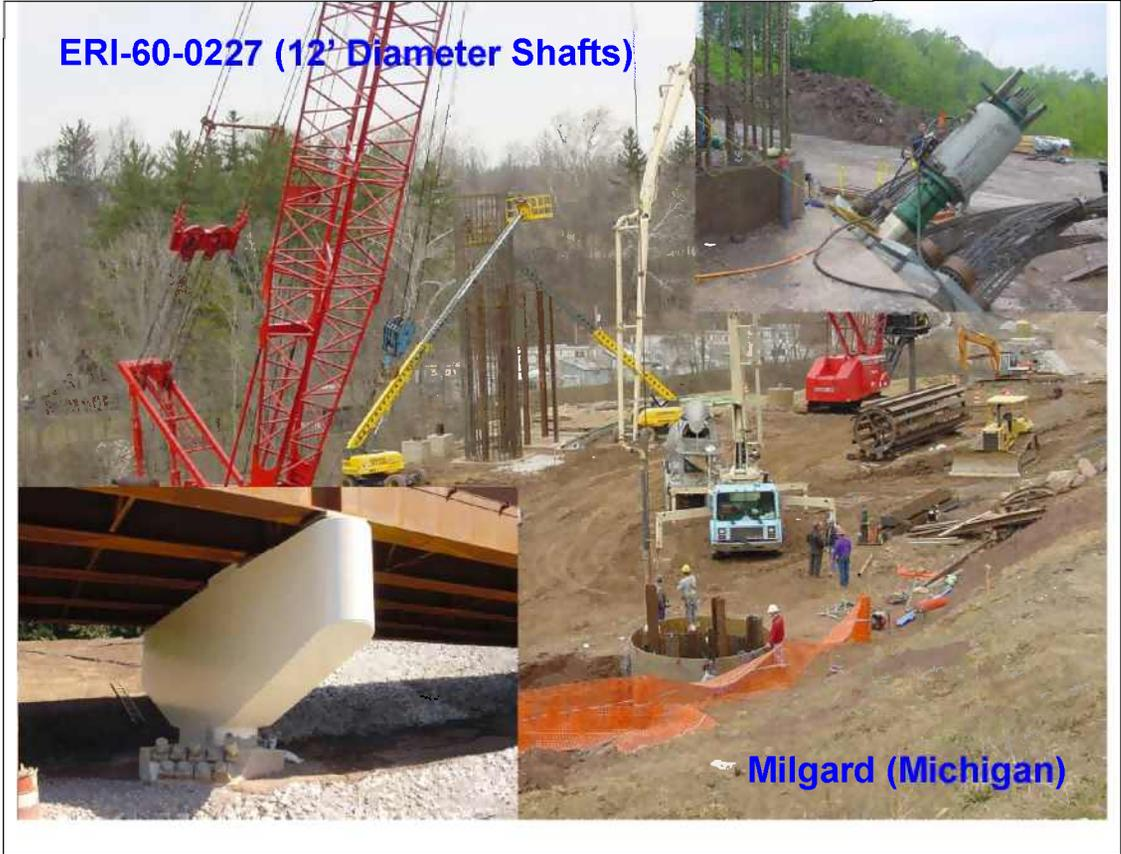
Figure 9.6: Example of a drilled shaft tied back for resistance of lateral soil forces
