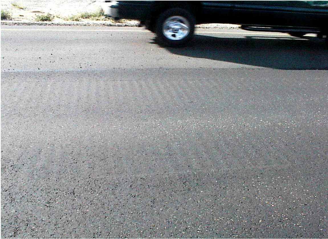
Figure 6. Visible Drum Impacts from Excess Roller Speed.
