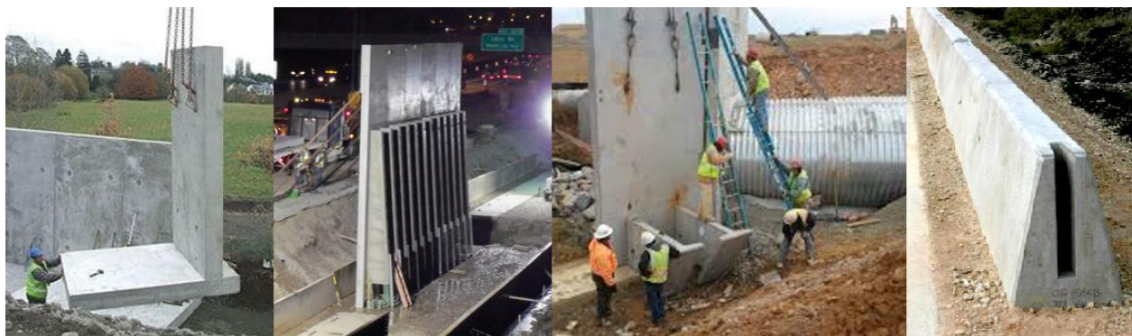
Figure 1500-7: Precast Gravity and Semigravity Walls
