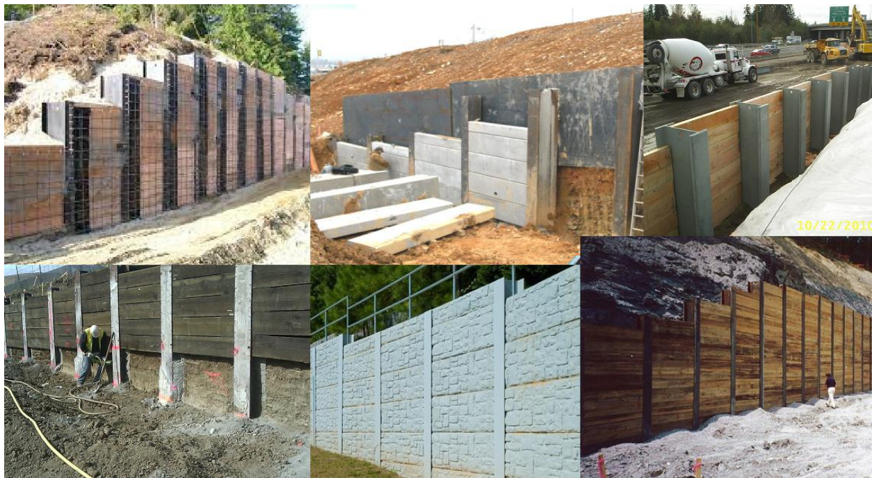
Figure 1500-17: Soldier Pile Walls
