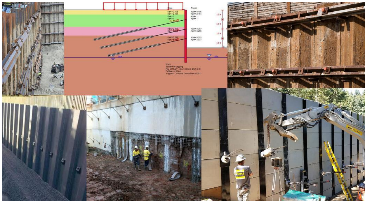
Figure 1500-19: Anchored Walls
