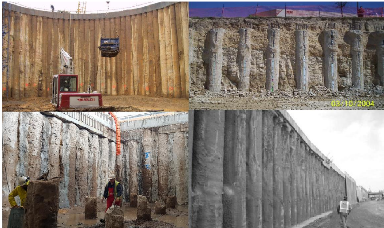
Figure 1500-16: Drilled Shaft Walls
