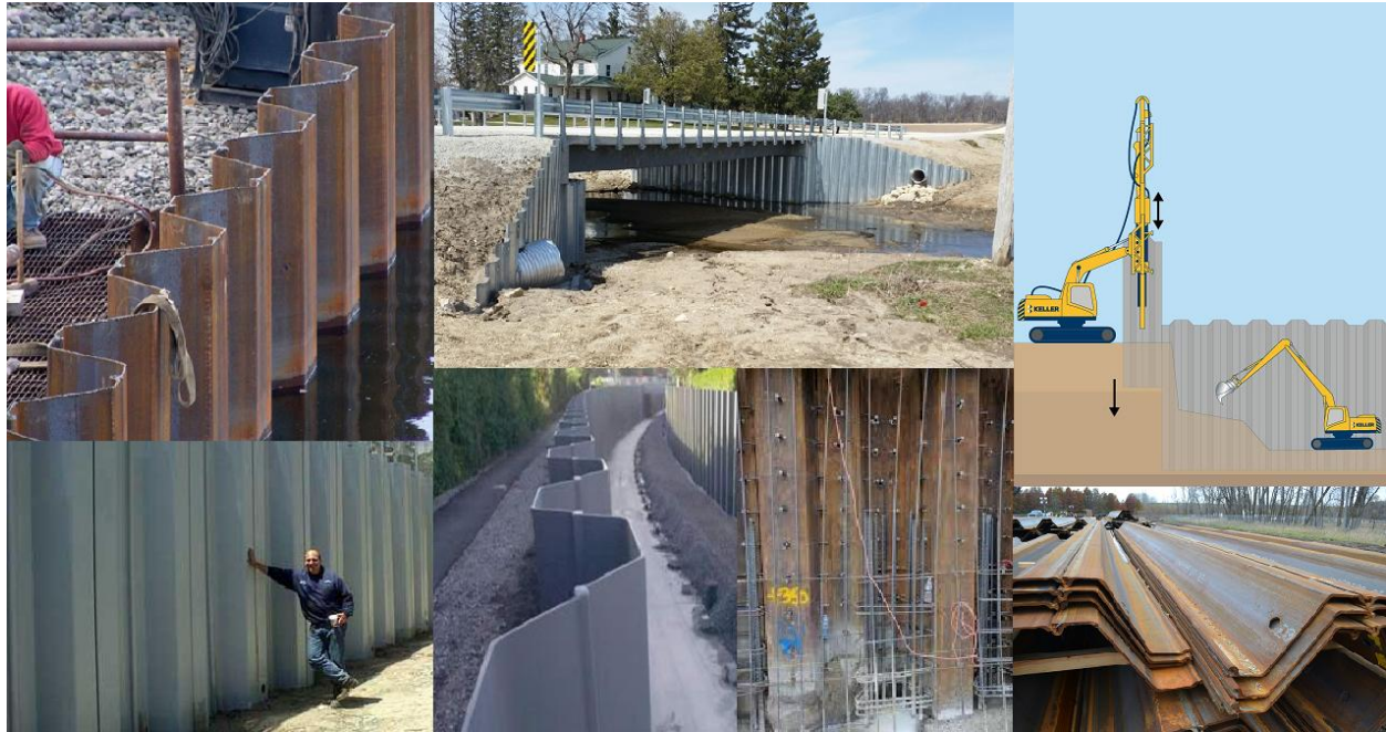
Figure 1500-18: Steel Sheet Pile Walls
