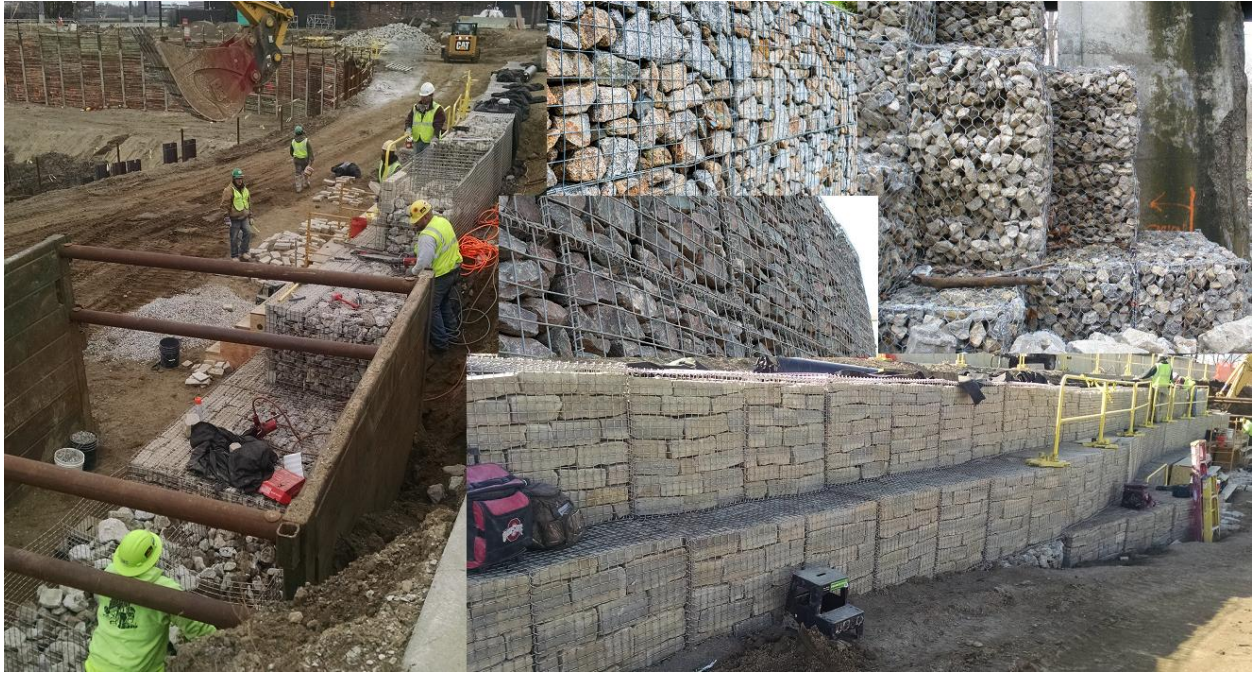
Figure 1500-13: Gabion Walls
