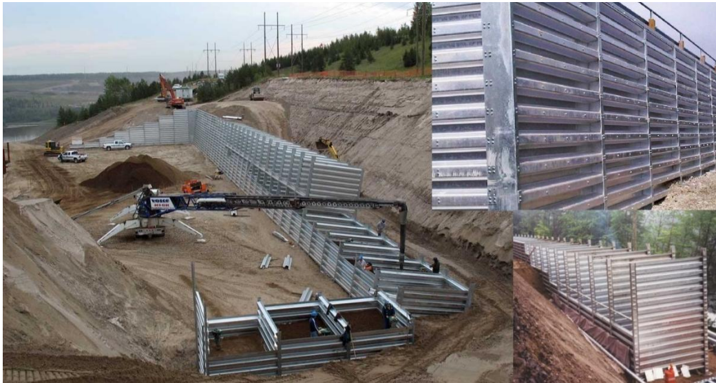
Figure 1500-10: Metal Bin Walls
