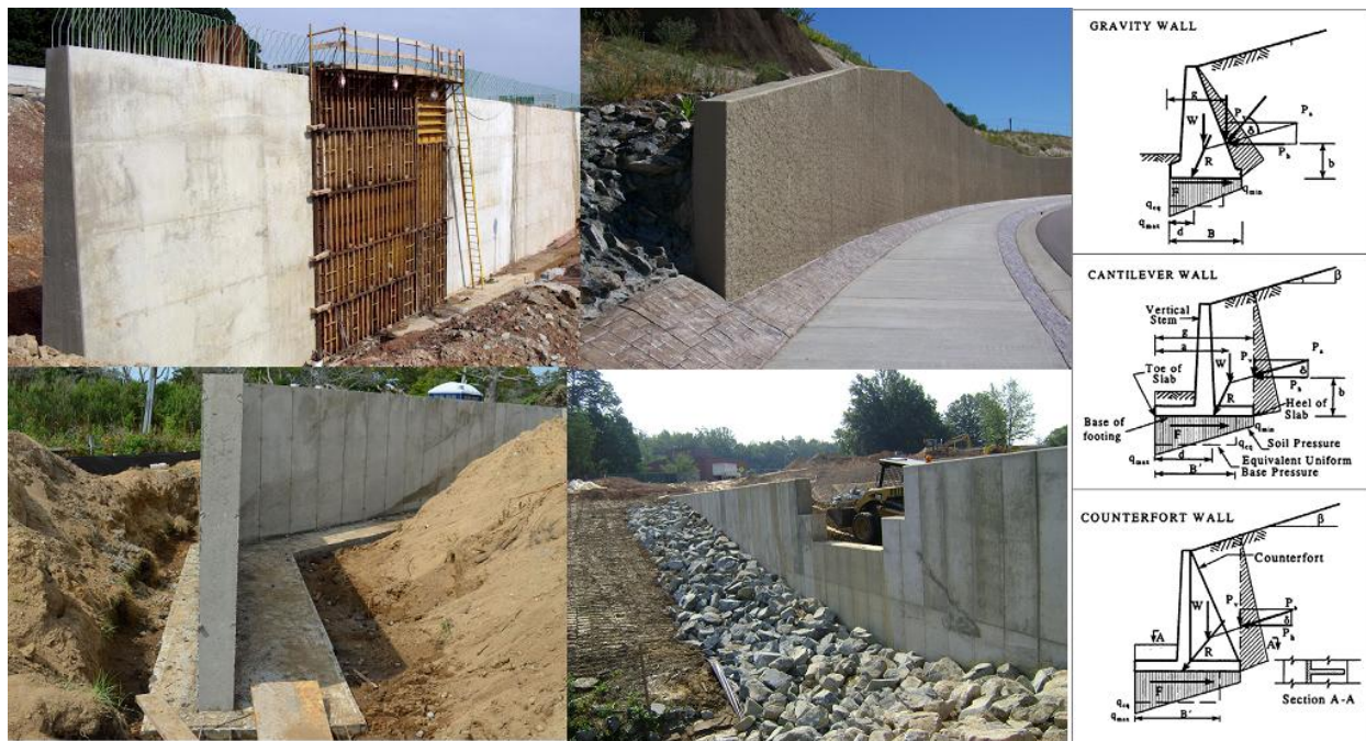
Figure 1500-6: Rigid Gravity and Semigravity Walls
