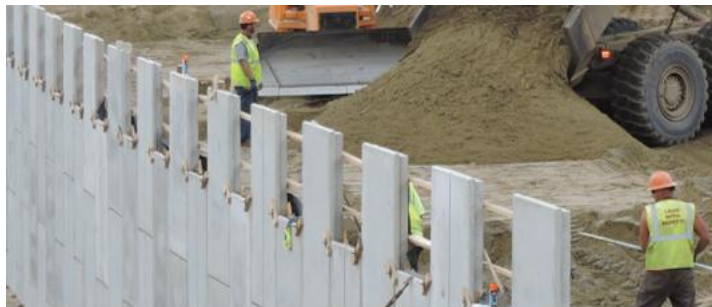
Figure 1500-14: Mechanically Stabilized Earth (MSE) Walls
