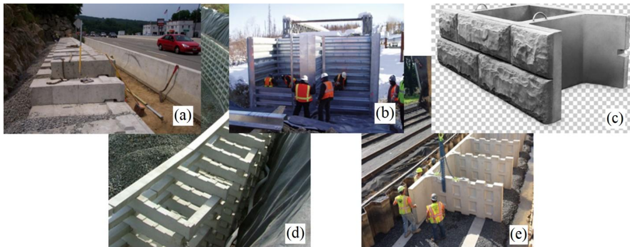
Figure 1500-8: Prefabricated Modular Walls
