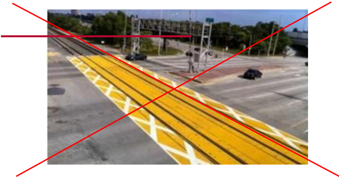
Figure 11-65: Reserved for Future Use Example Dynamic Envelope Markings with Cross Hatching with Optional Supplemental “Do Not Block Intersection” Markings (Source: Federal Railroad Administration)
