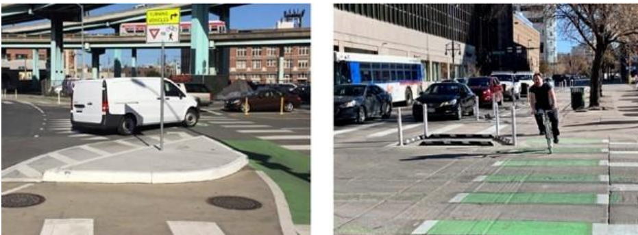
Figure 6-31: Protected Corner Treatment Examples: Concrete Corner Island (left) and Flexible Delineators and Rubber Parking Stops (right)
