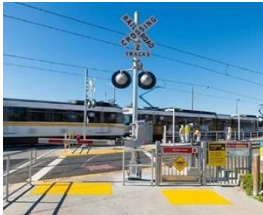
Figure 11-98: Automatic Gate for Pedestrian Facilities with an Emergency Swing Gate (Source: Los Angeles County Metropolitan Transportation Authority)
