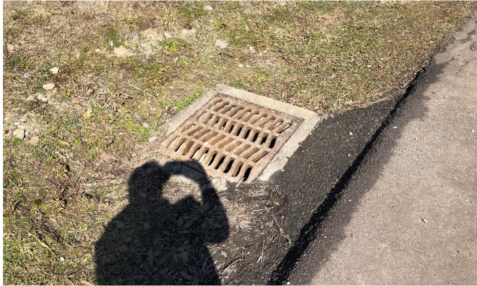
Photograph 3. Underdrains at end of Drainage Ditches
