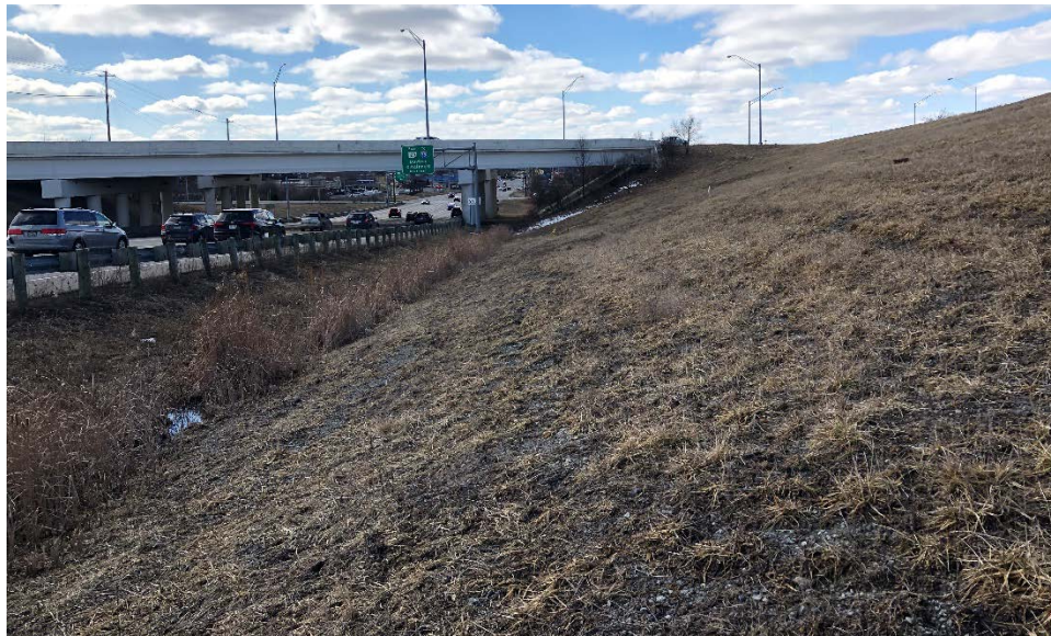
Photograph 2. Slope of Embankment Between SR-129 and Northern Access Ramps
