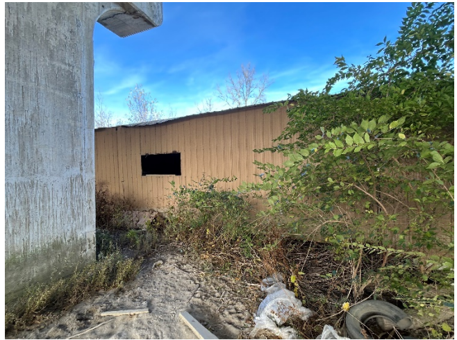
View of the southern side of the building.
