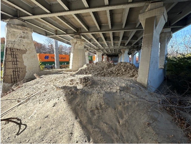
View of stockpiled material facing west.
