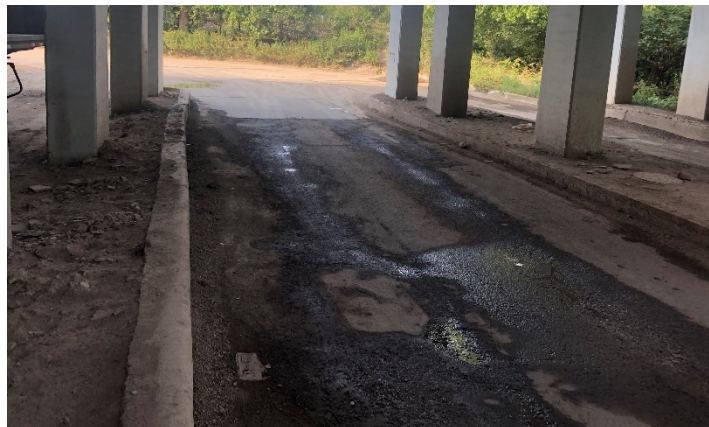
Photograph 3: Asphalt portion of Chaincraft Rd
