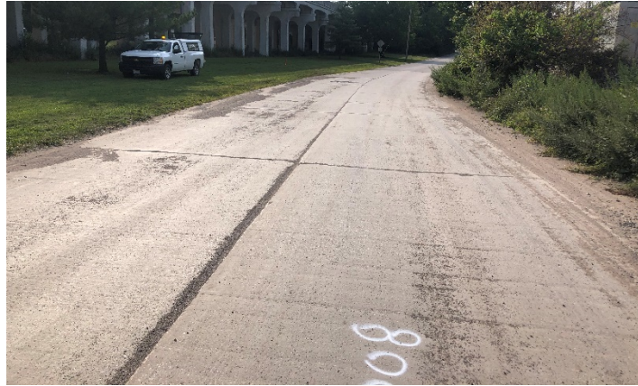
Photograph 4: Concrete portion of Chaincraft Rd
