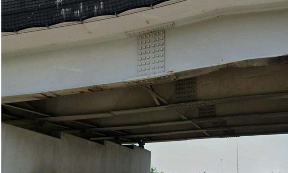
Photograph 3: Failed Expansion Joint Above Eastern Abutment
