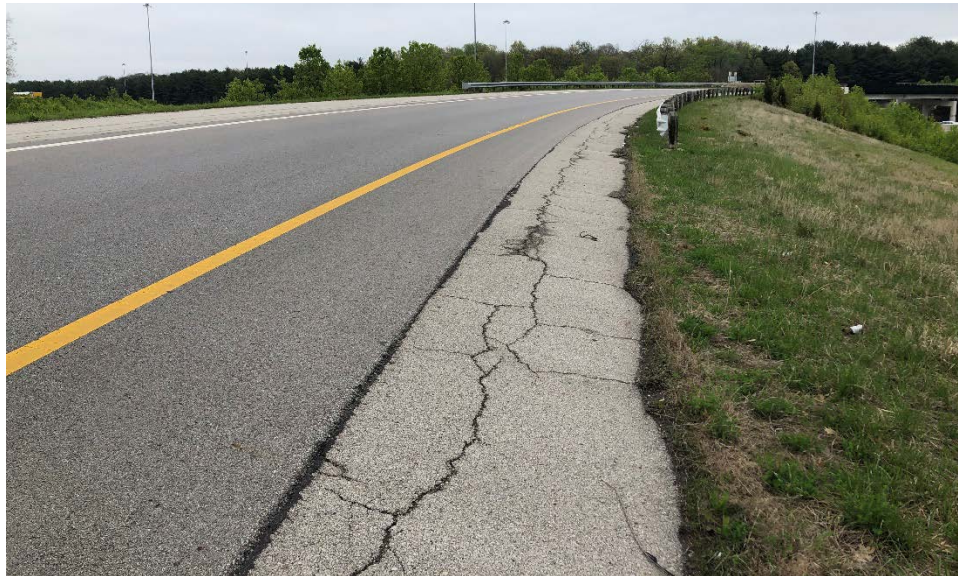
Photograph 9: Overall Pavement Condition of Ramp O
