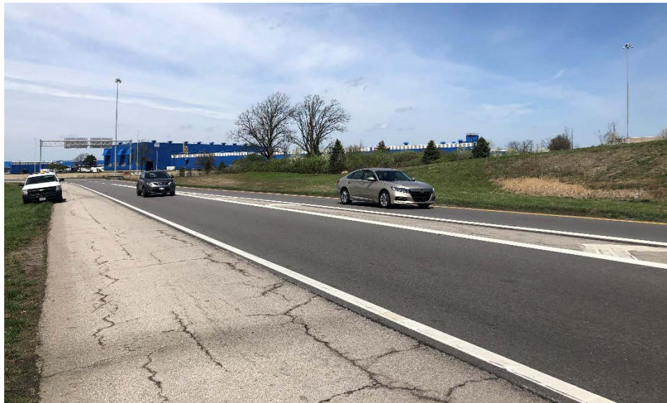
Photograph 1: Overall Pavement Condition of Ramp P and Ramp M
