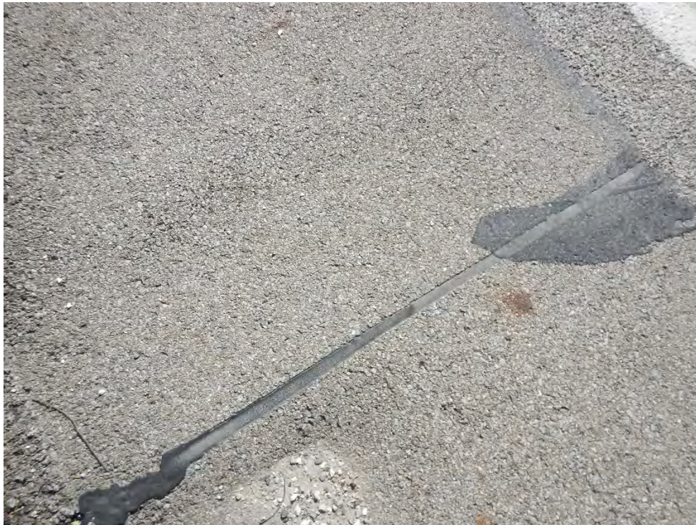
Photo 12: Tar from the structure deck
