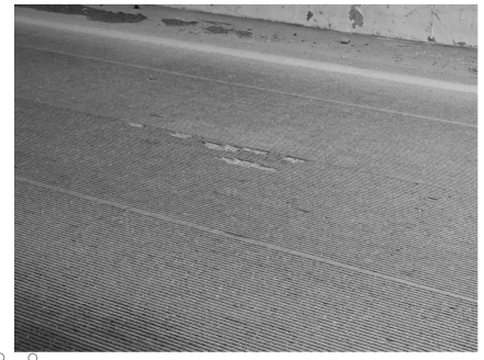
2'X2' REPAIR PHOTO
