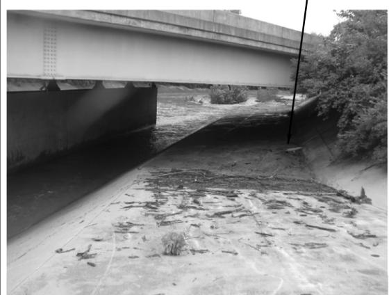
**DAMAGED DRAINAGE OUTLET AT REAR ABUTMENT**
