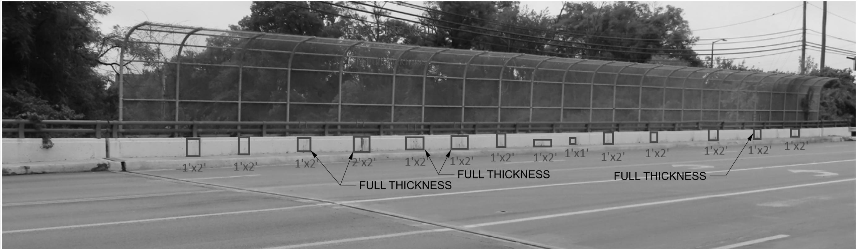
**EAST PARAPET (INTERIOR FACE) PATCHING & FULL DEPTH REPAIR DETAILS**
