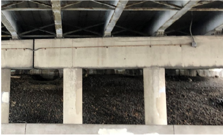
Photograph 3: Riprap on Spill-through Slope
