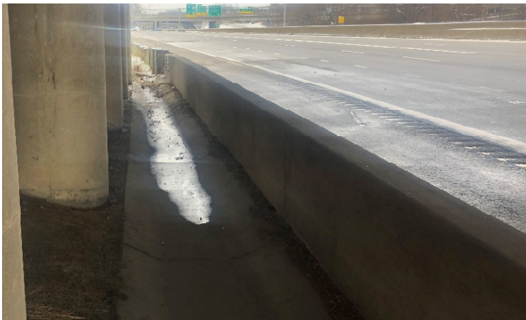
Photograph 4: Concrete Drainage Channels
