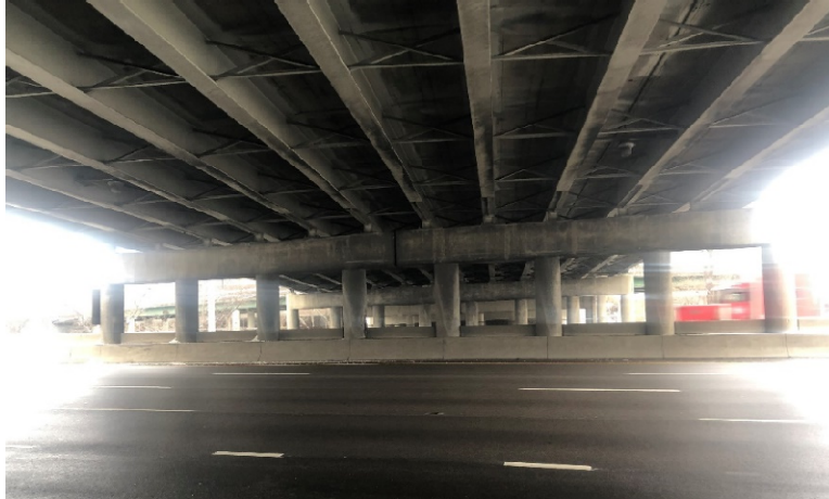
Photograph 1: Overall Condition of Underside of Deck
