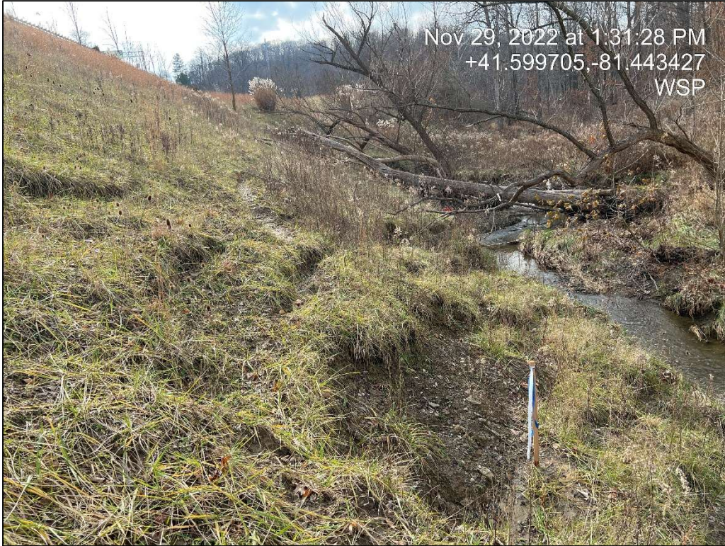
Figure 4: Existing Conditions at the Toe (Looking Southwest)
