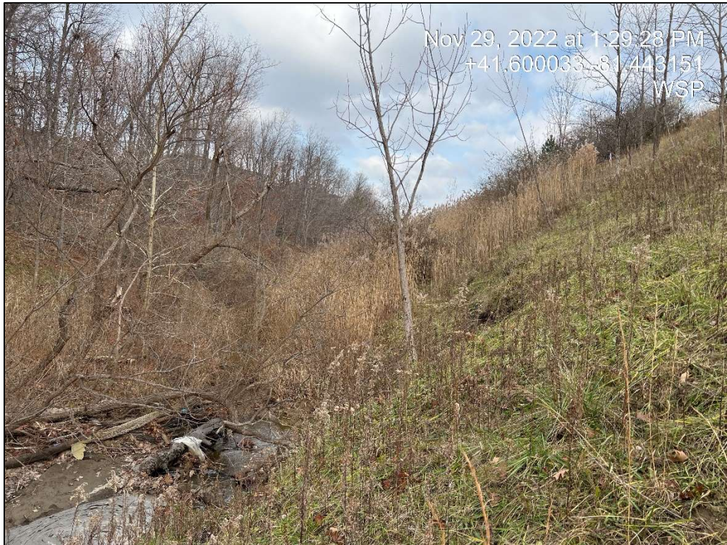
Figure 3: Existing Conditions at the Toe (Looking Northeast)
