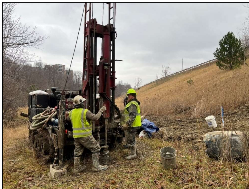
Figure 7: Site Photograph Taken During Drilling
