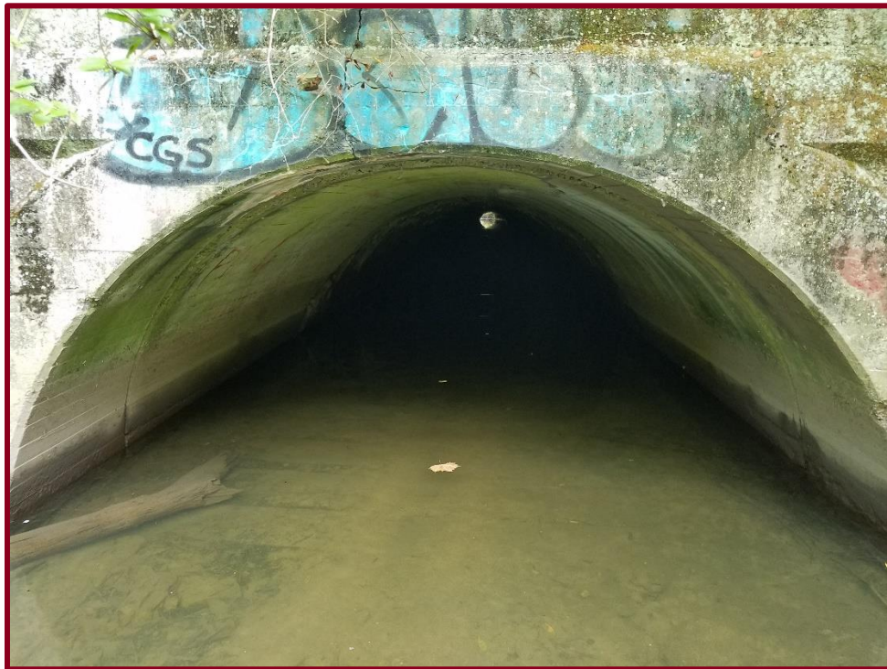
Inlet Showing Concrete Struts
