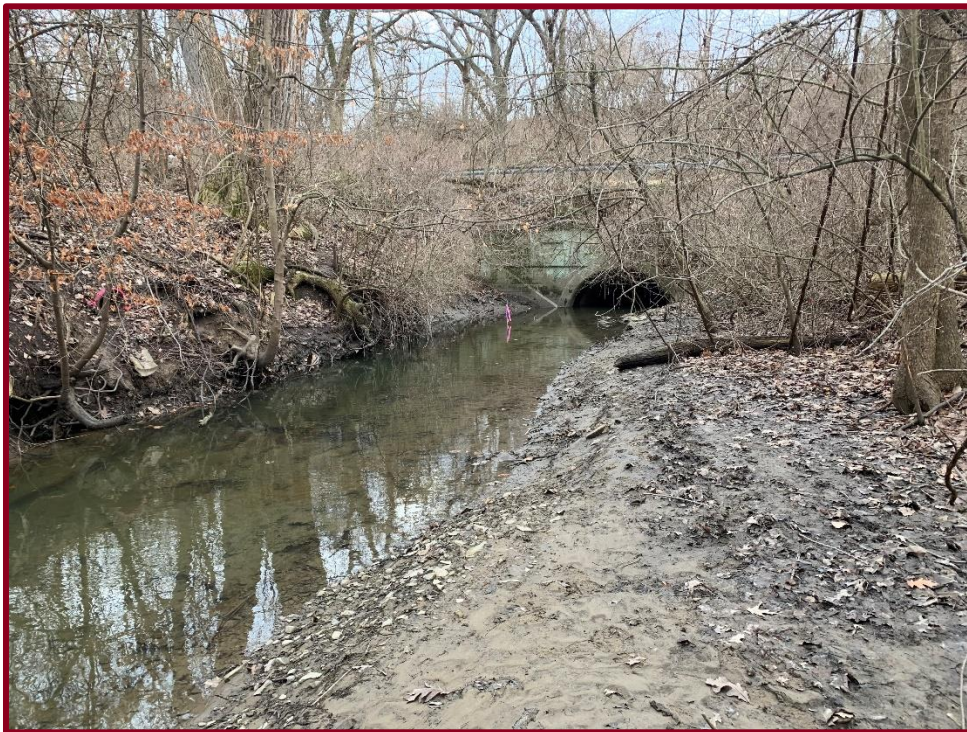
Channel Downstream of Culvert Looking Upstream (West)
