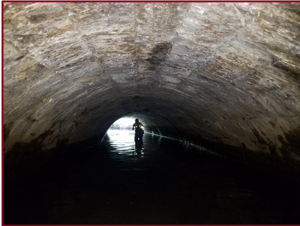
Inside Culvert Looking Downstream (East)
