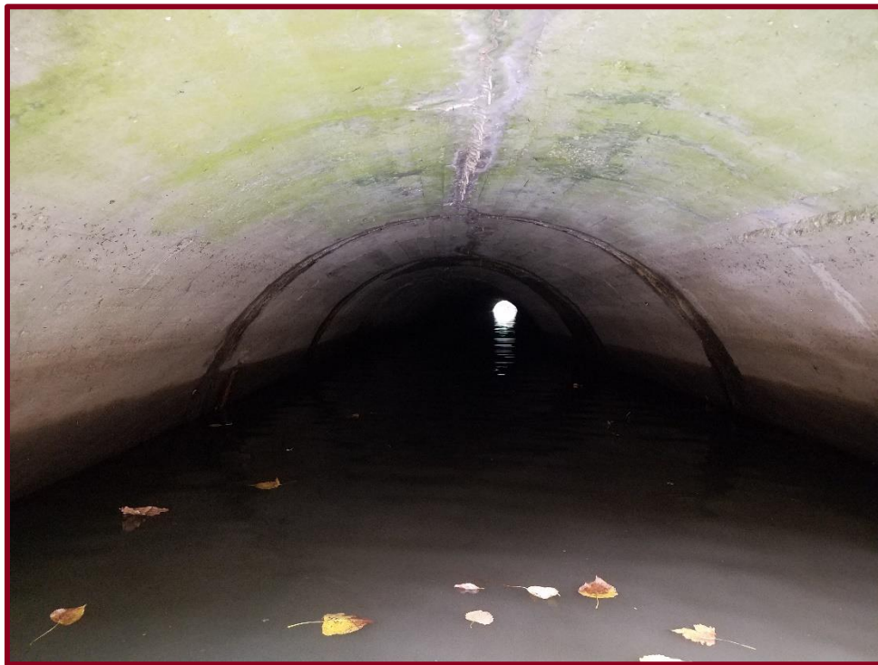
Inside Culvert Near Outlet Looking Upstream (West)
