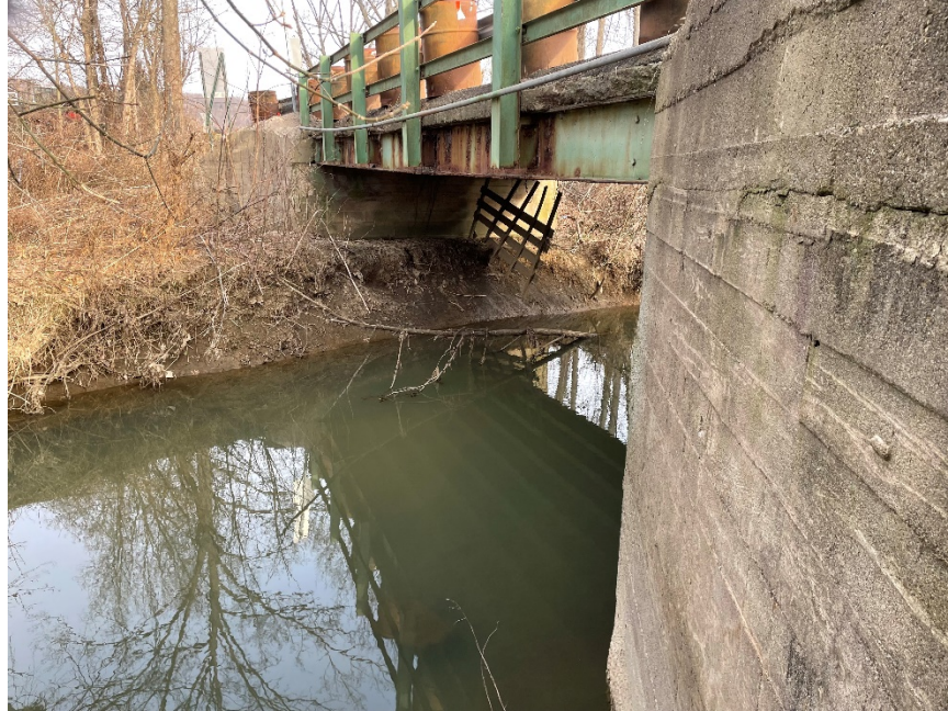
Upstream Bridge opening
