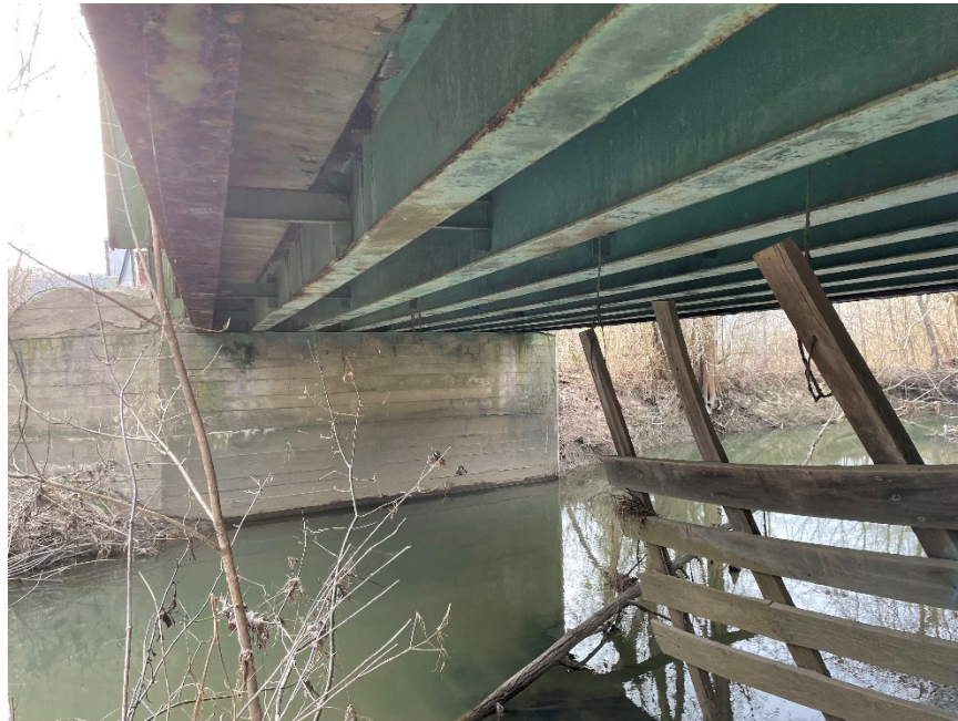
Typical Underside of Bridge opening
