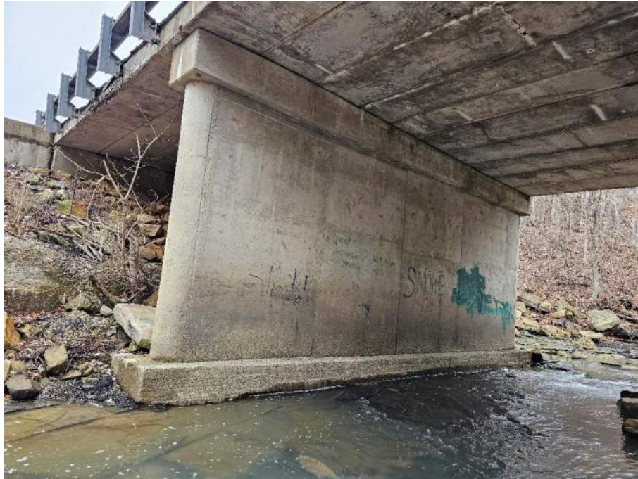
Photograph 2: Scour evidence at the base of the northern pier
