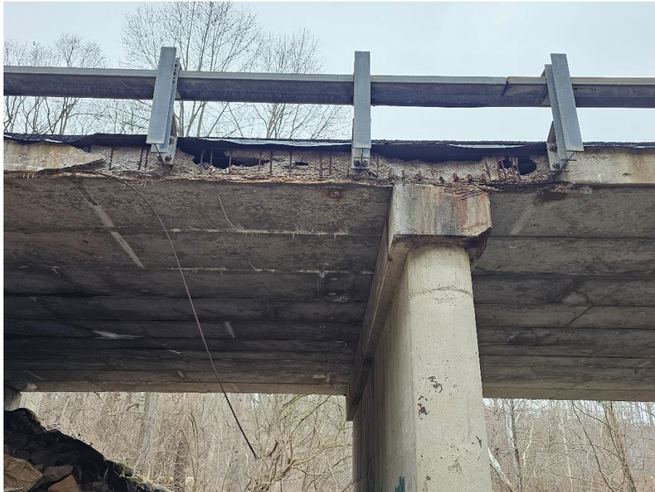
Photograph 5: Bridge deck and box beam
