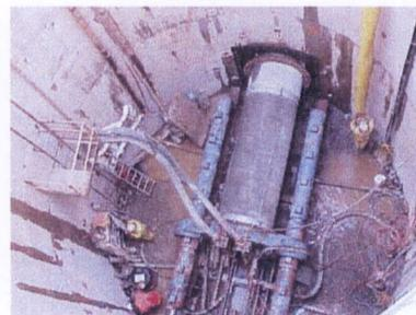
Microtunneling from a caisson
