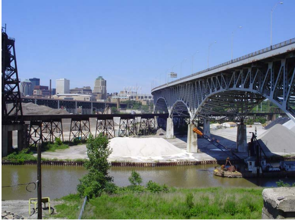
Photo 3: East facing view of east bank of Cuyahoga River bulkhead to be replaced.
