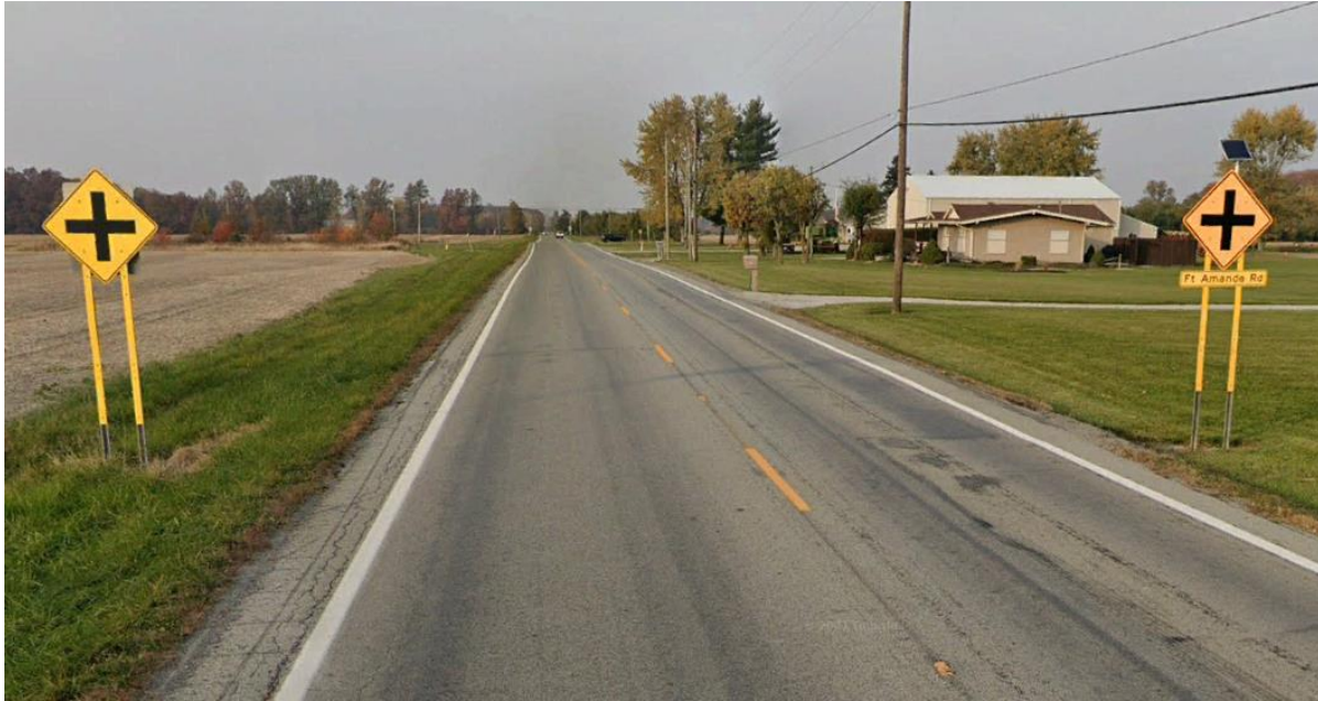
Figure 3: Northbound SR 501 - Dual, LED Enhanced Intersection Warning Signs
