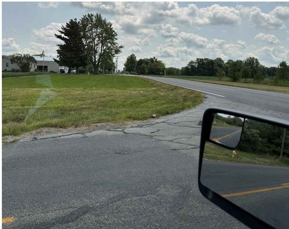
Figure 8: Westbound Ft Amanda Rd looking South
