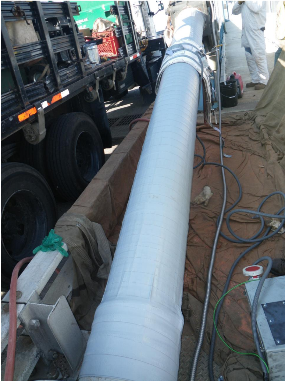
Figure 4.11- Neoprene Wrap Heat-Bonding Operation
