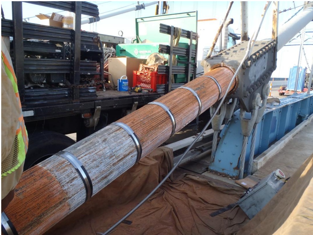
Figure 4.9– Recompacted Cable with Banding Straps
