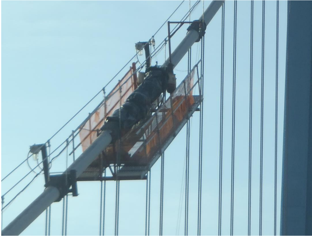
Figure 4.2 – Access Platform Installation
