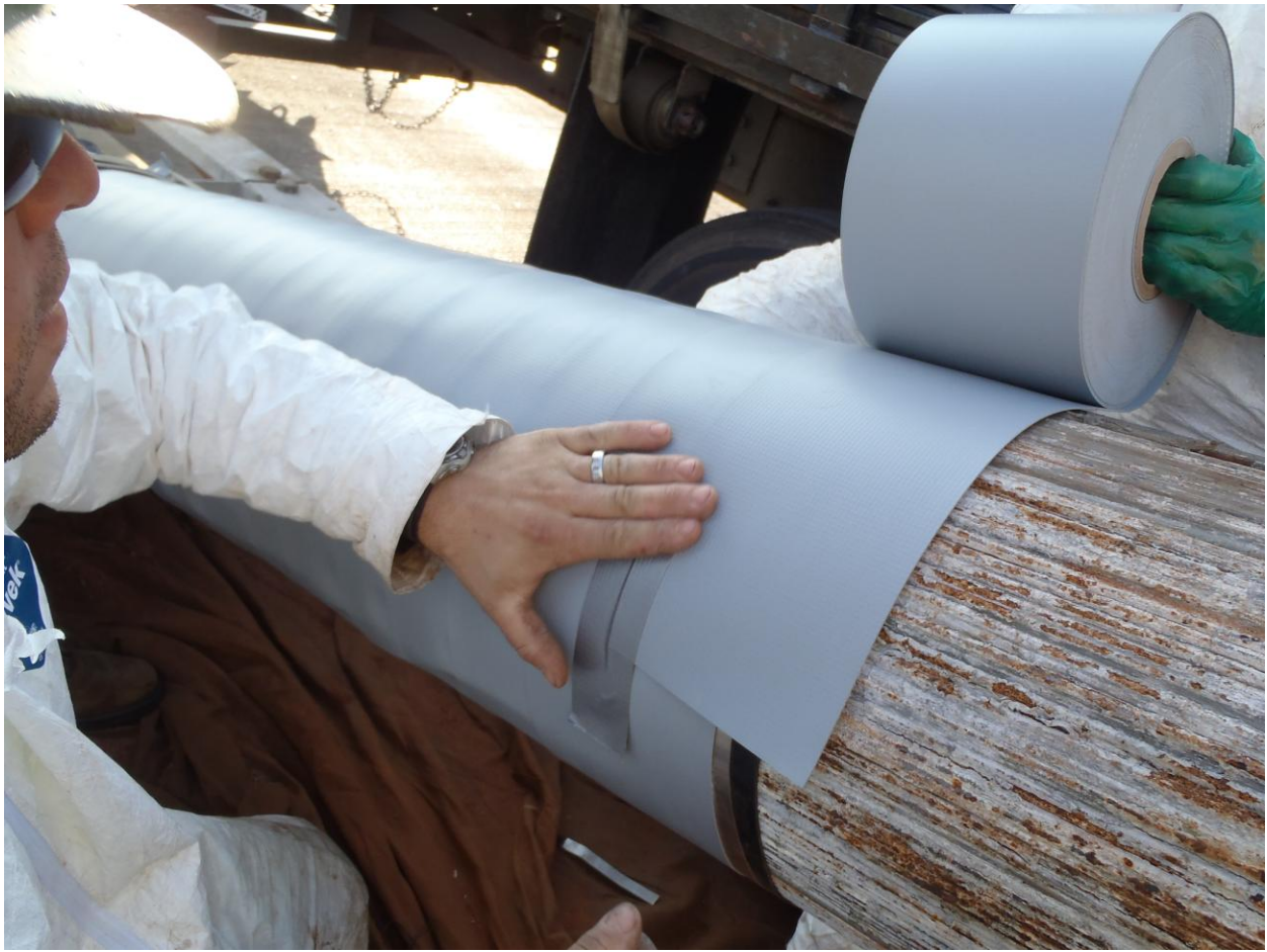
Figure 4.10– Neoprene Wrap Installation
