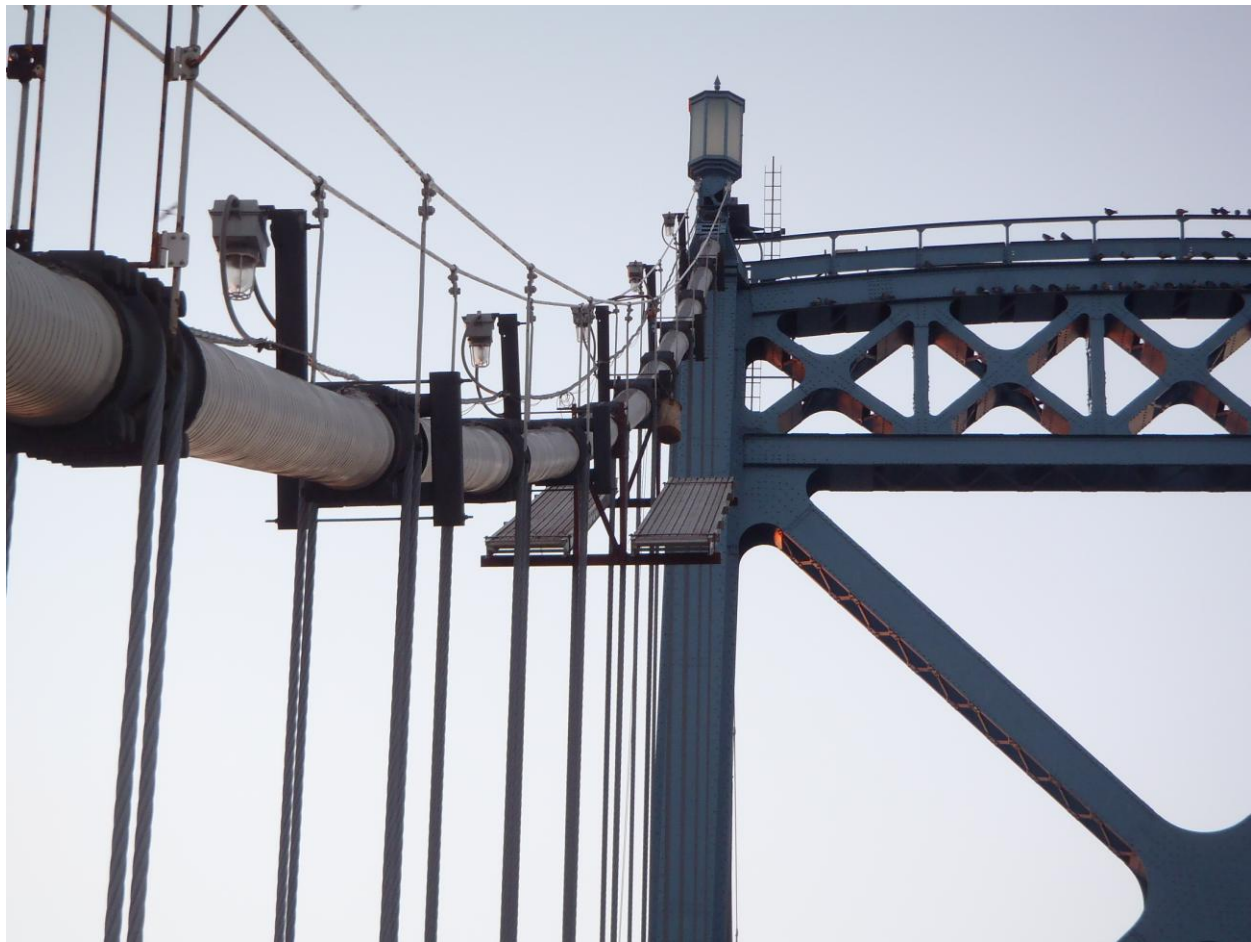
Figure 4.1 – Access Platform Installation
