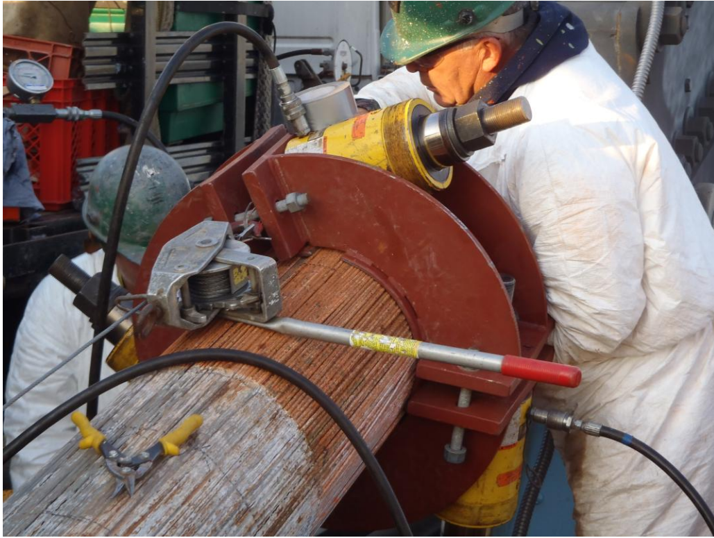
Figure 4.8– Recompacting Cable
