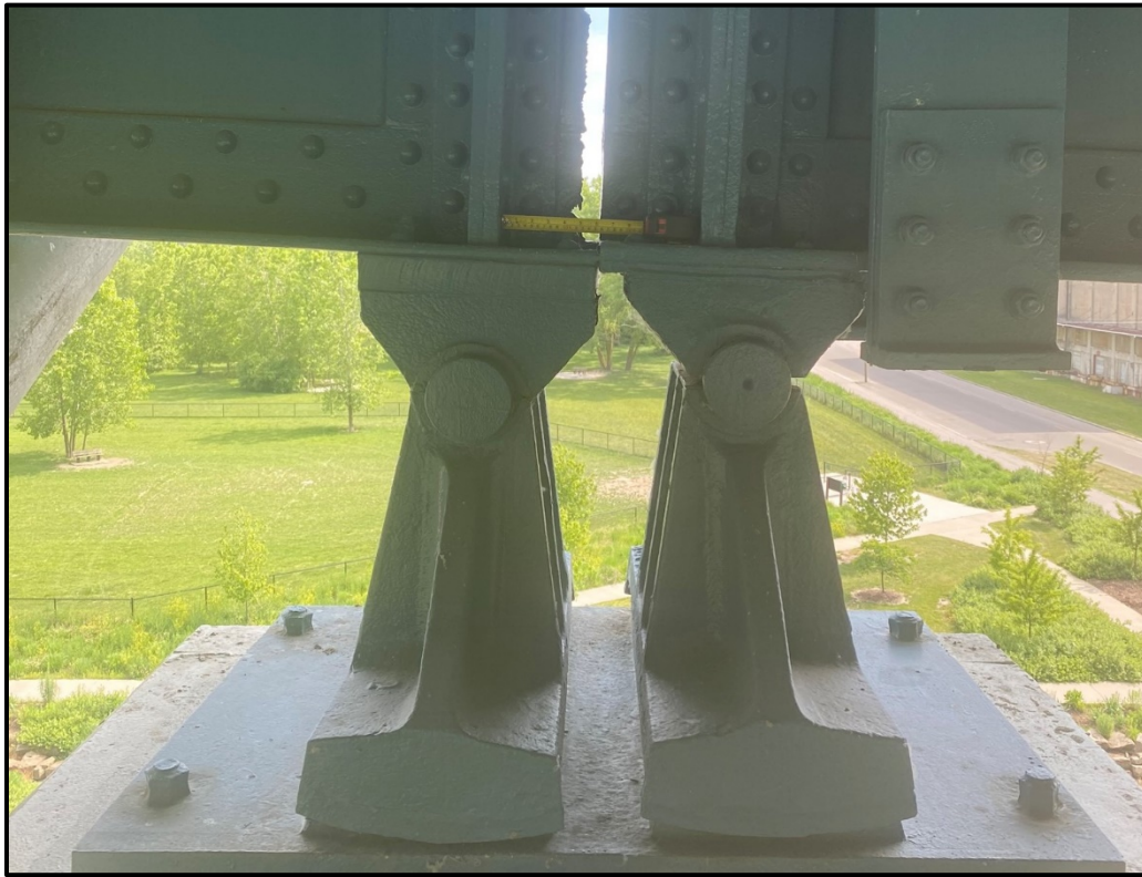
Photo 25 - LG Bearings at Pier 2W are both Tilted approximately 10 Degrees Towards Each Other, Resulting in Girder Contact and Restricted Movement
