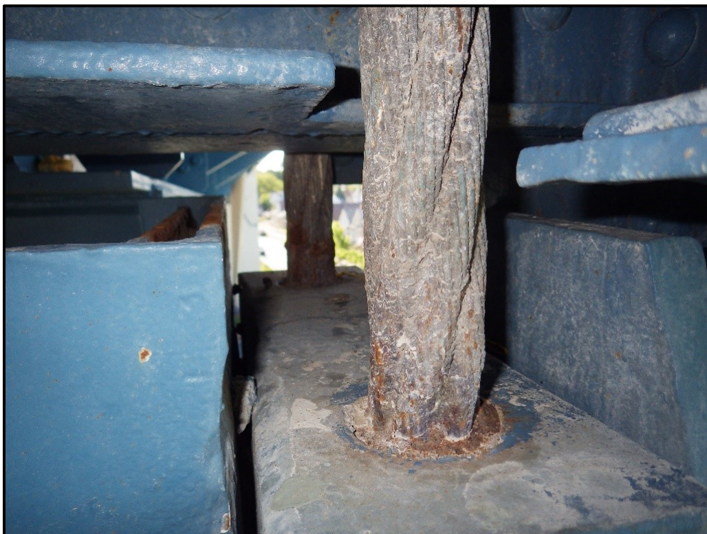
Photo 51 - Typical Corrosion and Section Loss at the Base of the Wire Ropes at the Cable Bents. East cable bent, south column, northwest suspender rope shown.
