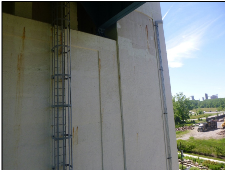
Photo 29 - Typical Rust Staining of Pier Wall (West Face of Anchorage A shown)
