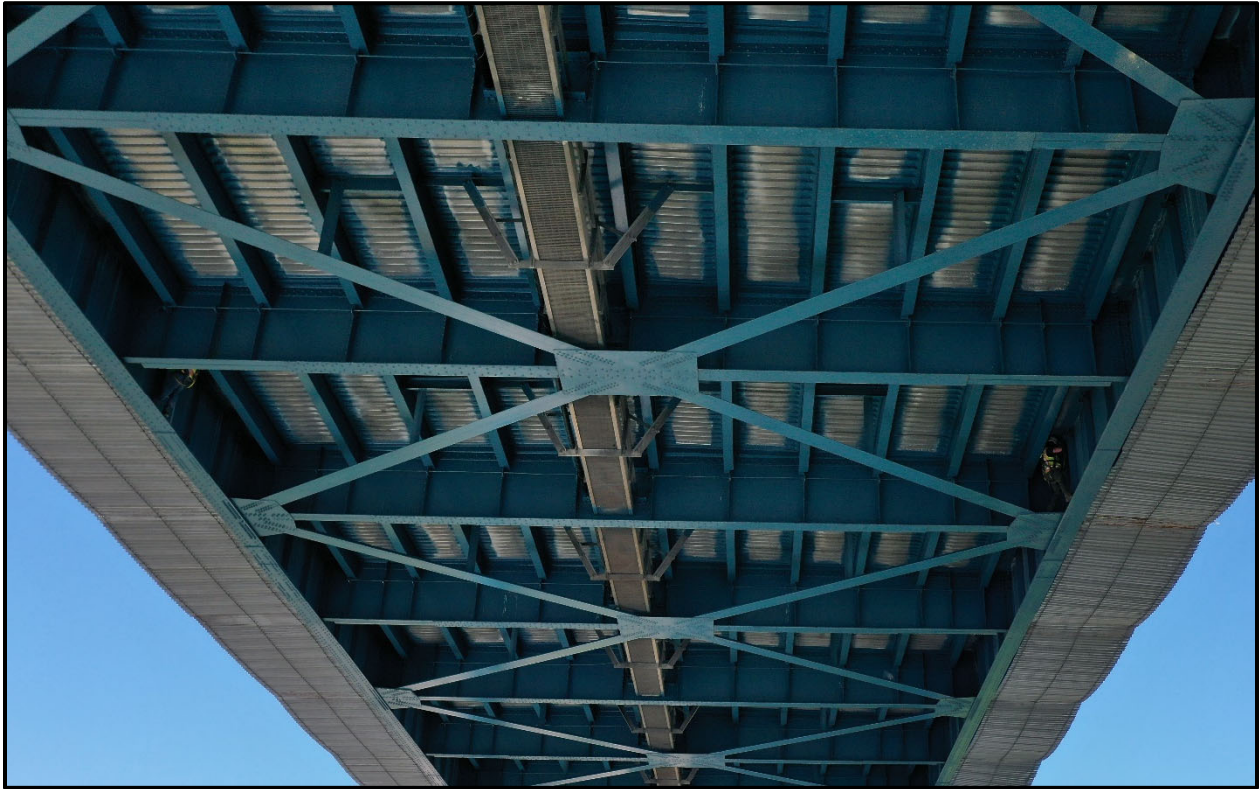
Photo 4 - Suspension Span Girders
