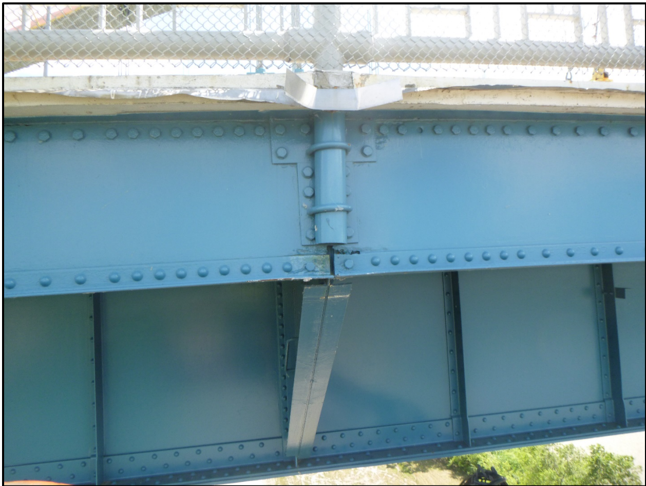
Photo 19 – Typical Painted Over Section Loss at Sidewalk Stringer Connections
