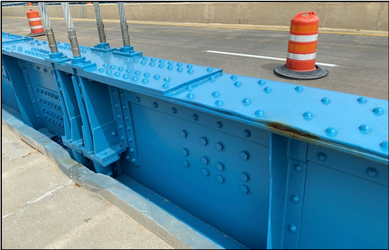
Photo 16 - Typical Condition of Top Flange/Web of Suspension Girders
