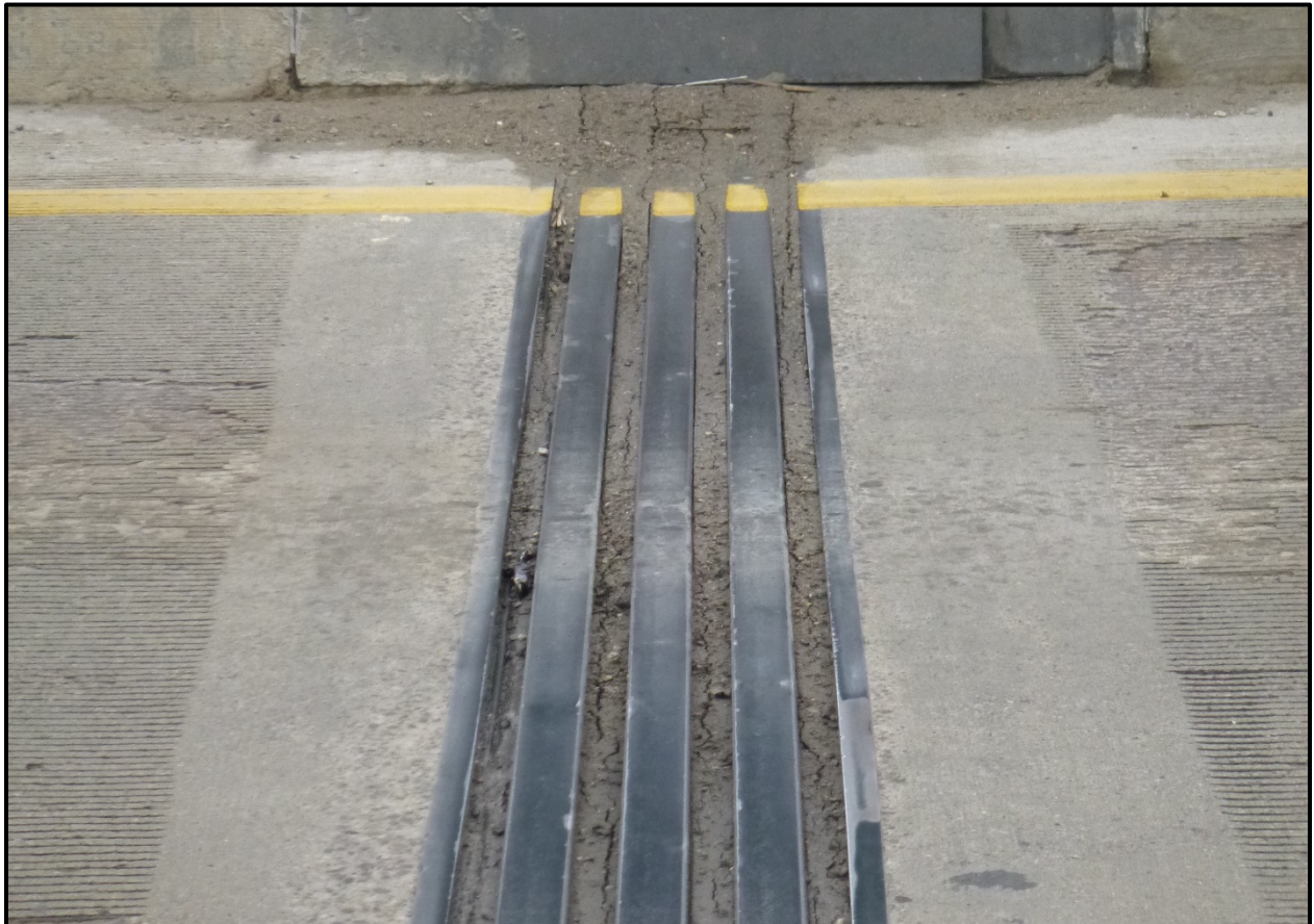
Photo 9 - Typical Modular Expansion Joint Condition
