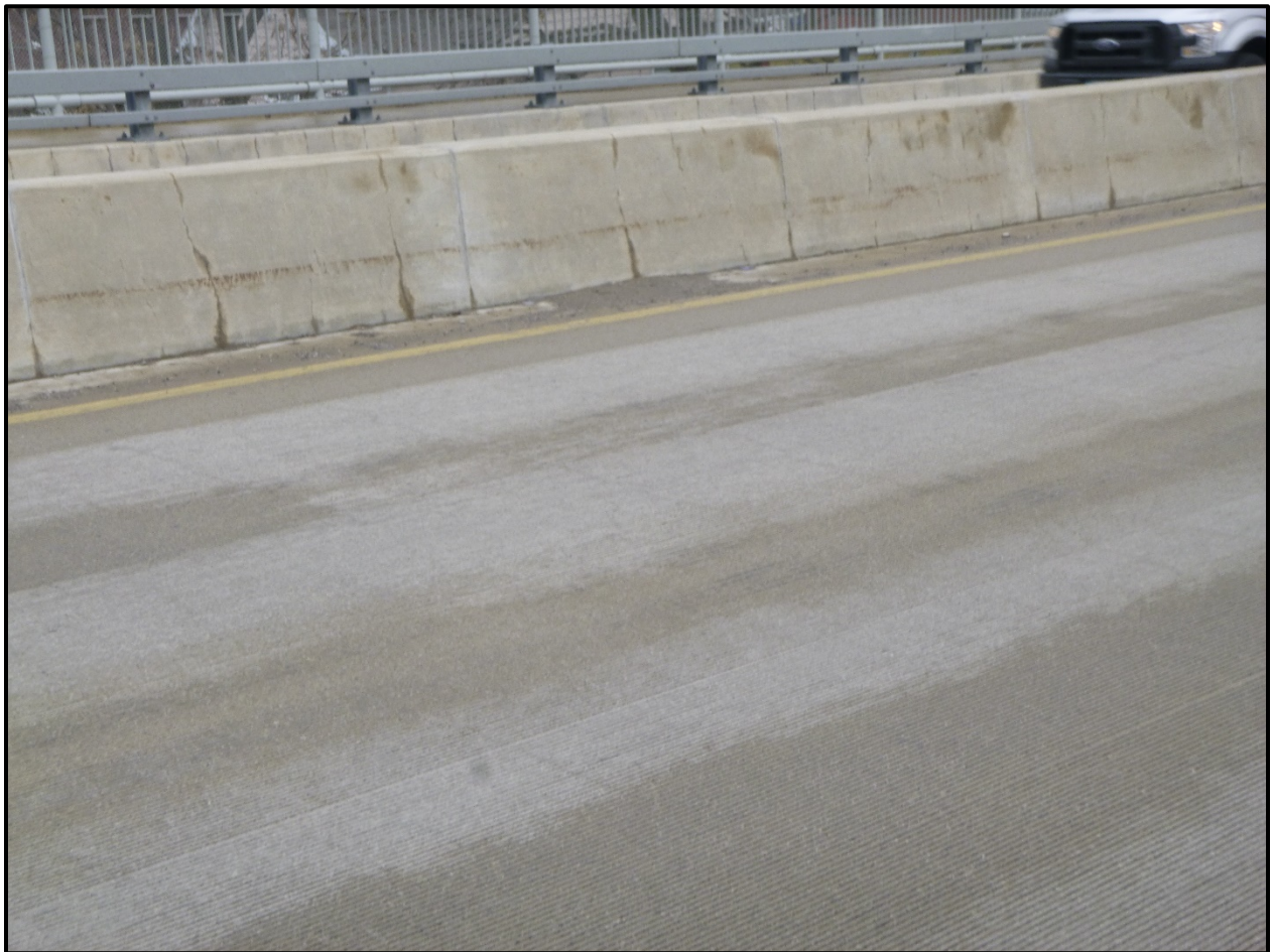
Photo 11 - Typical Vertical Cracks in Median Parapet
