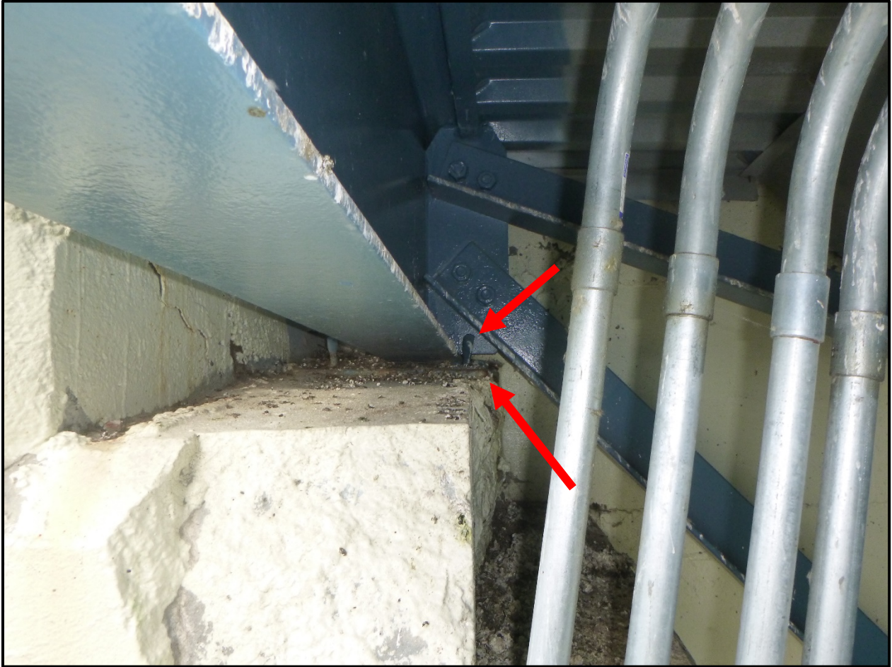
Photo 27 - S2 Bearing Plate at Anchorage A Beginning to Undermine. Also note Section Loss to Bearing Anchor Bolts
