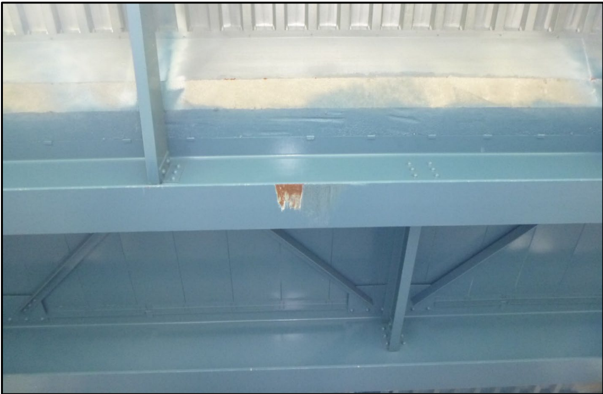
Photo 17 - Impact Damage to Bottom Flange of Beam S02 in Span 14E
