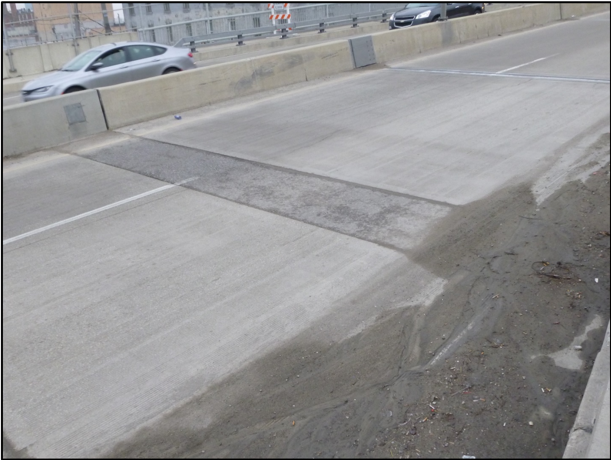
Photo 69 - Typical Approach Slab Termination Condition (Eastbound, West Approach shown)
