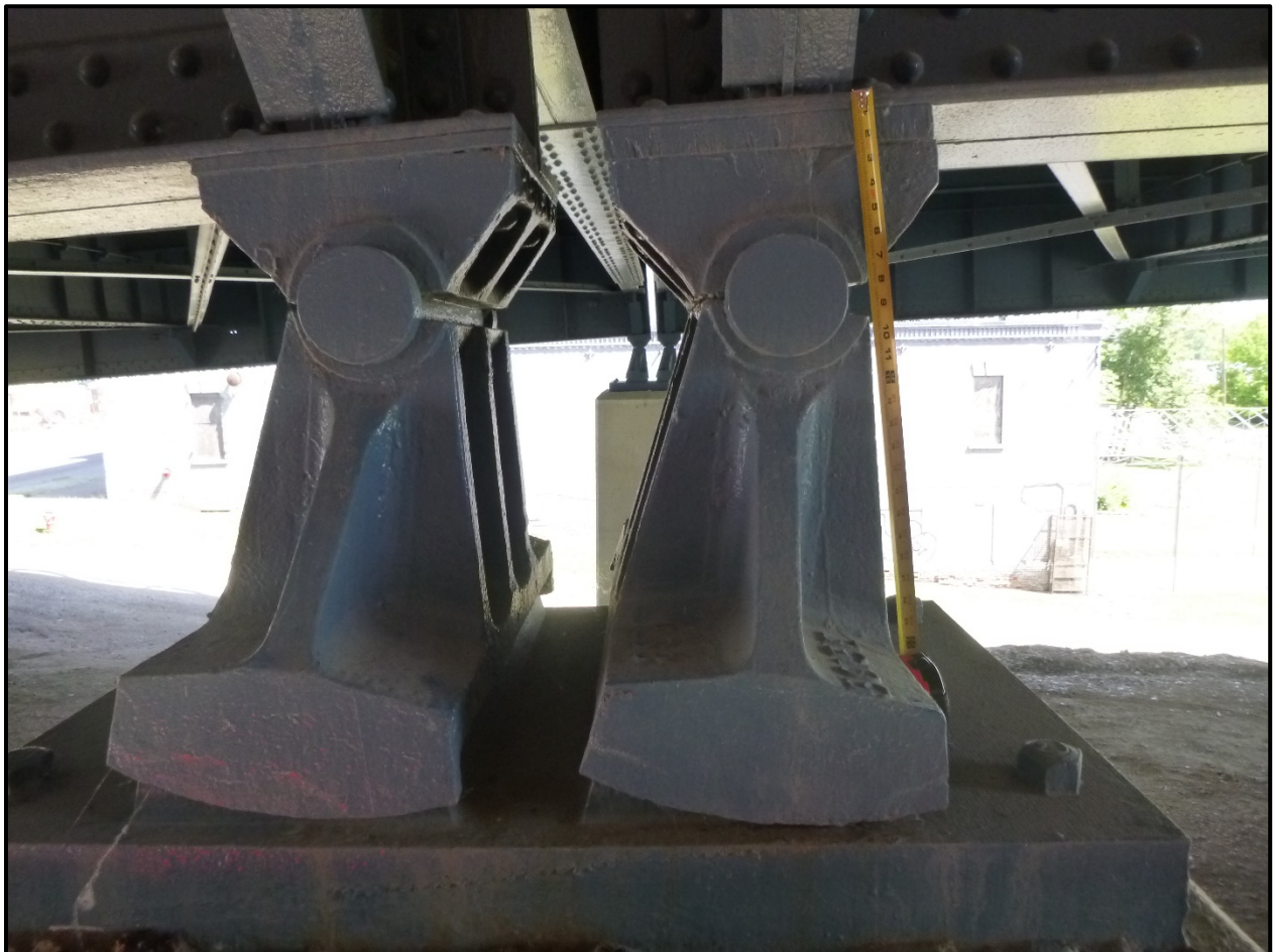
Photo 24 – Bearings below Span 6W Girders at Pier 6W are Tilted approximately 10 degrees East, Opposite of Temperature (RG shown, LG similar)
