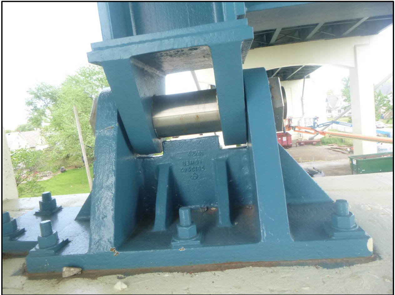
Photo 33 - Unpainted Bearing Pin at Pier E (South Bearing shown, North similar)
