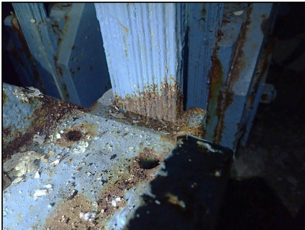
Photo 43 - Severe Corrosion of the Main Cable Wires just above the top of the Strand Shoe. Location - Northeast anchorage, east half of 2nd cable strand from West at 5th row of eyebar pairs.
