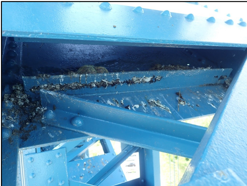
Photo 59 - Large Corrosion Hole in Stiffening Angle of Tower Bracing Batten Plate in Tower C Strut above Roadway
