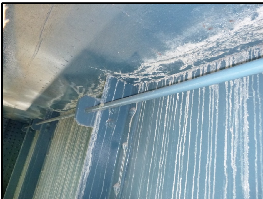
Photo 6 - Longitudinal Cracking & Efflorescence at Edge of Deck Underside (Typical, South Girder in Bay 15 shown)
