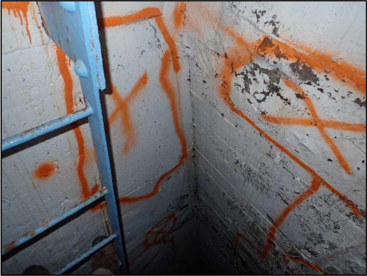
Photo 30 - Unsound Areas of Concrete Marked for Repair (Northeast Anchorage Chamber show, others similar)
