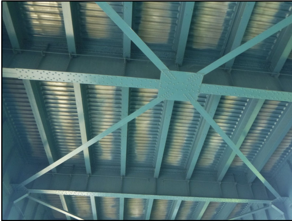
Photo 6 - Floor Beams in 2-Girder Approach Span
