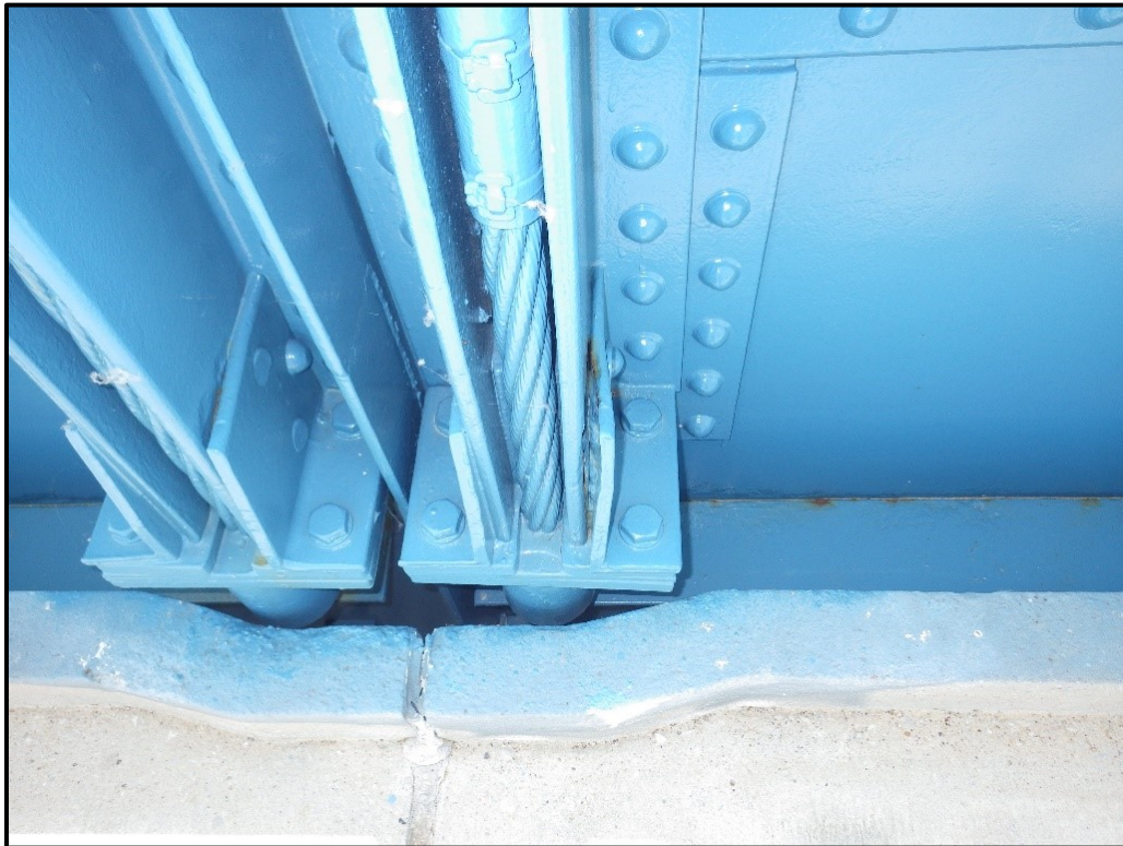
Photo 50 - Typical Suspender Rope at Stiffening Girder Socket Connection
