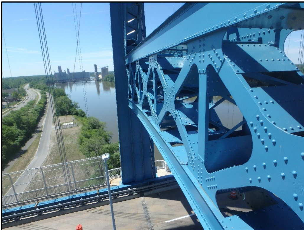
Photo 57 - Tower D Strut Above the Roadway. Note numerous repairs have been made to strut bracing members.
