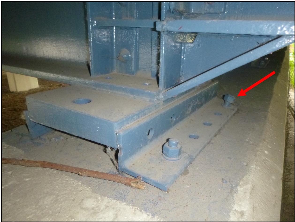
Photo 28 - Bent Anchor Rod and Loose Nut on Northeast Corner of S05 Bearing at Pier 12E
