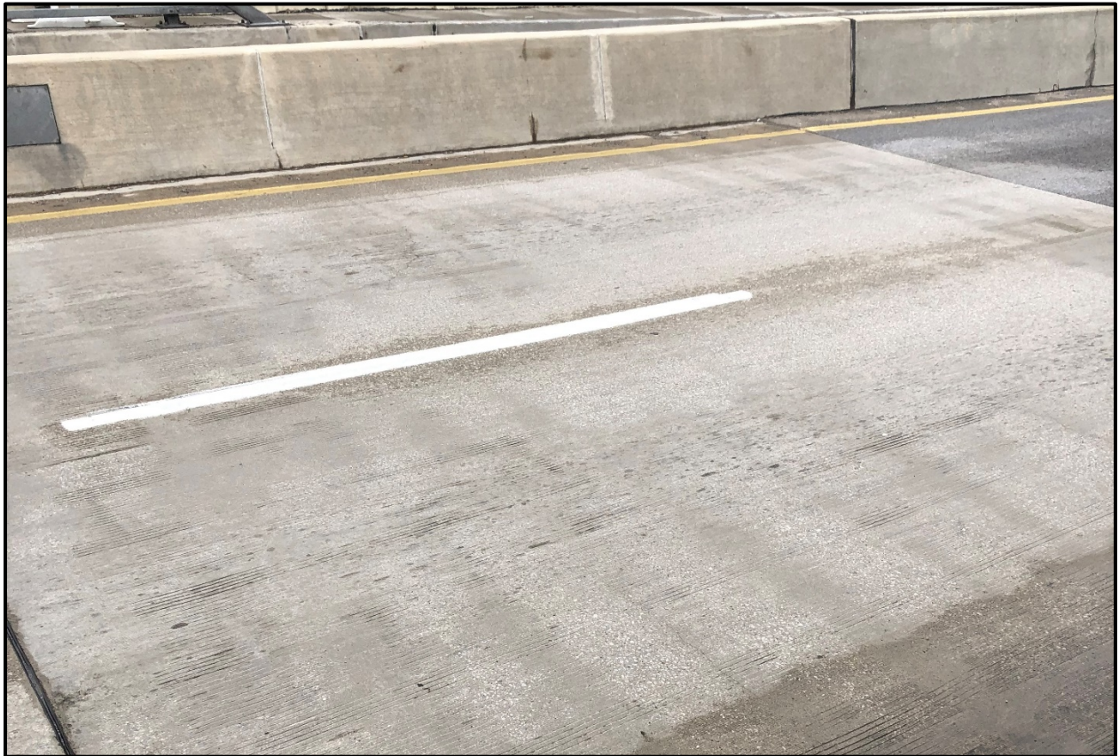
Photo 68 - Typical Approach Slab Condition (Eastbound, East Approach shown)
