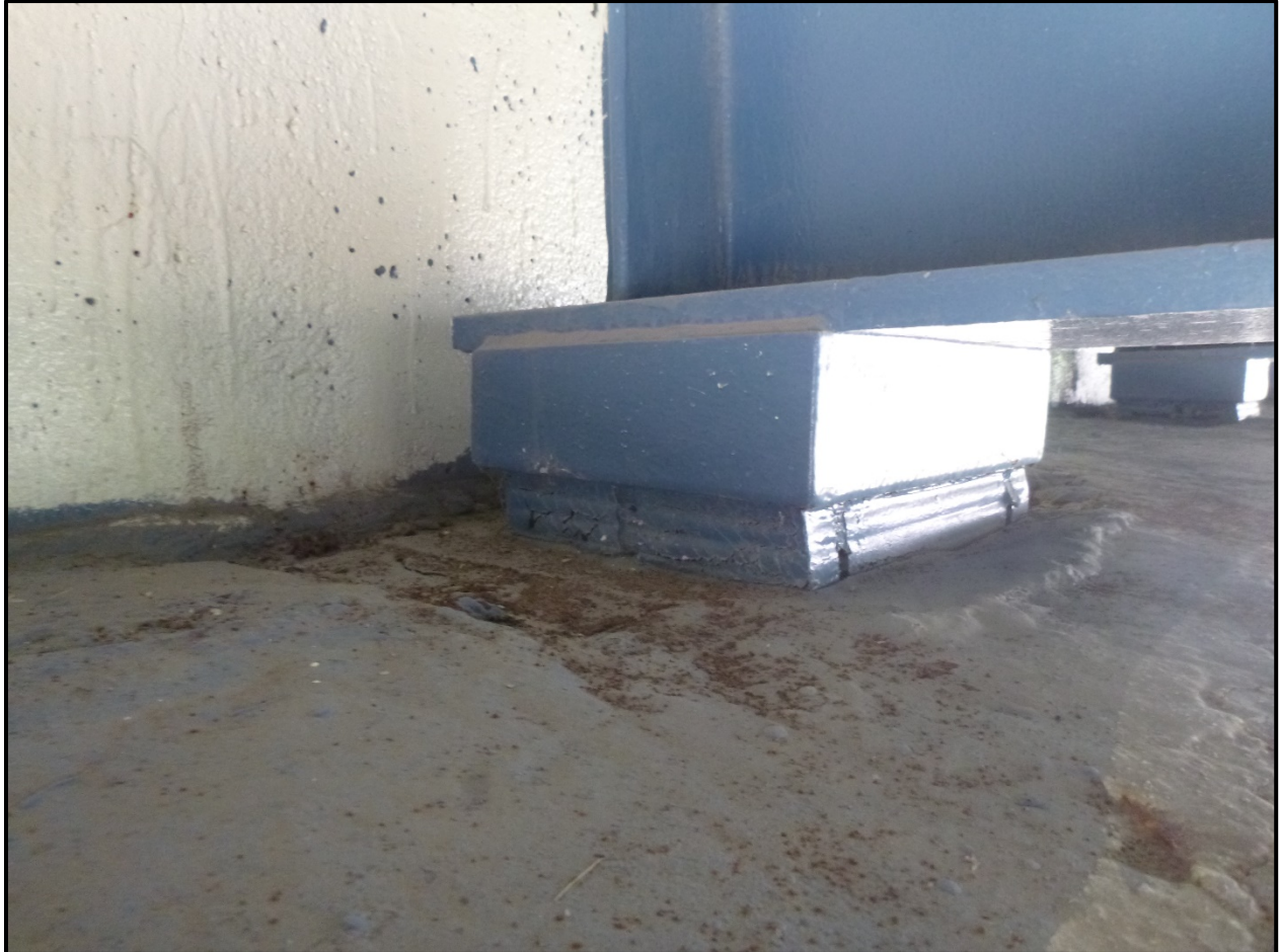
Photo 23 - 1/4" Bulge Rear Abutment Elastomeric (S08 shown, S03 & S09 similar)
