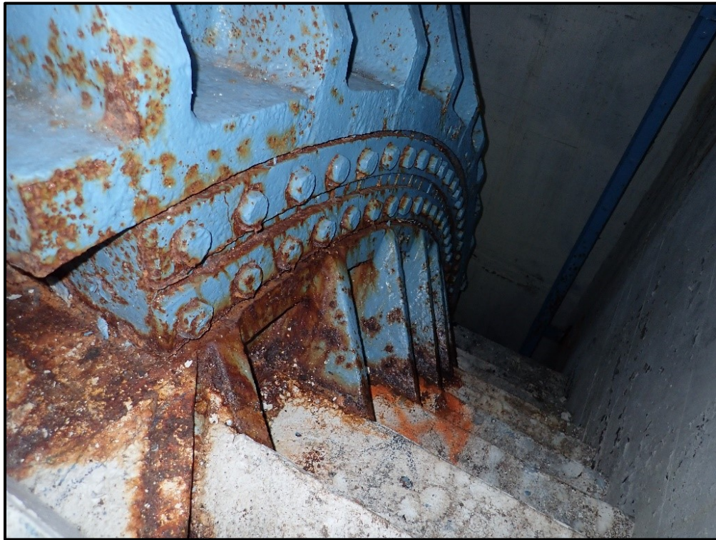
Photo 42 - Moderate to Severe Corrosion of the Splay Saddle Castings in the Northeast Anchorage
