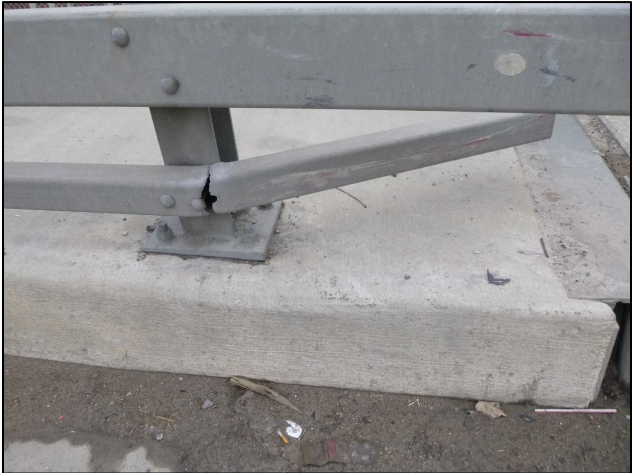
Photo 10 – 4 feet of Impact Damage to Guardrail at First Post on Southwest Corner of Bridge
