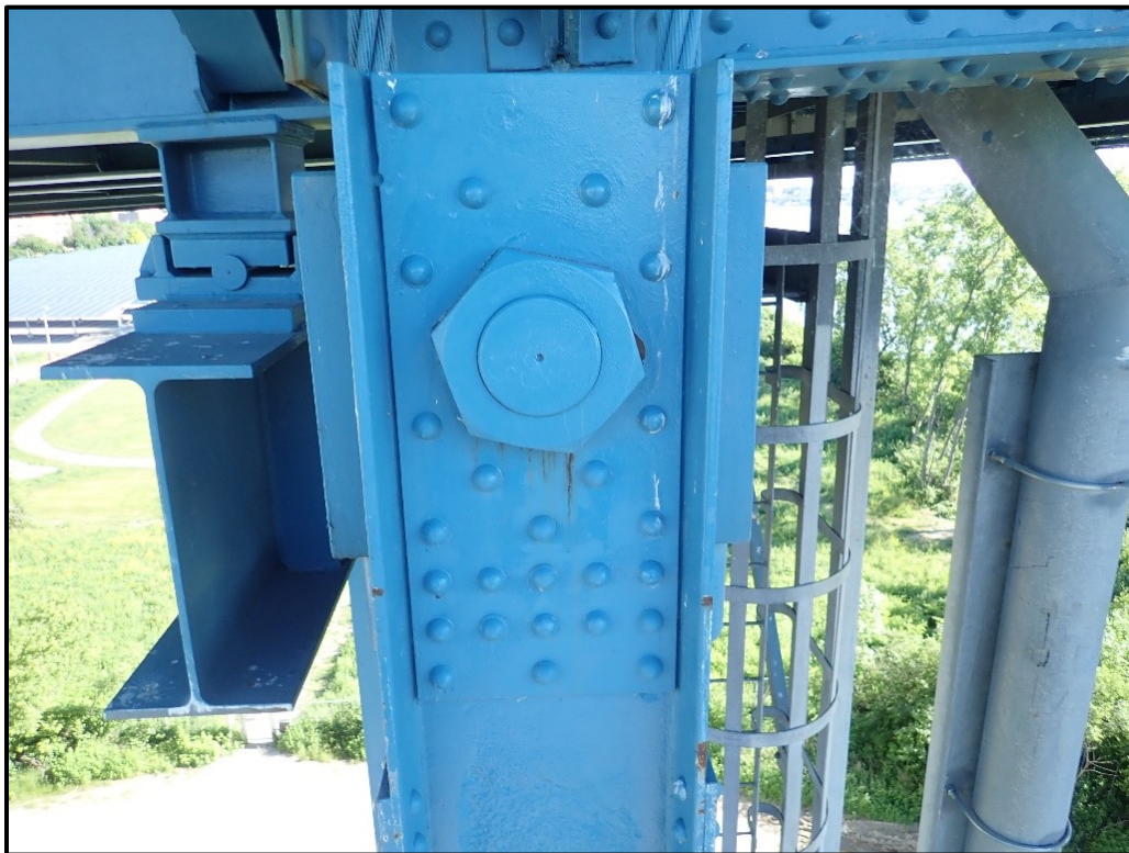
Photo 48 - Typical Connection for Hold-Down Suspender Ropes below Roadway. East Cable Bent, South Link Upper Pin shown
