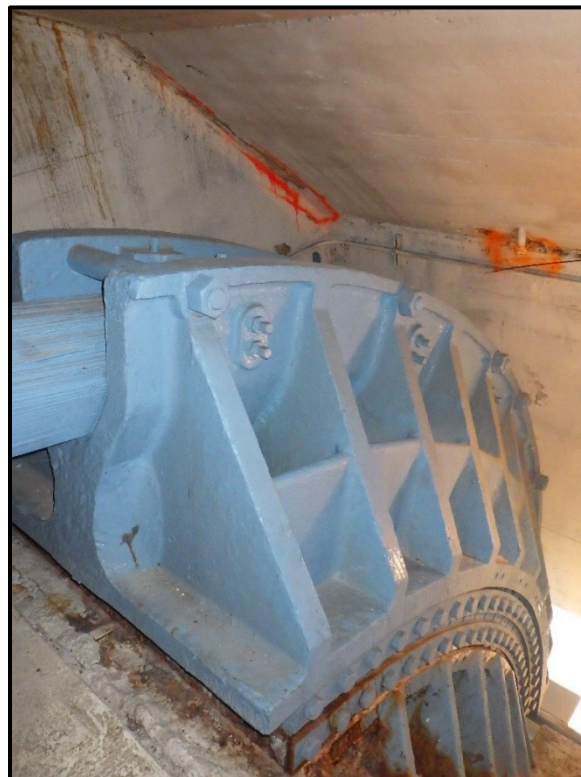
Photo 39 - Deviation Saddle Inside Northwest Anchorage Chamber. Note that the main cable enters the saddle at the left side of the picture.
