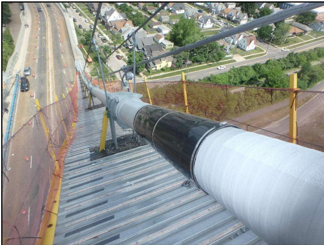
Photo 37 - South Main Cable in the East Side Span. Note that a portion of the cable wrap has been removed to accommodate the dehumidification collar and the area has been temporarily covered with a clamped rubber sheet.
