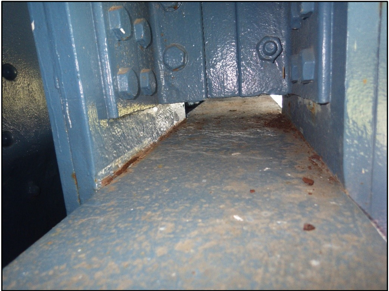
Photo 53 - Typical Hard Contact between Tower Link Plates and Tower Metalwork which Retains the Lower Pin
