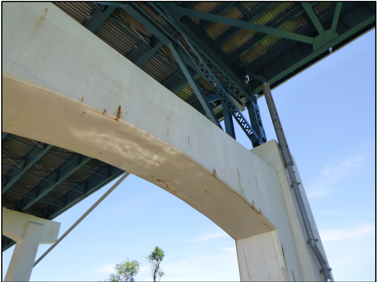
Photo 34 - Typical Sealed Cracks and Rust Staining of Pier Cap (Pier B shown)
