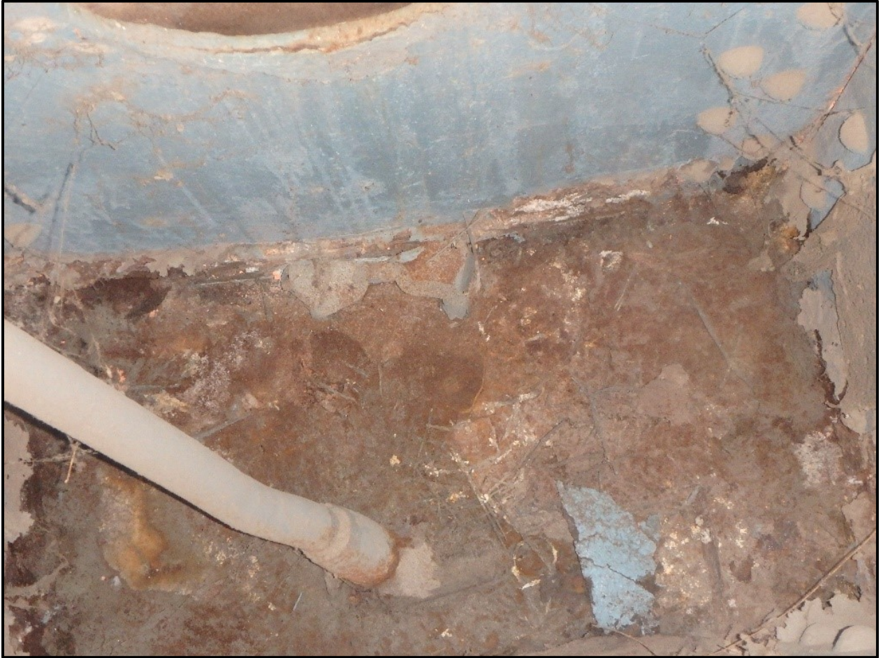
Photo 64 - Typical Minor Section Loss to the Lower 2" of Chamber Walls. Center Chamber at Base of Tower C shown.
