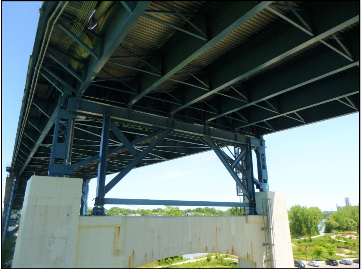
Photo 32 - Steel Frame Supporting Span RW-1 @ Pier B
