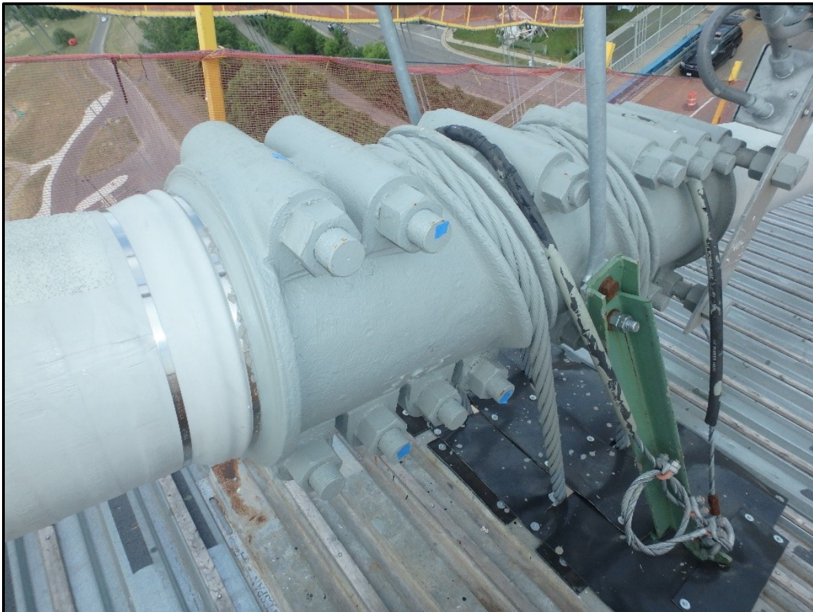
Photo 45 - Cable Band and Suspender Ropes of South Cable in East Side Span
