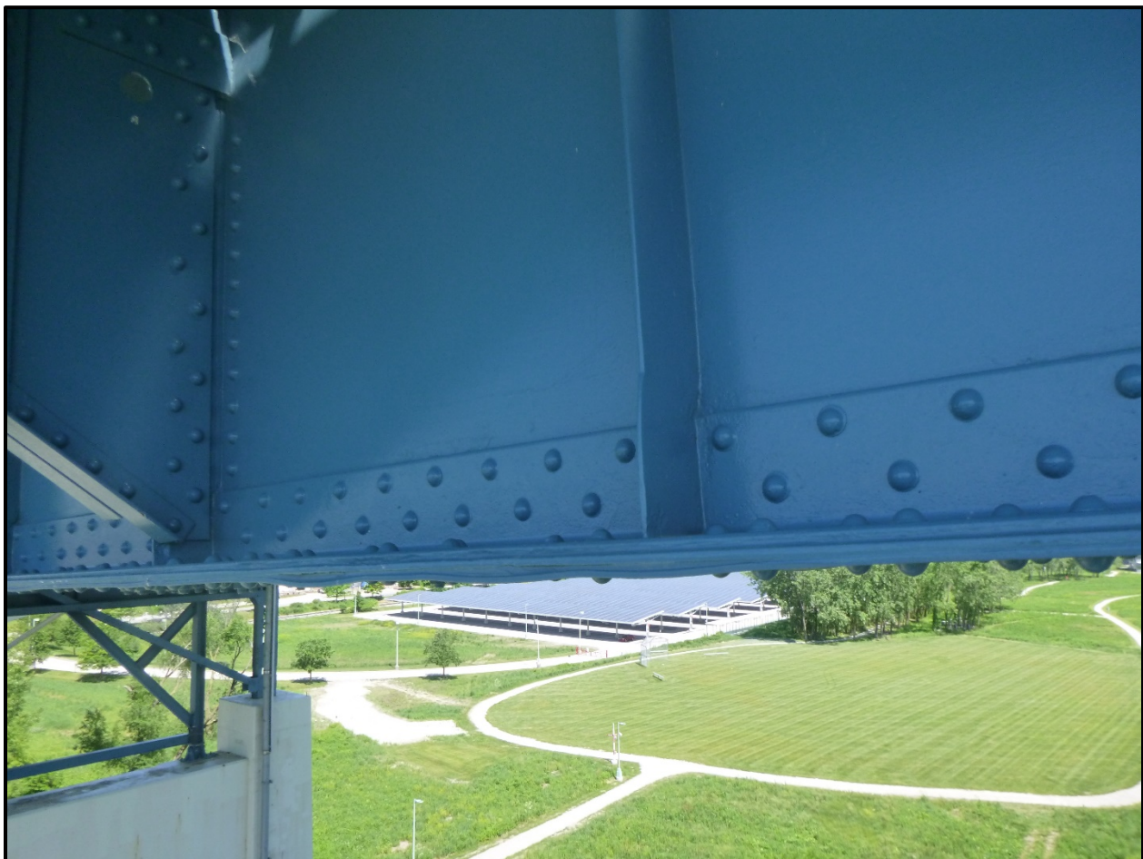
Photo 15 - Typical Pack Rust Induced Distortion of Suspension Span Girder Bottom Flange
