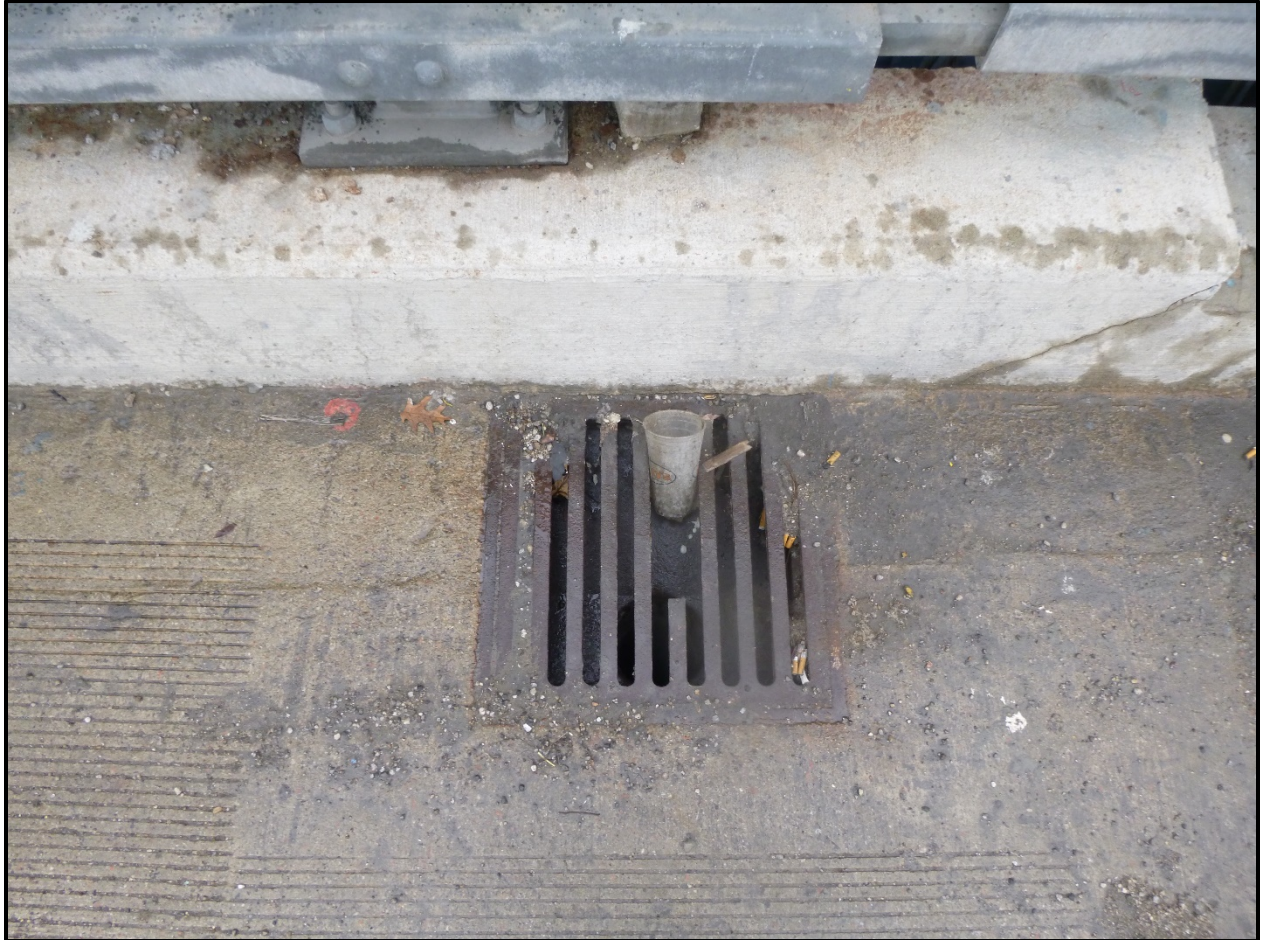
Photo 13 - Broken Deck Drainage Grate at South Curb near Pier B
