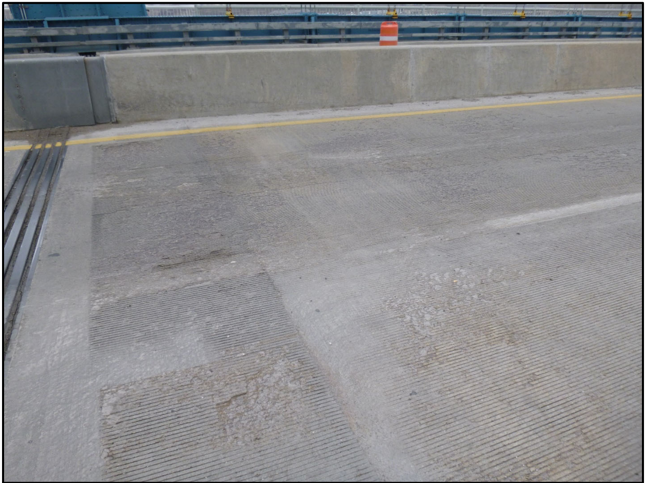
Photo 7 - Wearing Surface Abrasion
