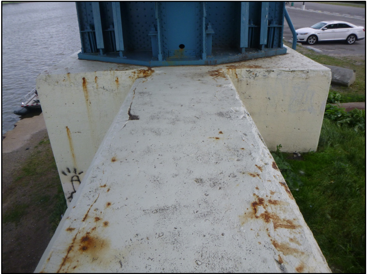
Photo 35 - Typical Condition of Partially Buried Cap Supporting Suspension Towers (Pier E shown)
