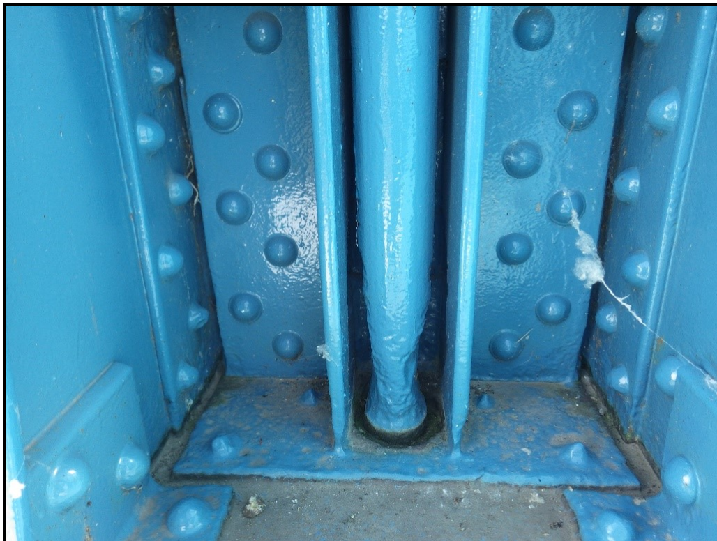
Photo 61 - Up to 40% Loss to the Anchor Bolt at the Northeast Corner of North Leg of Tower D
