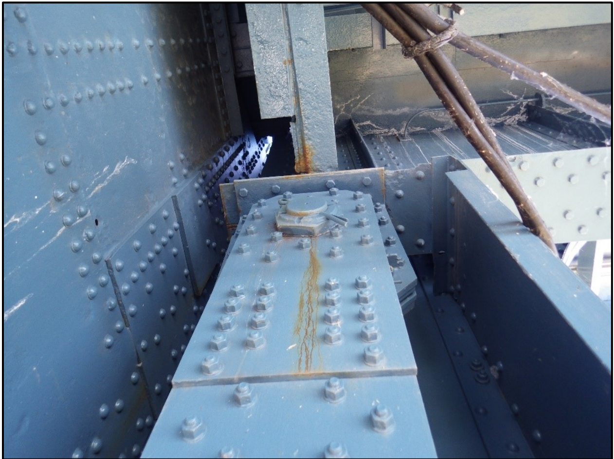
Photo 52 - Minor Corrosion Staining Emanating from the Tower D, South Leg, West Link, Top Pin
