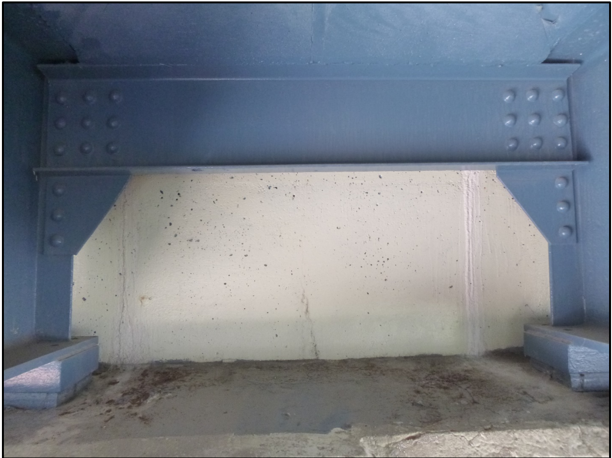
Photo 36 - 2' Wide Delamination between B5 & B6 at the Rear Abutment
