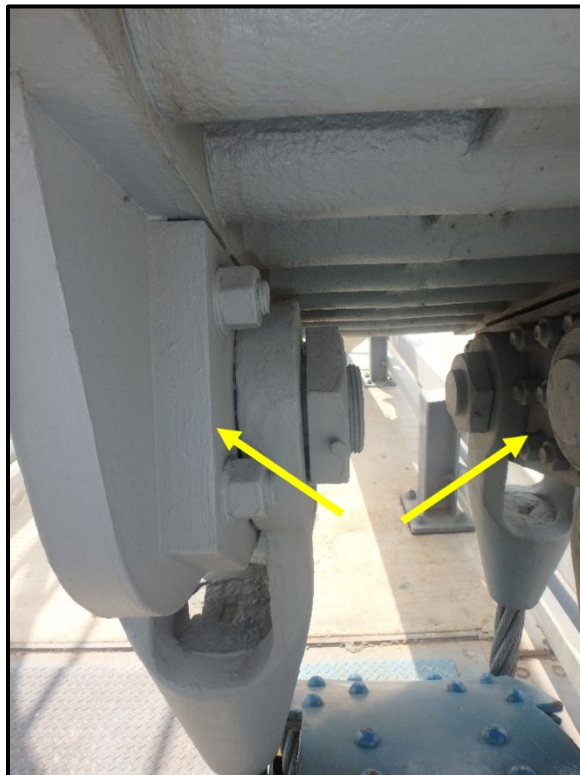
Photo 47 - West Hold-Down Ropes on South Cable. Note that the previously crack welded pin plates have been replaced with bolted plates.
