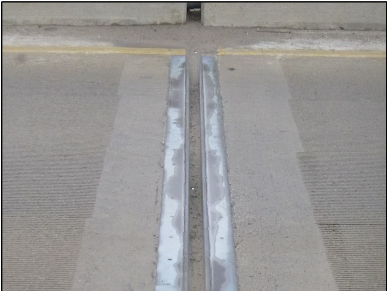
Photo 8 - Typical Strip Seal Expansion Joint Condition
