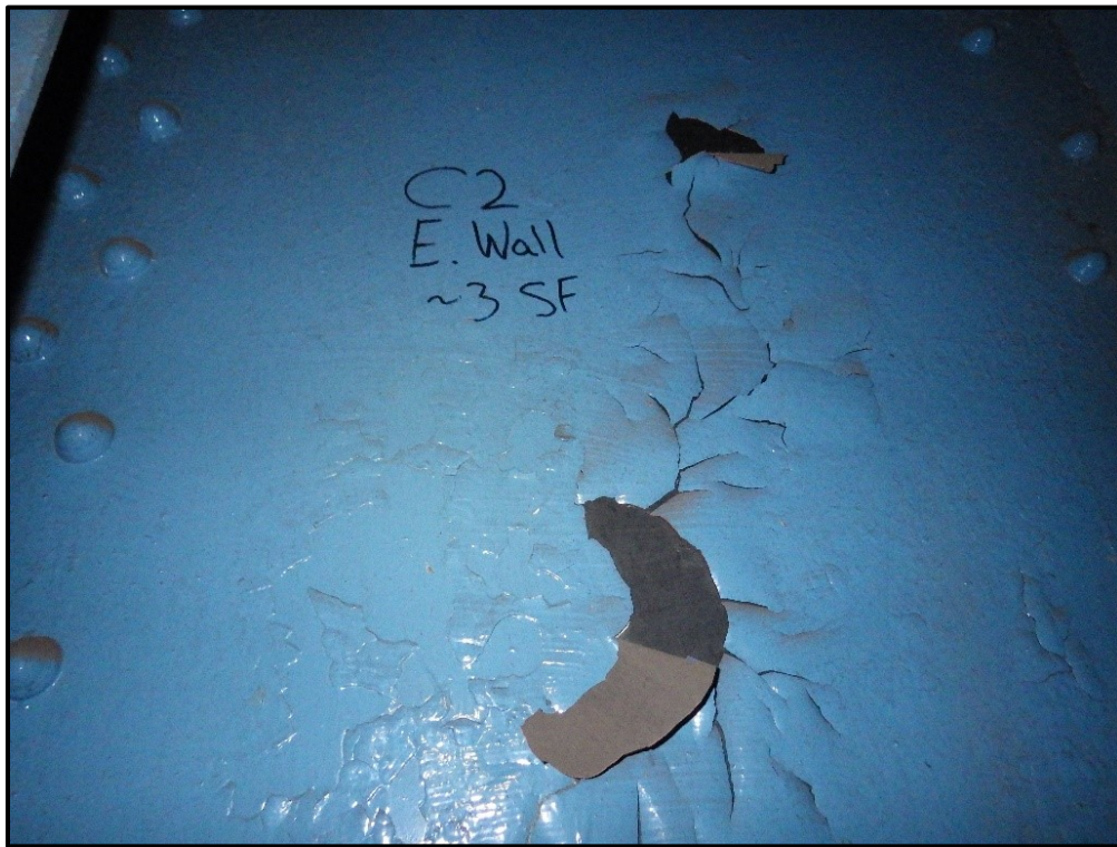
Photo 62 - Typical Paint Peeling in Tower Interior Chambers. Center Chamber at 2nd Cell above Roadway Level in South Leg of Tower C shown.
