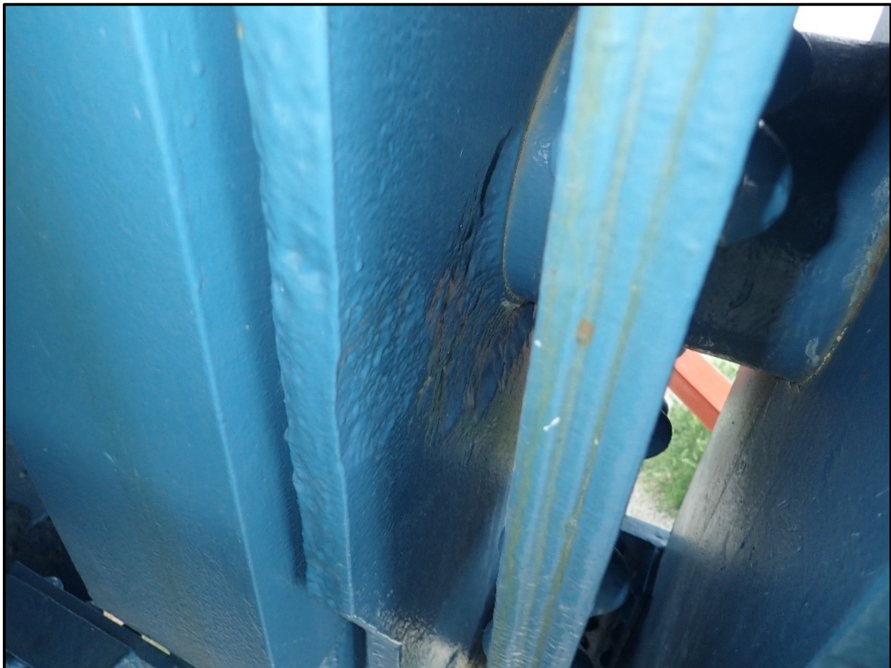
Photo 54 - 5/16" Pitting Section Loss in the East Cable Bent, North Column, Outboard Face of the Inboard Link Plate at the Top Pin
