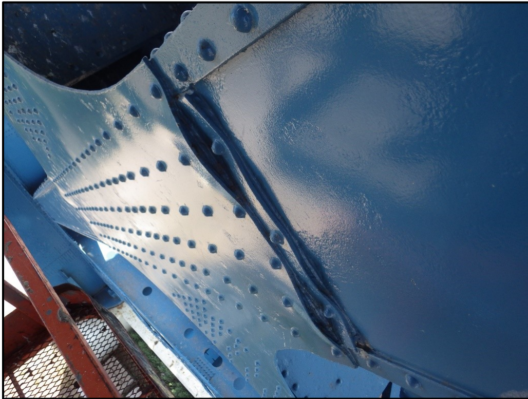
Photo 60 - The Center Gusset Plate below Roadway Level in Tower D Bracing has up to 1.5" Pack Rust Distortion between Gusset and Fill Plates
