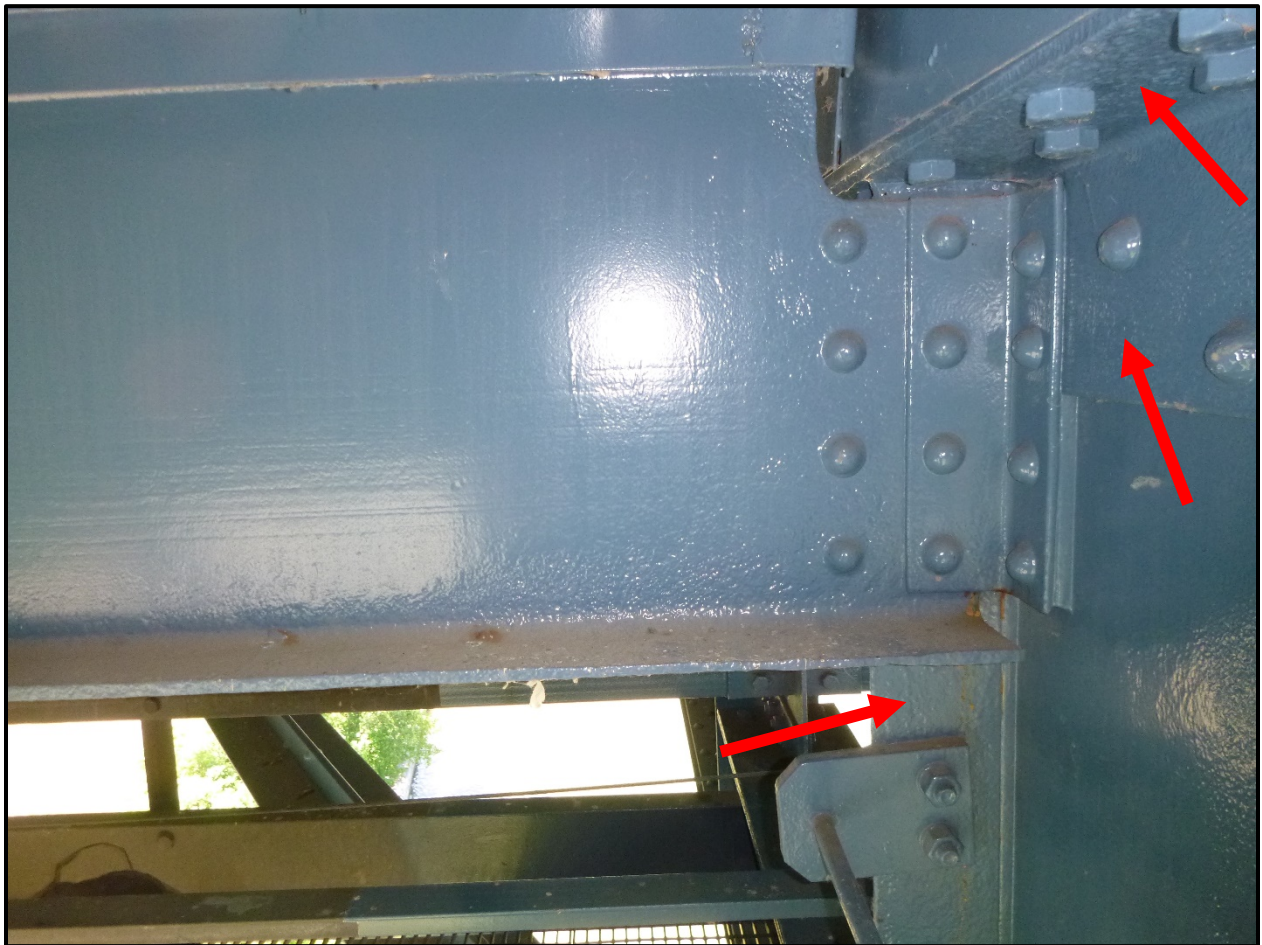
Photo 20 - Floor Beam Top Flange Section Loss
