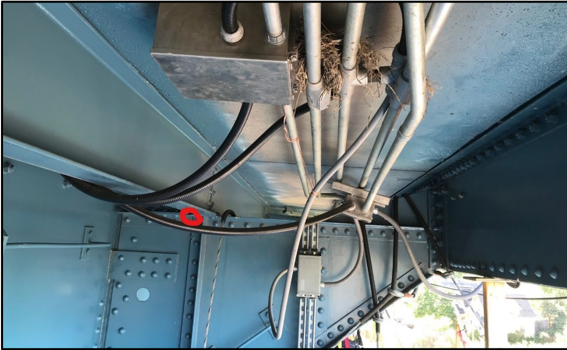
Photo 21 - Location of Cracks in Floor Beam Cantilever Top Flange
