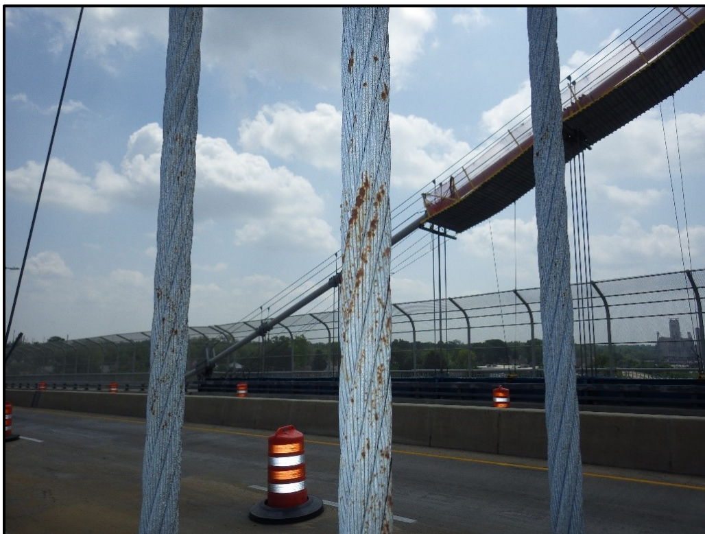
Photo 49 - Typical Suspender Ropes with Areas of Moderate Corrosion near the Roadway Level
