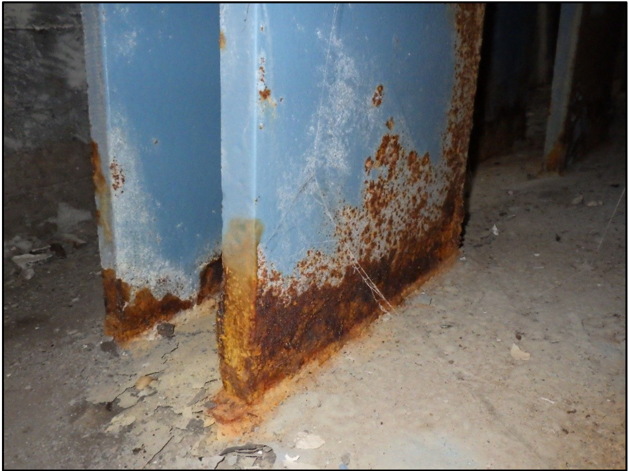
Photo 44 - Typical Corrosion and Section Loss at the Base of the Eyebars, Southeast Anchorage Chamber at Southwest Eyebars Pair Shown
