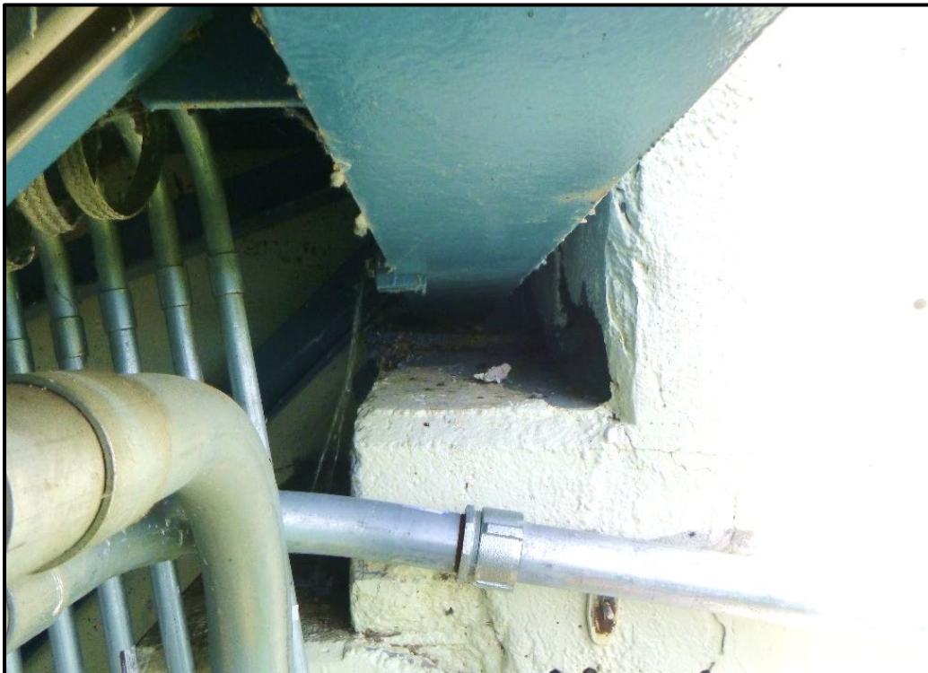
Photo 26 - S1 Bearing Plate at Anchorage A Overhangs Beam Seat by 1/2"
