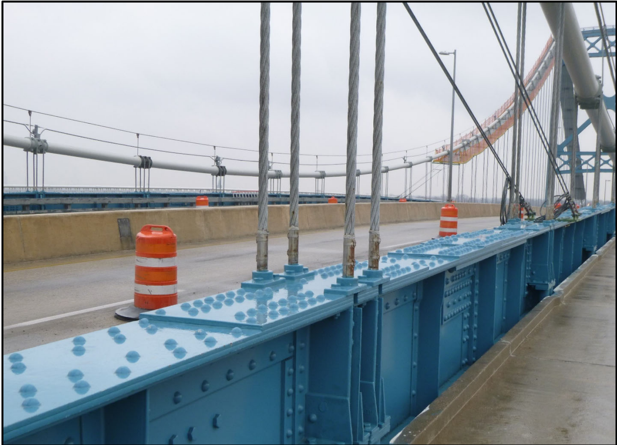
Photo 3 - Hanger Cable - Suspension Girder Connection
