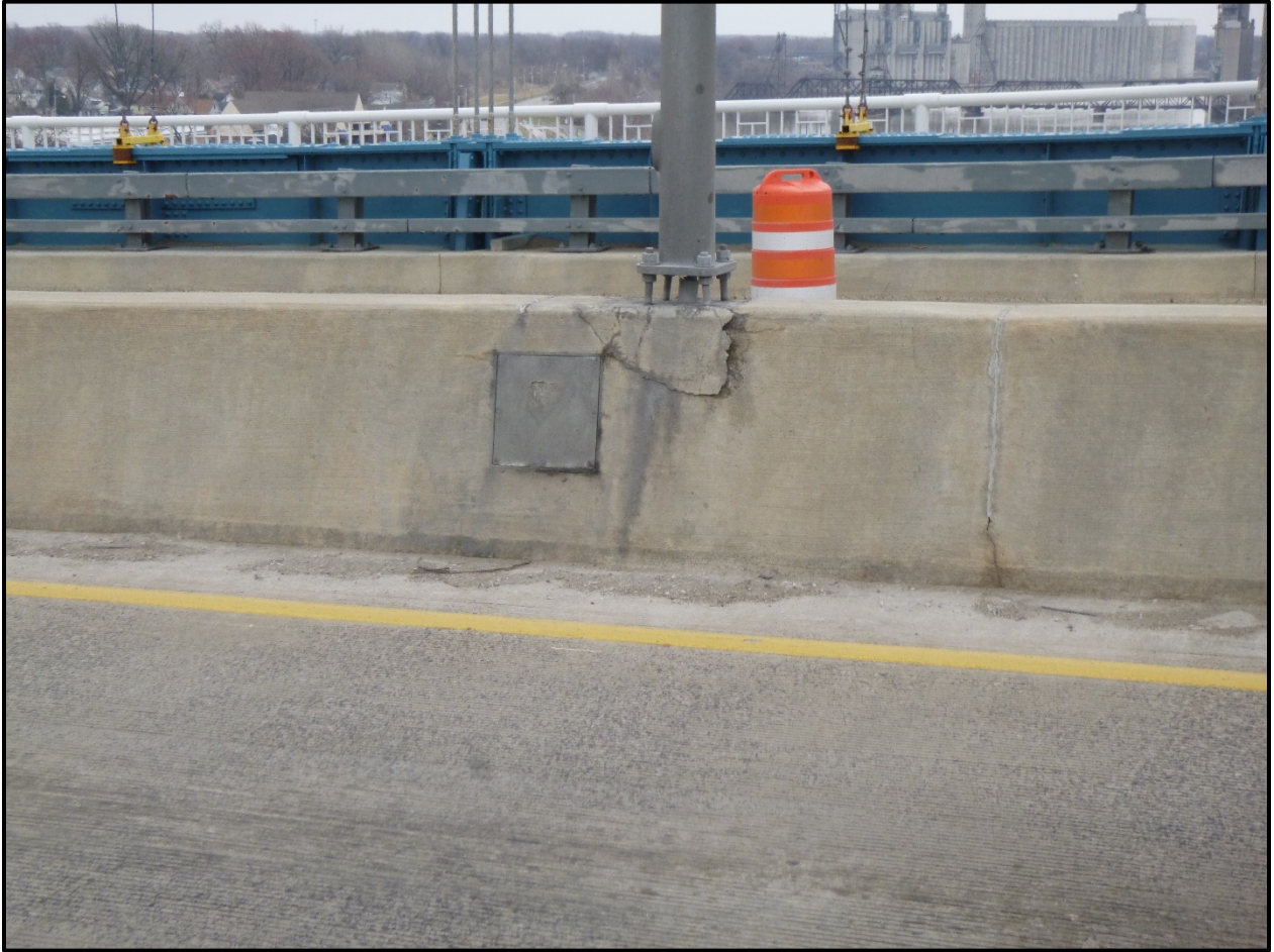
Photo 12 - Delamination and Spalling at Light Pole Adjacent to Tower D
