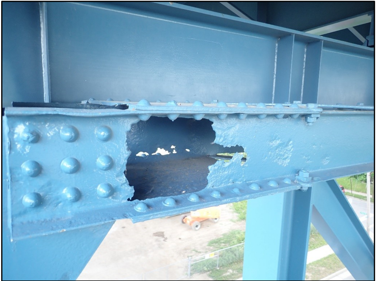
Photo 55 - Large Corrosion Hole in the West Web of the East Cable Bent Upper Strut near the North Link Column. Note corrosion holes are also present in the east web of the strut
