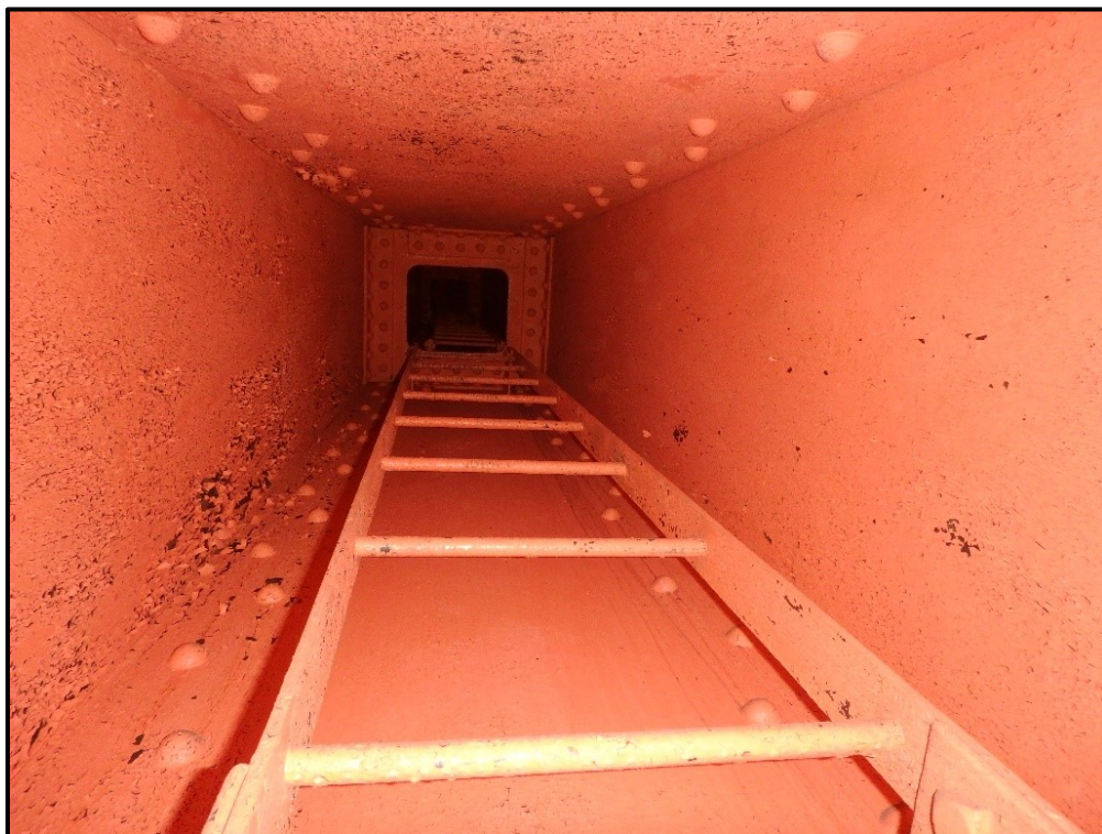
Photo 63 - Typical Brittle and Peeling Orange Primer Paint in Tower Side Chambers. West Chamber at 7th Cell above Roadway Level in South Leg of Tower C shown.
