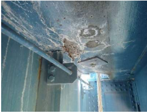
Photo ES-025: Spall on underside of deck, at Left Girder and FB64, looking northeast
