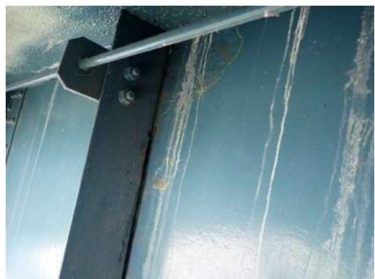
Photo MS-081: Pitting (3/16" deep by 6" high) to the web of Right Girder near top flange, north face, east of FB47, looking southeast
