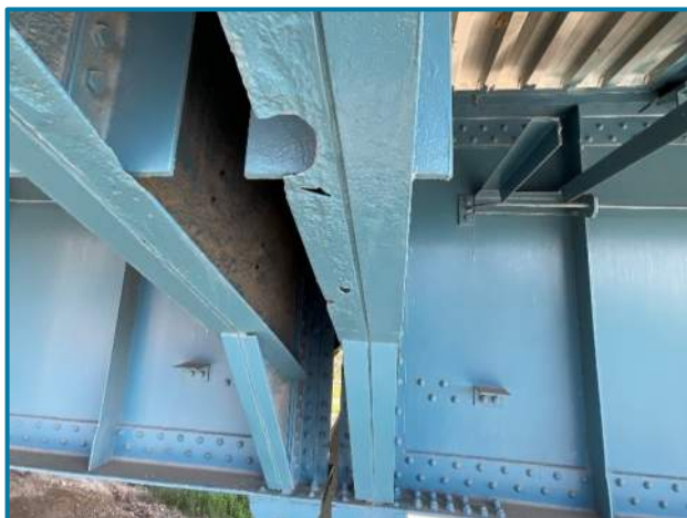
Photo 30 – Areas of 100% section loss to Floorbeam 0 bottom flange in Span 5W at south cantilever floorbeam bracket (looking north).
