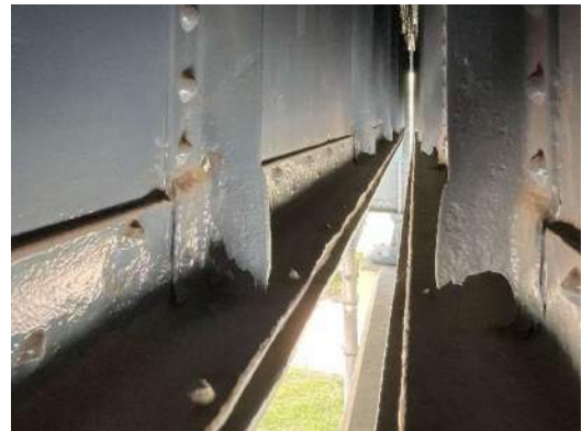
Photo 2E-006: 100% section loss in transverse stiffeners on east face of FB4
