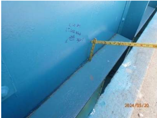
Photo ES-019: Pack rust (3/8" thick) and pitting (1/8" deep) on north face of Left Girder, between FB62 and FB63, looking southwest
