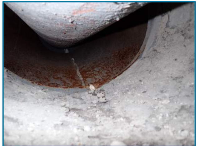
Photo 52 – Surface corrosion of North Cable sleeve at entrance into Anchorage F (looking west).
