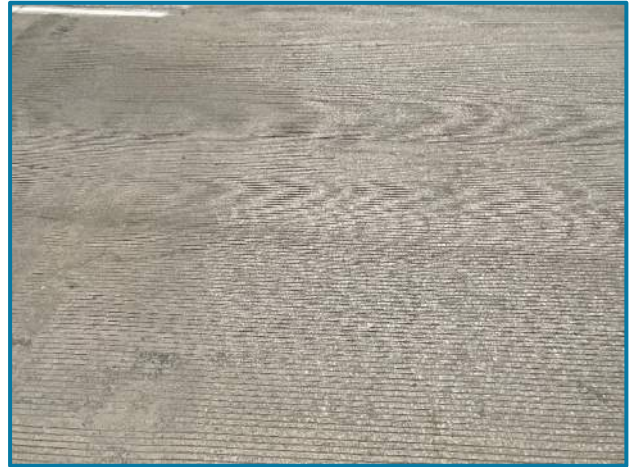
Photo 88 – Typical widespread map cracking in the Rear Approach Slab, westbound lanes (looking south).
