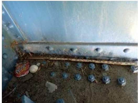
Photo MS-071: Pitting (up to 1/4" deep by full height) on vertical leg of bottom flange on north face of Right Girder at west face of FB43, looking south
