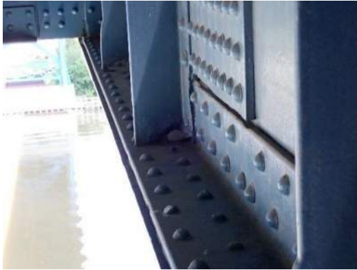
Photo MS-084: 100% section loss (up to 2.5" high by full width) on transverse stiffeners on Left Girder between FB48 and FB49, looking west
