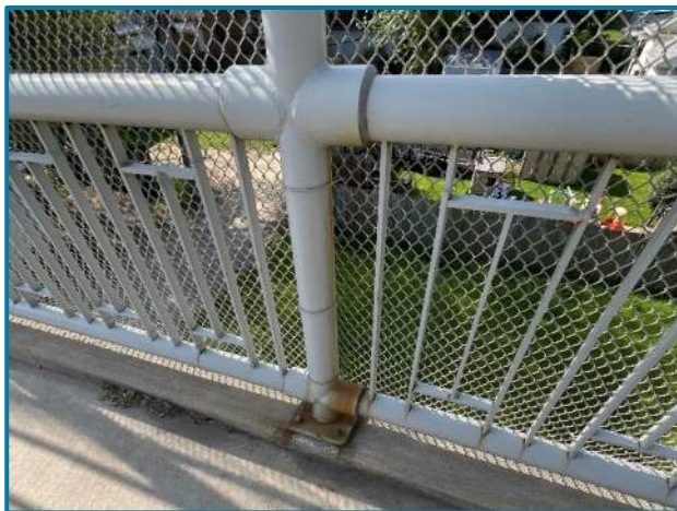
Photo 20 – Typical condition of the sidewalk railing in Span 12E at the south sidewalk (looking south).
