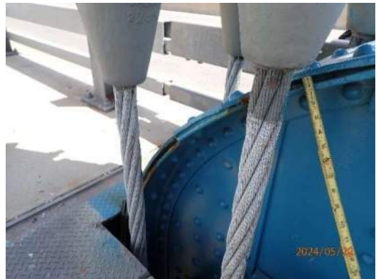
Photo ES-028: Pack rust (5/8" thick) between built up top flange plates at Left Girder and cable 65 anchorage, north face, looking southeast
