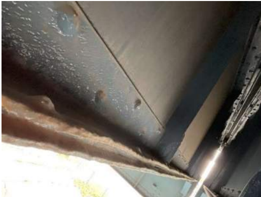
Photo 5E-003: Painted section loss on top and bottom flange of FB0 west face and bottom 4" of stiffeners, pack rust between bottom flange plates with wavy action, between S1 and S7
