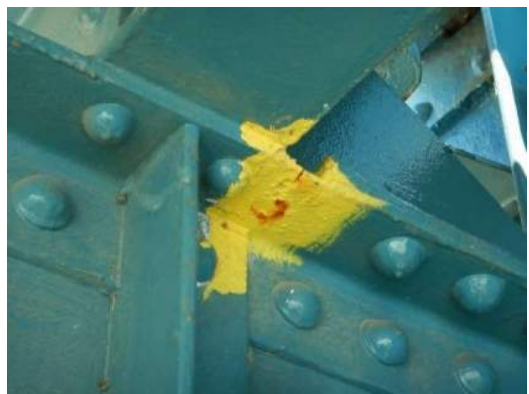
Photo WS-012: Top flange cracked on east side of FB10 south cantilever between Right Girder and RS1, looking northwest
