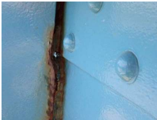
Photo WS-003: Kneebrace with 3/4" thick pack rust and up to 100% section loss on Left Girder south face at FB0, looking northwest
