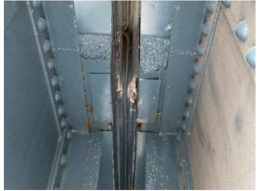
Photo 5E-014: Active corrosion to top flange of FB4 south overhang and deck pan flashing, with efflorescence, between RS1 and RS2
