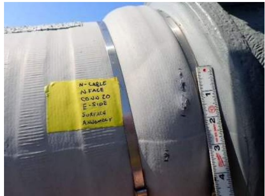
Photo NC-004: Main cable at suspender cable 20, surface defect, left and right side of connection, north face
