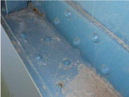
Photo MS-066: Up to 90% section loss on rivet heads on top of south face bottom flange of Left Girder between FB42 and FB43, looking northwest
