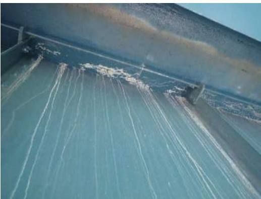
Photo ES-011: Efflorescence staining on Left Girder web, between FB58 and FB59
