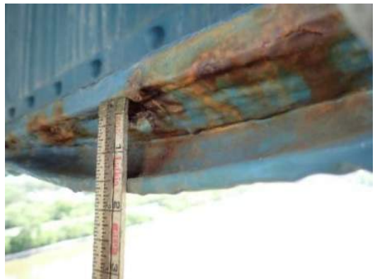
Photo MS-036: Pack rust (1 1/2" thick) between bottom flange plates with minor reactivated corrosion on north edge of Right Girder, east of FB30, looking southwest
