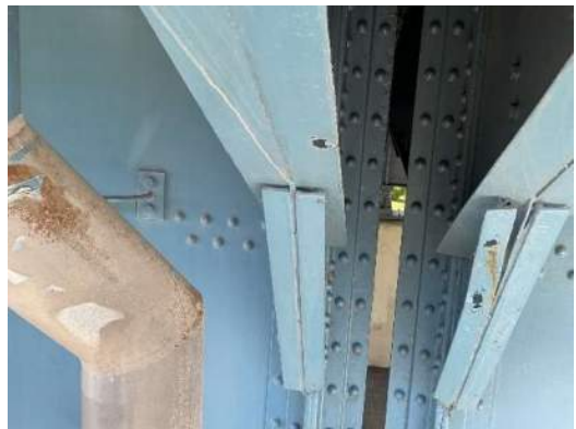
Photo 6E-012: 100% section loss in bottom flange of FB4 south overhang, near Right Girder, looking north
