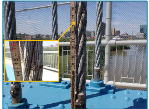
Photo 56 – Minor surface corrosion on North Suspender Cable 10 in the splash zone (looking northwest).
