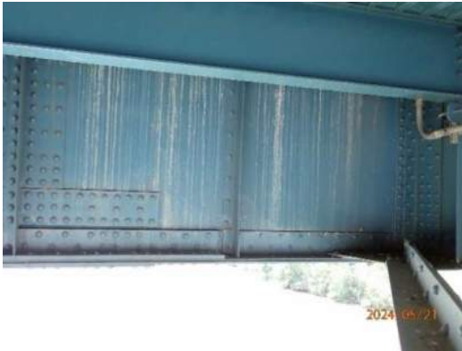
Photo MS-044: Pitting and efflorescence staining on north face web of Right Girder, between FB33 and FB34, looking south
