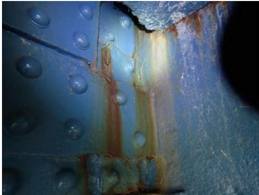
Photo MS-086: Pack rust (3/4" between FB49 plates on west face, with 1/16" deep pitting, looking east
