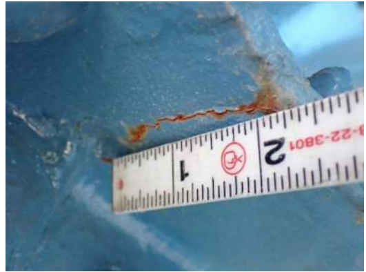
Photo MS-091: Crack (1 3/4" long) with light rust staining in top flange of north sidewalk cantilever on FB51
