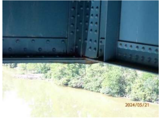
Photo MS-055: Pack rust (1" thick) between bottom flange plates on north face of Right Girder at FB36, looking south
