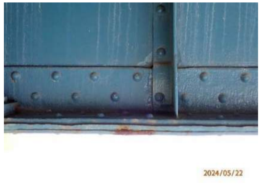
Photo MS-016: Pack rust between bottom flange plates of Left Girder south face between FB18 and FB19, looking north
