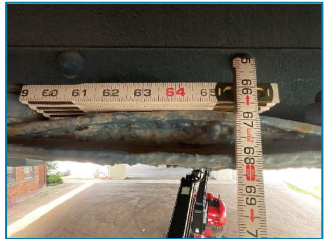
Photo 33 – Pack rust up to 1" thick along FB3 bottom flange in Span 7W at midspan (looking west).
