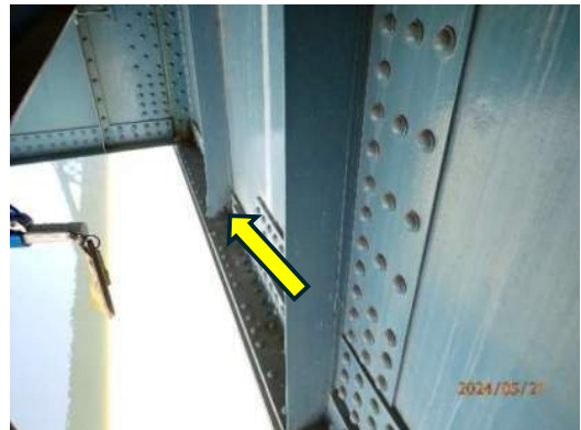
Photo MS-051: 100% section loss (4.5" high by full width) on transverse stiffener on north face of Right Girder, between FB35 and FB36, looking southeast
