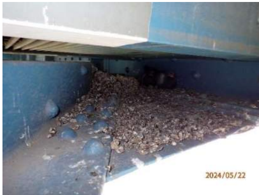
Photo MS-021: Typical granular and bird debris on lateral bracing connection plate, west side of FB25, between S6 and S7, looking east
