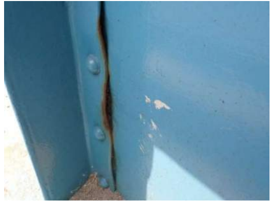
Photo ES-026: Pack rust (18" high by 1/2" thick) and pitting (8" high by 1/8" deep) between transverse stiffener and Left Girder web, between FB64 and FB65, looking northwest
