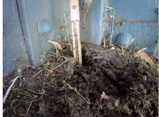
Photo MS-057: Typical granular and bird debris (4" high) on lower lateral brace connection plate to Left Girder, at FB37, looking north
