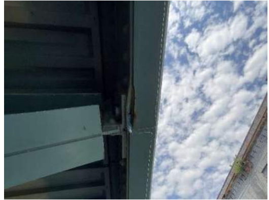
Photo 6W-002: Pack rust between bottom angle/web of stringer LS2 at FB1, looking west
