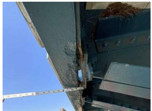
Photo 5W-004: 100% section loss on bottom flange angle of RS2 at FB0, with pack rust causing gap between stringer web and bottom flange
