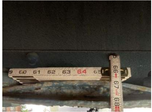
Photo 7W-008: Pack rust along the east face bottom flange of FB3 in multiple locations between S1 and S4, looking west
