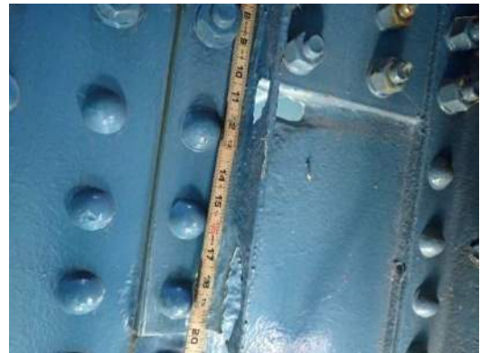
Photo MS-093: 100% section loss on outstanding leg of FB50 kneebrace, east face at Right Girder, looking northwest
