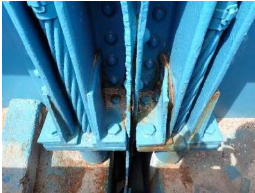
Photo ES-021: Pack rust between vertical cable plates and anchorage horizontal bearing plate at top of vertical legs of connection angle, at Left Girder south face, at FB63, looking north
