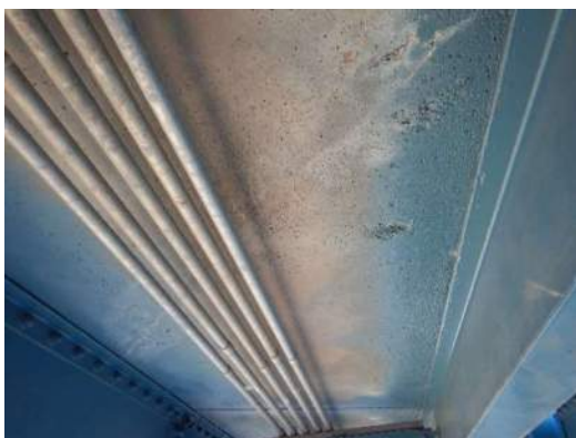
Photo MS-088: Hairline cracks between RS1 and RS2 and FB49 and FB50, with light efflorescence
