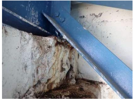
Photo RW-2-002: Beginning of undermining with slight section loss of bearing area (2' wide by 2' high by 2" deep) at anchorage A S2 bearing, looking southwest
