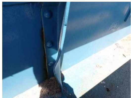
Photo WS-006: 2 1/4" impact damage to transverse stiffener outstanding leg on Left Girder south face east of FB1, looking north
