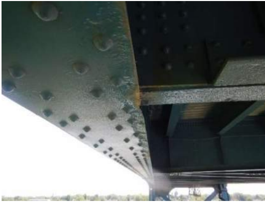
Photo WS-007: Section loss (20' long by 2" wide by 3/16" deep) on bottom flange of Left Girder near FB2, looking northeast
