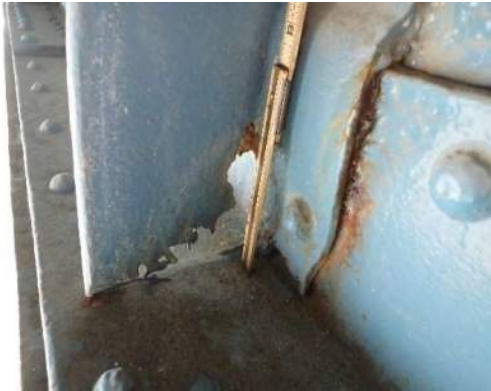
Photo MS-092: 100% section loss (up to 3" high by full width) in transverse stiffener on Left Girder near FB51, looking west
