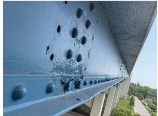
Photo 6W-004: Pack rust causing separation of bottom flange angle to web, with painted over 100% section loss, at FB2 south overhang, at RS2, looking east
