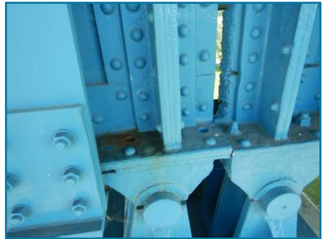
Photo 43 – 4 of 8 missing connectors at Left Girder rocker bearing sole plate, Pier 2W (looking south).
