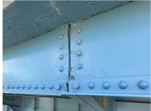
Photo 2E-002: Pack rust and painted over section loss of LS2 at FB2 overhang, looking southeast
