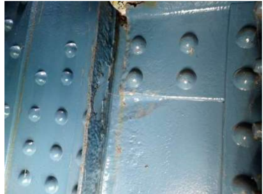
Photo MS-087: 100% section loss on outstanding leg of FB49 kneebrace, east face at Right Girder, looking southwest
