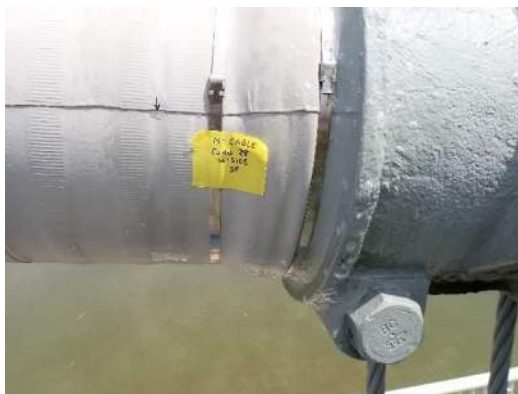
Photo NC-005: Main cable at suspender cable 28, two leaks, west end, south face
