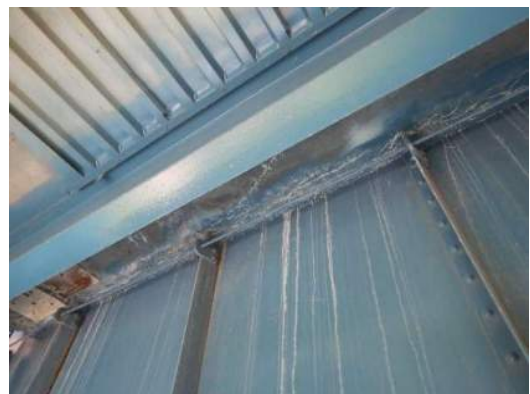
Photo WS-004: Typical efflorescence staining on Left Girder web, between FB0 and FB1
