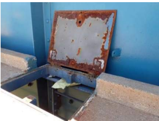
Photo MS-041: Broken hold down bolt in access hatch on LS1 between FB22 and FB23
