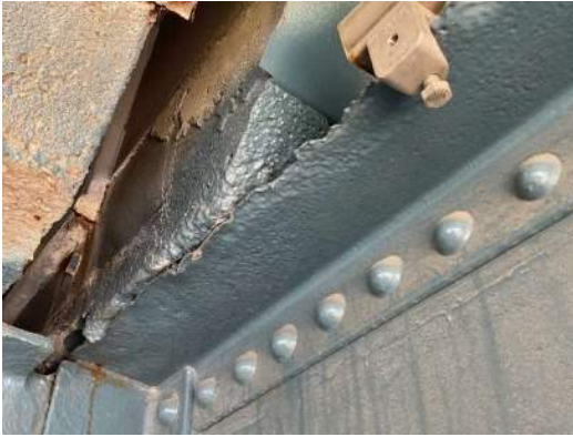
Photo 7W-001: Painted over 100% section loss on top flange of FB0 north overhang at LS2
