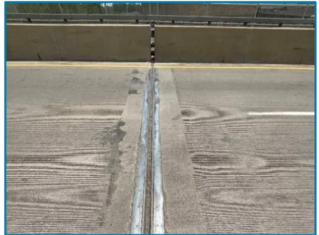
Photo 6 – Debris accumulation and minor header popouts at Pier 3W, westbound lanes (looking south).
