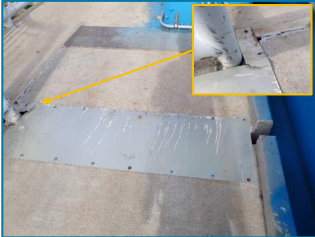
Photo 18 – Aluminum plate covering 5" gap between sidewalk panels with a 4 1/2" long tear at the railing post on the south sidewalk, east of Tower C (looking west).
