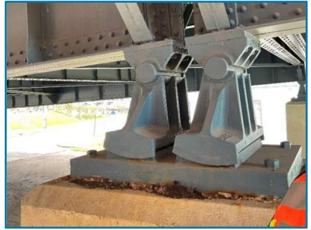
Photo 42 – Right Girder rocker bearing tilted up to 10° to the east at Pier 6W (looking northwest).
