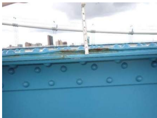
Photo MS-030: Pack rust (up to 3/4") between cover plate and top flange of Right Girder, between FB28 and FB29, looking north
