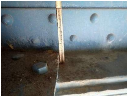
Photo MS-052: Pack rust (1" thick) between lower lateral brace connection plate and Left Girder, near FB35, looking north
