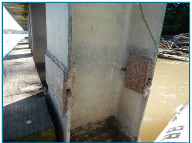
Photo 84 – Poor quality at northernmost pile at Tower C pier protection (looking south).
