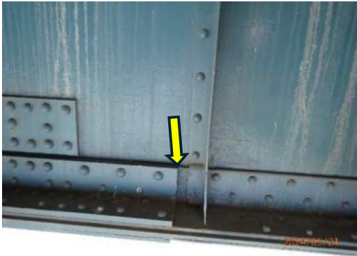
Photo MS-056: Pitting (3/8" deep by 2" wide by 8" high) on north face bottom flange of Right Girder, between FB37 and FB38, looking south
