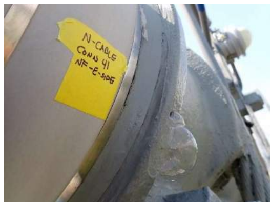
Photo NC-006: Main cable at suspender cable 41, connection leakage, east end, north face
