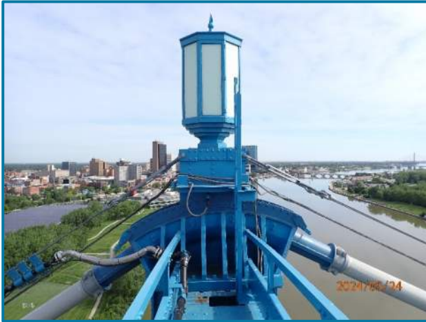
Photo 49 – North Cable saddle at Tower C (looking north).
