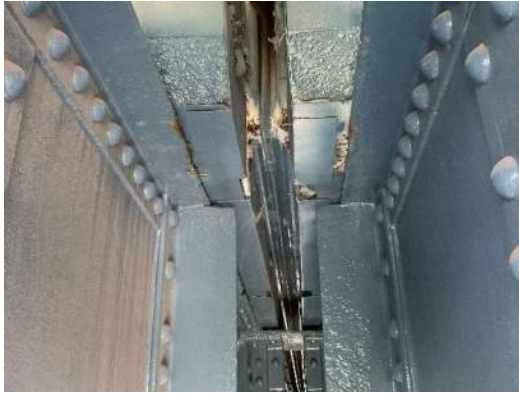
Photo 6E-001: Active corrosion and efflorescence through joint on east face FB0, with painted over section loss on top and bottom flange of FB0, north overhang
