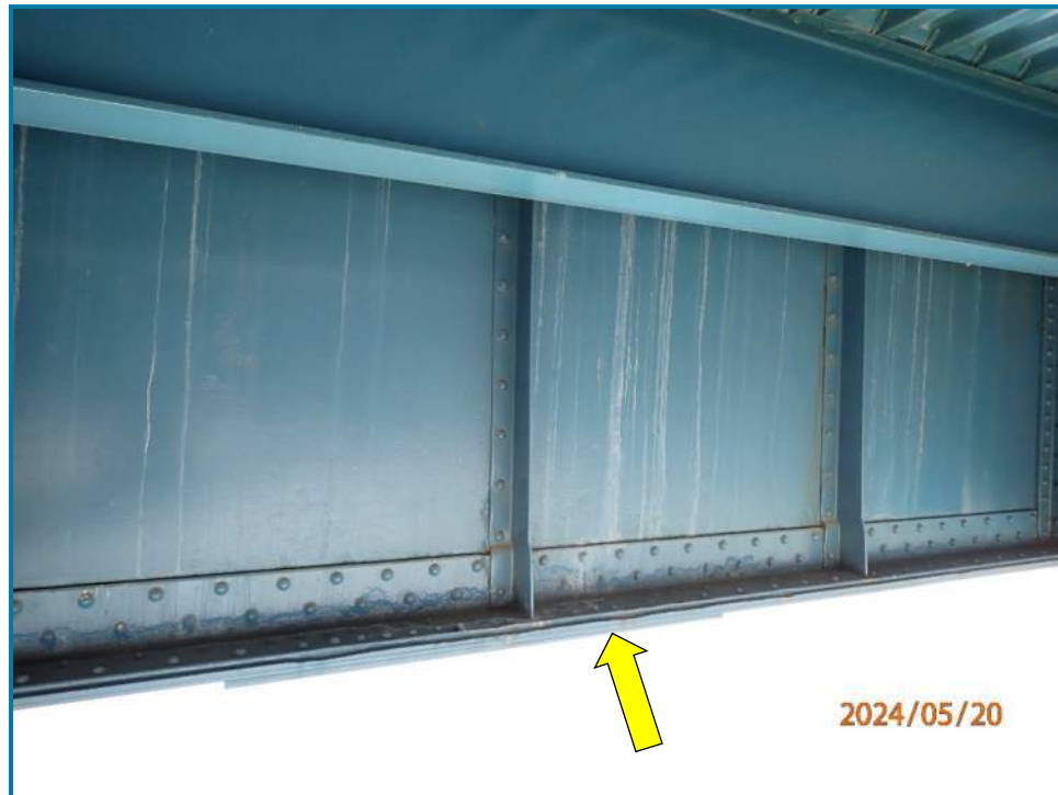
Photo 4 – Typical built-up girder shown in the Main Suspension Span (other spans similar)
