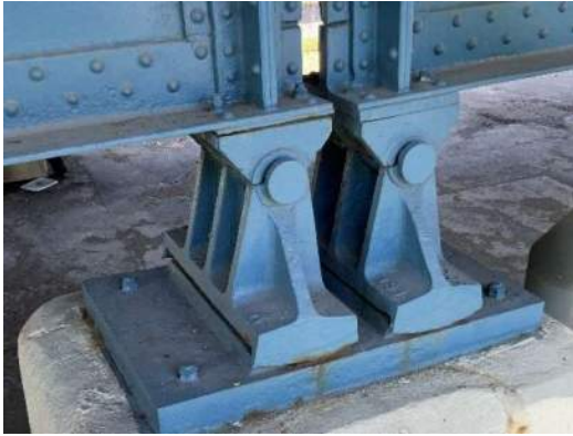
Photo 7E-001: Corrosion and pack rust between rocker assembly and masonry/sole plates at Pier 6E north bearing, looking southwest
