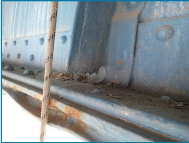
Photo 24 – Pack rust between the bottom flange cover plates with rust staining on the Right Girder between Floorbeams 30 and 31 in the Main Suspension Span (looking southeast). Note the 100% section loss to the base of the transverse stiffener.
