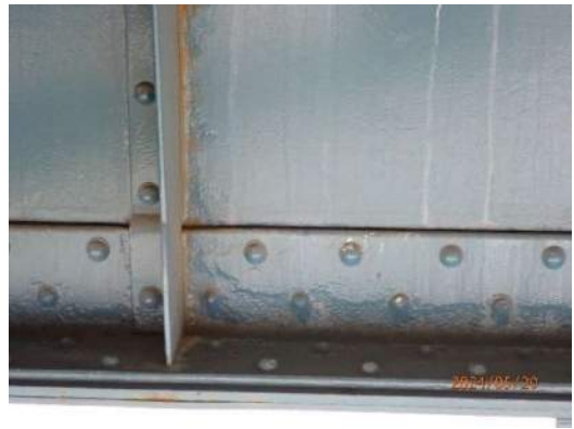
Photo MS-079: Pitting (1/8" deep) along bottom flange and stiffeners on Right Girder north face, between FB46 and FB46, looking south
