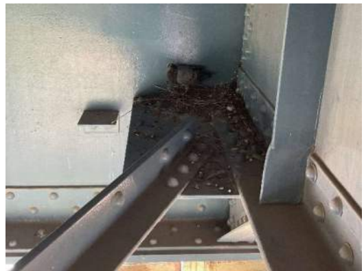
Photo 6W-006: Granular and bird debris on lateral bracing connection plate on east side of Right Girder at FB2, looking south
