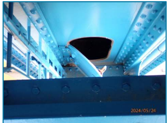
Photo 71 – Unsecured upper access hatch at the north leg of Tower D (looking north).
