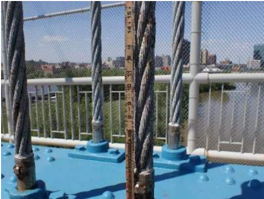
Photo NC-003: Suspender cable 10, areas of surface corrosion with active rust
