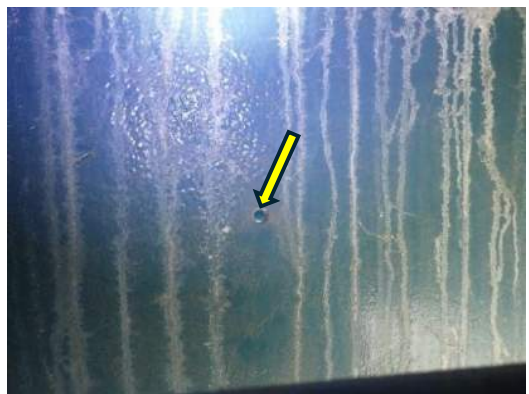
Photo MS-065: 3/8" drilled hole in Left Girder web, between FB42 and FB43, looking north. Fatigue category D detail
