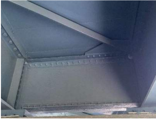
Photo 12E-001: Minor painted over pitting on cross frame, at pier 12E, between S11 and S12
