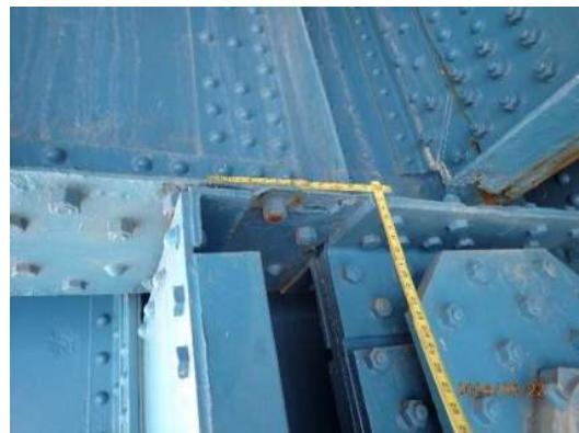
Photo MS-006: 1' long by 3" wide corrosion hole in Right Girder bottom flange north face at FB13, looking southwest
