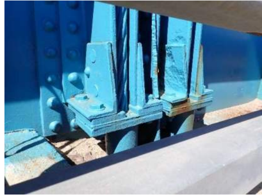
Photo ES-020: 6" wide portion of kneebrace removed above deck at Left Girder and FB63, looking northeast
