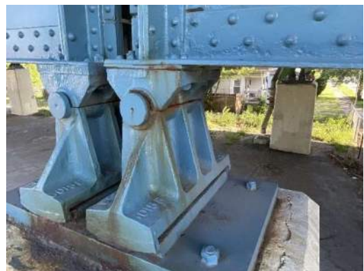
Photo 7E-006: Surface corrosion with pack rust on top of south bearing at pier 6E, looking northwest
