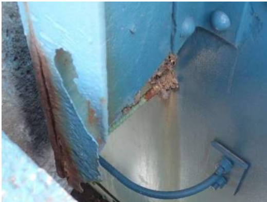
Photo ES-027: 100% section loss (11" high by 2" wide) on vertical gusset plate, south face connection angle leg, at Left Girder and FB65, looking northwest
