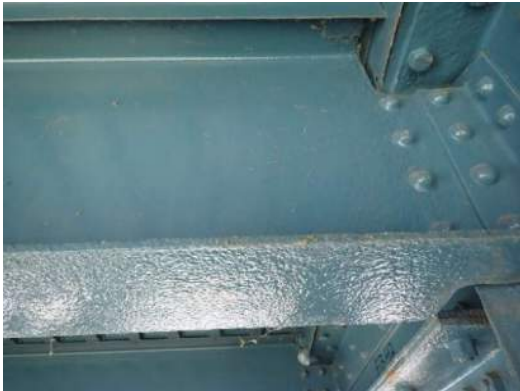
Photo MS-068: Pitting (1/16"-1/8" deep by full flange width by 36" long) on bottom flange of S6 east of FB42. Also pitting (full web height x 7" long) on web of S6. Looking southwest
