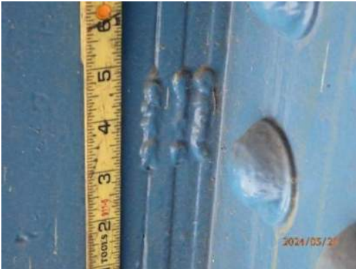
Photo MS-050: Tack weld between transverse stiffener angle and fill plate on north face of Right Girder, between FB35 and FB36, looking southeast
