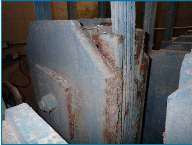
Photo 55 – Active pack rust between the eyebars and strand shoe (looking northwest, North Cable, Anchorage F).
