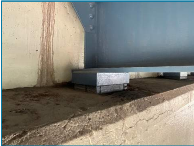
Photo 37 – Minor bulging of Beam 11 elastomeric bearing at Rear Abutment (looking northwest).
