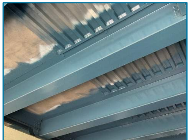
Photo 1 – Typical condition underside of deck and stay-in-place forms (looking up and northwest between Girders 9 and 11 in Span 14E).
