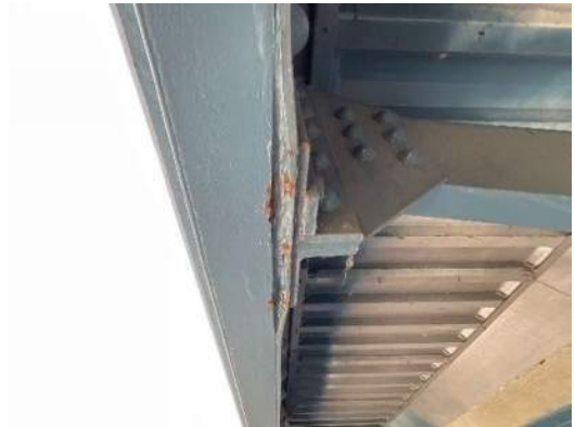
Photo 4E-002: Pack rust and painted over section loss to LS2 web, at intermediate bracket between FB0 and FB1, looking east
