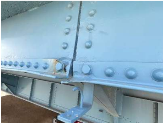
Photo 7W-003: Pack rust and painted over section loss at FB1 north overhang, at LS2, with minor active corrosion
