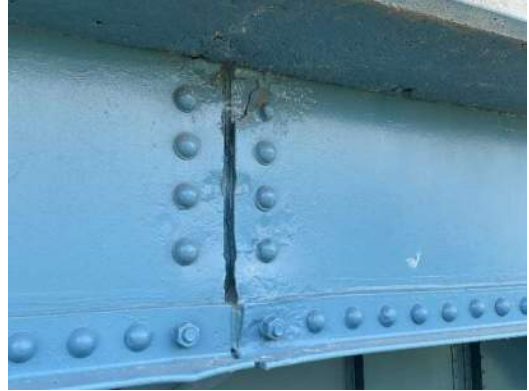
Photo 5E-008: Pack rust and painted over section loss on LS2 at FB2 overhang, looking southwest
