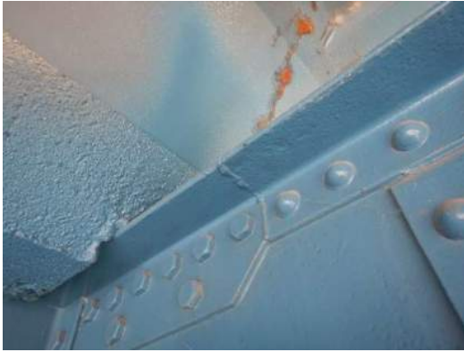
Photo 3W-001: Transverse weld in top flange of FB2 south cantilever between RS1 and RS2, looking east
