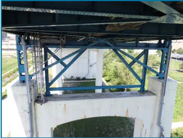
Photo 78 – Steel Pier Cap frame at Pier B (looking west).
