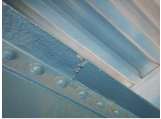
Photo 3W-004: Transverse weld in top flange of FB3 south cantilever between RS1 and RS2, looking west
