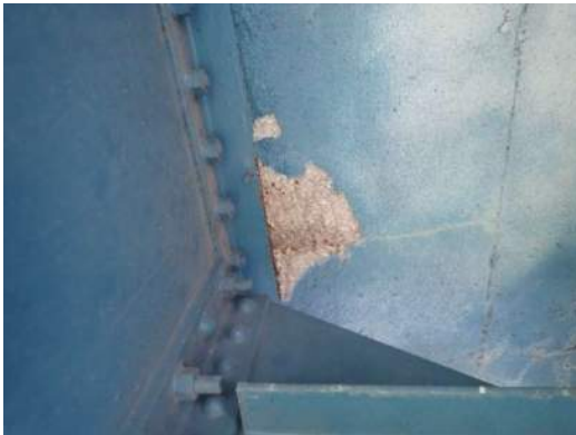
Photo ES-003: Spall (6" diameter by 1/2" deep) on underside deck south overhang, west of FB53
