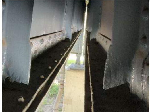
Photo 6E-008: 100% section loss on transverse stiffeners at bottom flange, FB4 east face, full length of FB4
