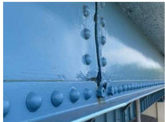
Photo 2E-004: Pack rust and painted over section loss of RS2 at FB2 overhang, looking northeast
