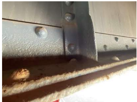
Photo 6E-002: Painted over section loss top and bottom flange, with active corrosion and painted pack rust intermittent along bottom flange of FB0, between S3 and S4
