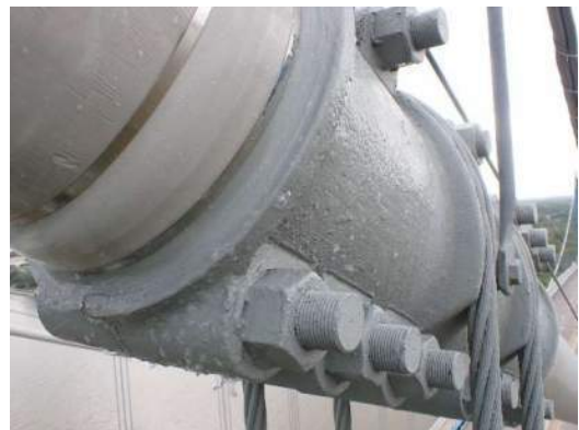
Photo SC-004: Main cable at suspender cable 15, leak, west end, south face
