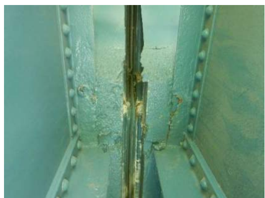
Photo 4W-006: Section loss up to 100% (2" long by 1" wide) on east side of FB4 top flange between LS1 and LS2, looking south
