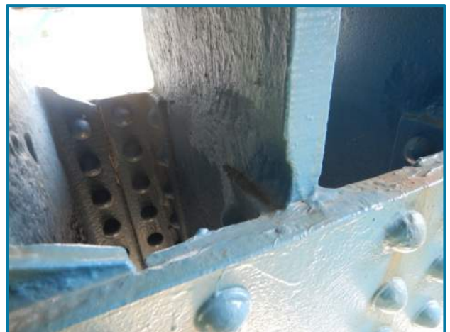
Photo 62 – 1/8" deep pitting of south link plate of the south column at Pier B (looking northwest).
