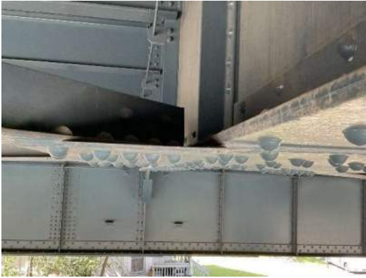
Photo 6E-007: Pack rust and bowing to lateral bracing connection plate, east and west of FB3, at S4
