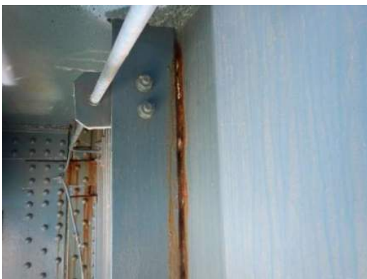
Photo MS-023: Pack rust (30" high by 3/4" thick) between transverse stiffener and Left Girder web, south face between FB26 and FB27, looking northwest
