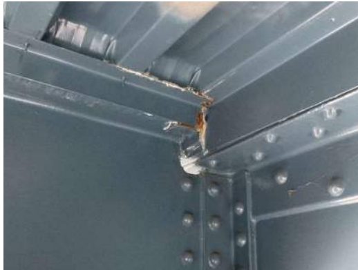
Photo 5E-009: Active corrosion and efflorescence at top flange of S4 and FB2
