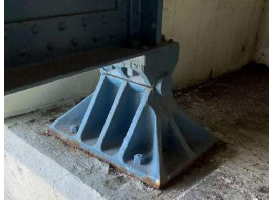
Photo 1E-002: Minor corrosion into masonry plate on Right Girder bearing at anchorage F
