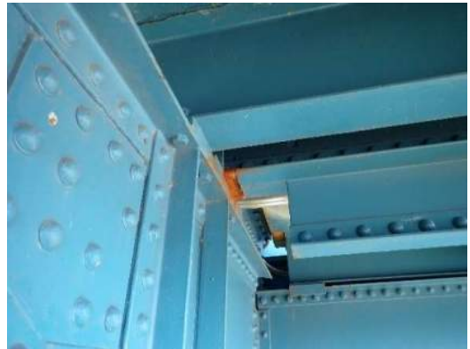
Photo MS-008: South sidewalk Stringer RS2 at FB13 with signs of expansion/contraction (2" on east side, 4" on west side), looking northwest
