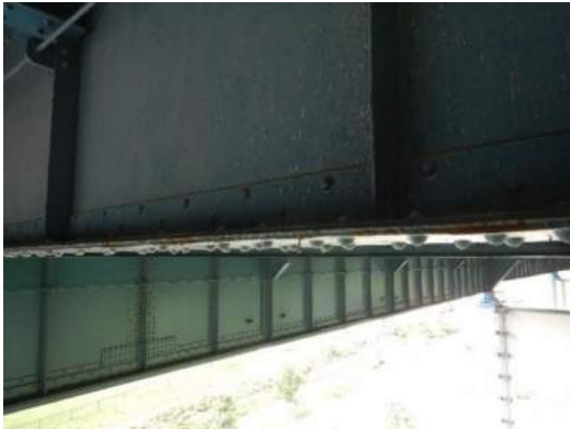
Photo 1W-003: Up to 1/2" thick pack rust between bottom flange and cover plate on FB4 at S3, looking southeast
