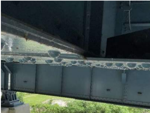
Photo 4E-003: Pack rust and bowing in lateral bracing connection plate at FB1 and S4
