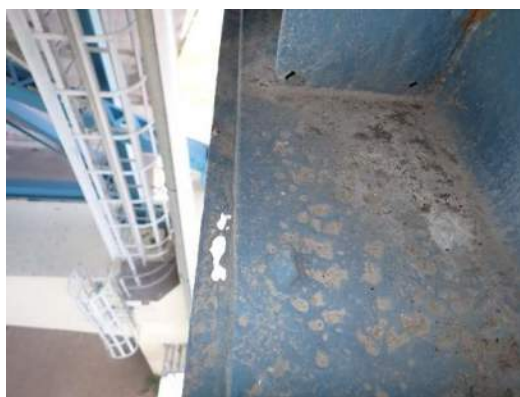
Photo ES-023: Pitting on top of bottom flange with up to 100% section loss on Right Girder, between FB64 and FB65
