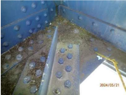
Photo MS-048: 100% section loss (1.75" diameter) in lateral bracing connection plate, west of FB35, at Right Girder, looking southeast
