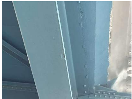
Photo 8W-002: Painted over gouge (3" long) on bottom flange of S13, between midspan sidewalk bracket and intermediate sidewalk bracket west of midspan
