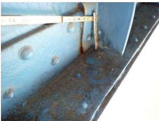
Photo MS-094: 100% section loss (4" high by full width) on transverse stiffener on Right Girder north face, west of FB51, looking west
