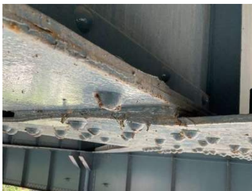
Photo 2E-005: Bowing on both sides of lateral bracing connection plate with painted over pack rust, at S4 and FB3 connection
