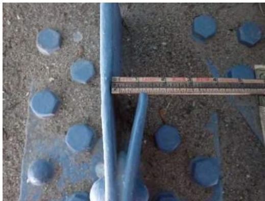
Photo MS-058: Pack rust between lower lateral brace angles, causing 1 1/8" deformation, at FB39 to Left Girder connection, looking north
