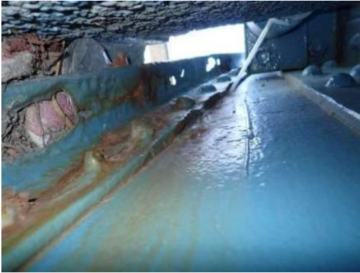
Photo MS-025: 100% section loss (up to 3" diameter) in multiple location on outstanding leg of Floorbeam Kneebrace, west face of FB27 at Right Girder, looking up and east
