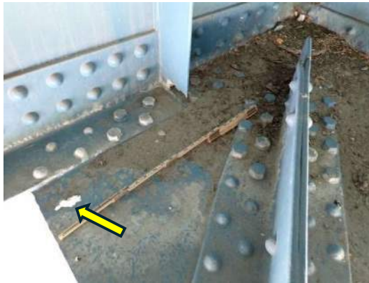
Photo MS-074: 100% section loss to lower lateral brace connection plate at Right Girder and FB45, looking southeast
