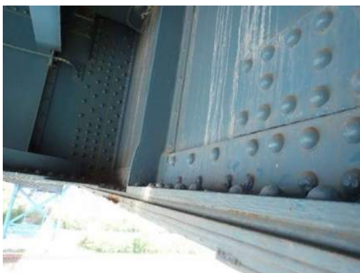
Photo MS-035: Pack rust between bottom flange plates on north edge of Right Girder, between FB29 and FB30, looking southeast
