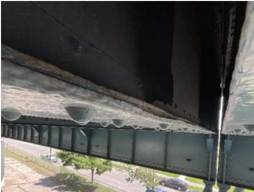
Photo 3E-003: Pack rust on bottom flange cover plate, causing waves on FB0 between S3 and S4
