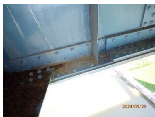
Photo MS-083: Section loss (25%-90%) of rivet heads on bottom flange of Left Girder, south face, between FB47 and FB48, looking northeast
