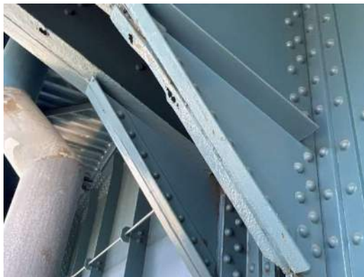
Photo 7E-005: Painted over pitting and 100% section loss in angle on FB0, between at RS2
