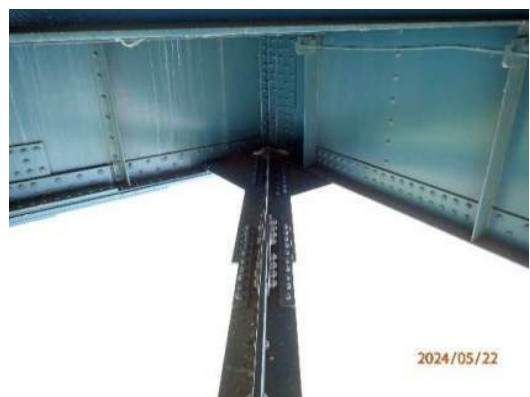
Photo MS-018: Bolted repair on lower lateral brace west of FB22 at Left Girder, looking northeast
