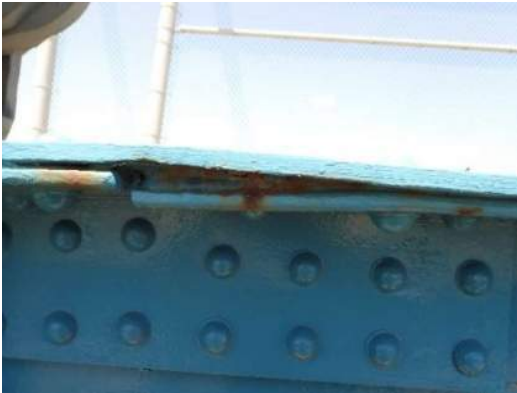
Photo WS-001: Pack rust between top flange plates of Left Girder at FB0, looking north
