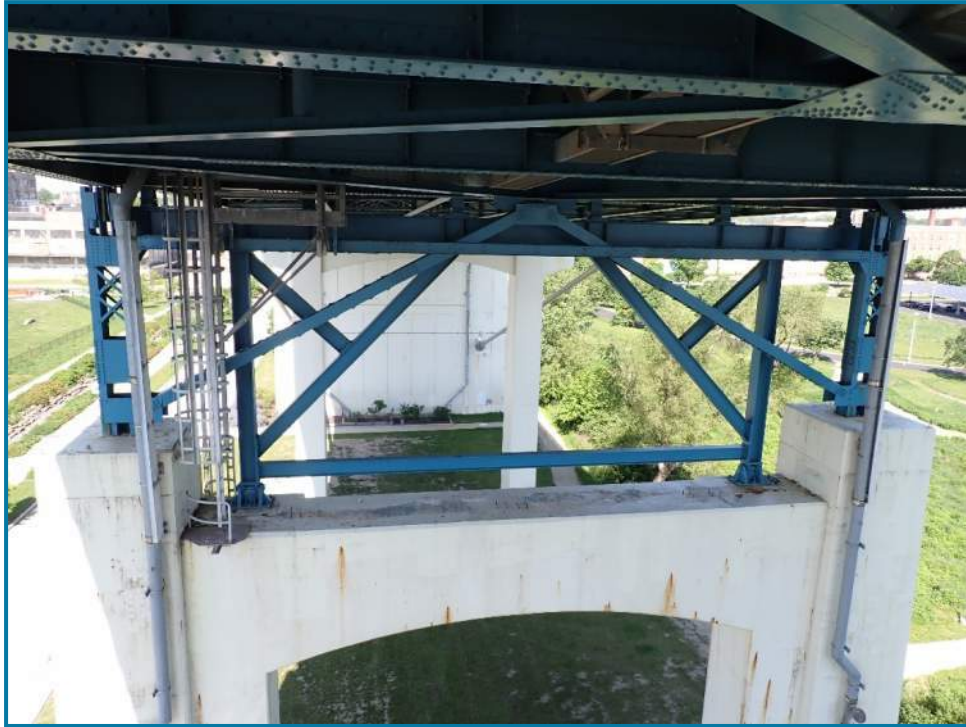
Photo 5 – Steel frame (Pier B shown, Pier E similar)
