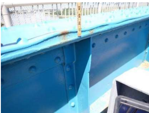
Photo WS-011: Pack rust between top flange plates on Left Girder between FB6 and FB7, looking northeast
