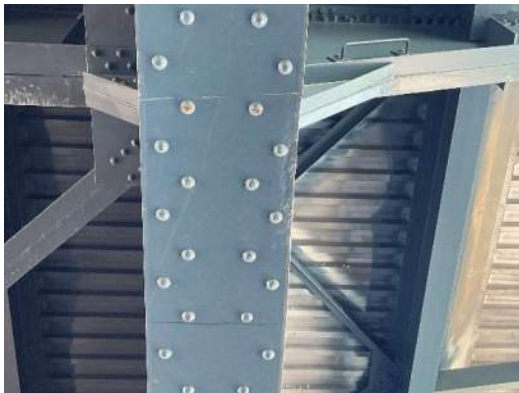
Photo 7E-009: Typical painted over section loss to bottom flange of Right Girder, intermittent for full length, shown at FB2
