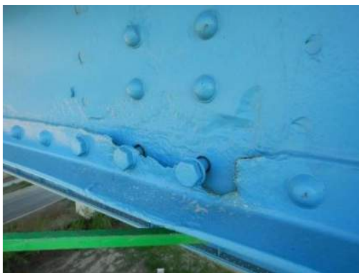
Photo 3W-005: 100% section loss by full height of vertical angle on exterior angle of RS2 near FB4, looking north
