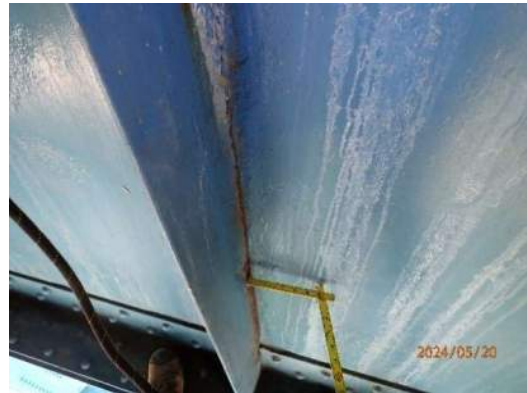
Photo MS-099: Pitting (1/16" deep by 2" wide by full height) on north face of Right Girder at stiffeners, between FB51 and FB52, looking south
