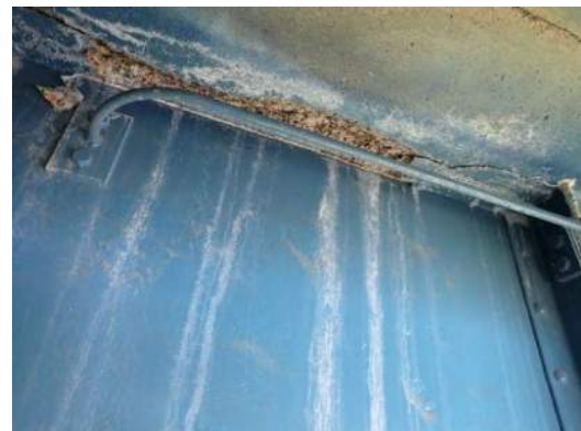
Photo MS-063: Spall (6" wide by 3' long) and delamination (6" wide by 16" long) on underside of deck along north face of Right Girder, west of FB41, looking southwest
