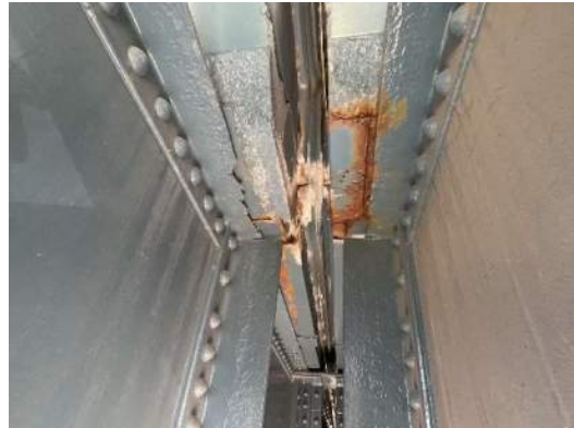
Photo 3E-010: Corrosion and efflorescence on joint above RS1 top flange and deck pan flashing on FB4 east face
