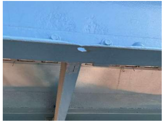
Photo 7E-008: 100% section loss in bottom flange angle of RS2 south face, between FB0 and FB1, looking north
