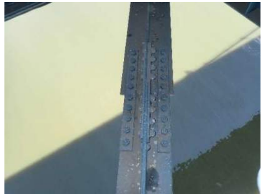
Photo MS-045: Bolted repair on lower lateral bracing at FB35 near Left Girder, looking northeast
