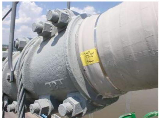
Photo SC-006: Main cable at suspender cable 46, leak in cable gouge, east end, south face
