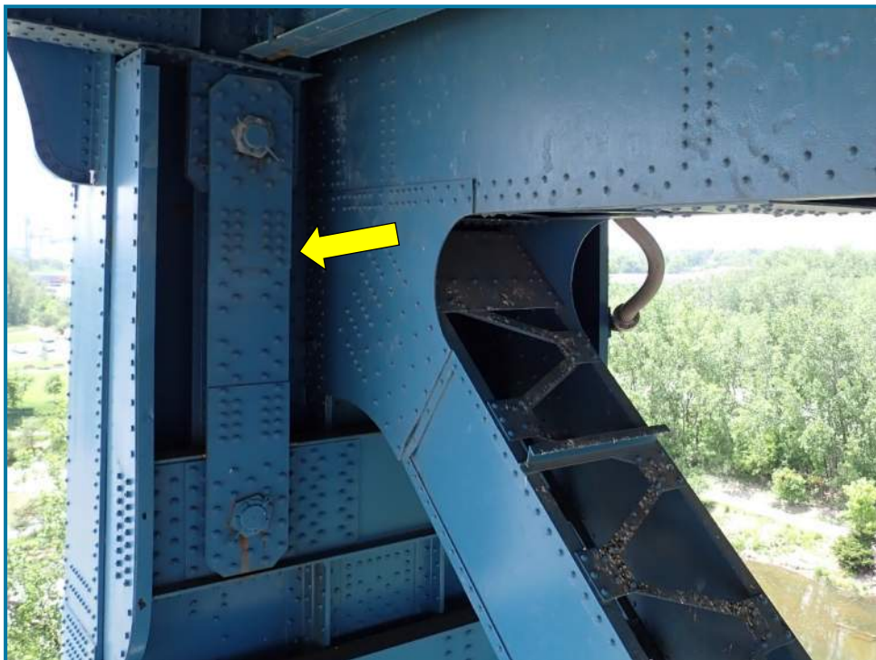
Photo 6 – Typical link pin and hanger assembly at the tower
