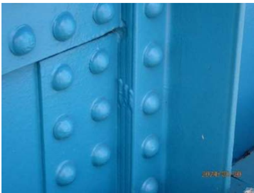
Photo ES-017: Tack welds on north face of Left Girder transverse stiffener, between FB61 and FB62, looking southwest
