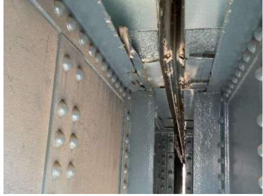
Photo 5E-002: Painted pitting on stiffeners and bottom flange of FB0 north overhang, active corrosion to top flange and deck pan flashing, with efflorescence, looking south
