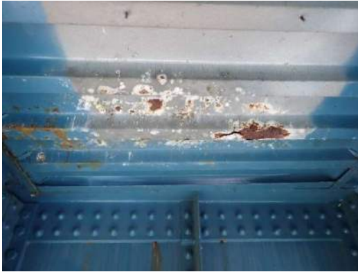
Photo ES-007: Laminate corrosion (3' wide by 1' long) on underside of pan between S1 and S2 and between FB54 and FB55
