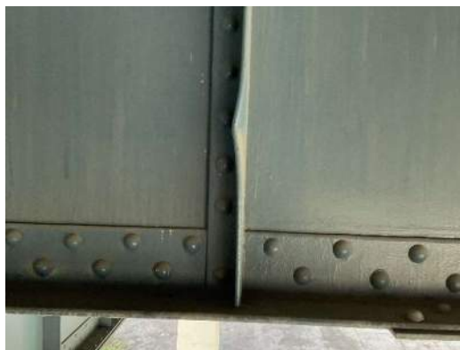
Photo 3E-005: Impact damage to transverse stiffener, painted over, on S2, west of FB1
