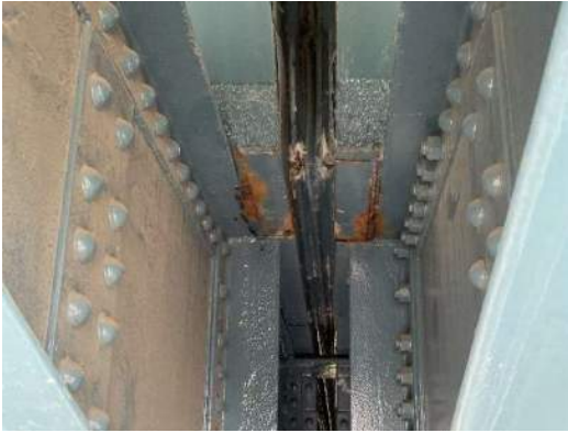
Photo 4E-001: Active corrosion to top flange of FB0 north overhang and deck pan flashing, looking south
