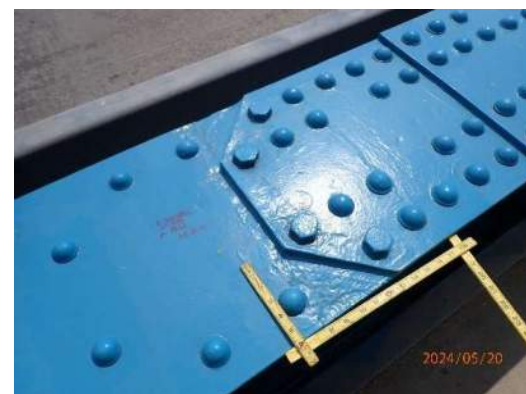
Photo ES-018: Section loss (1/8" deep by 5" wide by 6" long) top flange of Left Girder, between FB61 and FB62, looking southwest
