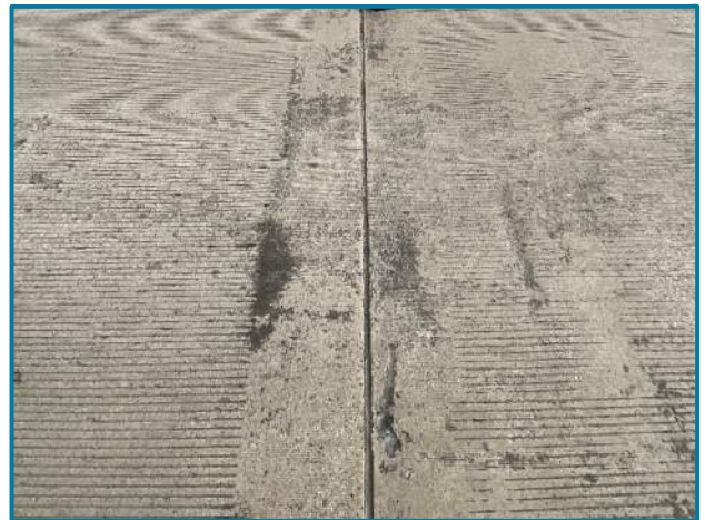
Photo 7 – Pourable strip seal at Forward Abutment, eastbound lanes (looking north).
