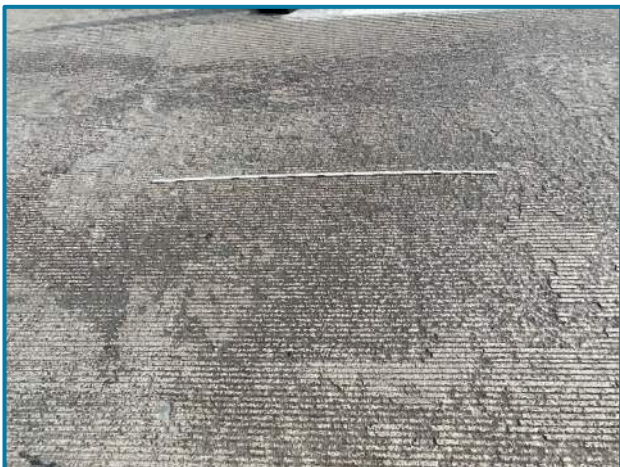
Photo 4 – Isolated area of moderate abrasion/wear in the Main Suspension Span near Tower C (looking north).
