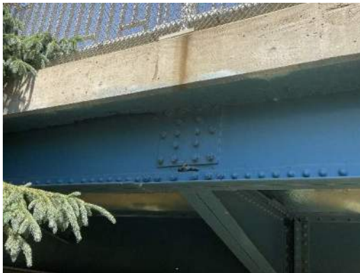
Photo 13E-003: Painted over corrosion with 100% section loss and pack rust between bottom angle/web of S13 at pier 12E, looking northeast
