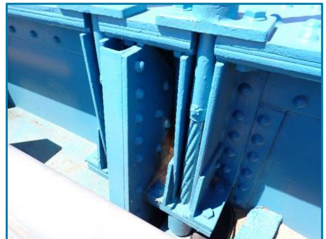
Photo 57 – Accumulation of roadway debris between the stiffeners at deck level at the North Suspender Cable 5 at Left Girder (looking northwest)
