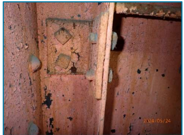
Photo 69 – Missing nuts at ladder connection and typical paint condition of the easternmost cell of Tower D in the south leg (looking southeast).
