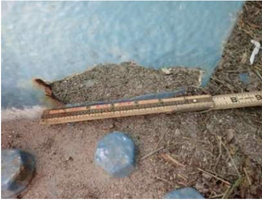
Photo MS-042: 100% section loss (7" long by 3.5" high) in lower lateral bracing web angle at FB33 near Left Girder, looking west
