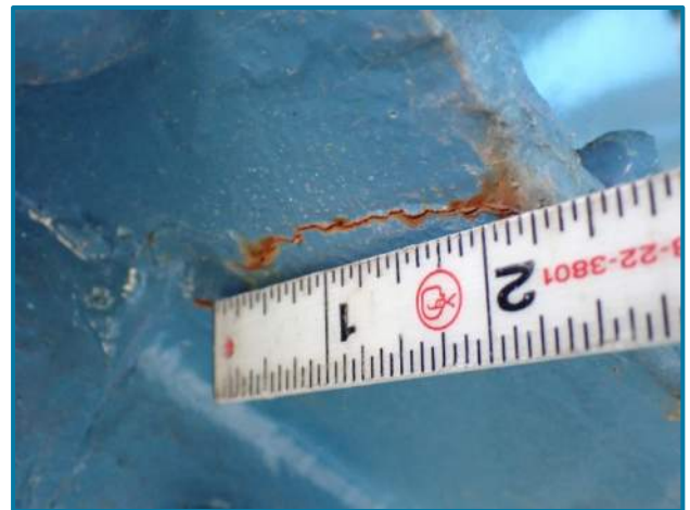
Photo 35 – Cantilever sidealk bracket at Floorbeam 51, top flange with 1 3/4" long crack between Left Stringer 1 and Left Girder in Main Suspension Span (looking southwest). Note the arrest hole filled with caulk.
