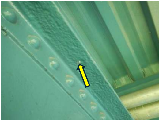
Photo 3W-003: 100% section loss (1/4" diameter) in top flange of FB3 east face between LS1 and LS2, looking northwest
