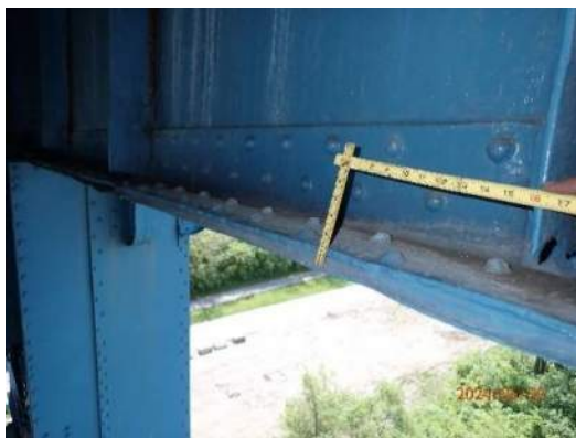
Photo MS-100: Pack rust (1/2" - 1" thick) between Right Girder bottom flange connection angle and bottom plate, between FB51 and FB52, looking southeast
