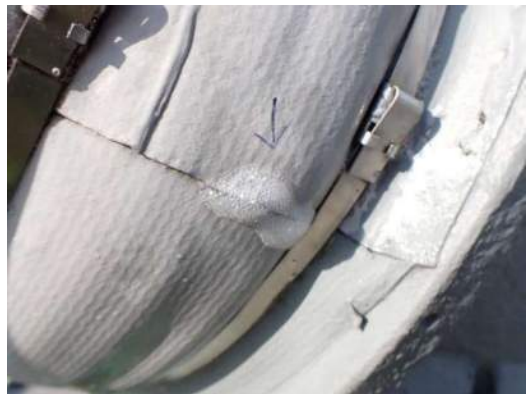
Photo SC-002: Main cable at suspender cable 5, slight leak at tape seam, east end, south face
