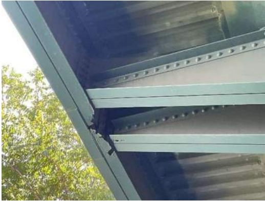
Photo 9E-001: Painted over corrosion and 100% section loss and pack rust between bottom angle/web of S1 at pier 9E
