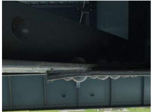
Photo 4E-010: Painted over pack rust and bowing of lateral bracing connection plate under lateral bracing angle and FB3 bottom flange, at S4
