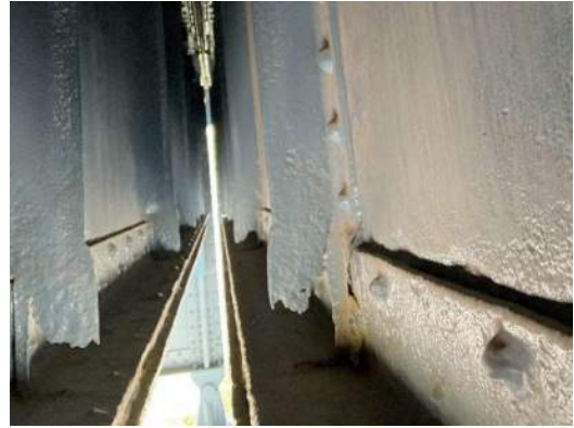
Photo 3E-002: 100% section loss on transverse stiffeners on west face of FB0, between S3 and S4
