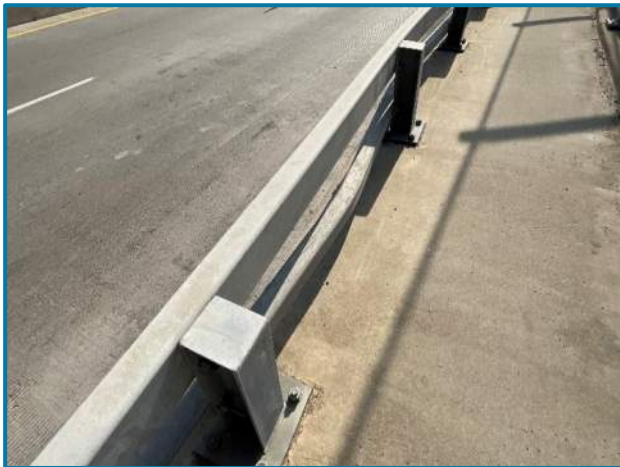
Photo 11 – Impact damage to south railing in Span 8W at Rear Abutment (looking northeast).
