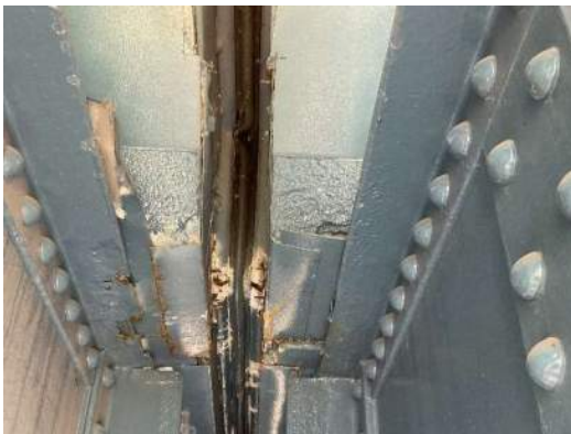
Photo 4E-011: Painted over corrosion on top flange of FB4 north overhang, with active corrosion and efflorescence on deck pan flashing above FB4, looking south
