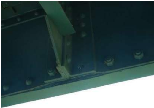
Photo 4W-003: Missing bolt at utility hanger connection on LS2 between FB3 and FB4, looking north
