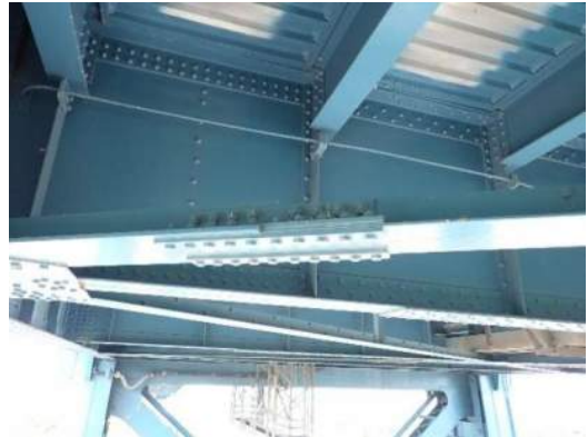
Photo ES-008: Bolted repair plates on lower lateral bracing between FB56 and FB57, near S11
