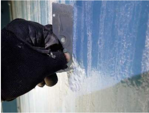
Photo MS-019: Pitting (3/16" deep by 3" diameter) on web of Right Girder between FB22 and FB23
