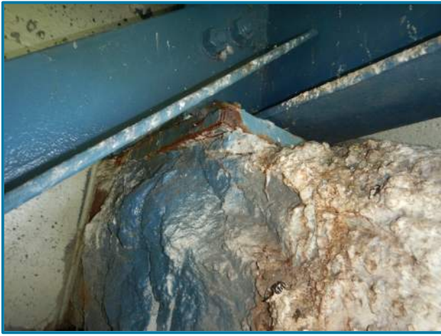
Photo 41 – Bearing seat spalled exposing up to a 1/2" wide by full length of the the masonry plate under Stringer 1 at Anchorage A (looking northwest).
