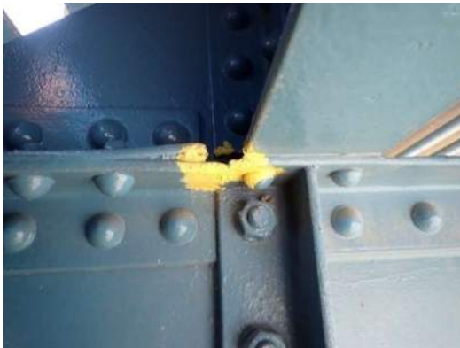
Photo MS-080: Crack highlighted with yellow paint in top flange of south sidewalk cantilever of FB47 west face, looking east
