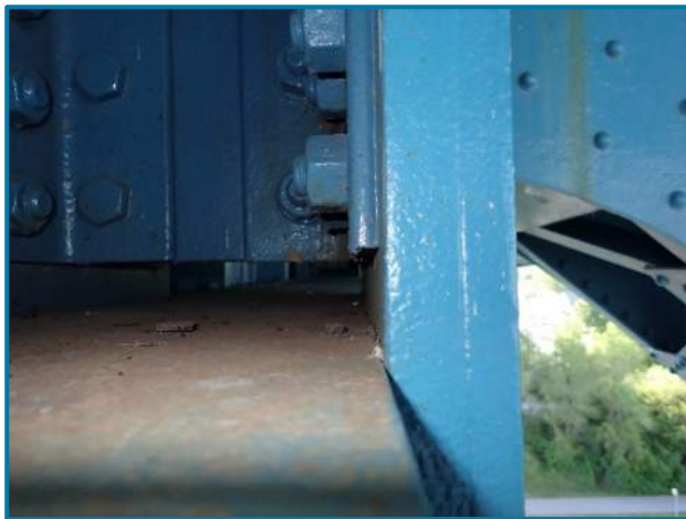
Photo 61 – Contact between link plates and tower pin tie beam at the lower west pin at the north leg of Tower D (looking east).
