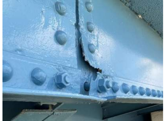
Photo 1E-004: Pack rust and painted over section loss of LS2 at FB1 overhang, looking west
