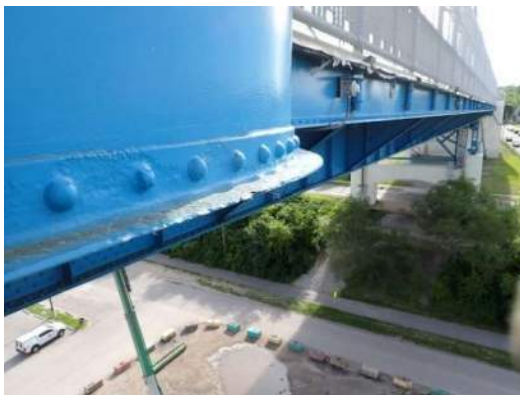
Photo ES-005: 100% section loss and knife edge on exterior bottom flange at tower D, south sidewalk exterior stringer, looking northeast
