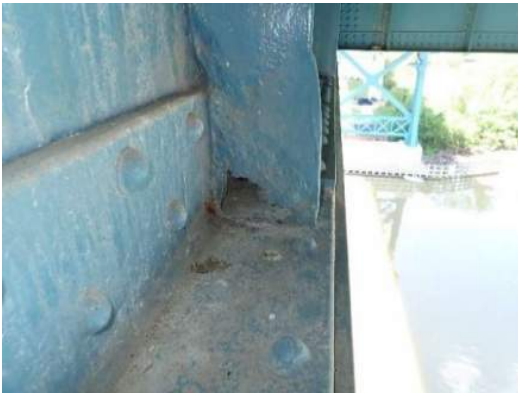
Photo MS-027: 100% section loss (4" wide x 3" high) to transverse stiffener on Right Girder north face, between FB27 and FB28, looking west
