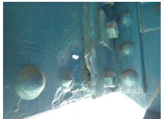
Photo ES-022: Pack rust (1" thick) and pitting (1/8" deep) with areas of 100% section loss at FB63 connection to RS2
