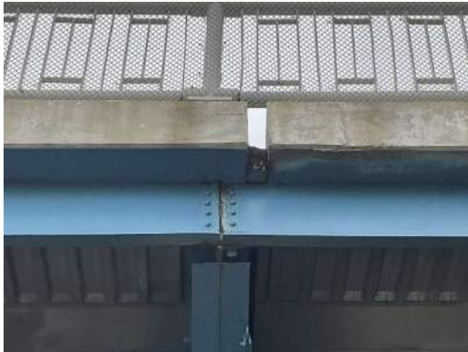
Photo 8W-003: Typical connection painted over section loss on south face of S14 at midspan sidewalk bracket, looking north
