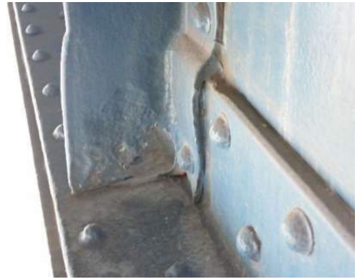
Photo MS-073: 100% section loss (3" high by full width) on transverse stiffener on south face of Left Girder, between FB44 and FB45, looking west
