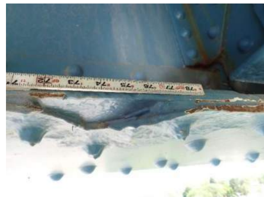
Photo ES-012: 100% section loss on rivet heads and pitting on bottom flange of Left Girder, between FB58 and FB59
