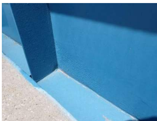
Photo WS-005: Pitting to the web of the Right Girder, near FB1
