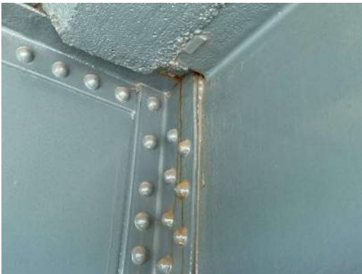
Photo 3E-009: Pack rust and bowing on RS1 at FB3 connection
