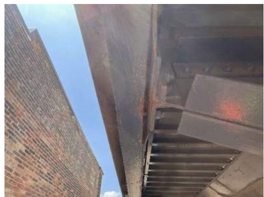
Photo 7W-006: Pack rust between bottom angle/web of stringer RS2 at FB2, looking west
