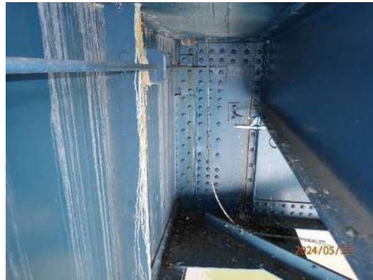
Photo MS-020: Typical efflorescence staining on east face of FB24 web, between S11 and Right Girder, looking west
