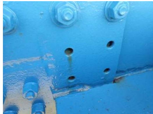
Photo MS-022: Eight bolt holes in repair plate, north web of Left Girder, east of FB25, looking south
