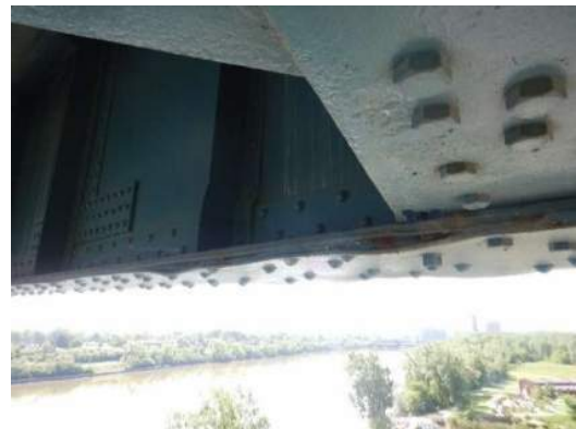
Photo WS-010: Pack rust between bottom flange plates on Right Girder between FB5 and FB6, looking southeast
