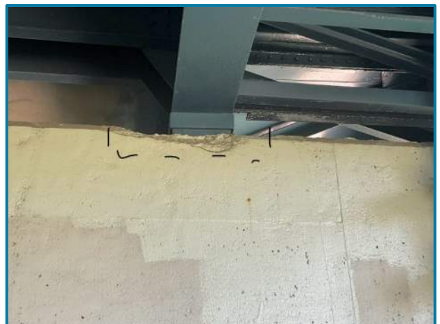
Photo 80 – 2' wide by 6" high by 3" deep spall on the west face of the Pier 11E cap under Beam 11 (looking east).
