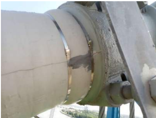
Photo SC-003: Main cable at suspender cable 9, slight leak at tape seam, west end, north face
