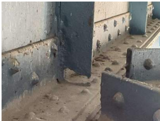
Photo 1E-005: 100% section loss to transverse stiffener below S4, west side of FB2, looking south
