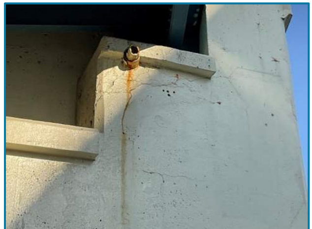
Photo 76 – Isolated 2' wide delamination and rust staining from the existing conduit at the Rear Abutment under Beam 1 (looking west).
