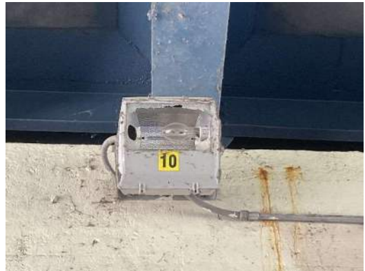
Photo 14E-002: Broken light cover below S7, at pier 13E, looking west
