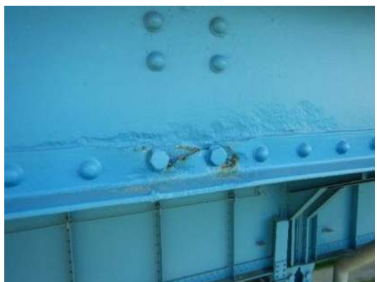
Photo 3W-006: 100% section loss by full height of vertical angle on exterior angle on RS2 between FB4 and FB5, looking north
