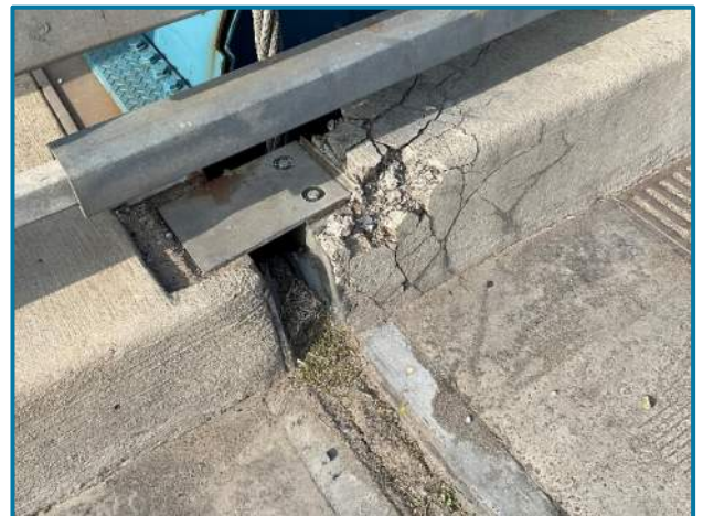
Photo 5 – 1' long by 6" wide by 1" deep curb spall with surrounding delaminated area at Pier E expansion joint, south curb (looking south).
