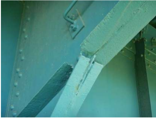
Photo 1W-001: 100% section loss on FB4 north cantilever bracket bottom flange, looking up and south
