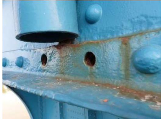
Photo ES-004: Two missing rivet heads at tower D, between south exterior stringer and sidewalk bracket, east most railing connection, looking north
