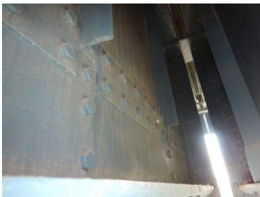
Photo 5W-005: 12" flame cut from bottom of stiffener on FB3 east face, at Left Girder, looking north
