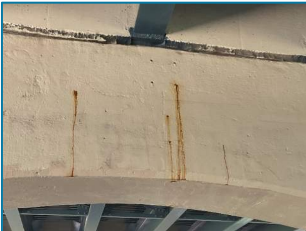
Photo 79 – Typical minor rust staining on the east face of the Pier 9E cap (looking west).
