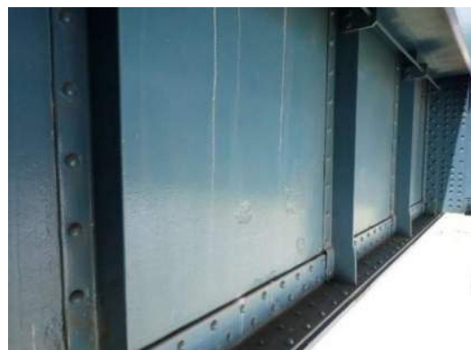
Photo MS-069: Pitting on north face web of Right Girder between FB42 and FB43, looking southwest
