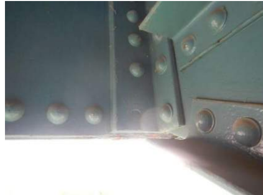
Photo 4W-004: Popped rivet head at the LS2 and FB4 connection, looking northwest
