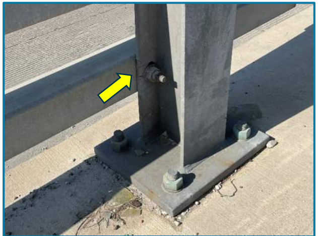
Photo 10 – Crack extending from the lower bolt hole on the east flange of the north railing post in Span 15E at Forward Abutment (looking southwest).
