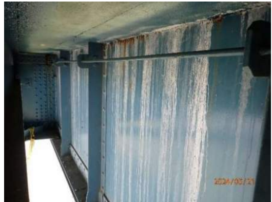
Photo MS-040: Efflorescence staining on north face web of Right Girder, between FB32 and FB33, looking southeast
