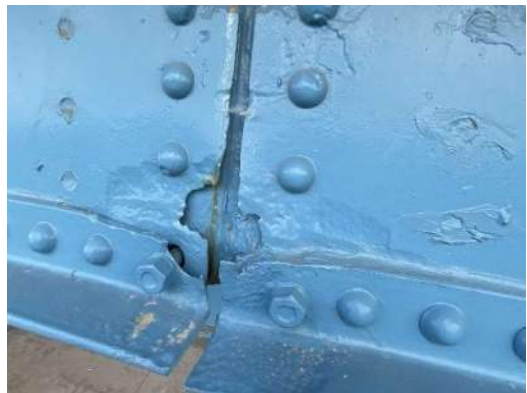
Photo 4E-008: Pack rust and painted over section loss of RS2 at FB2 south overhang, looking northwest
