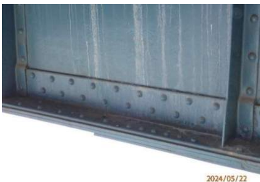
Photo MS-017: Rivets heads with 100% section loss and pitting on bottom flange of Right Girder north face between FB18 and FB19, looking south
