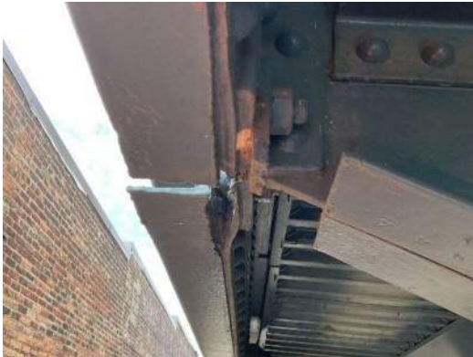
Photo 6W-003: Pack rust between bottom angle/web of stringer RS2 at FB1, looking west
