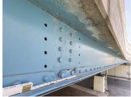
Photo 7W-004: Pack rust and painted over section loss on FB2 north overhang, at LS2, looking southwest
