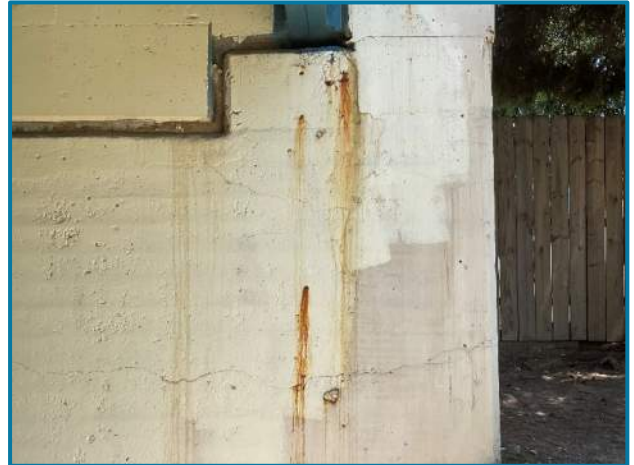
Photo 77 – Typical areas of moderate width horizontal and diagonal cracking with rust staining at the Forward Abutment under Stringer 13 (looking east).
