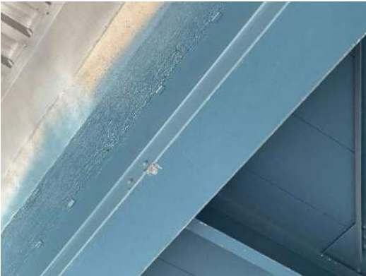
Photo 14E-003: Minor impact scrapes on bottom flange of S12 near midspan
