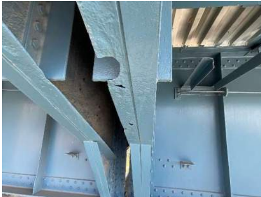
Photo 5W-003: 100% painted over section loss on bottom flange of FB0 south overhang, between RS1 and RS2
