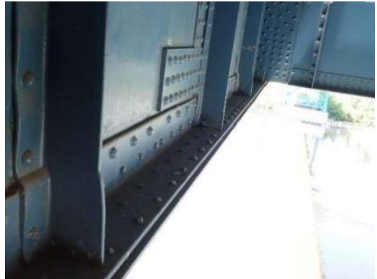
Photo MS-085: 100% section loss (up to 2" high and full width) on 3 transverse stiffeners on north face of Right Girder, between FB48 and FB49, looking west
