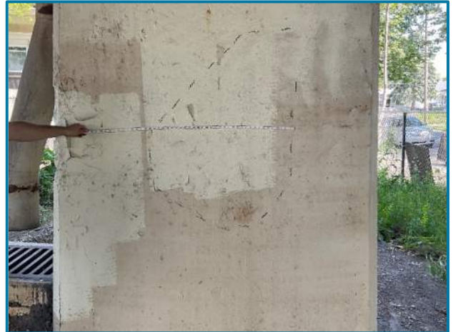
Photo 74 – Isolated delamination on the south face of Column 1
