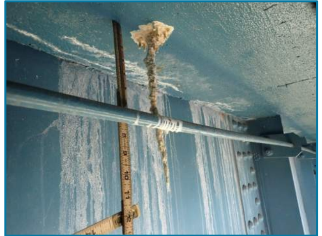
Photo 2 – Typical efflorescence along girders in suspension spans and isolated location of a stalactite (looking southwest at the north face of Right Girder between Floorbeams 29 and 30 in the Main Suspension Span).
