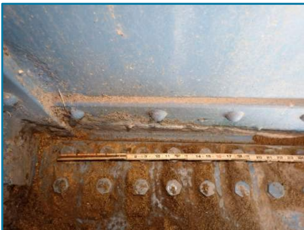
Photo 22 – 1/4" deep pitting of bottom flange angle and rivet head loss up to 100% at Left Girder in Main Suspension Span at Floorbeam 39 (looking north).
