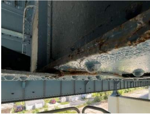
Photo 1E-007: Pack rust with minor deformations to lateral bracing connection plate, at S4 and FB2 interface
