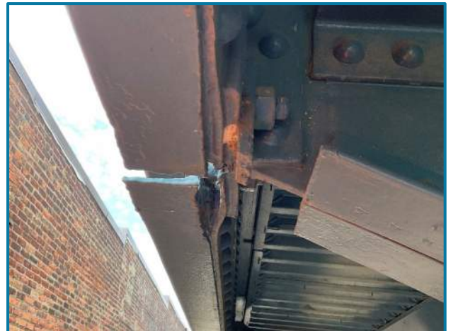
Photo 29 – Pack rust between bottom flange angle and web plate of Right Stringer 2 at Floorbeam 1 in Span 6W (looking west).
