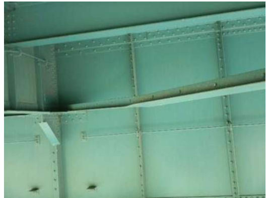
Photo 1W-002: Distorted and twisted up to 2' long on north lateral bracing between FB4 and FB5, looking north
