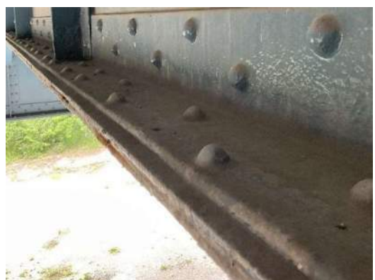
Photo 4E-006: Pack rust between bottom flange plates and pitting along top of bottom flange on FB2 west face
