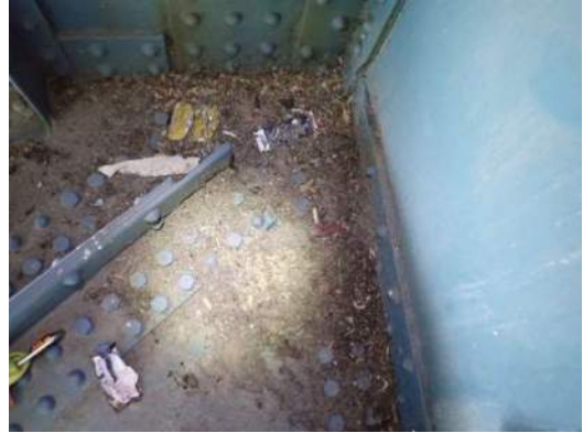
Photo MS-097: Dirt and debris accumulation on lateral bracing connection plate between FB51 and FB52, south face of Left Girder, looking northwest
