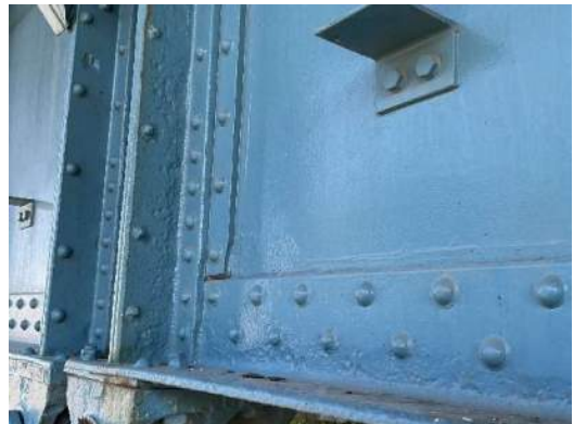
Photo 7E-004: Painted over pitting on FB0 angles, west face, near RS1, looking northeast
