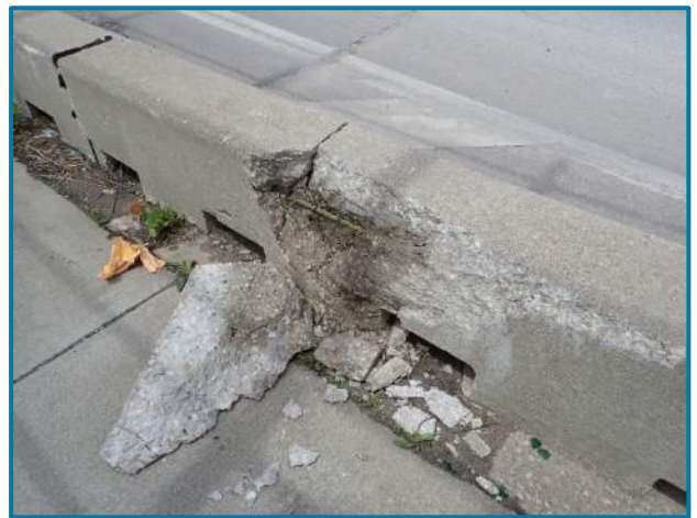
Photo 89 – Rear Approach guardrail with 4' long by 2' high by 6" deep spall with exposed reinforcement (looking north).
