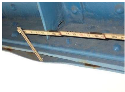
Photo MS-053: Pack rust (2" thick) between bottom flange plates of Left Girder, between FB36 and FB37
