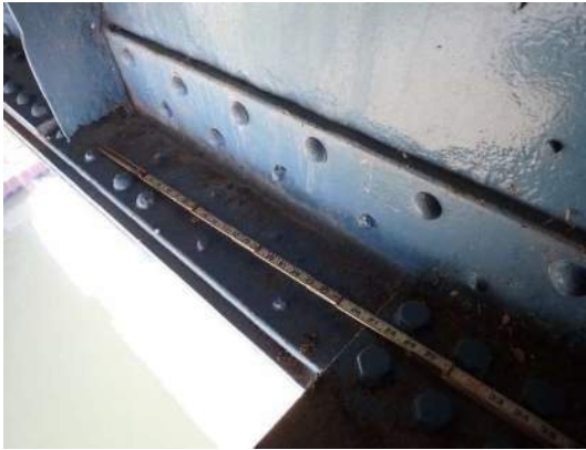
Photo MS-072: Up to 100% section loss on rivet heads on bottom flange on north face of Right Girder, east of FB43, looking southeast
