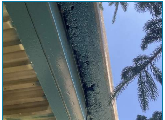
Photo 19 – Poorly consolidated concrete along Stringer 13 in Span 12E (looking east).
