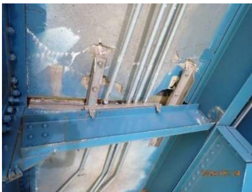
Photo MS-005: Spalling (2' long by 18" wide x full depth) with exposed reinforcement at south cantilever sidewalk at first intermediate bracket east of FB13, looking west
