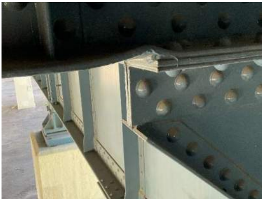
Photo 6E-003: Minor impact damage to bottom flange of FB1, south of Left Girder, looking northwest
