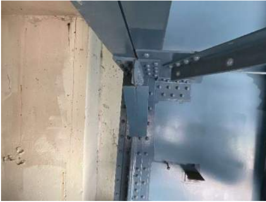
Photo 1E-001: Painted over pack rust and minor distortion to bottom angle of kneebrace under FB0 at Left Girder
