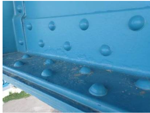
Photo ES-014: Pitting (1/16" - 1/8" deep) on bottom flange of Right Girder, between FB60 and FB61
