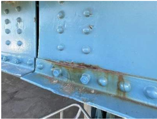
Photo 7E-007: Pack rust and painted over section loss to RS2 at FB0, looking northwest
