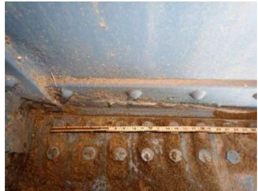
Photo MS-059: Pitting (up to 3/16" deep) and 100% section loss on rivets on Left Girder web angle, at FB39, looking north
