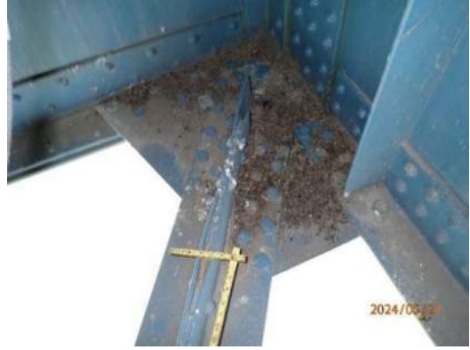
Photo MS-043: Pack rust (1" thick) between vertical flanges of lower lateral bracing, east side of FB33, at Right Girder, looking southwest
