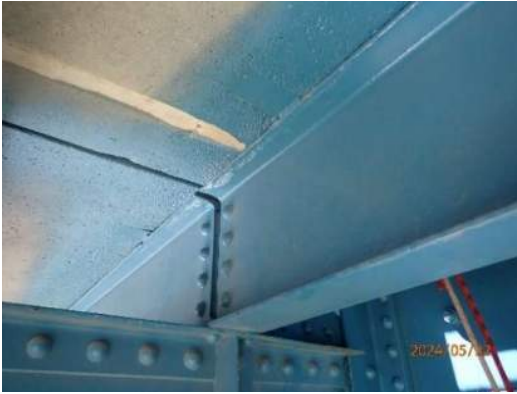
Photo MS-060: Pitting (2.5' long by 1.5" wide by up to 1/4" deep) on top flange north and south face of RS1, east and west of FB39, looking northwest
