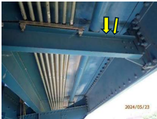
Photo MS-015: Two 3/4" diameter holes through top flange north overhang utility hanger between FB17 and FB18, looking west
