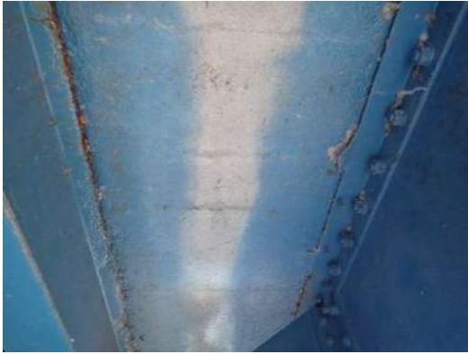
Photo ES-001: Hairline transverse cracks spaced 12" apart between LS1 and LS2, between FB53 and FB54
