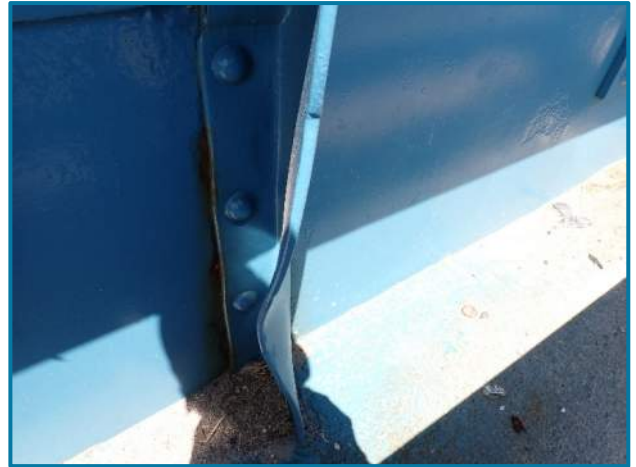
Photo 25 – Impact damage to transverse stiffener above deck of the Left Girder between Floorbeams 1 and 2 in the West Suspension Span (looking northeast).
