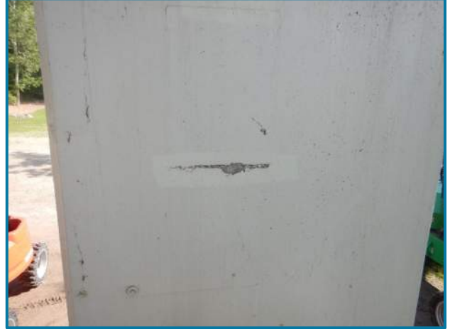
Photo 75 – Isolated spall on the south face of Column 1 at Pier 4W below an existing patched area (looking north).
