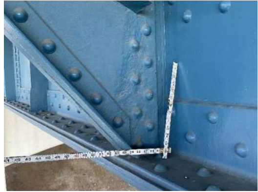
Photo 5W-008: Painted over pitting near FB2 and RS1 interface
