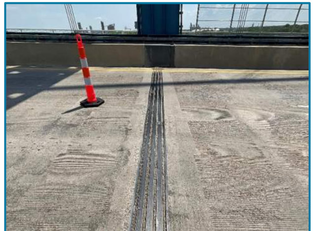
Photo 8 – Debris accumulated in Tower C modular expansion joint, westbound lanes (looking south).
