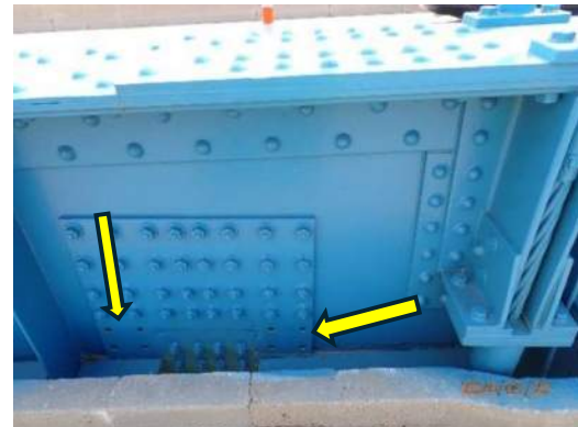
Photo ES-016: Eight open holes in north face repair plate on Left Girder, between FB61 and FB62, looking south
