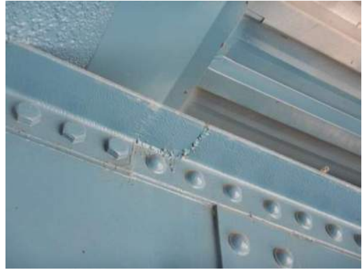
Photo 4W-008: Transverse weld in top flange of FB4 south cantilever between RS1 and RS2, looking southeast
