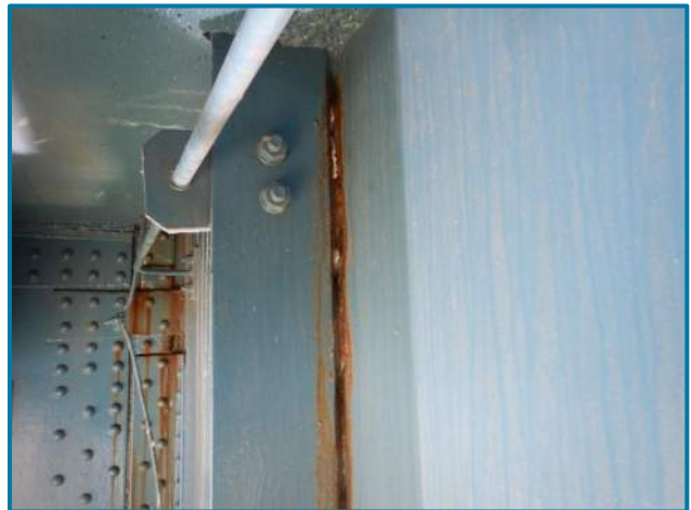
Photo 23 – Laminate corrosion to the edge of fill plate and girder web along the edge of the transverse stiffener on the Left Girder between Floorbeams 26 and 27 in the Main Suspension Span (looking west).
