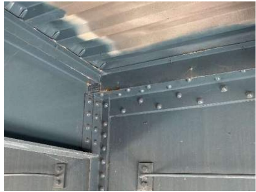
Photo 3E-008: Corrosion to deck pan flashing, along FB3, with efflorescence on north and south sides of S4
