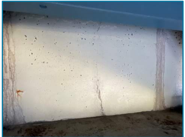
Photo 81 – Hairline cracking and isolated 2' wide delamination on the Rear Abutment backwall between Beams 11 and 12 (looking west).
