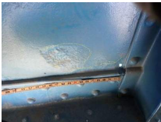
Photo MS-070: Hole (1/2" diameter) with advanced section loss (1/4" deep by 9" long by 4" high) on north face web of Right Girder between FB42 and FB43, looking south
