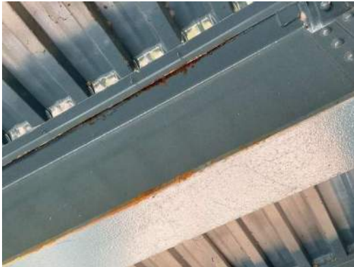
Photo 1E-009: Active corrosion (8' long) to top and bottom flange of S5, east of FB3
