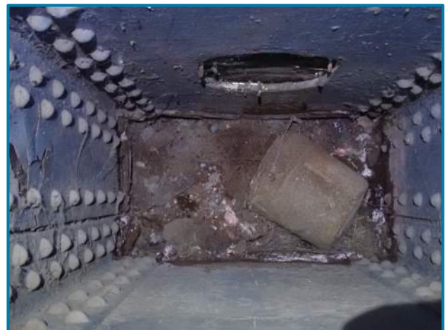
Photo 73 – Debris and laminate corrosion in the center cell of Tower D at the north leg base (looking east/down).
