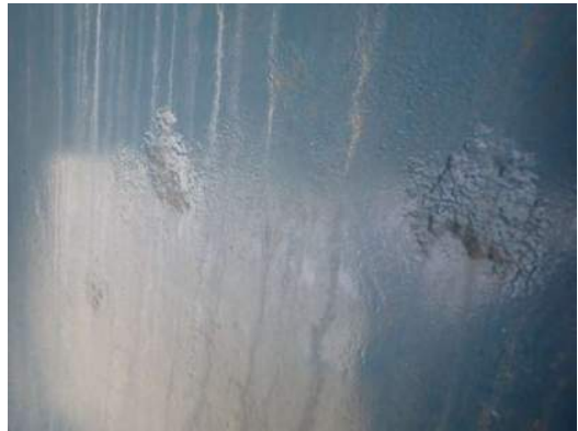
Photo MS-067: Pitting (1/16"-1/32" average depth) for 50% south web area on Left Girder between FB42 and FB43. Isolated locations up to 3/16" deep x 4" diameter, looking northwest
