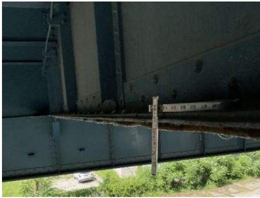
Photo 3E-007: 100% section loss on transverse stiffener on FB2 and pack rust along bottom flange of FB2, between S3 and S4
