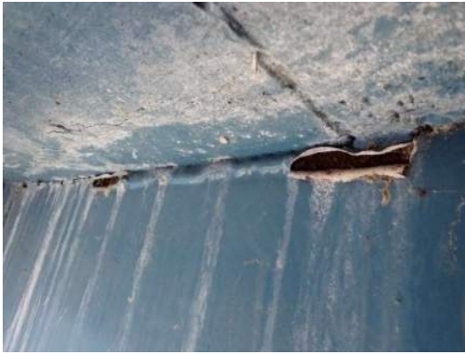
Photo MS-031: Peeling paint with laminate corrosion along edge deck and minor rust staining on north face of Right Girder, between FB28 and FB29, looking southeast
