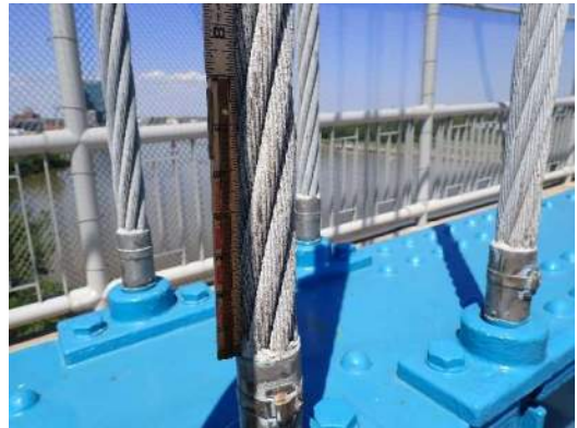
Photo NC-002: Suspender cable 8, coating failure
