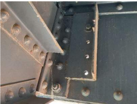
Photo 6W-005: Three missing bolts on stiffener angle on FB2 south overhang, at RS2
