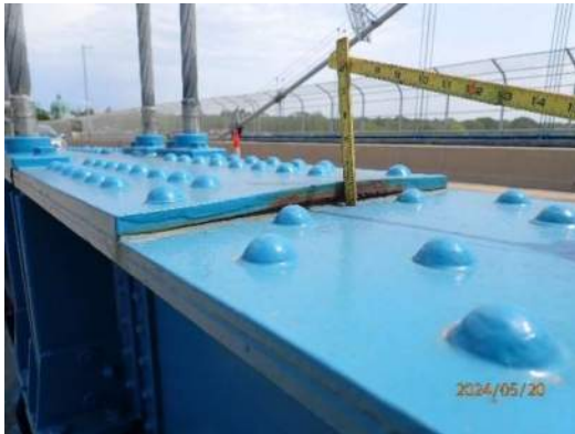
Photo ES-015: Pack rust (3/8" thick) on top of Left Girder between top flange plates, between FB60 and FB61, looking southeast
