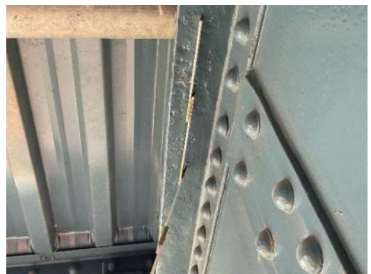
Photo 5W-006: Minor perforations in top flange of FB2 north overhang, near LS1, looking south
