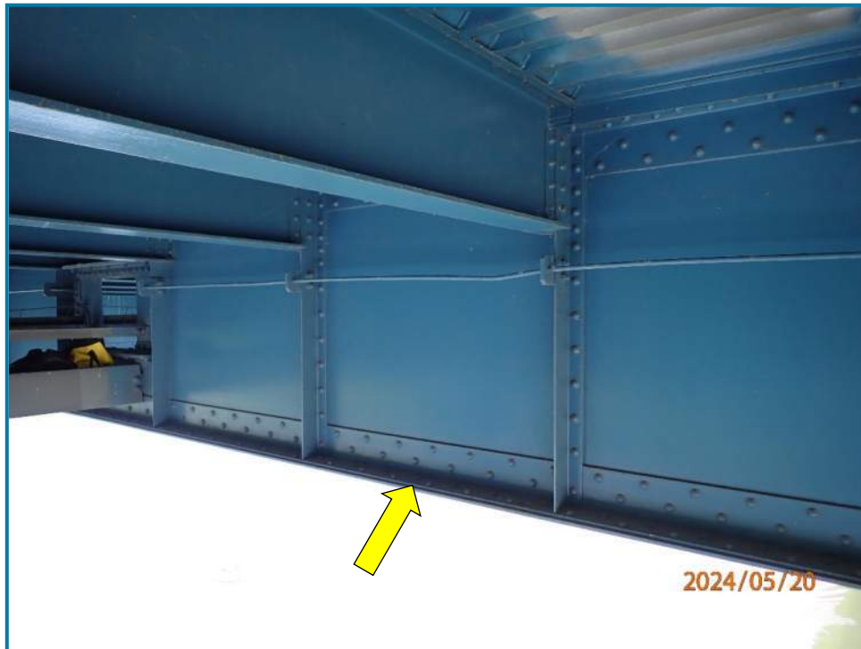
Photo 3 – Typical built-up floorbeam shown in the Main Suspension Spans (other spans similar)
