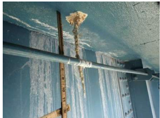
Photo MS-034: Efflorescence on underside of deck between FB29 and FB30, along Right Girder, looking southwest
