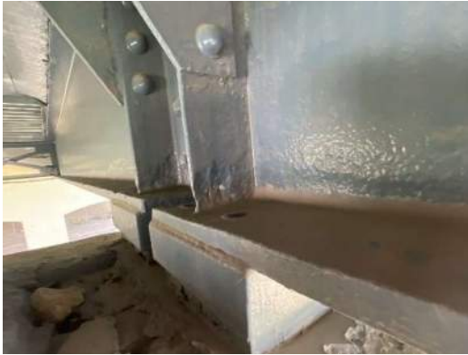
Photo 8E-001: Painted over pitting on throughout S9 at pier 8E, looking southeast
