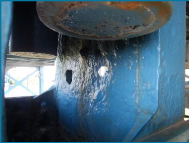
Photo 64 – 3/16" deep pitting with perforations up to 2 1/2" diameter through the north channel of the south column at Pier E (looking northwest).
