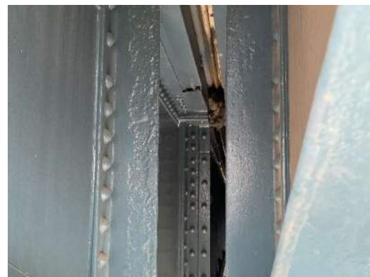
Photo 4E-012: Painted over pitting on transverse stiffener opposite of RS1 on east face of FB4, looking north
