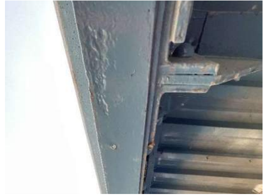
Photo 1E-006: Minor corrosion and painted over pitting of bottom flange angle of LS2 at intermediate channel bracket between FB2 and FB3, looking east
