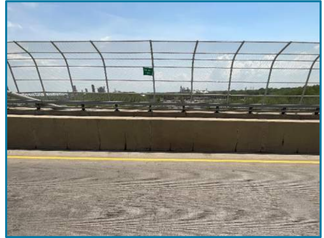
Photo 14 – Typical cracks with rust staining at 3' spacing, (looking south at the north face in Span RW-1).
