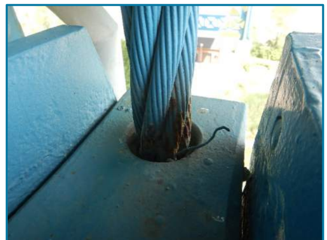
Photo 59 – Broken wire at southeast suspender cable of South Suspender Cable 0 (looking east).
