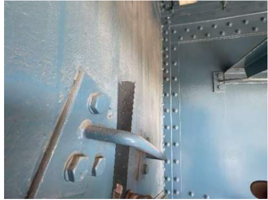
Photo 5W-002: Minor bowing to FB0, between RS1 and RS2
