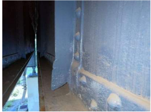
Photo 7E-002: 100% section loss to stiffeners 6 and 7 on west face of FB0, at bottom flange, between S4 and S5, looking north
