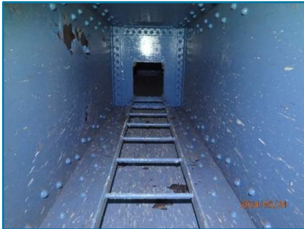
Photo 68 – Typical paint condition and paint flaking of the center cell of Tower D in the north leg (looking north).
