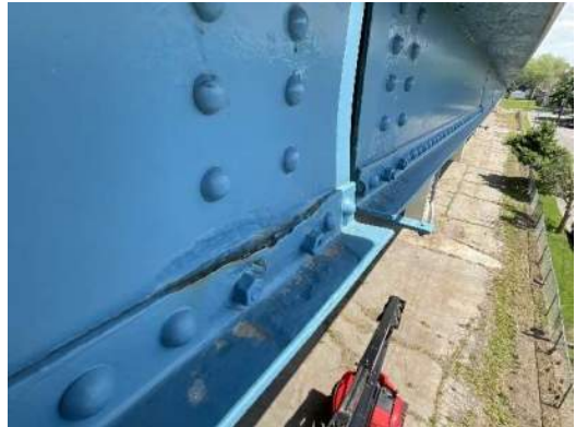
Photo 1E-010: Pack rust and painted over section loss of RS2 at FB4 overhang, looking east
