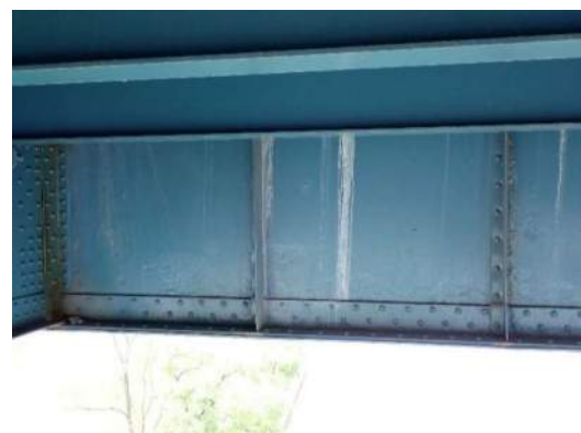
Photo MS-089: Pitting (1/8" deep) throughout web and flanges of Right Girder north face, west of FB50, looking south
