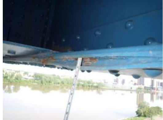
Photo ES-010: Pack rust between bottom flange plates on Left Girder, between FB58 and FB59
