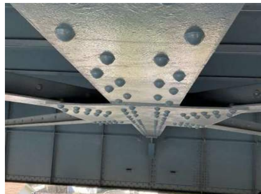
Photo 6E-004: Pack rust and bowing in lateral bracing connection plate on west side of FB1, at S4
