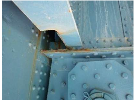
Photo ES-002: Pack rust (up to 1/2" thick) between bottom flange plates at Left Girder and FB53
