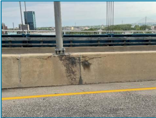
Photo 13 – Longitudinal cracking and delamination under light pole in Main Suspension Span between Floorbeams 47 and 48 on the south face (looking north).
