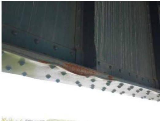
Photo WS-009: Pack rust between bottom flange plates on Left Girder between FB4 and FB5, looking northeast
