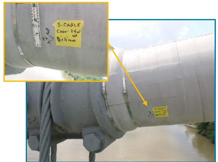
Photo 48 – Gouge in South Cable wrap at Suspender Cable 24 (looking south). Note there were not leaks associated with this gouge.
