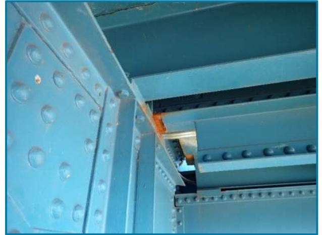
Photo 17 – Signs of expansion at the sidewalk stringers (looking north at Right Stringer 2 on at Floorbeam 12).
