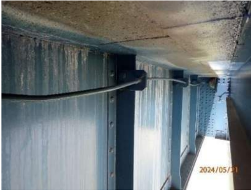
Photo MS-054: Offset handrail 2.5" high by full length, along Right Girder north face between FB36 and FB37, looking west
