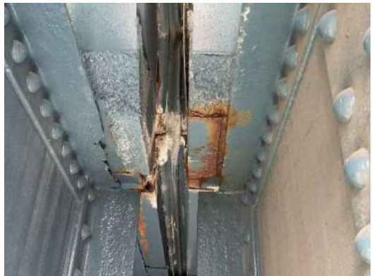
Photo 4E-004: Corrosion and efflorescence on top flange of RS1, top flange of FB0, and deck pan flashing, with rust staining, looking north
