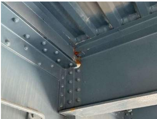
Photo 5E-011: Active corrosion to top flange of FB3 west face and top web of S4, dripping to bottom flange of S4, looking southeast
