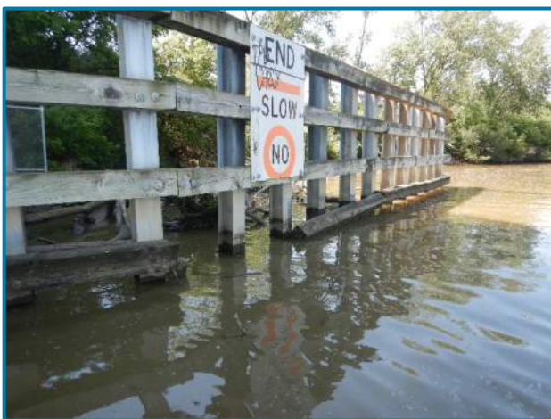
Photo 83 – Missing timber waler at Tower C pier and one waler with several missing fasteners (looking northwest).
