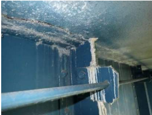
Photo MS-062: Efflorescence staining on north face of Right Girder, west of FB 41, looking southwest
