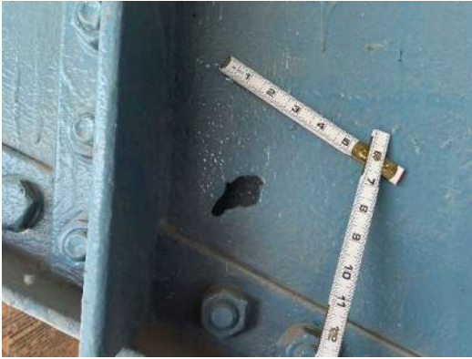
Photo 5W-001: 100% section loss and painted over pitting throughout east face web of FB0, between RS1 and RS2
