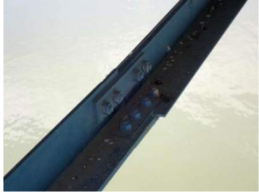
Photo MS-038: Bolted repair in lower lateral bracing near FB32 under S6
