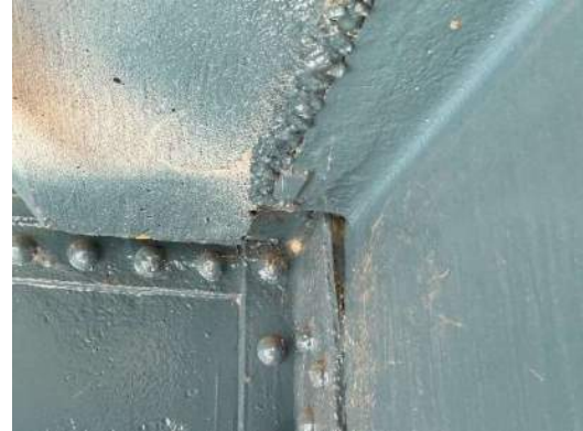
Photo 3E-004: Painted over pitting and pack rust on top of stringer RS2 at connection to FB2
