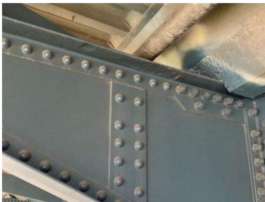
Photo 7W-005: Painted over pitting on top flange of FB2 north overhang, near LS1, looking west
