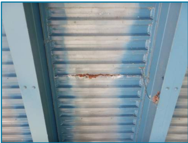
Photo 3 – Isolated corrosion of the stay-in-place forms and minor efflorescence between Beams 4 and 5 in Span 1W (looking east).
