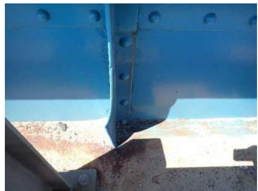
Photo MS-095: Impact damage on 3 stiffeners on Left Girder, between FB51 and FB52, looking north at center stiffener
