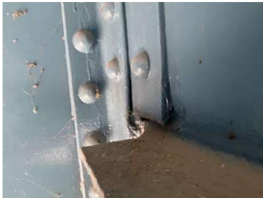
Photo 2E-003: Painted over pack rust between stringer web and angle connection, causing bowing, on S4 at connection to FB2, looking southeast
