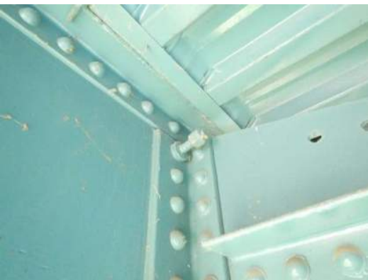
Photo 4W-005: Bolt backed off 2" at the LS2 and FB4 connection, looking northwest
