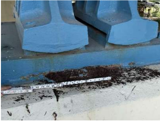
Photo 5E-013: Active area of minor corrosion on south side of masonry plate at south bearing on pier 5E, looking north
