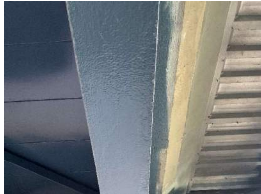
Photo 12E-002: Painted over section loss on bottom flange of S2, just east of pier 11E, looking north
