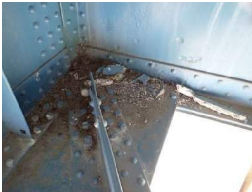
Photo MS-064: Granular and bird debris on lower lateral connection plate at Right Girder and west face of FB41, looking southeast
