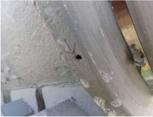
Photo SC-001: Main cable at suspender cable 2, leak, east end, north face
