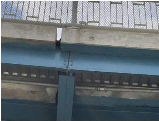
Photo 8W-001: Typical connection painted over section loss on north face of S1 at midspan sidewalk bracket, looking south
