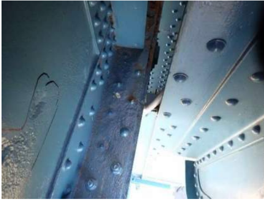
Photo MS-001: Rivet heads up to 100% section loss on north face of Left Girder bottom flange east of FB13, looking southwest
