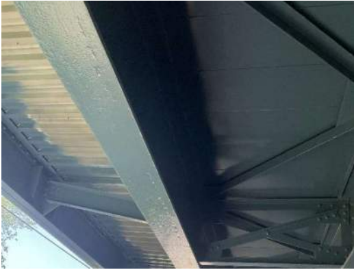
Photo 11E-001: Painted over section loss along S12
