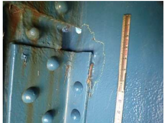
Photo MS-075: Pitting on web of Right Girder north face, west of FB45, looking southeast
