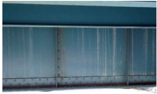
Photo MS-032: Pack rust (up to 3/4" thick) between north edge of bottom flange plates on Right Girder, between FB28 and FB29, looking south
