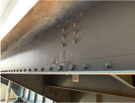
Photo 7W-007: Painted over pitting on south face of RS2, near FB2, looking northwest
