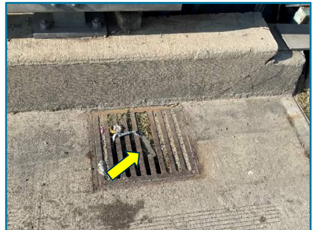
Photo 15 – Broken and partially clogged drainage grate at Pier B, West Suspension Span along the south curb (looking south).
