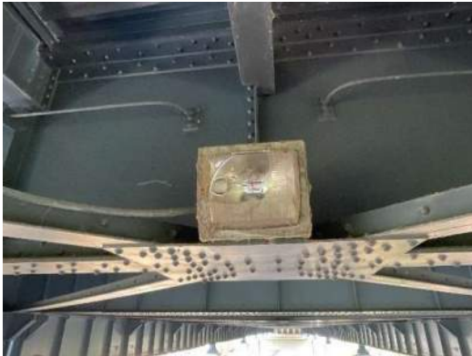
Photo 7E-003: Broken light under bridge at S4 and FB1 connection
