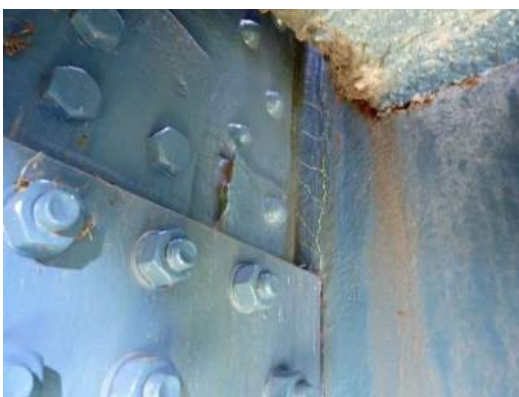
Photo MS-082: Pitting (3/16" deep by 2" wide by 24" high) in web of Right Girder west face of FB48, looking southeast and up
