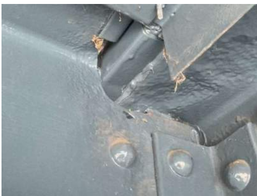
Photo 4E-005: 100% section loss on top of S1 web near at cope, at FB2
