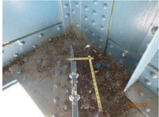
Photo MS-049: Pack rust (3/4" thick) between web angles of lower lateral bracing at connection plate, east of FB35, at Right Girder, looking southwest
