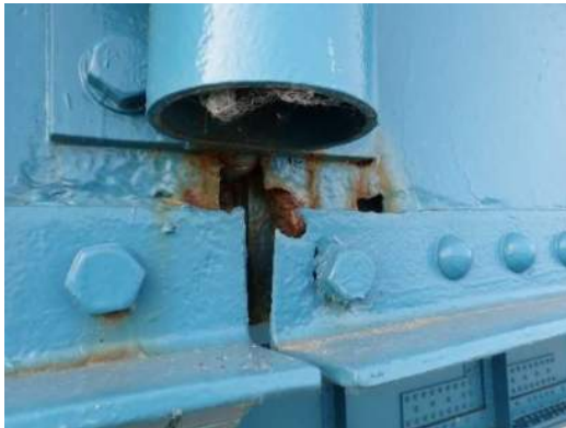
Photo ES-009: Pack rust (1" thick) and pitting (1/8" deep) with areas of 100% section loss at LS2 and FB58 connection
