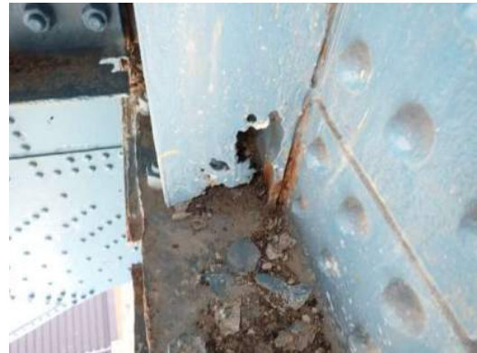
Photo MS-004: 100% section loss to transverse stiffener on Left Girder near FB13
