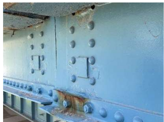
Photo 6E-006: Active corrosion and section loss on bottom flange angle and web of LS2, at FB4 north overhang, looking southeast
