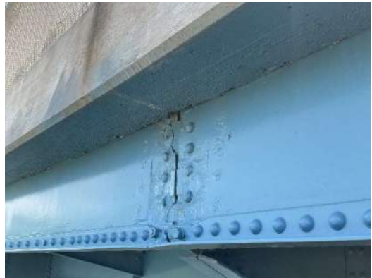
Photo 1E-008: Pack rust and painted over section loss of LS2 at FB3 overhang, looking southeast
