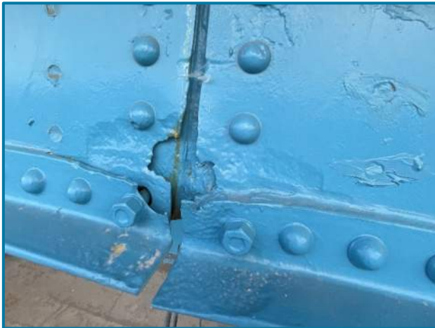
Photo 28 – Typical advanced section loss to the bottom flange angle and web plate at the cantilever sidewalk brackets (looking north at Right Stringer 2 at Floorbeam 2 in Span 4E).
