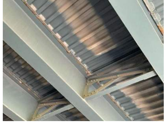
Photo 10E-002: Typical active corrosion along top flange for 50% length of stringers, shown along S9
