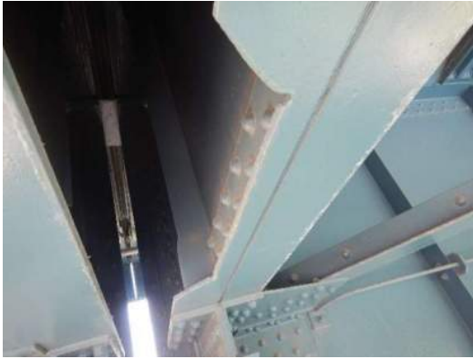
Photo 4W-001: Coped bottom flange (13" length) on FB0 near Left Girder, looking northwest
