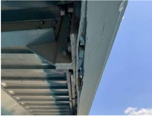
Photo 5E-007: Pack rust and painted over section loss on RS2 at intermediate overhang brace between FB1 and FB2, looking east
