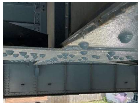
Photo 5E-012: Pack rust and bowing of lateral bracing connection plate and bottom flange of FB3, with sporadic, active corrosion to bottom flange cover plate FB3 west face
