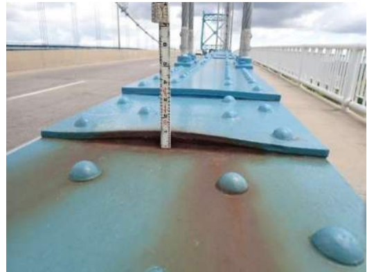
Photo MS-014: 3/4" thick pack rust between top flange plate and cover plate on Right Girder between FB17 and FB18
