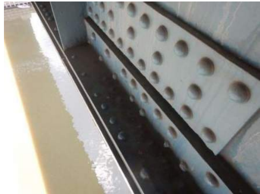
Photo MS-026: Rivet heads with up to 100% section loss on bottom flange of Left Girder, south face, between FB27 and FB28, looking northwest
