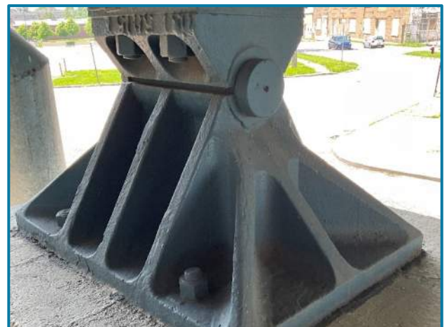
Photo 45 – Right Girder fixed bearing at Pier 7W (looking southwest).
