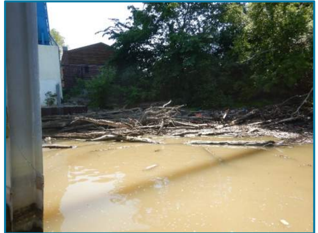
Photo 85 – Debris accumulation behind the north end of pier protection at Tower C (looking west).
