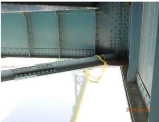
Photo MS-046: Bolted repair on lower lateral bracing on west side of FB35 at Right Girder, looking east
