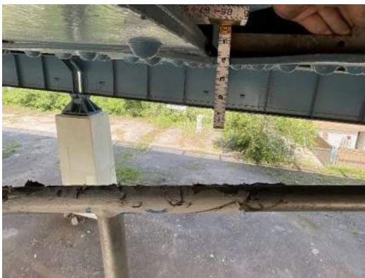
Photo 5E-005: Pack rust and bowing (up to 1/2") in connection plate for lateral bracing at bottom flange of FB1, at S4
