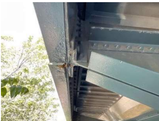
Photo 6E-005: Pack rust and painted over section loss of LS2, at FB2 north overhang, looking east
