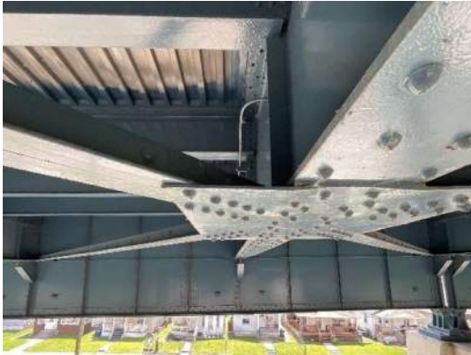
Photo 2E-001: Bowing on both sides of lateral bracing connection plate with painted over pack rust, at S4 and FB1 connection
