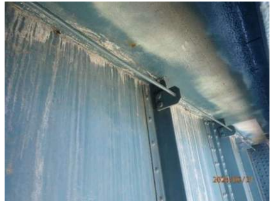
Photo MS-061: Efflorescence staining on north face web of Right Girder, between FB39 and FB40, looking southwest
