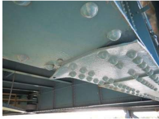
Photo WS-008: Section loss (3" wide by 1/4" deep) on bottom flange of Right Girder between FB3 and FB4
