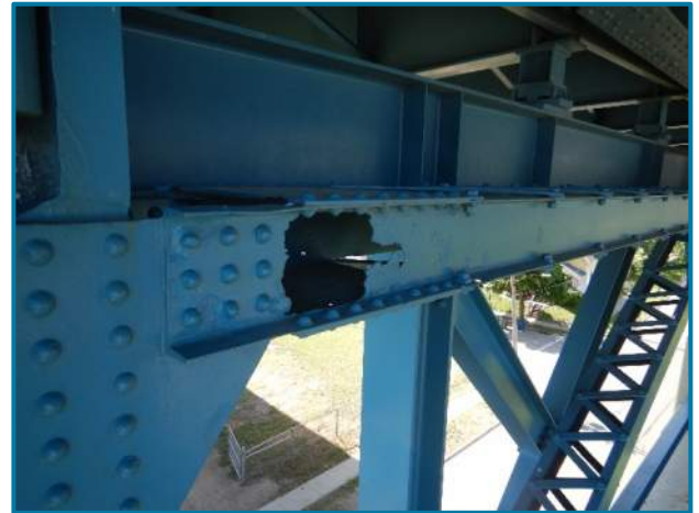
Photo 65 – Numerous corrosion holes through the upper strut at Pier E near the north column (looking southeast).
