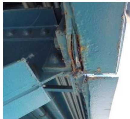
Photo ES-006: Pack rust (1" thick) and pitting (1/8" deep) at connection between LS2 and FB54
