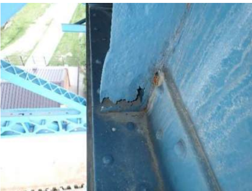
Photo MS-011: 100% section loss (3" high by full width) to transverse stiffener at bottom flange of Left Girder between FB14 and FB15, looking northwest
