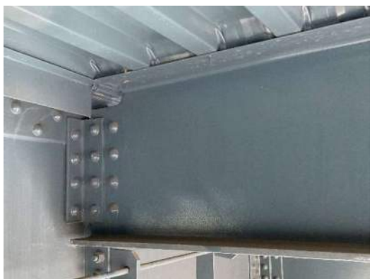
Photo 5E-006: Unpainted area (1 1/2' long by 4" high) with primer exposed on web of S7, west of FB2
