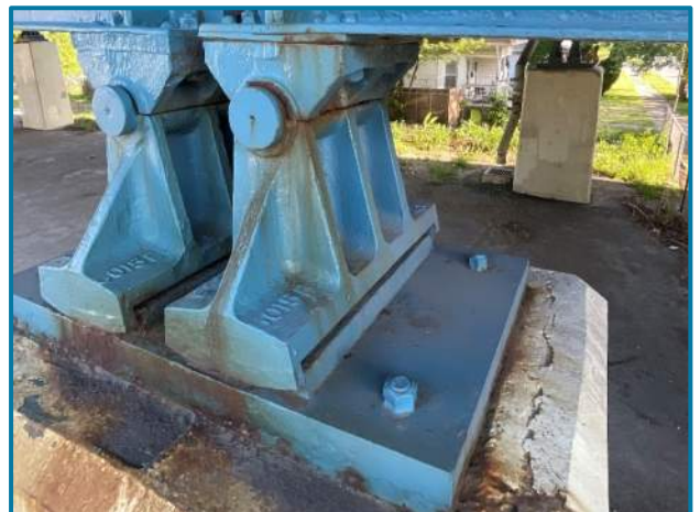
Photo 40 – Right Girder rocker bearing at Pier 6E (looking north).
