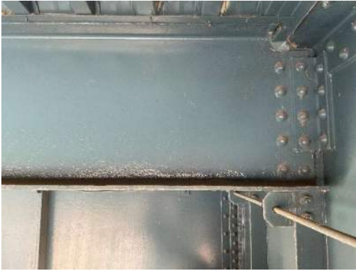
Photo 5W-007: Painted over pitting on south face web of S1, at FB2, looking north
