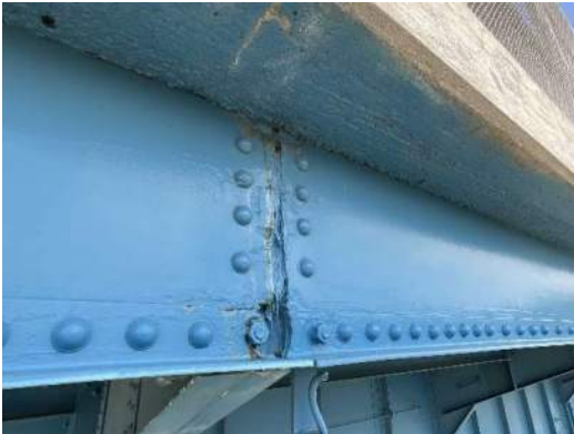
Photo 1E-003: Pack rust and painted over section loss of RS2 at FB1 overhang, looking northeast
