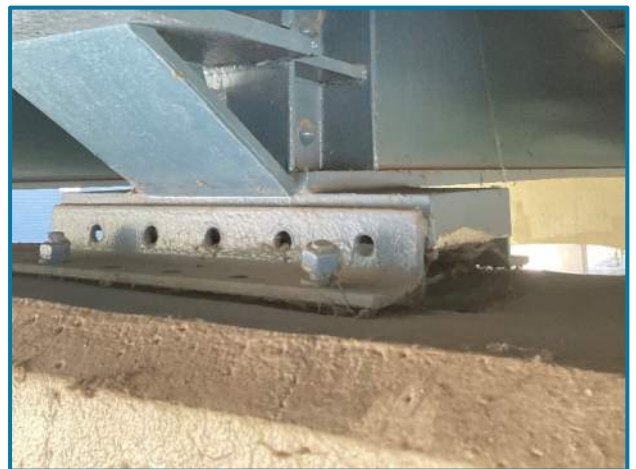
Photo 38 – Backed off northeast anchor rod nut of Beam 11 at Pier 12E (looking southwest).
