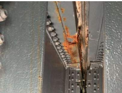
Photo 6E-011: Active corrosion and efflorescence at top flange FB4 and deck pan flashing, on south overhang
