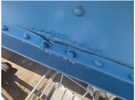
Photo 6E-010: Painted over corrosion and section loss on bottom flange angle and web of RS2, at intermediate bracket south overhang, between FB3 and FB4, looking north
