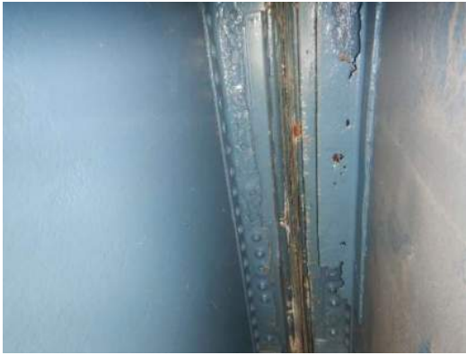
Photo 3W-007: 100% section loss throughout flanges and stiffeners on FB5 at north cantilever, looking up and south
