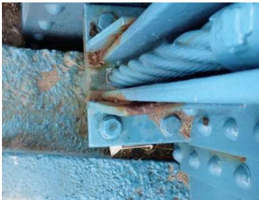
Photo MS-076: Pack rust between bearing and connection angles of Suspenders Cable 44 connection to Right Girder
