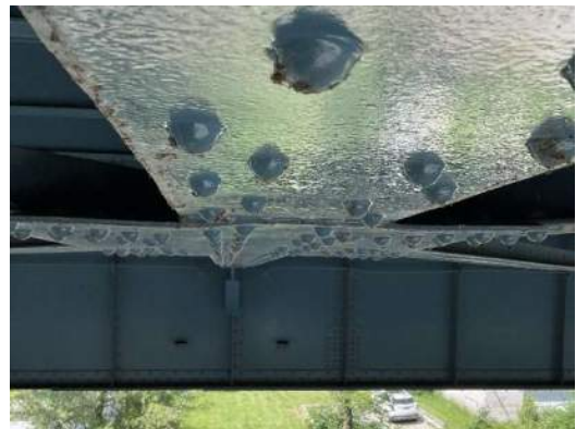
Photo 3E-006: Pack rust and minor bowing between bottom flange of FB1 and lower lateral connection plate at S4
