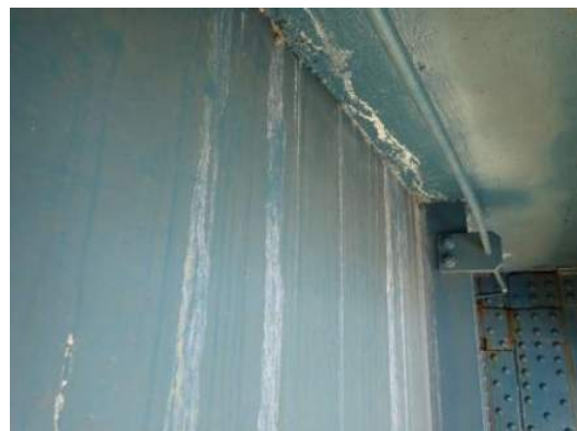
Photo MS-024: Typical efflorescence staining on north face of Right Girder, between FB26 and FB27, looking southwest
