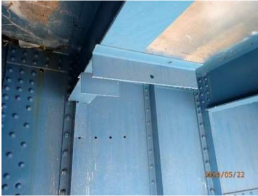
Photo MS-007: Stray angles welded longitudinally along S11 bottom flange on east side of FB13, looking northwest
