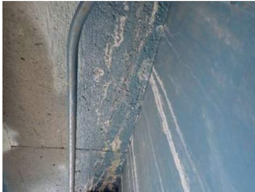
Photo MS-096: Efflorescence staining on south face of Left Girder web near FB51, looking west
