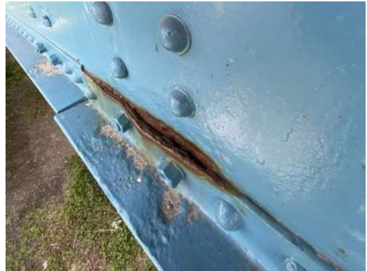
Photo 5E-010: Pack rust and painted over section loss on LS2 at FB4 overhang, looking southeast
