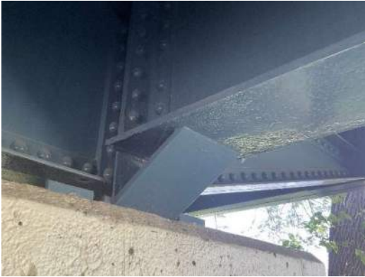
Photo 13E-001: Painted over section loss on S2, west end, looking northwest
