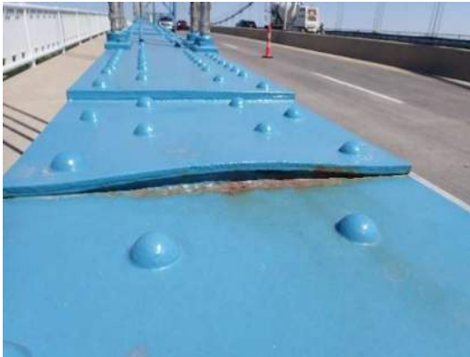
Photo MS-013: 12" wide by 3/4" thick pack rust between top flange and cover plate on Left Girder between FB16 and FB17, looking east
