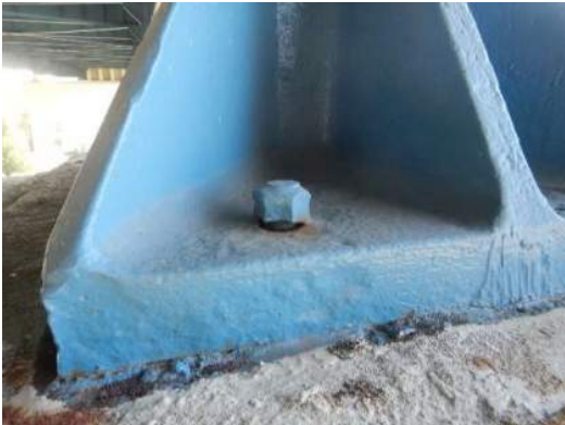
Photo 4W-009: Up to 50% section loss in northwest anchor rod of pier 3W Right Girder bearing, looking southeast
