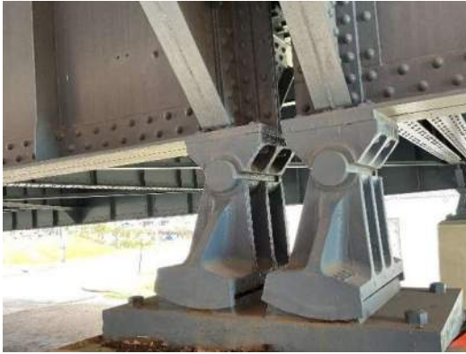
Photo 6W-001: Bearing tilted 10 degrees to the east at Pier 6W south bearing, looking north
