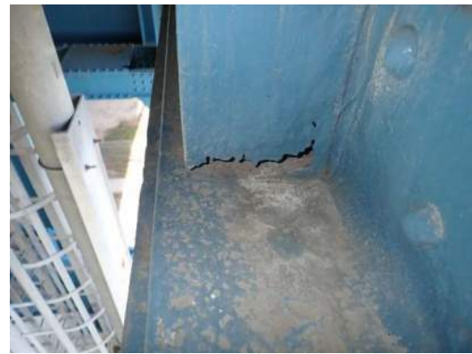
Photo ES-024: 100% section loss on transverse stiffeners on Right Girder, between FB64 and FB65
