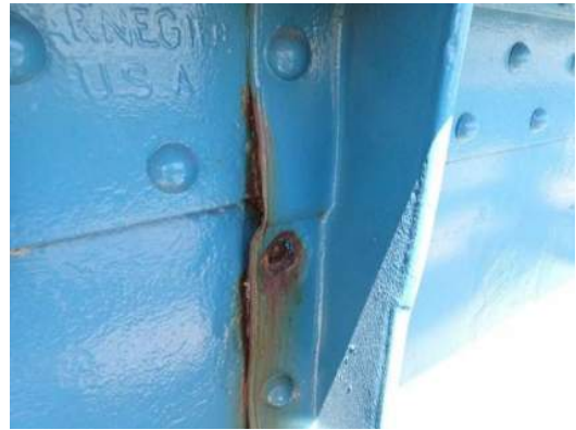
Photo WS-002: Punched hole with missing rivet at transverse stiffener on Left Girder south face east of FB0, looking northeast
