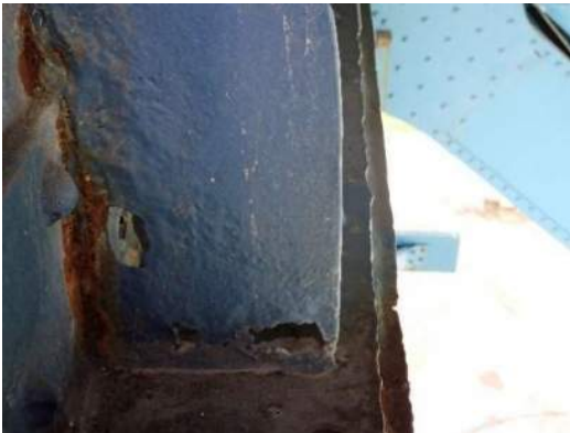
Photo MS-098: 100% section loss (up to 2" diameter) on transverse stiffener on south face of Left Girder, east of FB51, looking east
