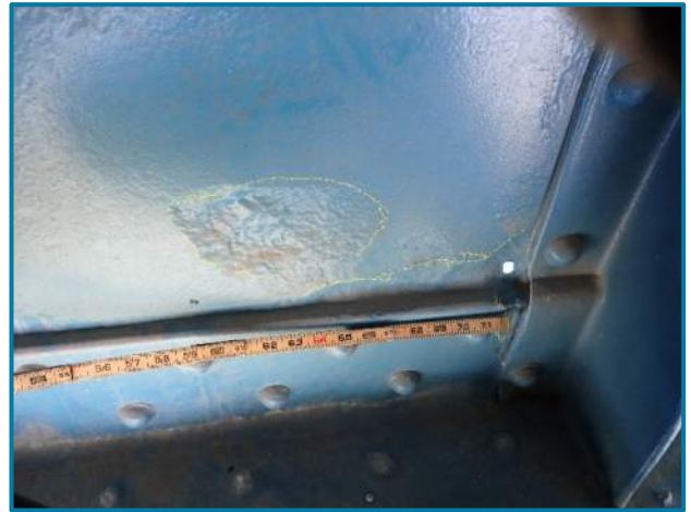
Photo 21 – 1/4" deep web pitting with 1/2" diameter corrosion hole through Right Girder in Main Suspension Span between Floorbeams 42 and 43 (looking south).
