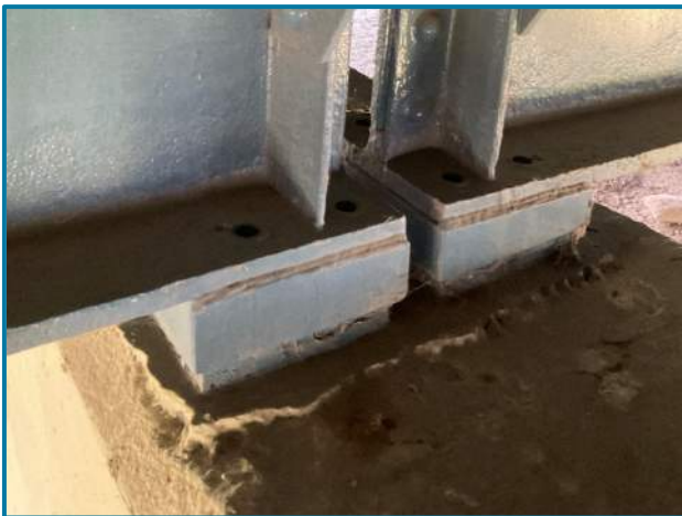
Photo 39 – Typical bearing retrofitted with an elastomeric bearing pad during a previous rehabilitation project (looking northeast)
