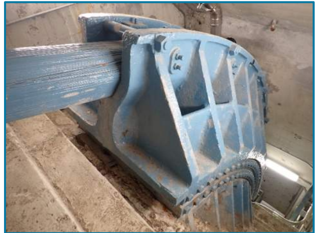
Photo 50 – North Cable saddle in Anchorage A (looking southwest).
