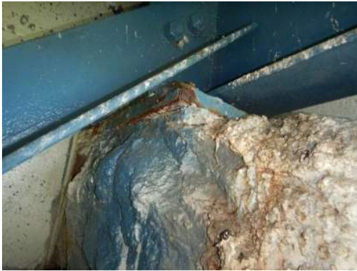
Photo RW-2-001: Spall undermining masonry plate (6" long by 1/2" deep) at anchorage A S1 bearing, looking northwest
