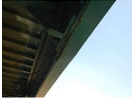
Photo 4W-002: 1/2" thick pack rust between sidewalk cantilever connection on LS2 between FB1 and FB2, looking northeast
