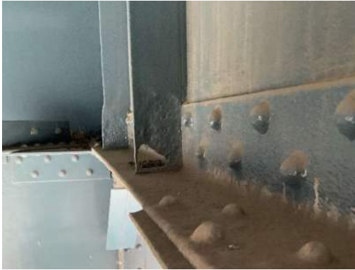
Photo 4E-007: 100% section loss in transverse stiffener on west face of FB2, between S3 and S4
