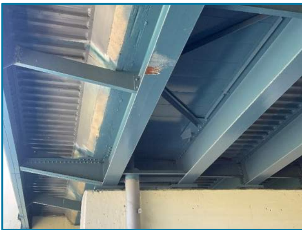
Photo 26 – Minor impact scrapes and surface corrosion of Girder S2 in Span 14E (looking east).
