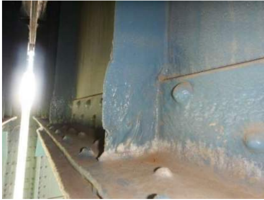
Photo 4W-007: Painted over section loss with caulking at stiffener base on east face of FB4 near S4, looking northwest
