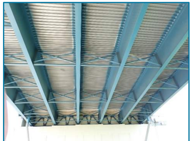
Photo 36 – Typical condition of steel protective coating, Span RW-2 (looking west).
