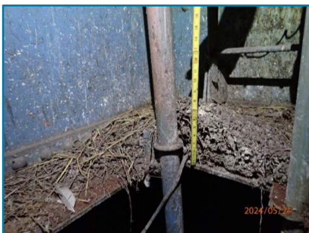
Photo 72 – Heavy accumulation of bird debris in the center cell of Tower D in the south leg, 2nd segment from the top (looking southeast).
