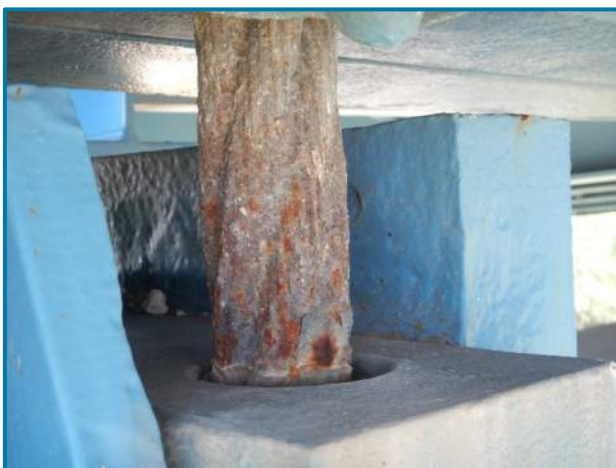
Photo 58 – Corrosion of strand at southwest suspender cable of North Suspender Cable 65 (looking southwest).
