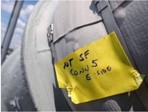
Photo NC-001: Main cable at suspender cable 5, leak, east end, south face
