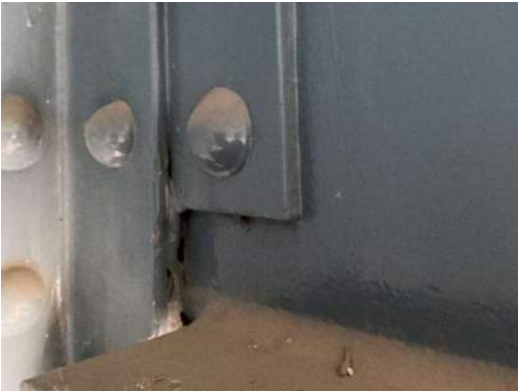
Photo 4E-009: Minor painted over pack rust between S1 web and vertical stiffener, at FB3
