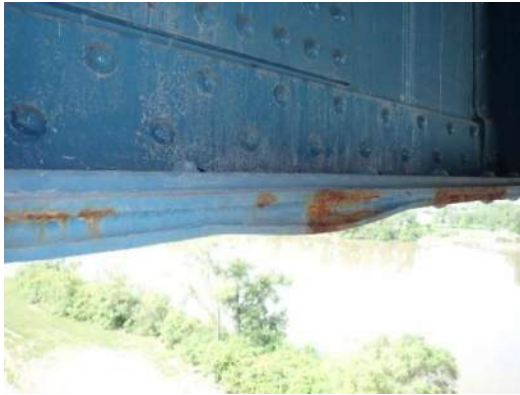
Photo ES-013: Pack rust between north face bottom flange plates of Right Girder, between FB59 and FB60
