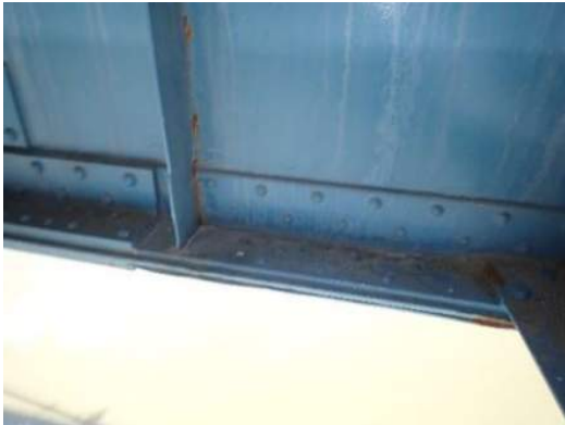
Photo MS-033: Pack rust between bottom flange and cover plate of Left Girder south face, between FB29 and FB30, section loss on transverse stiffener, looking north
