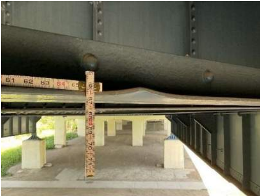
Photo 6E-009: Minor impact damage to angle of lateral bracing, near S7, between FB3 and FB4
