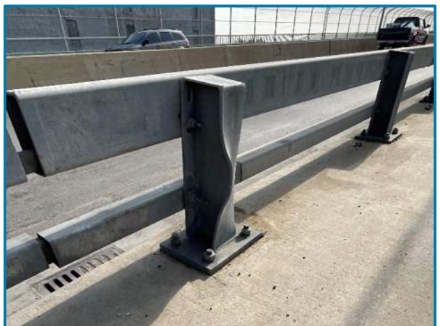
Photo 12 – Impact damage to south railing post in Span 7W at Pier 7W (looking northeast).
