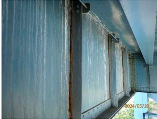
Photo MS-090: Efflorescence staining on southface of Left Girder, between FB49 and FB50, looking northeast
