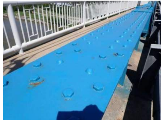
Photo MS-028: Isolated spots of peeling paint on top flange cover plate on Left Girder, between FB28 and FB29, looking northeast
