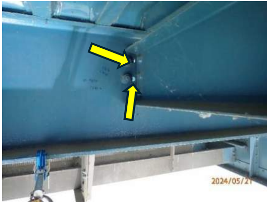
Photo MS-039: Two misdrilled holes in south face web of S8, between FB32 and FB33 at diaphragm, looking northeast
