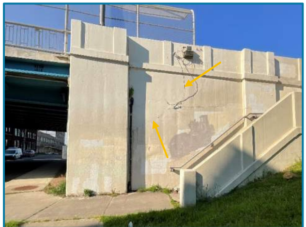
Photo 82 – 40'L horizontal crack and disconnected staircase light at the Rear Abutment North Retaining Wall (looking south).
