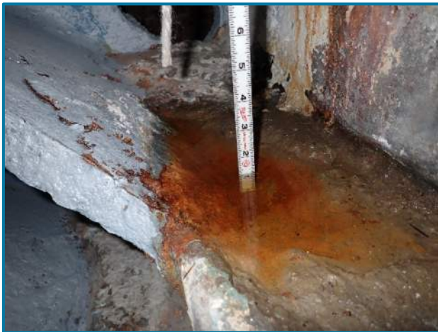
Photo 51 – Water ponding at South Cable saddle in Anchorage F (looking south).
