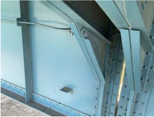
Photo 3E-001: 100% section loss and painted over corrosion to bottom angle of kneebrace on FB0 north overhang
