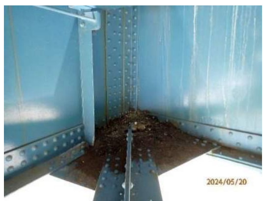
Photo MS-077: Dirt and debris on top of lateral bracing connection plate at Left Girder, east of FB47, looking northwest
