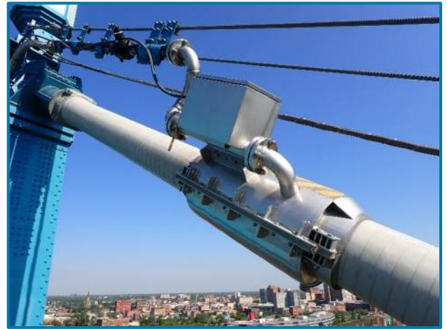
Photo 46 – Dehumidification system at North Cable east of Tower D (looking northwest).
