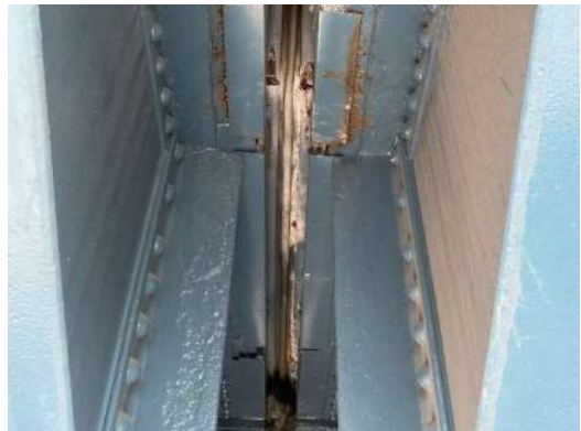
Photo 5E-004: Painted pitting on stiffeners and bottom flange of FB0 south overhang, active corrosion to top flange and deck pan flashing, with efflorescence, looking north
