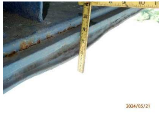
Photo MS-047: Pack rust (1 1/4" thick) between bottom flange plates on north face of Right Girder, between FB34 and FB35 at midspan, looking southwest
