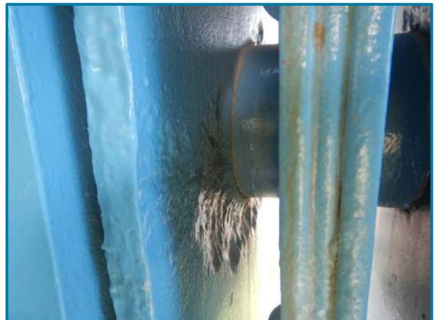
Photo 63 – 1/4" deep pitting on the inside face of south link plate of the north column at Pier E (looking west).
