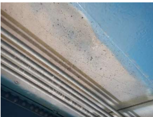
Photo MS-029: Hairline cracks (3' long by 5' wide) to underside of sidewalk, south overhang, east of FB28
