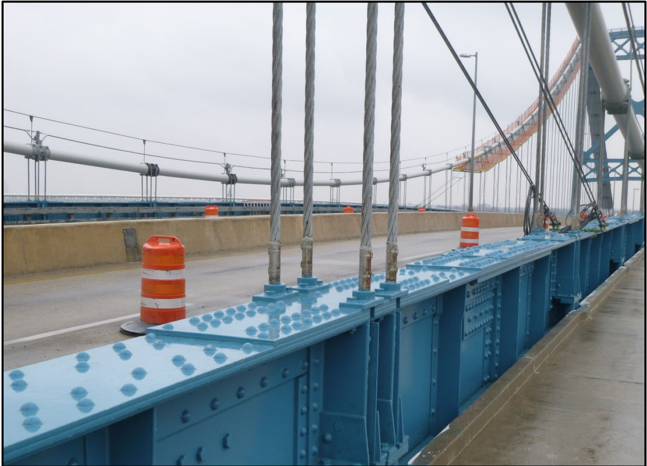
Photo 3 - Hanger Cable - Suspension Girder Connection
