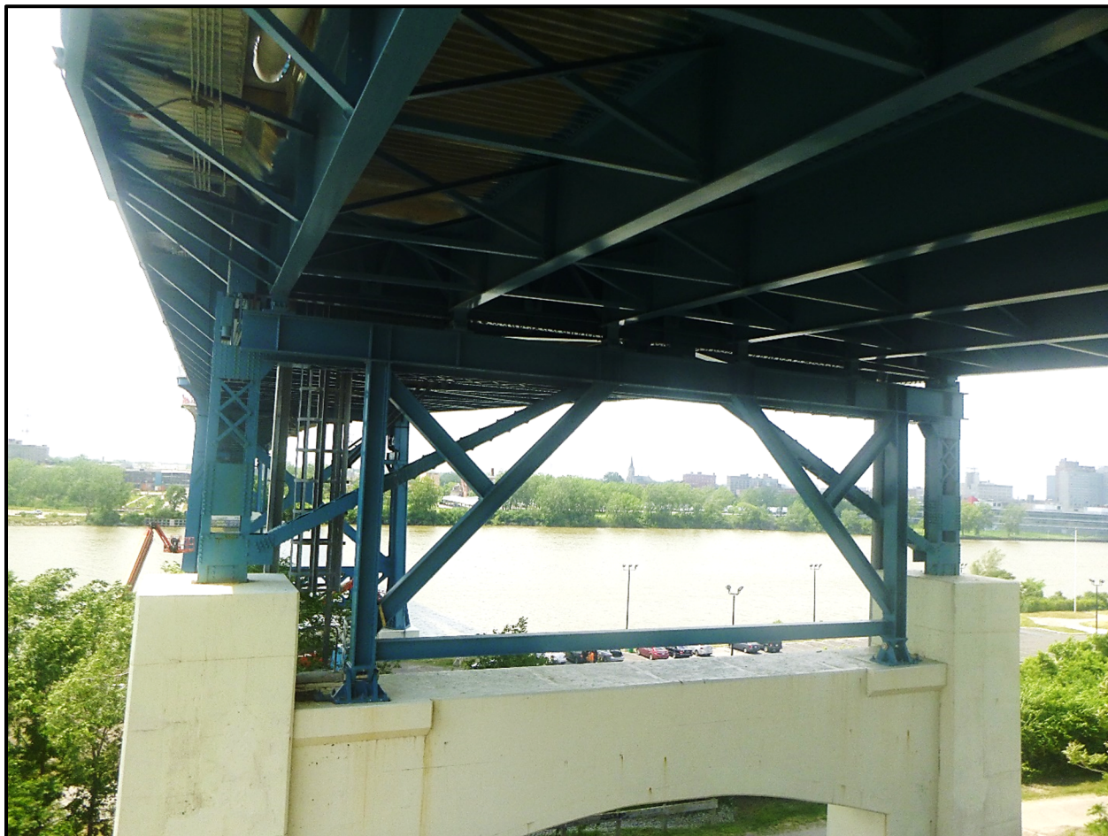
Photo 9 - Steel Frame Supporting New Replacement Span at Pier E (Frame at Pier B similar)
