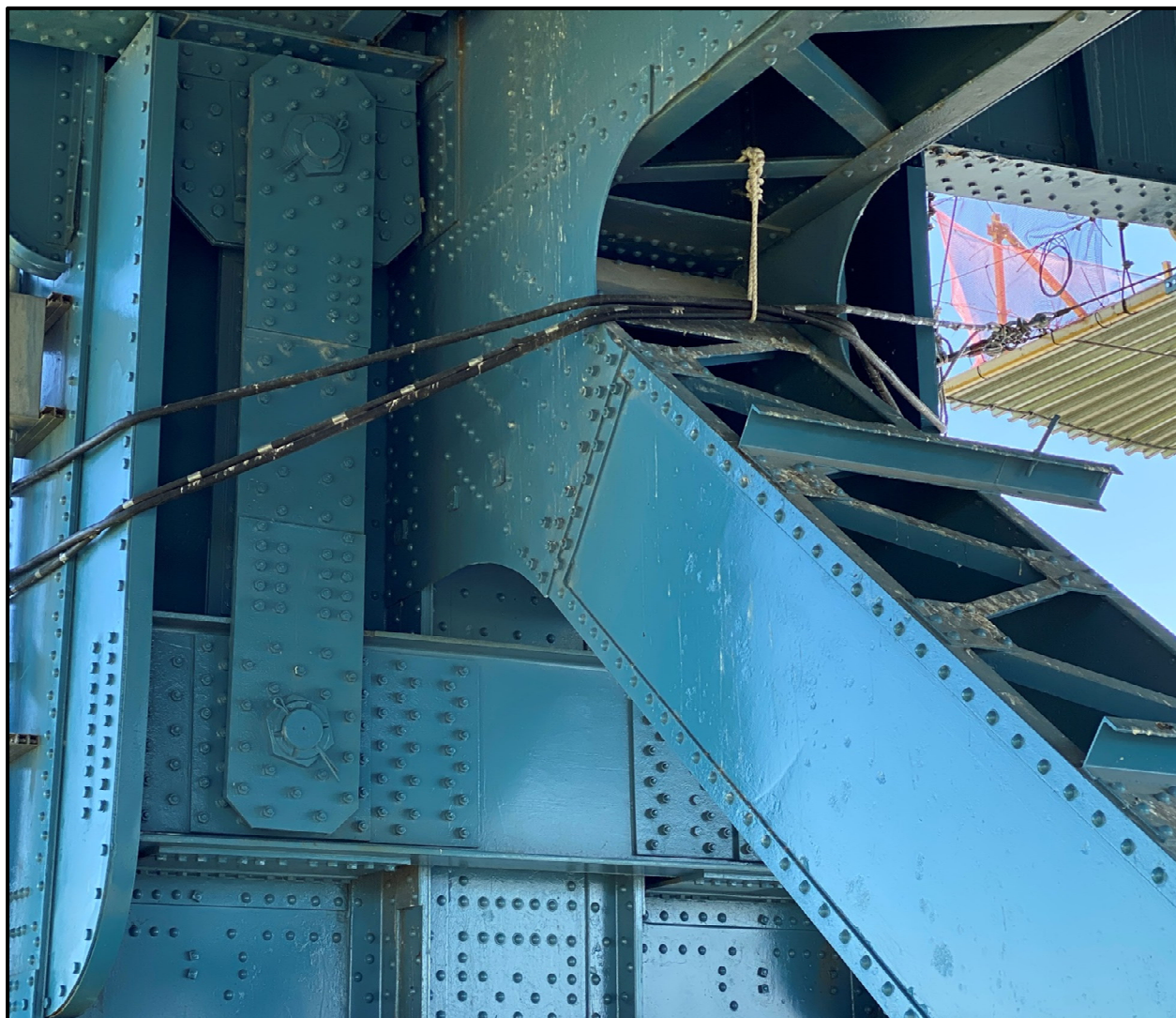
Photo 8 - Link Pins and Hangers at Tower C (Tower D similar)
