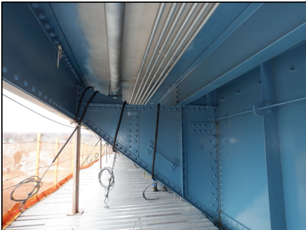
Photo 7 - Floor Beam Cantilever Supporting the Sidewalk
