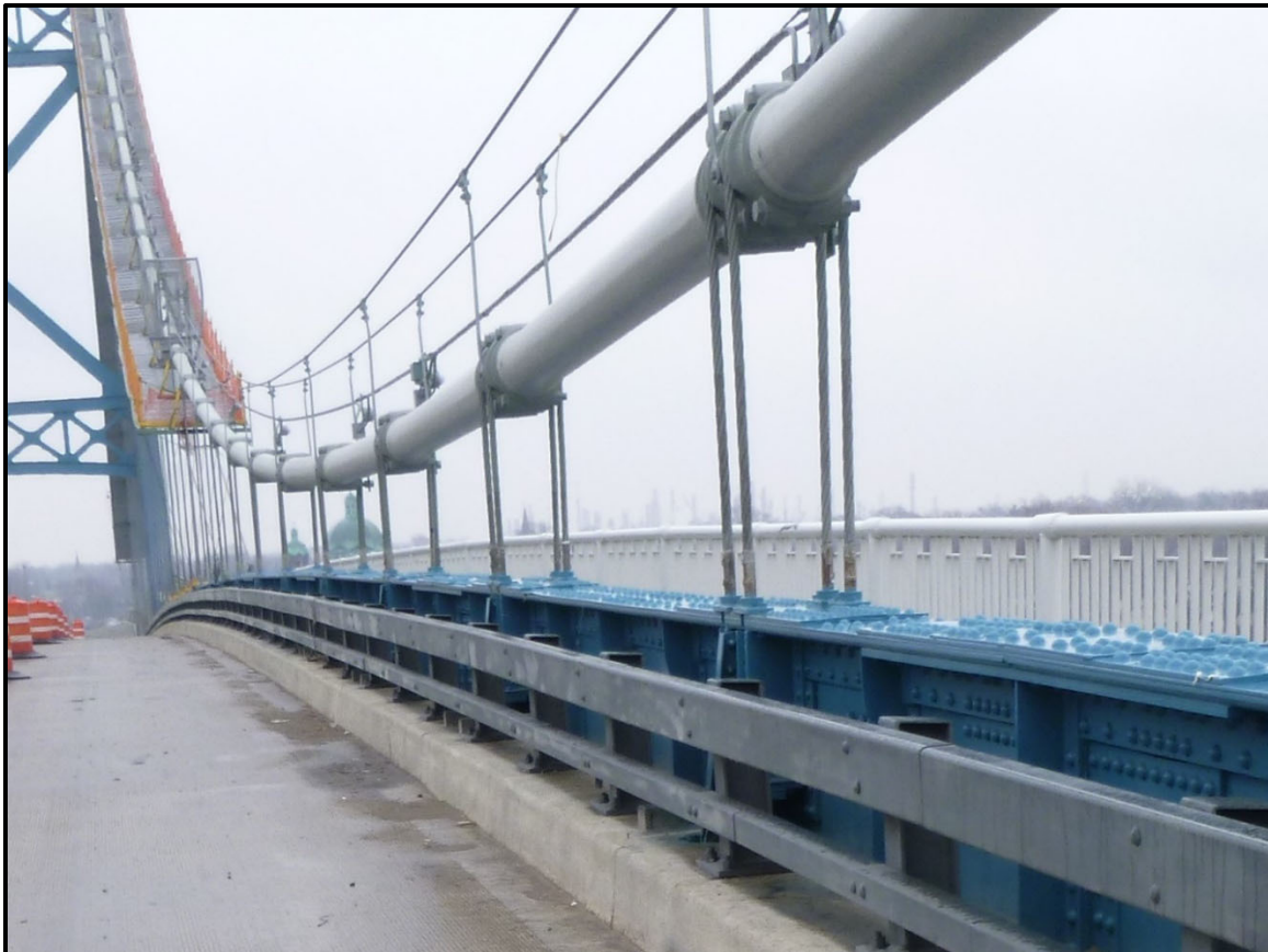
Photo 2 - Main Suspension Cables near Midspan
