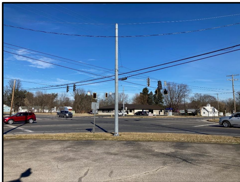
Image 1 - US 224 & SR 61 Signal from the Southwest Corner (February 2024)
