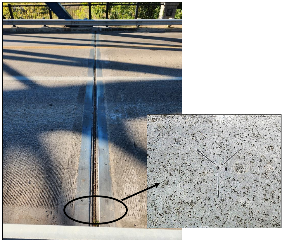
Picture 17: Rear expansion joint.
