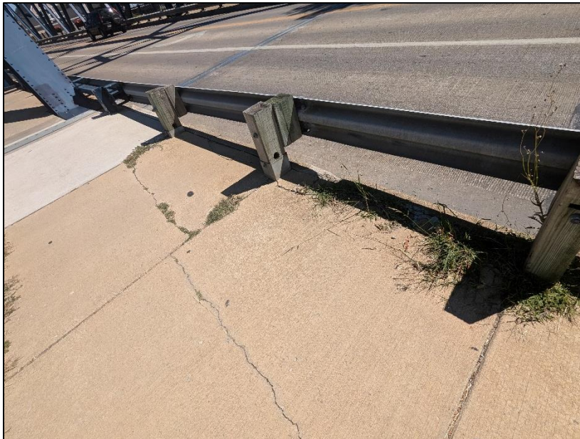
Picture 58: Approach sidewalk cracked at northwest corner.
