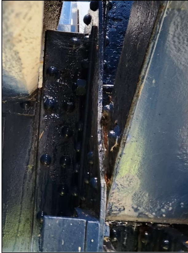
Picture 36: Pack rust bowing of L5 south truss inside gusset plate.
