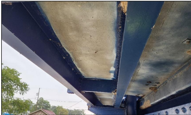
Picture 8: Typical sidewalk stringer condition.
