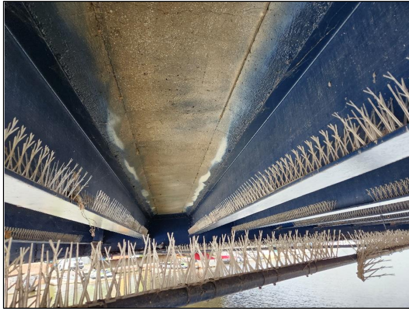
Picture 21: Pigeon spikes on floor system of Panel 8.
