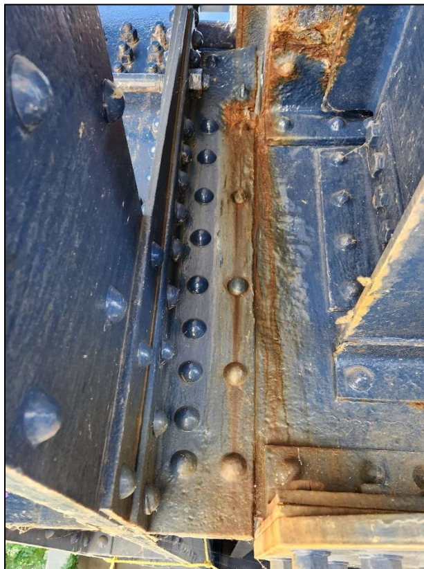
Picture 23: Floorbeam 1 south truss connection plate.
