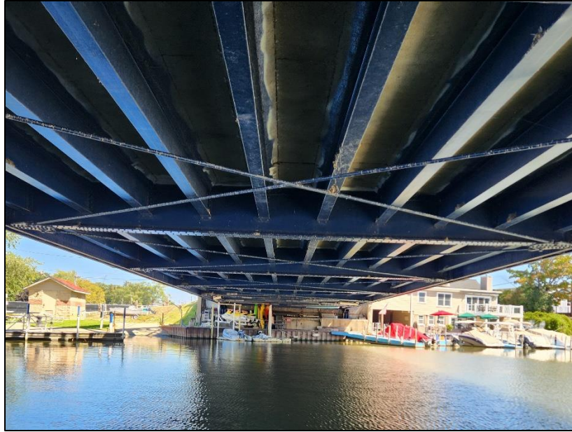
Picture 22: Typical floor system layout.
