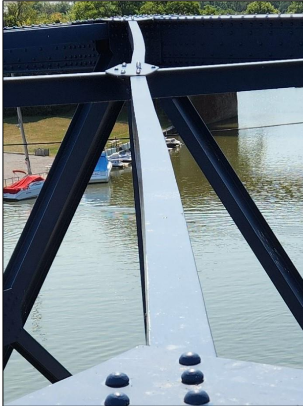
Picture 39: Looking at upper lateral bracing from U3N to U4S.
