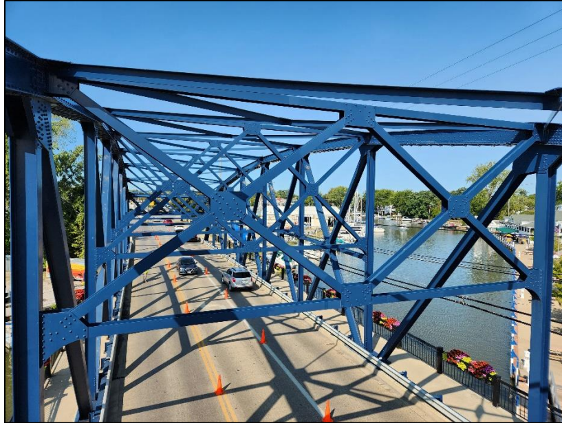
Picture 40: Sway bracing at PP7.
