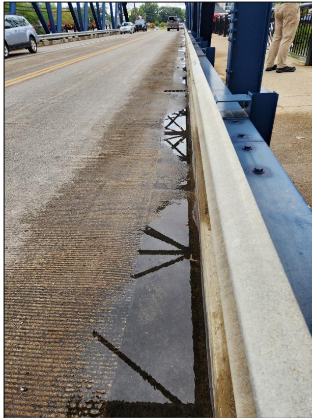
Picture 16: Ponding along south curb.
