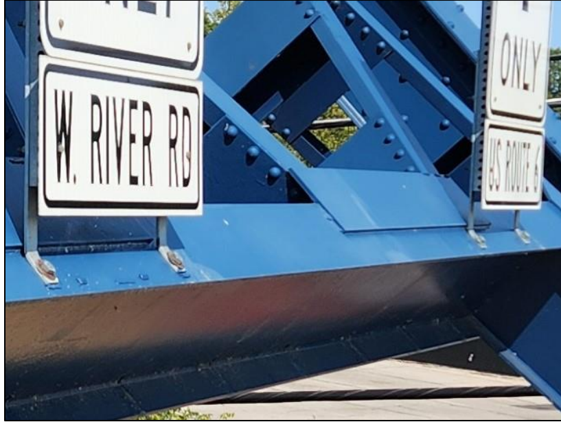
Picture 62: Lane sign support on east portal.
