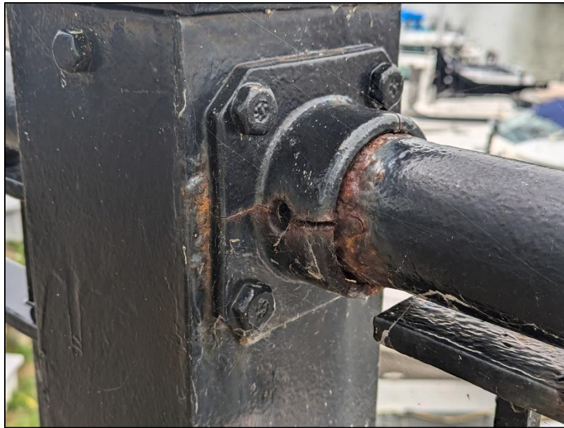
Picture 13: Broken connection plate.
