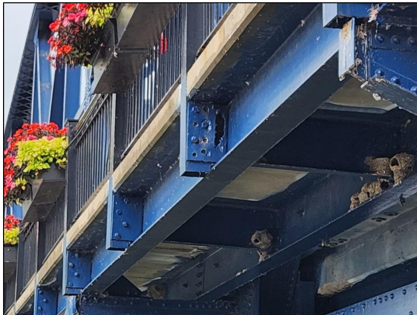
Picture 15: Hole in south truss pedestrian post connection between L6 and L7.
