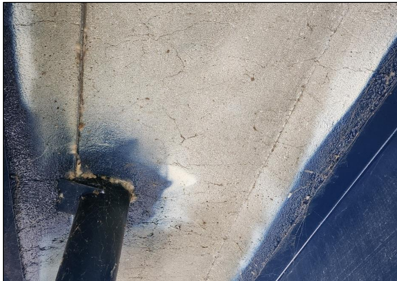
Picture 2: Typical map cracking around drainage pipe.
