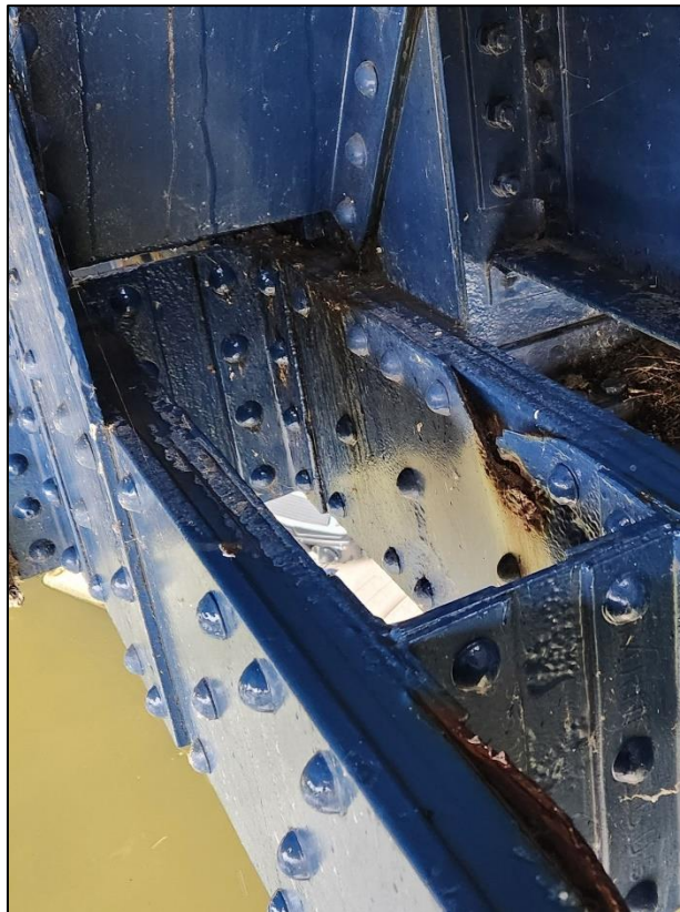
Picture 33: Hole in north inside plate of L3L4 at L3 of south truss.
