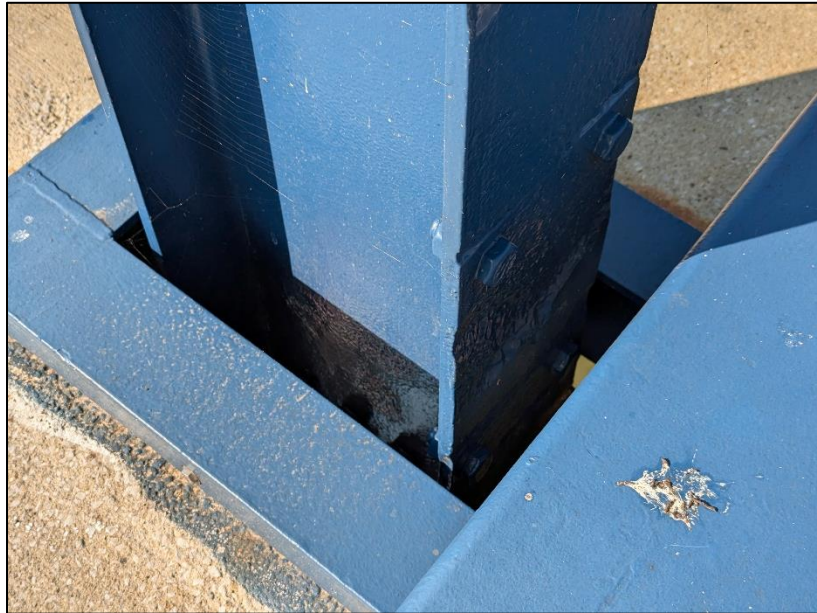
Picture 25: L8U8 of the south truss typical pitting in splash zone.
