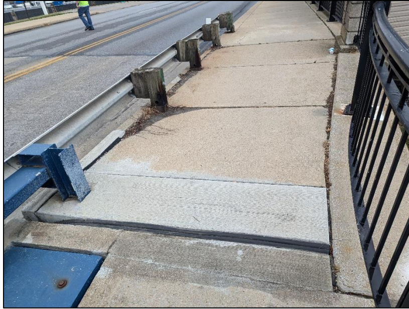
Picture 59: Southeast approach sidewalk settled.
