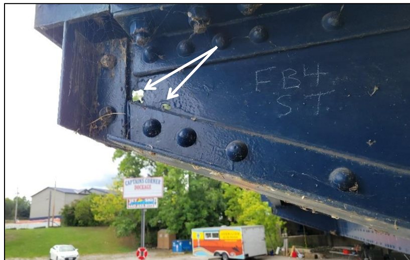
Picture 9: Looking west at hole in web of south cantilever bracket at L4.
