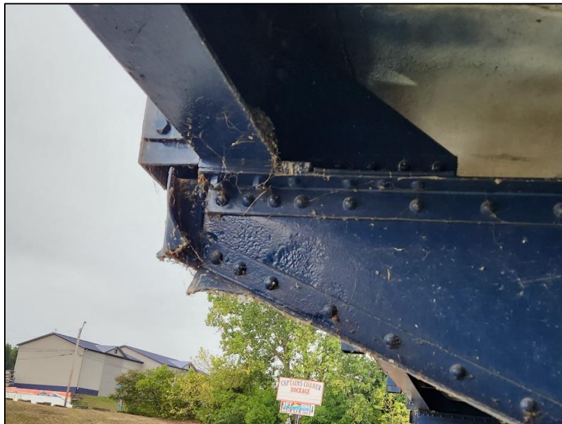
Picture 11: Bent south cantilever bracket.
