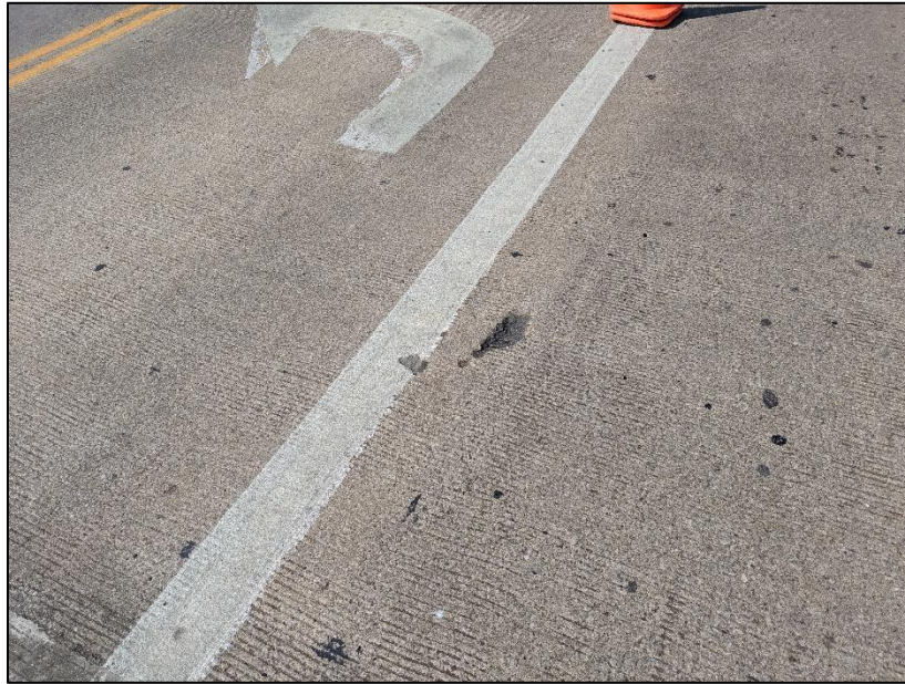
Picture 4: Small spall in wearing surface at east end.
