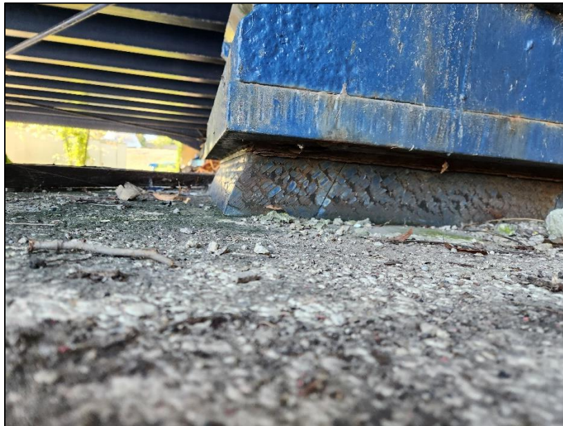
Picture 44: North elastomeric bearing on rear abutment.
