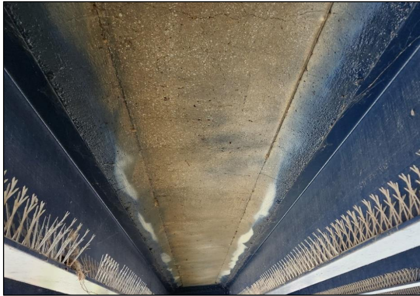
Picture 1: Typical map cracking in deck.
