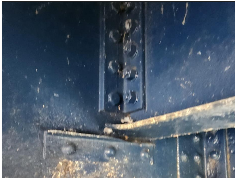
Picture 20: Typical bent stringer bottom flange.
