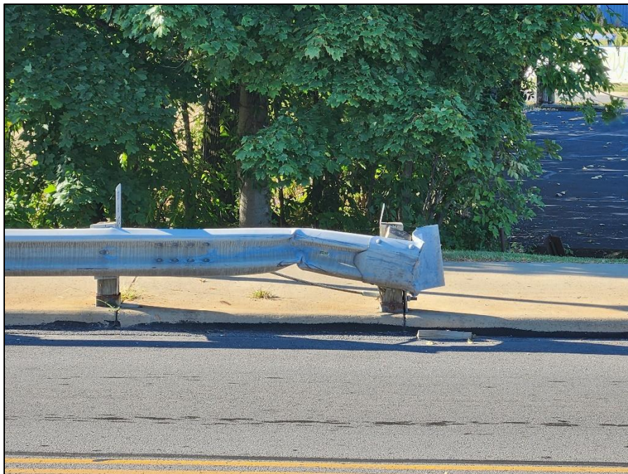
Picture 60: Impact damage at southwest corner.
