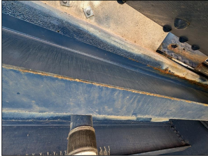
Picture 19: Rust along top and bottom flanges of Stringer 10 near The forward abutment.
