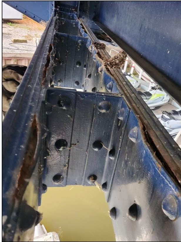
Picture 34: Pack rust in between plates of L3L4 of the south truss.
