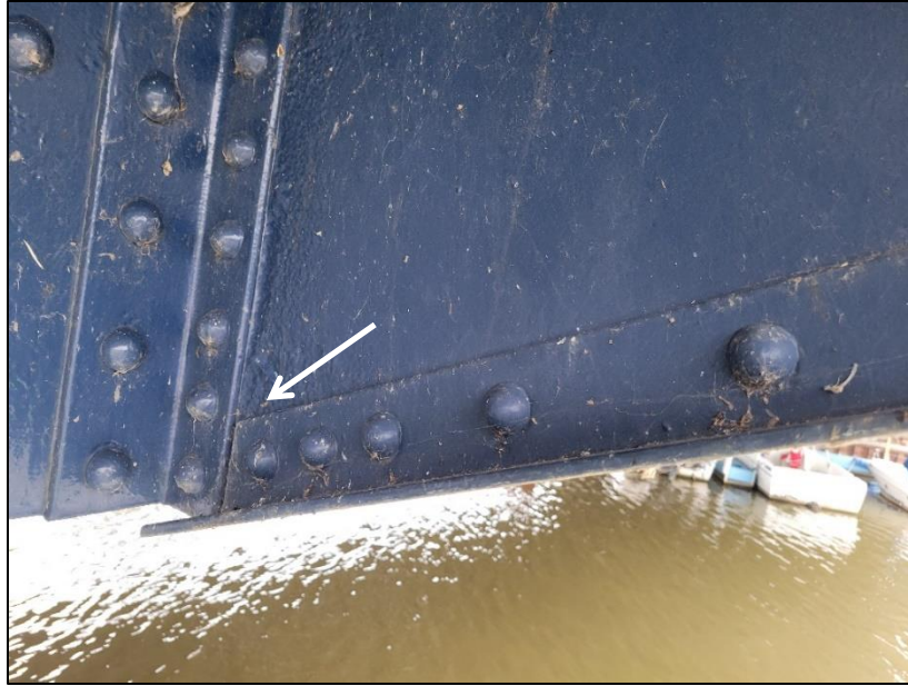
Picture 10: Looking east at pinholes in web of south cantilever bracket at L6.
