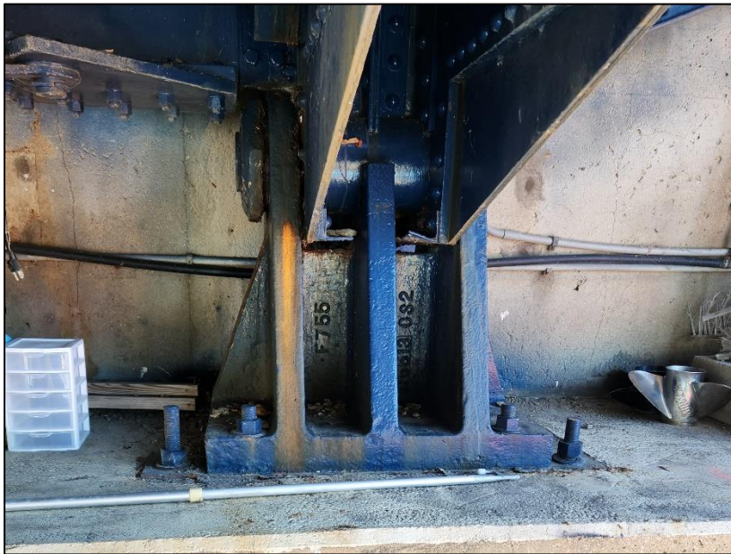
Picture 46: South bearing (bolster) on forward abutment.
