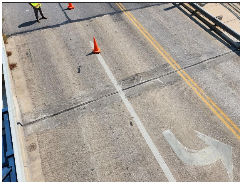
Picture 56: Forward approach slab.
