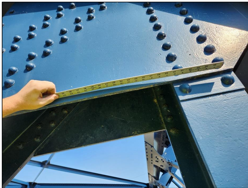
Picture 35: Misalignment bow of U8 south truss outside gusset plate.
