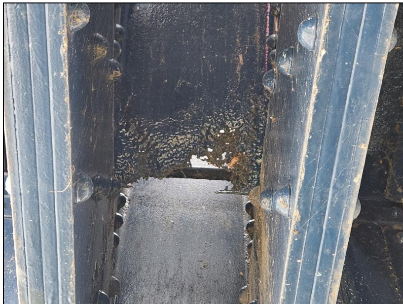
Picture 27: Reactivated pitting at the bottom of L7U8 of the south truss.
