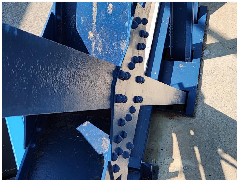
Picture 37: Bowing of M4.5 north truss inside gusset plate.
