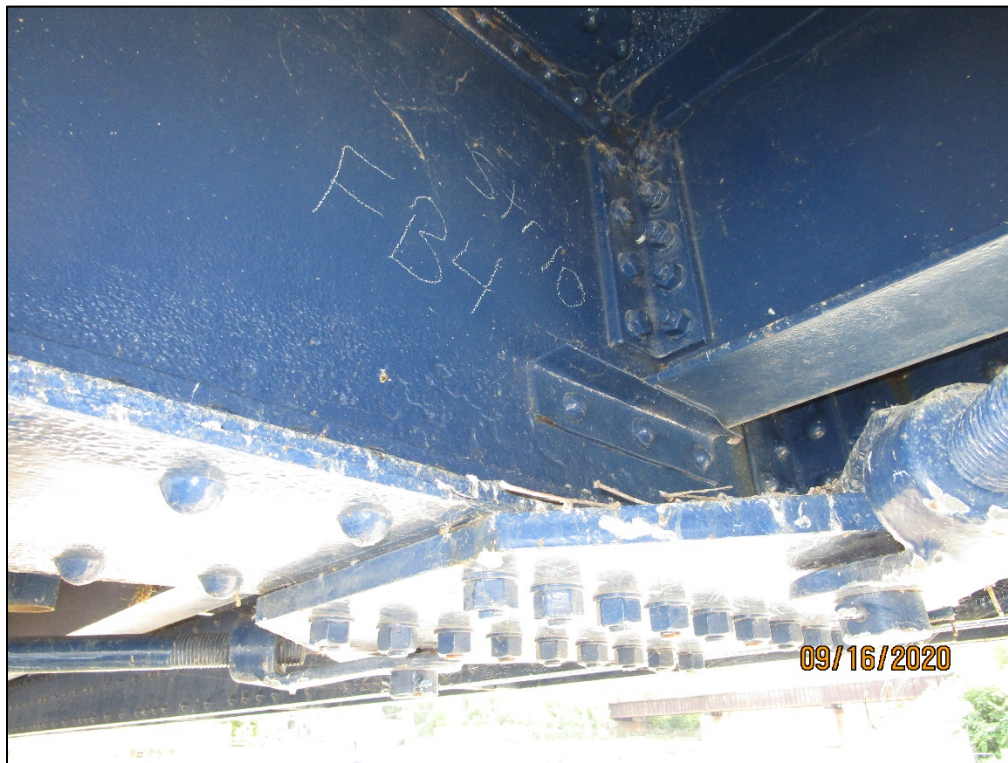
PHOTO 38 – TYPICAL PAINTED OVER PITTING, FLOORBEAM 4, SOUTH END
