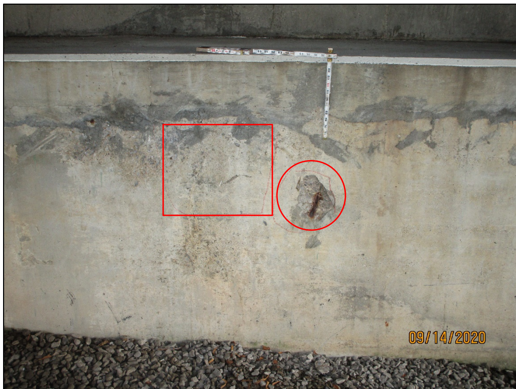
PHOTO 58 – DELAMINATION AND SPALL WITH EXPOSED REINFORCING, FORWARD ABUTMENT
