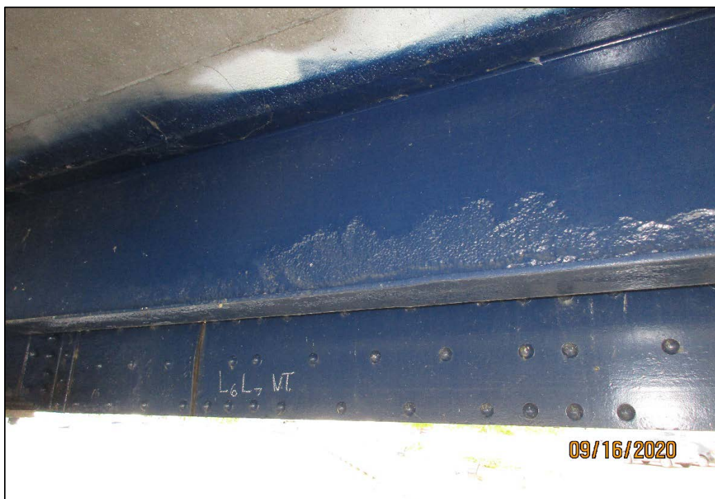
PHOTO 24 – PAINTED OVER PITTING ON SIDEWALK STRINGER, NORTH SIDE, PANEL 7
