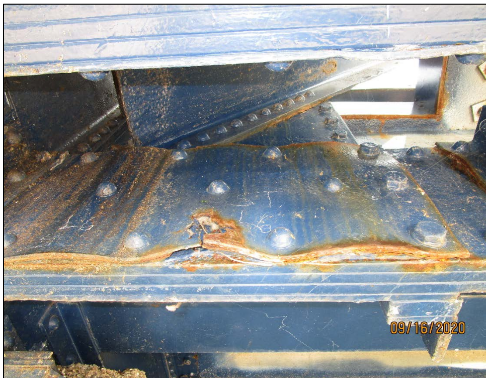
PHOTO 27 – LOWER CHORD WEB PLATE PERFORATION, L6, SOUTH TRUSS
