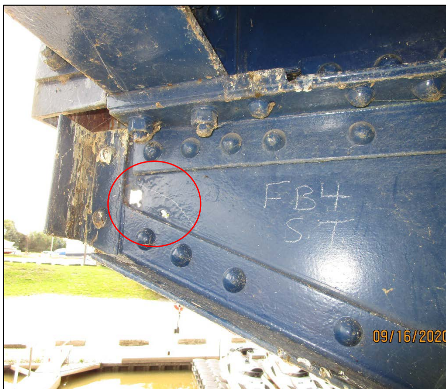
PHOTO 42 – PAINTED OVER PITTING WITH HOLE, FLOORBEAM 4 SIDEWALK CANTILEVER, SOUTH TRUSS
