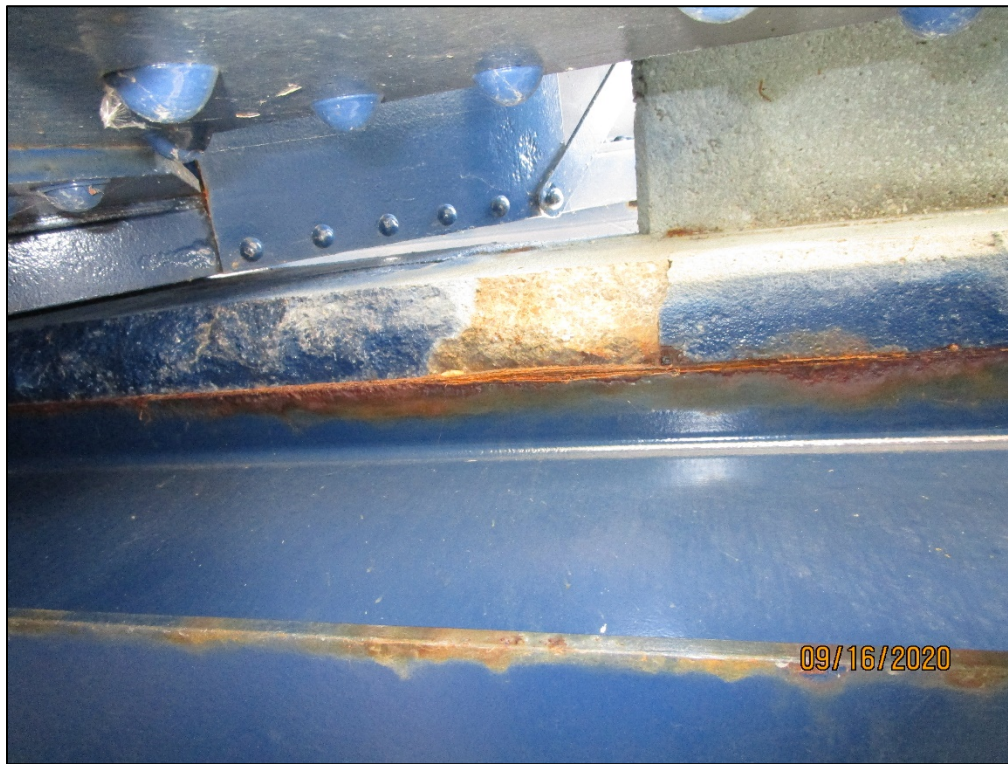
PHOTO 20 – ACTIVE CORROSION TO INSIDE EDGE OF EXTERIOR STRINGER TOP FLANGE, STRINGER 1, PANEL 9
