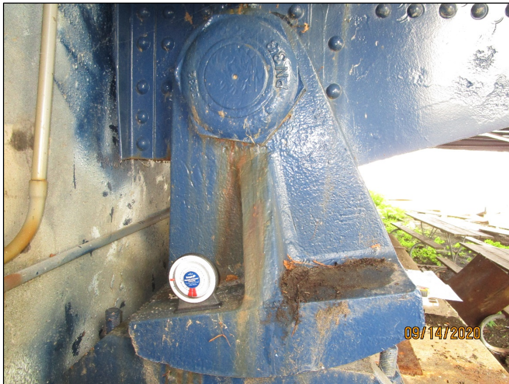
PHOTO 47 — ROCKER BEARING WITH ACTIVE CORROSION, REAR ABUTMENT, SOUTH TRUSS
