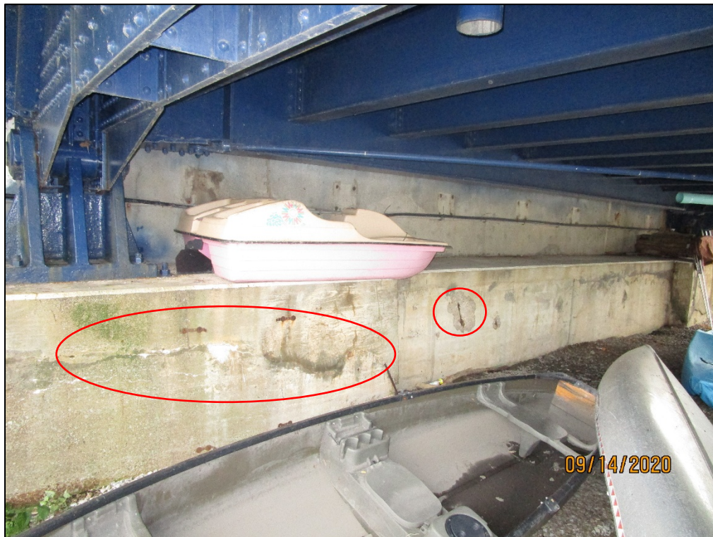
PHOTO 56 – PATCHED JOINT WITH EFFLORESCENCE AND SPALL WITH EXPOSED REINFORCING, FORWARD ABUTMENT
