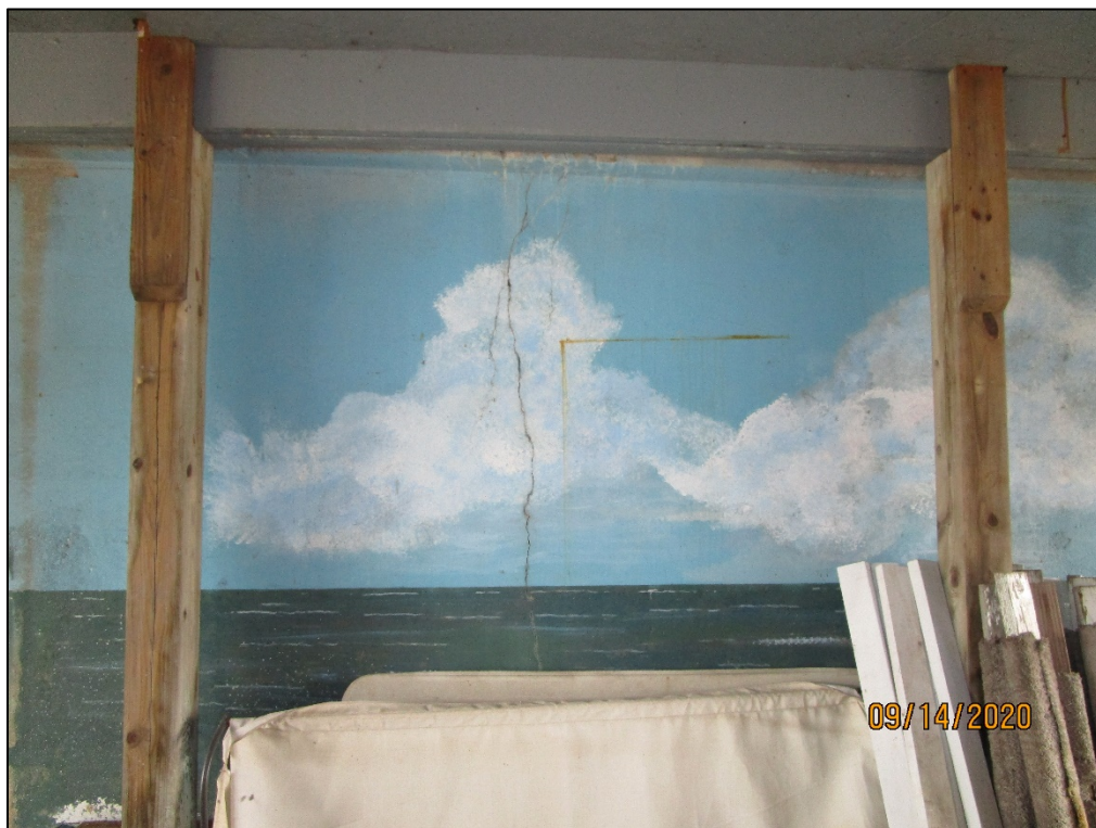
PHOTO 62 – CS3 VERTICAL CRACK ON SOUTHEAST WINGWALL
