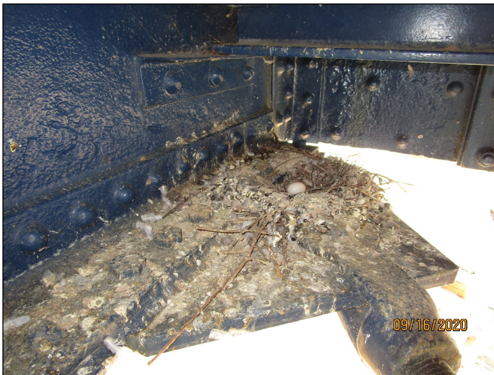
PHOTO 50 – TYPICAL PIGEON DROPPINGS ON LOWER LATERAL BRACING
