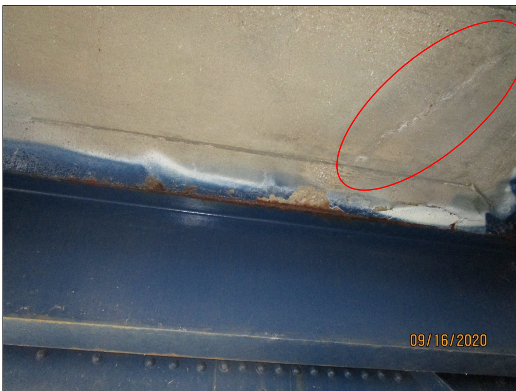
PHOTO 4 – HAUNCH SPALL AND TRANSVERSE CRACK WITH EFFLORESCENCE, STRINGER 1, FLOORBEAM 9
