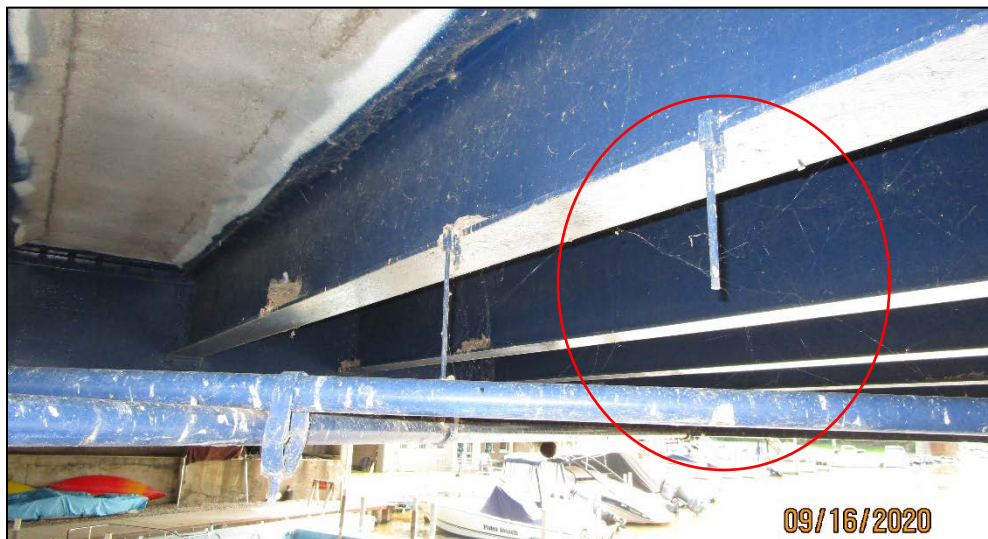
PHOTO 52 – BROKEN HANGER, PANEL 9
