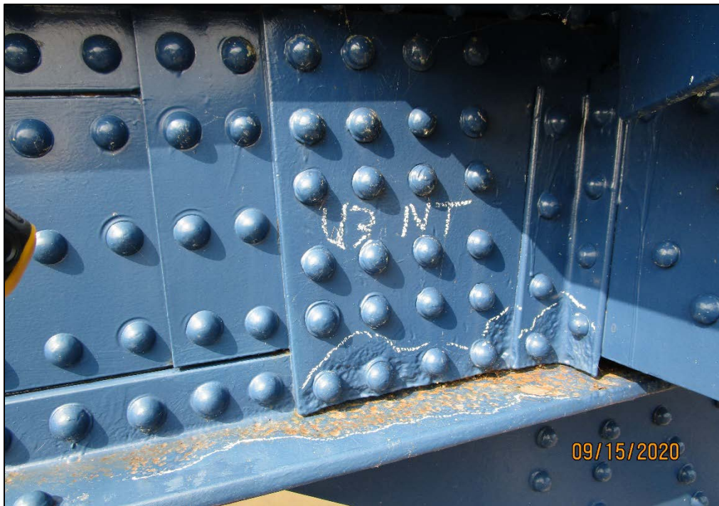
PHOTO 28 – UPPER CHORD PAINTED OVER PITTING TO BOTTOM FLANGE, U3, NORTH TRUSS
