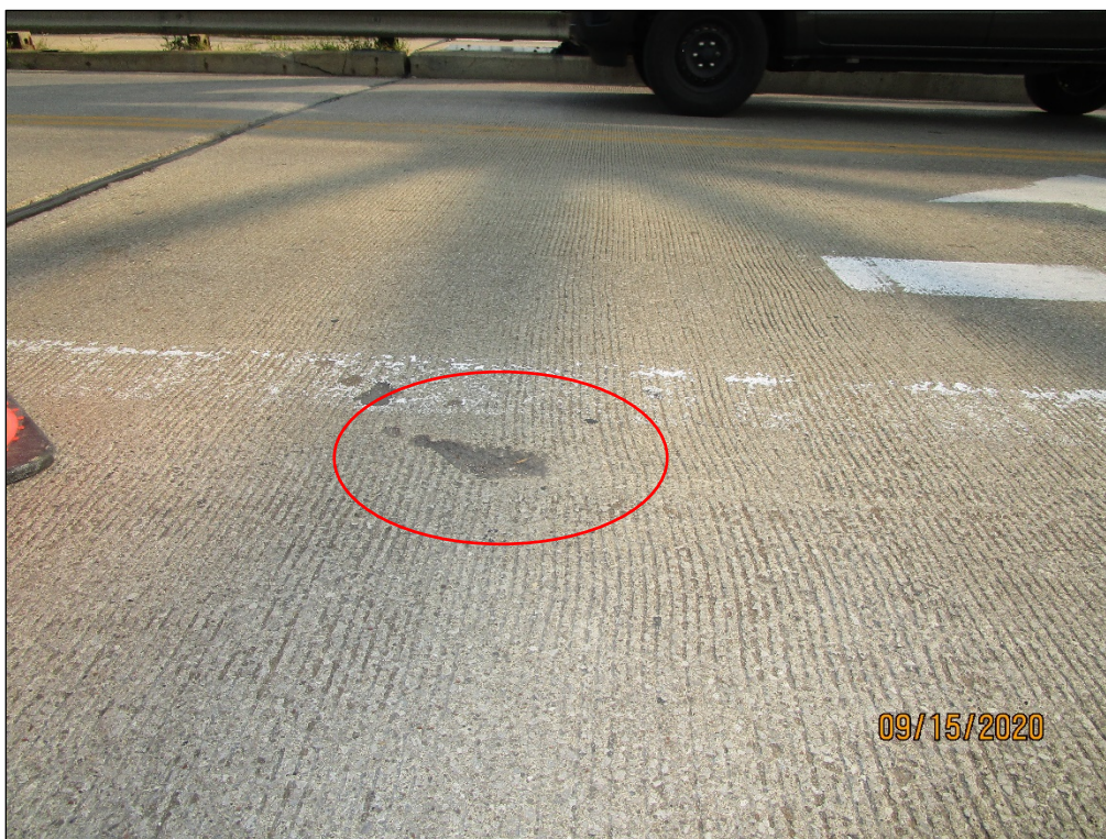
PHOTO 3 – 1'x1' SPALL IN DECK, CENTER LANE, FORWARD ABUTMENT
