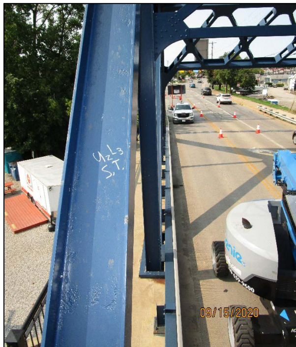
PHOTO 33 — PAINTED OVER PITTING, U2L3, SOUTH TRUSS
