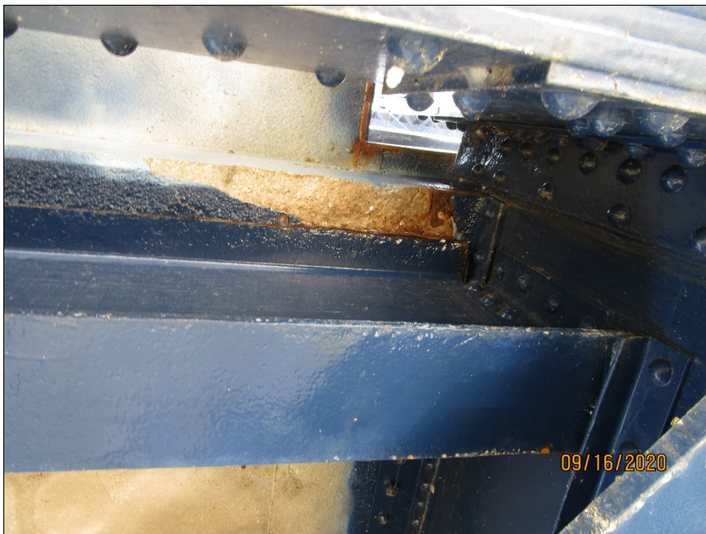
PHOTO 5 – HAUNCH SPALL, STRINGER 10, BETWEEN FLOORBEAMS 7 & 8
