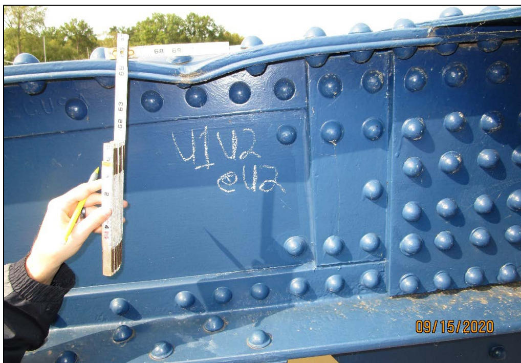
PHOTO 29 – BENT UPPER TOP FLANGE PLATE, U1U2 @ U2, NORTH TRUSS
