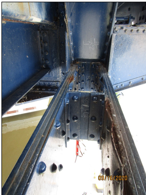
PHOTO 26 – LOWER CHORD, ACTIVE PACK RUST > ½", PANEL 4, NORTH TRUSS
