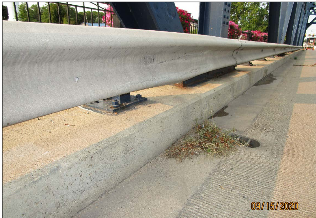
PHOTO 13 – IMPACT DAMAGE TO GUARDRAIL, SOUTH FACE
