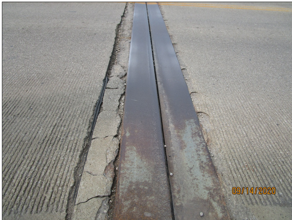
PHOTO 8 – SMALL SPALLS IN DECK ALONG EXPANSION JOINT, REAR ABUTMENT
