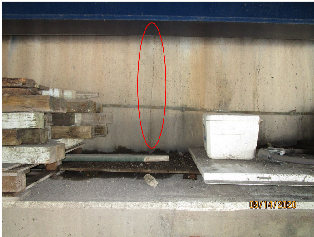
PHOTO 59 – VERTICAL CRACK NEAR MIDDLE OF REAR ABUTMENT
