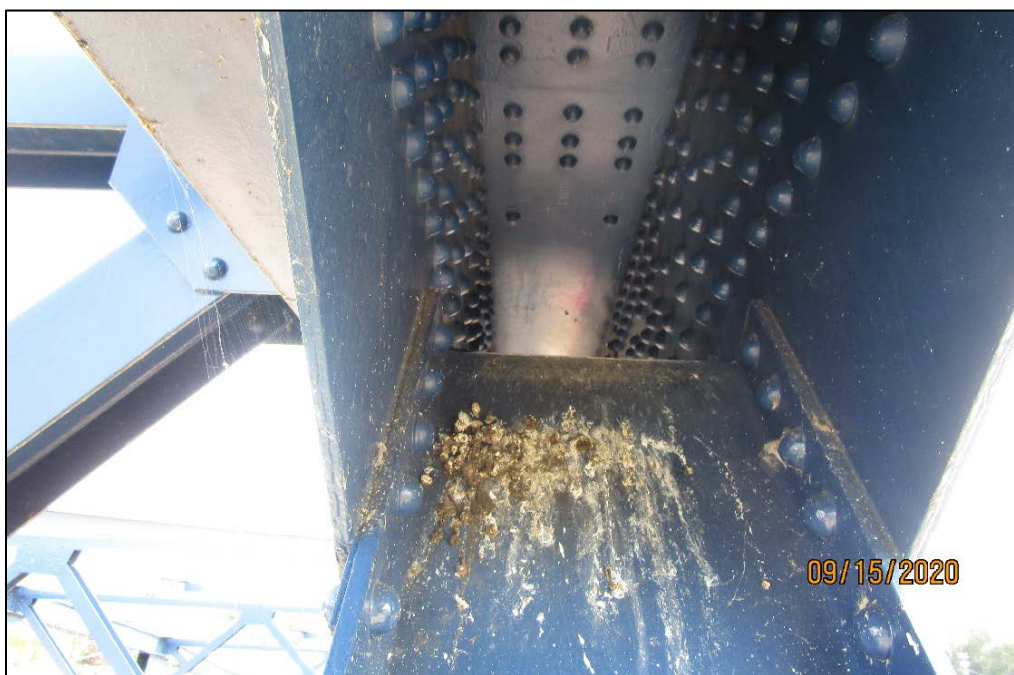
PHOTO 51 – TYPICAL PIGEON DROPPINGS ON DIAGONALS NEAR UPPER CHORD
