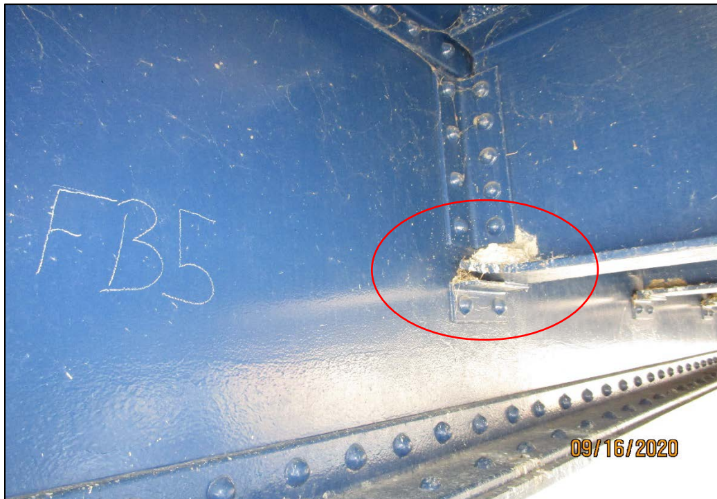
PHOTO 23 – BOTTOM FLANGE BENT AT FLOORBEAM CONNECTION, FLOORBEAM 5 AND STRINGER 6, PANEL 6
