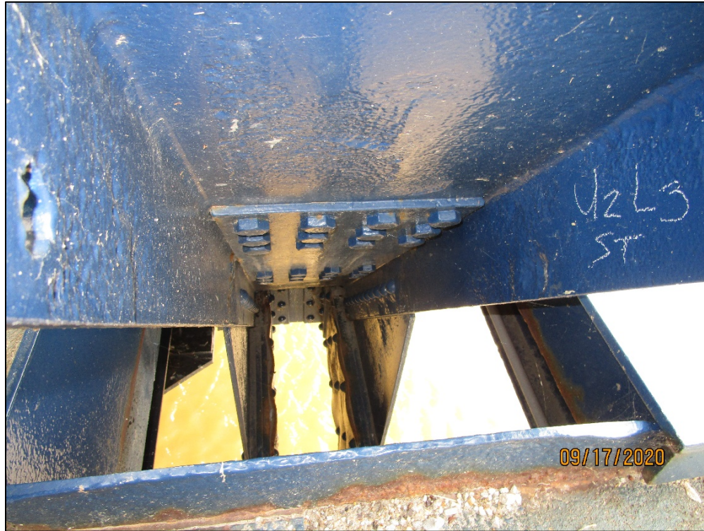
PHOTO 32 — PAINTED OVER PITTING WITH PERFORATION, U2L3, SOUTH TRUSS
