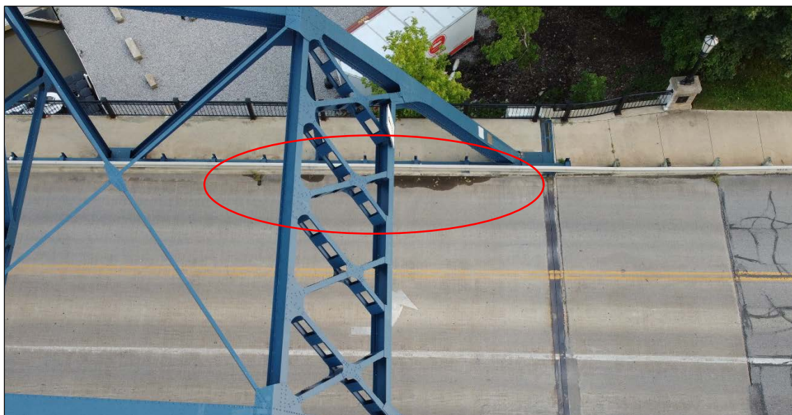
PHOTO 17 – MINOR PONDING ALONG THE SOUTH CURB NEAR THE REAR ABUTMENT
