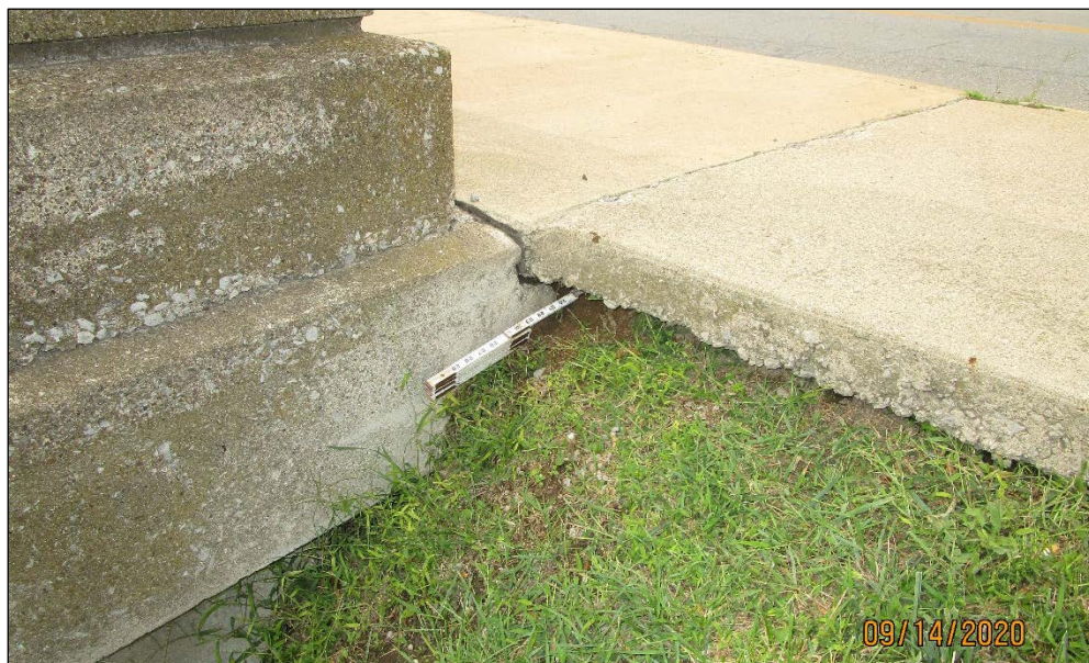
PHOTO 69 – EROSION OF SOUTHEAST EMBANKMENT UNDER SIDEWALK
