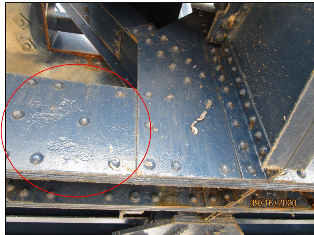
PHOTO 25 – TYPICAL LOWER CHORD PAINTED OVER PITTING
