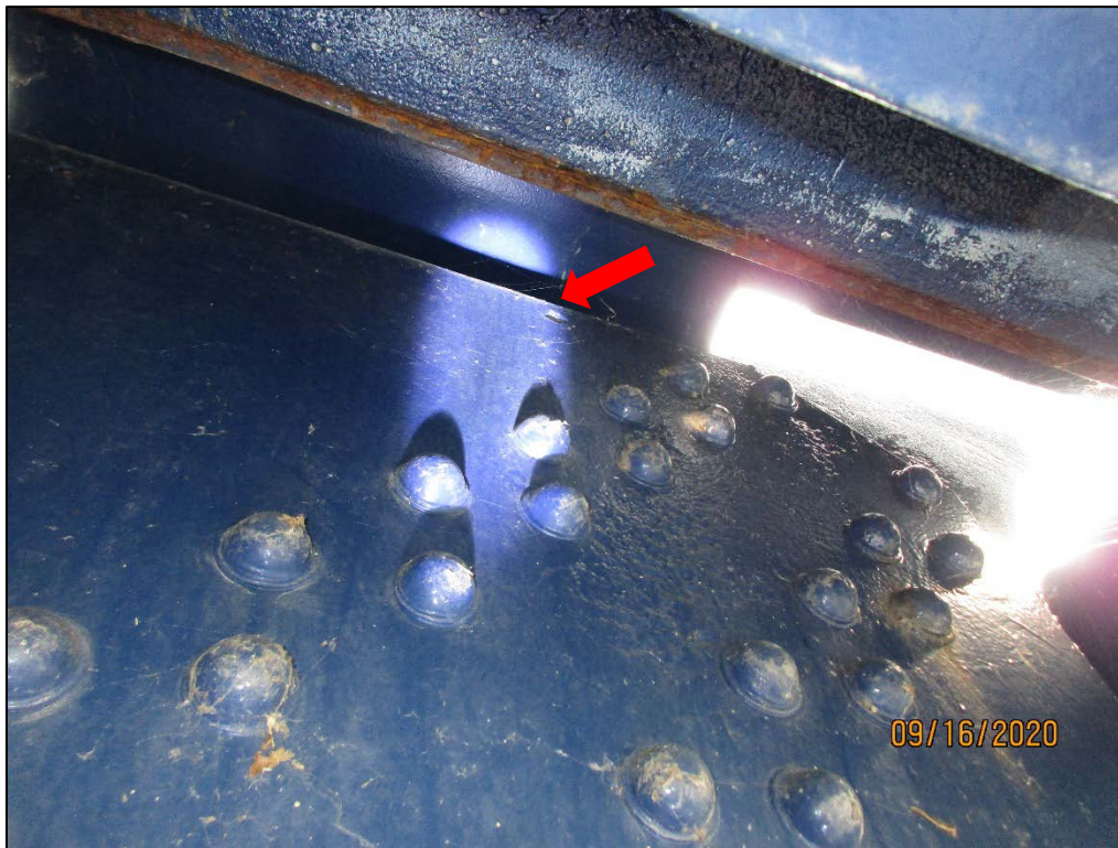
PHOTO 44 – PAINTED OVER PITTING AND PERFORATION, L2, INSIDE GUSSET, NORTH TRUSS
