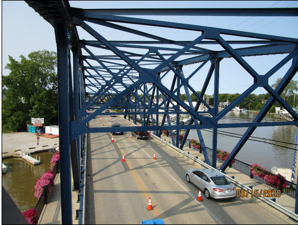
PHOTO 54 – SWAY BRACING, LOOKING WEST
