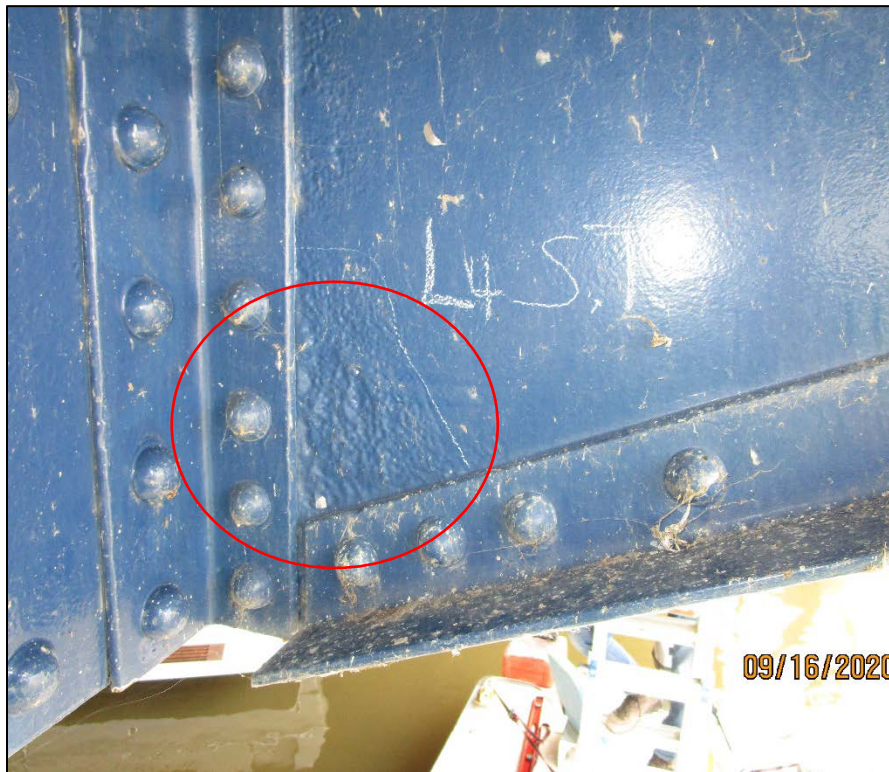
PHOTO 41 – PAINTED OVER PITTING WITH PINHOLE, FLOORBEAM 4 SIDEWALK CANTILEVER, SOUTH TRUSS
