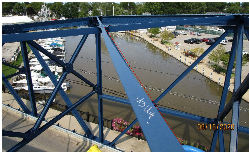
PHOTO 53 – TYPICAL UPPER LATERAL BRACING SAG
