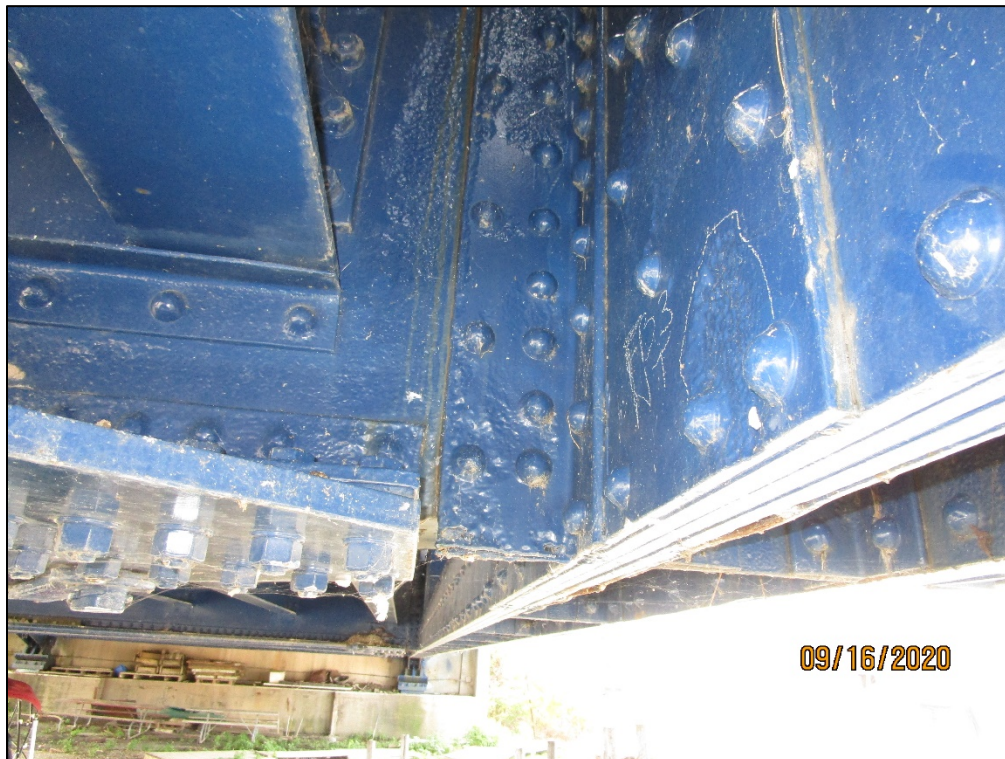
PHOTO 39 – ACTIVE CORROSION AT FLOORBEAM END & GUSSET, FLOORBEAM 3, NORTH END
