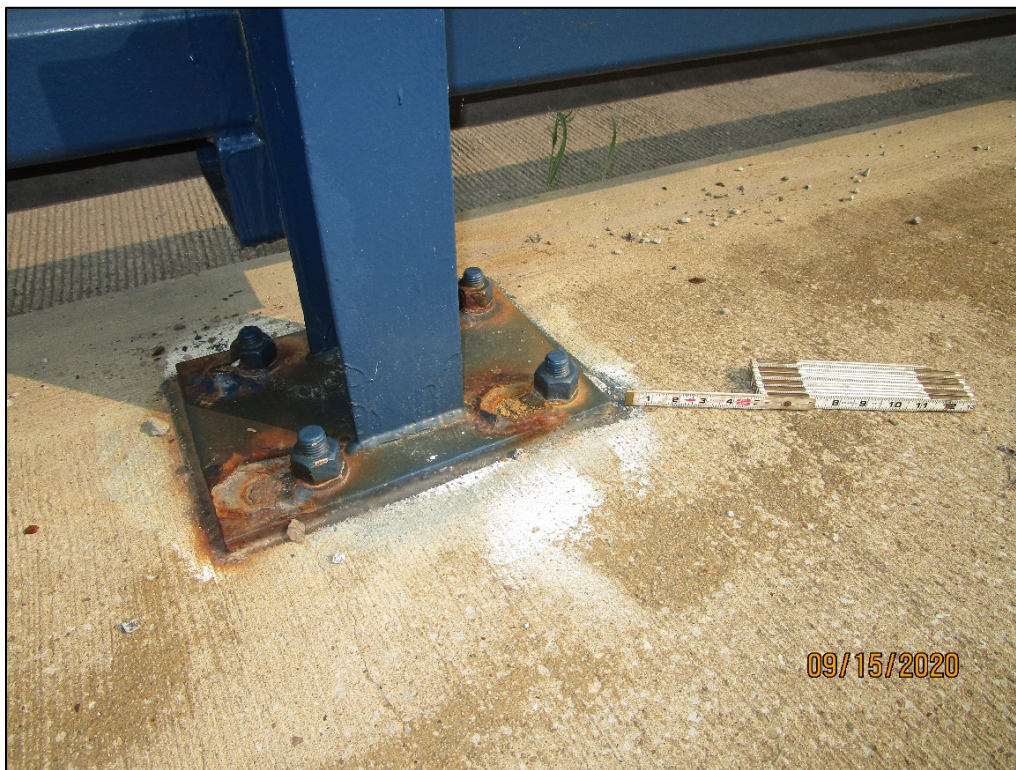
PHOTO 10 – CORROSION TO RAIL POST BASE PLATE
