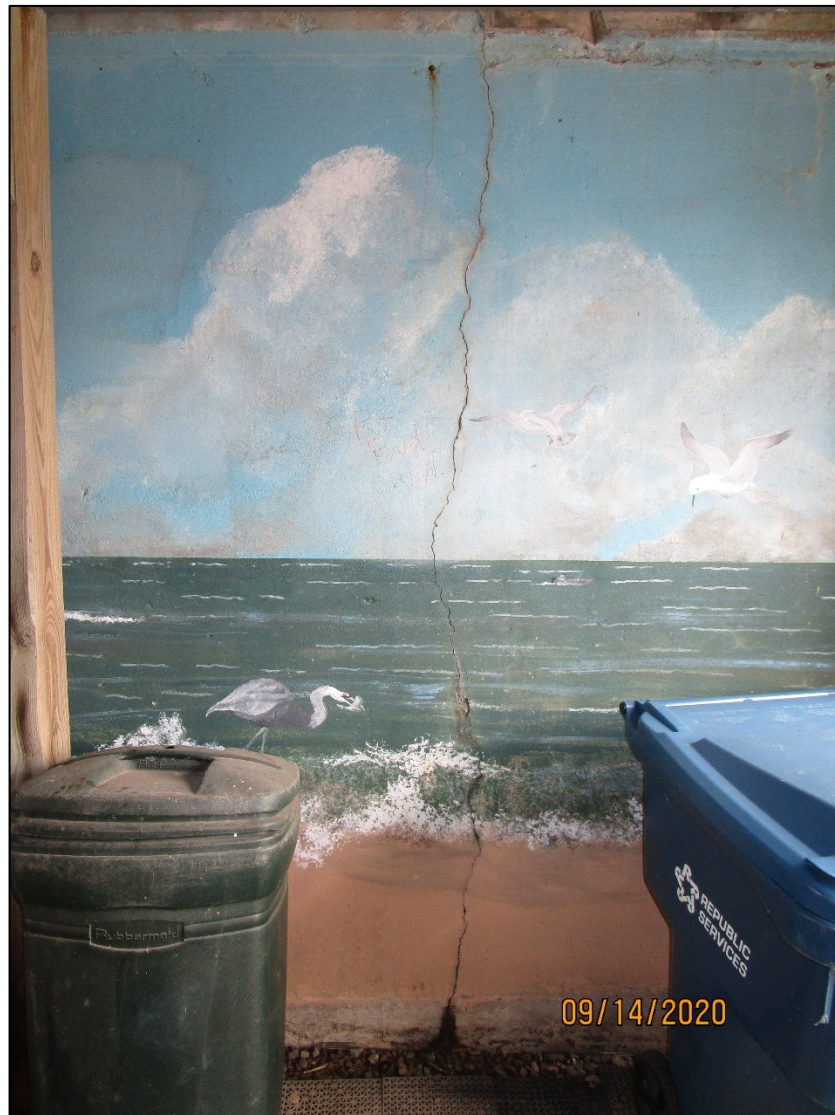
PHOTO 60 – CS3 VERTICAL CRACK ON SOUTHEAST WINGWALL
