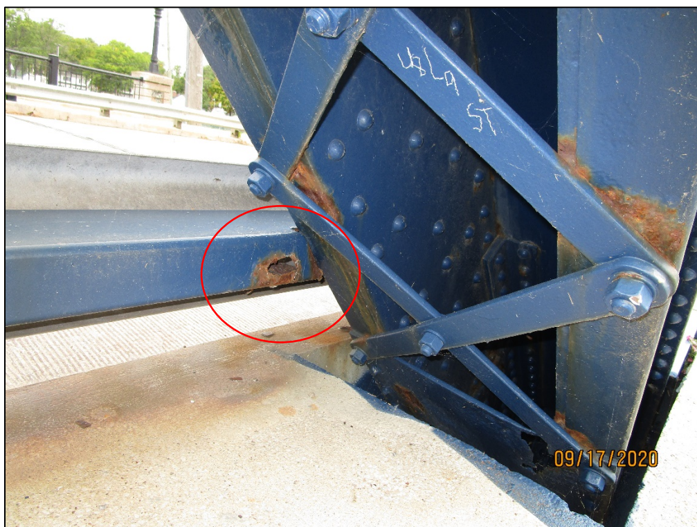
PHOTO 12 – ACTIVE CORROSION WITH PERFORATION ON BACKSIDE OF STEEL BACKUP, SOUTH TRUSS NEAR L9.
