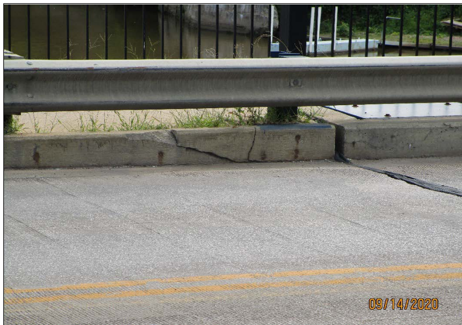
PHOTO 19 – SPALL AND DELAMINATED CURB ON SOUTHEAST CORNER
