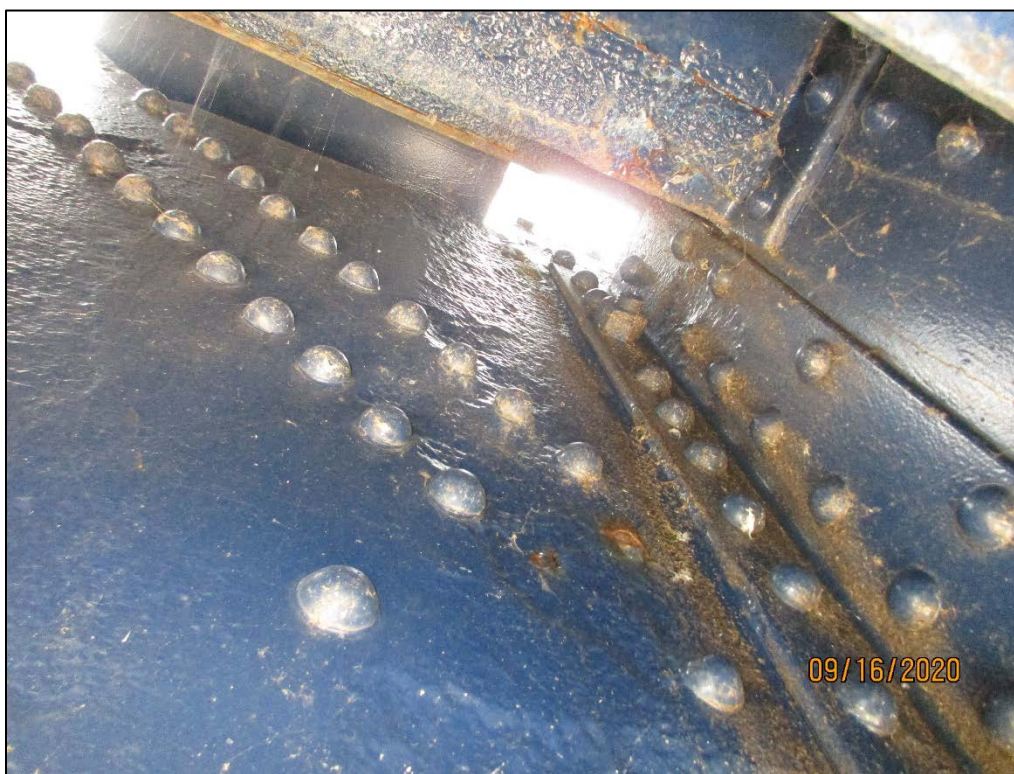
PHOTO 45 – PAINTED OVER PITTING, L6, INSIDE GUSSET, SOUTH TRUSS
