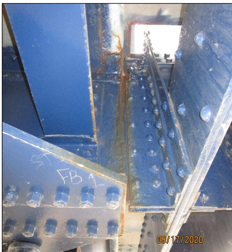
PHOTO 40 – ACTIVE CORROSION AT FLOORBEAM END, FLOORBEAM 1, SOUTH TRUSS
