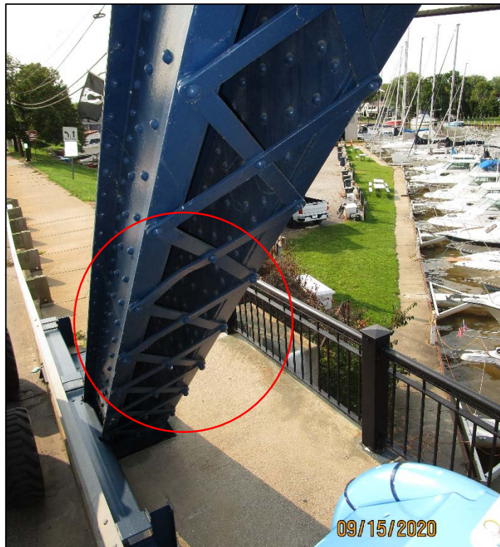
PHOTO 30 – TYPICAL BENT LACING BARS, LOU1, NORTH TRUSS
