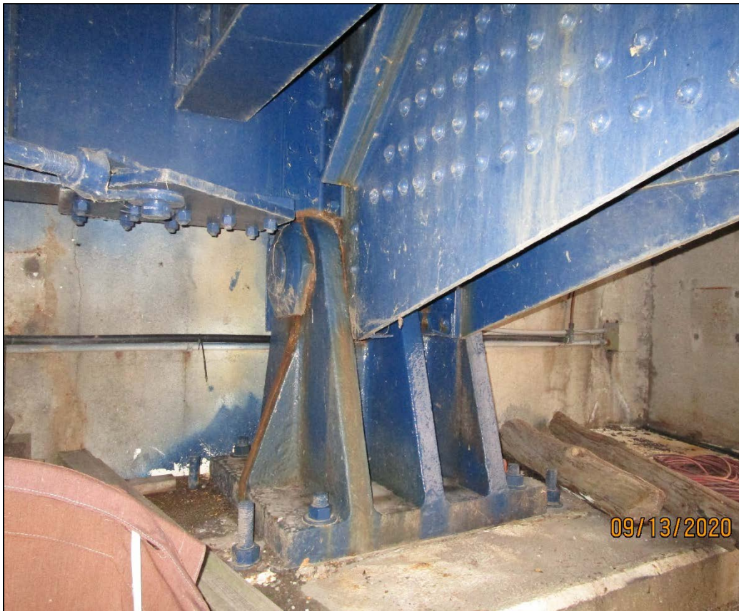
PHOTO 46 – FIXED BEARING AT FORWARD ABUTMENT, SOUTH TRUSS
