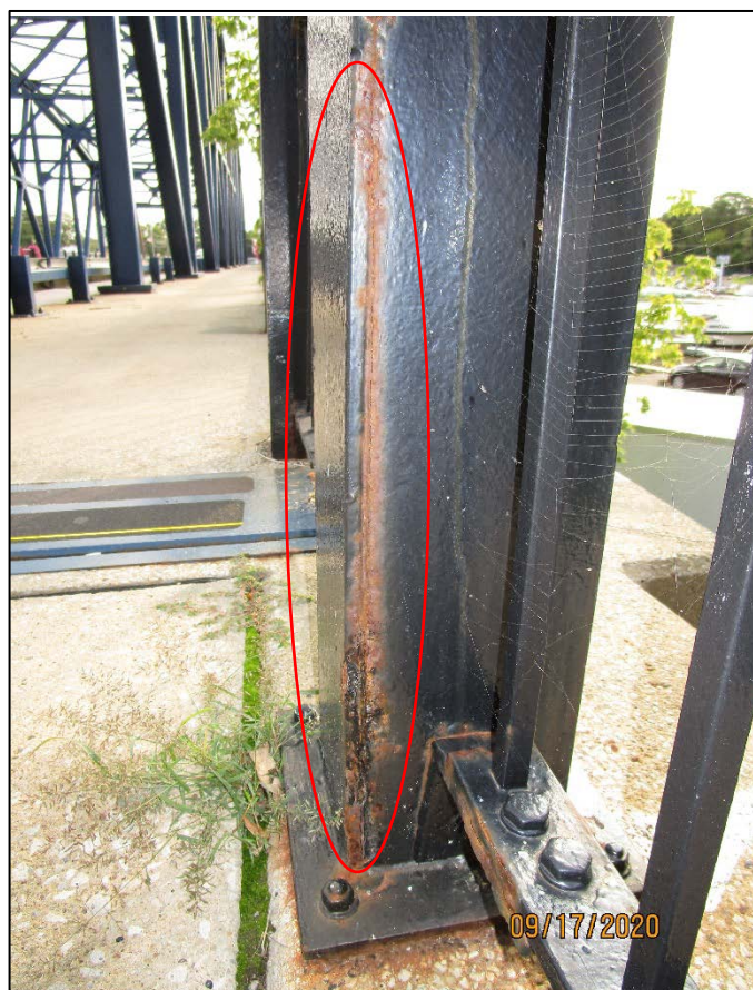
PHOTO 14 – VERTICAL CRACK IN SIDEWALK RAILING POST, SOUTHWEST APPROACH
