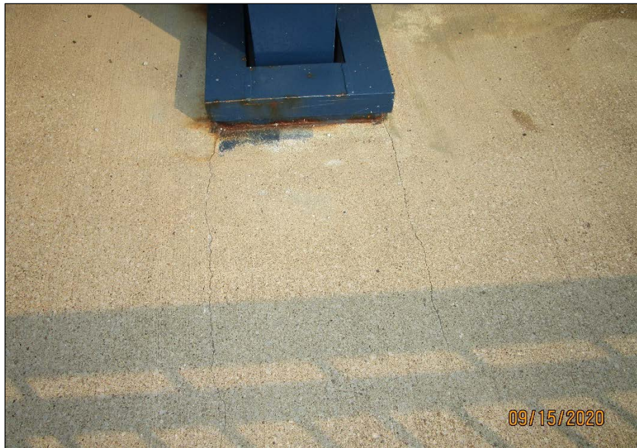
PHOTO 18 – TYPICAL TRANSVERSE HAIRLINE CRACKS ON SIDEWALK NEAR TRUSS BLOCKOUT
