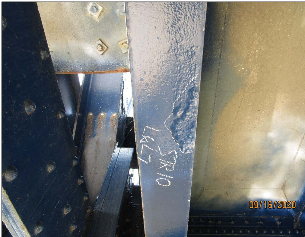
PHOTO 21 – BOTTOM FLANGE OF STRINGER WITH PITTING, STRINGER 10, PANEL 7
