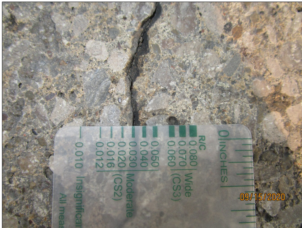
PHOTO 2 - TRANSVERSE CRACK IN DECK, 0.030" WIDE
