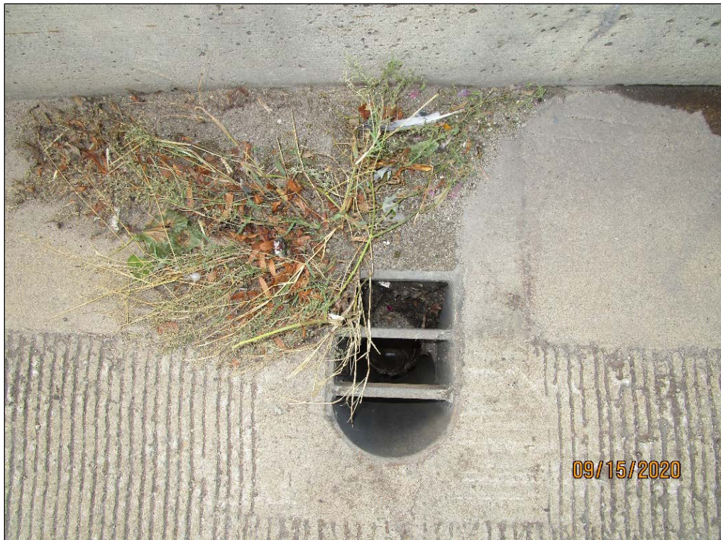
PHOTO 15 – TYPICAL SCUPPER WITH PARTLY CLOGGED INLET AND DEBRIS
