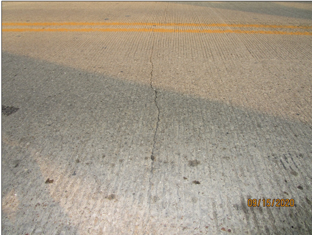
PHOTO 7 – TYPICAL WEAR OF SKID-RESISTANCE GROOVES IN WHEEL PATH AND TRANSVERSE CRACK
