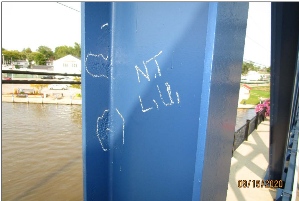
PHOTO 36 – PAINTED OVER PITTING, L1U1, NORTH TRUSS
