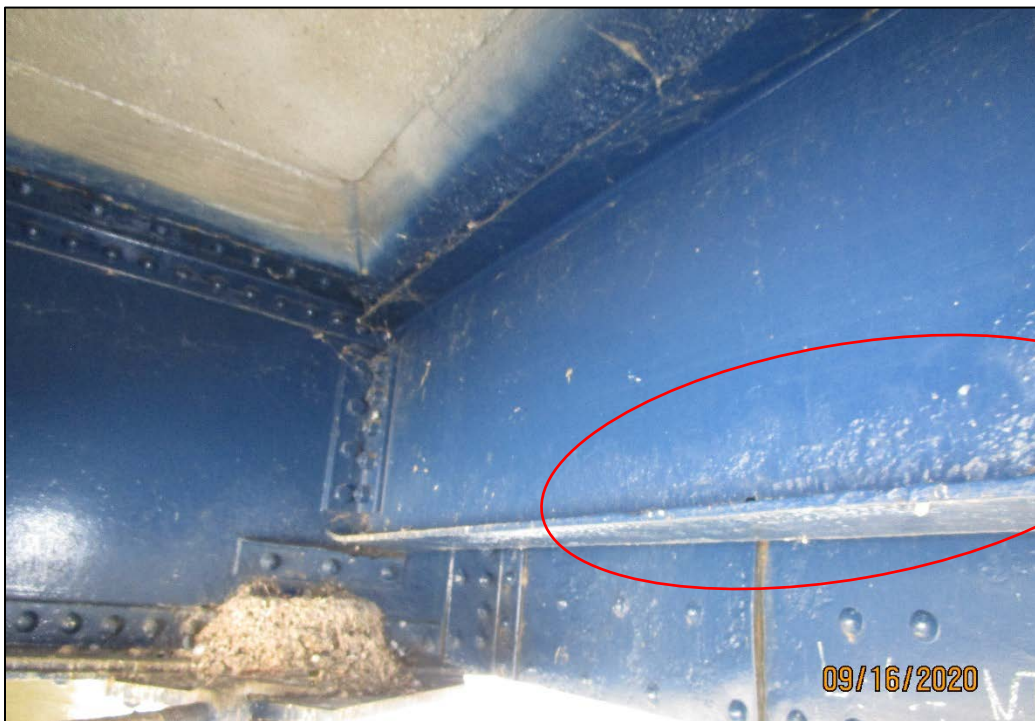
PHOTO 22 – BOTTOM FLANGE AND WEB PAINTED OVER PITTING, STRINGER 1, PANEL 7
