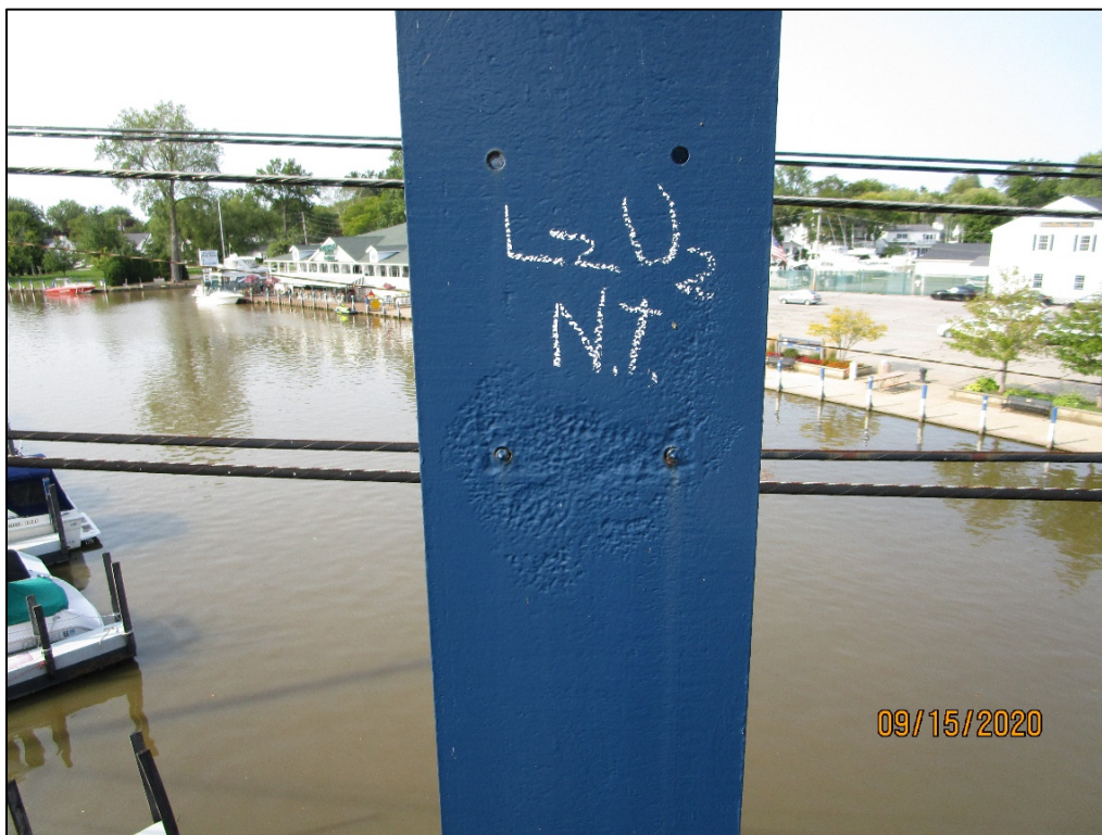
PHOTO 37 – HOLES AND PAINTED OVER PITTING, L2U2, NORTH TRUSS
