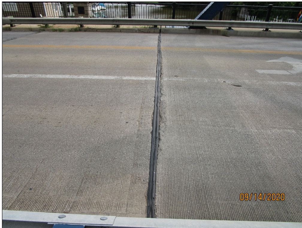
PHOTO 9 – TORN COMPRESSION SEAL WITH DECK SPALLS, FORWARD ABUTMENT
