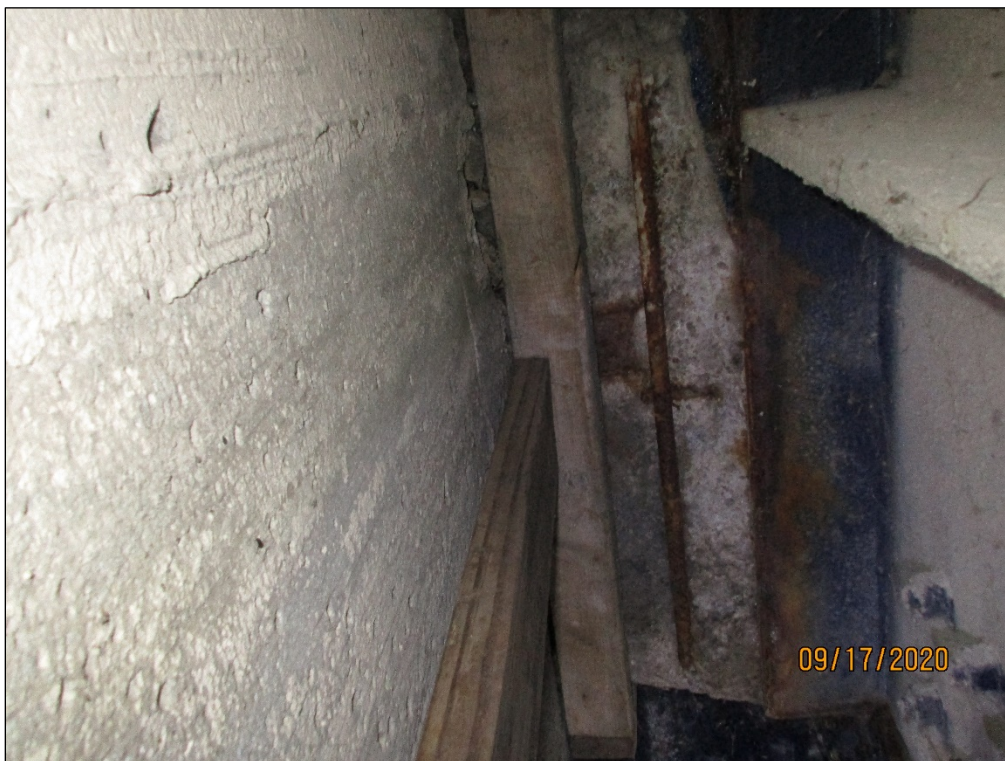
PHOTO 6 – SPALL ON UNDERSIDE OF DECK NEAR REAR ABUTMENT, FLOORBEAM 0
