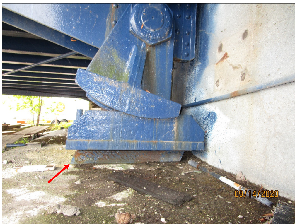
PHOTO 48 — DEFORMED ELASTOMERIC BEARING, REAR ABUTMENT, NORTH TRUSS
