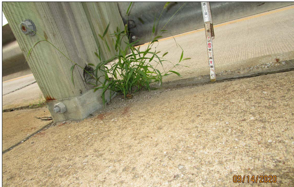
PHOTO 68 – SIDEWALK SETTLEMENT AT NORTHWEST APPROACH
