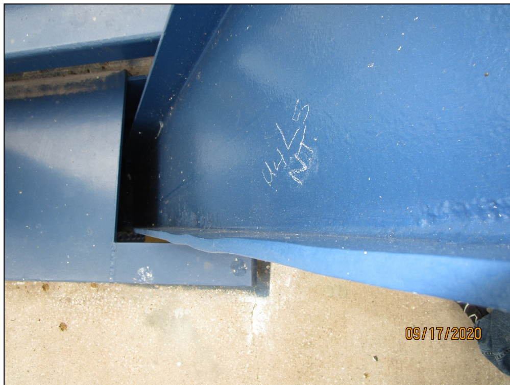
PHOTO 34 – WAVY DIAGONAL FLANGE, U4L5, NORTH TRUSS
