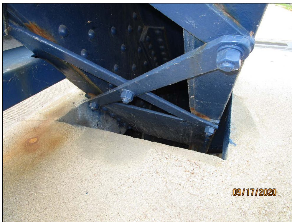
PHOTO 31 – TYPICAL ACTIVE CORROSION TO END POST IN SPLASH ZONE, SOUTH TRUSS
