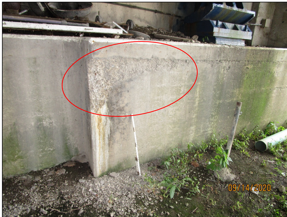
PHOTO 56 – SPALL WITH EFFLORESCENCE, REAR ABUTMENT
