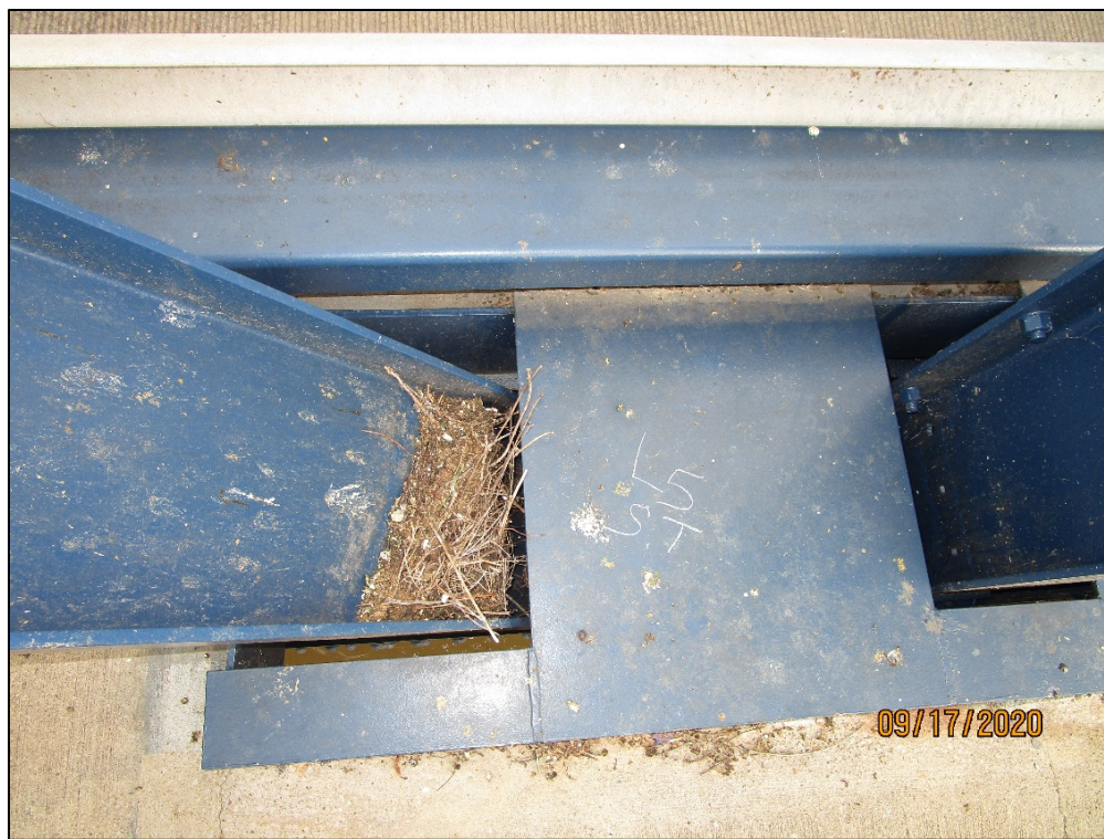
PHOTO 35 – TYPICAL BIRD DROPPINGS AND DEBRIS, L5, SOUTH TRUSS
