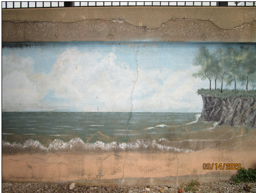
PHOTO 61 – CS3 VERTICAL CRACK ON SOUTHEAST WINGWALL
