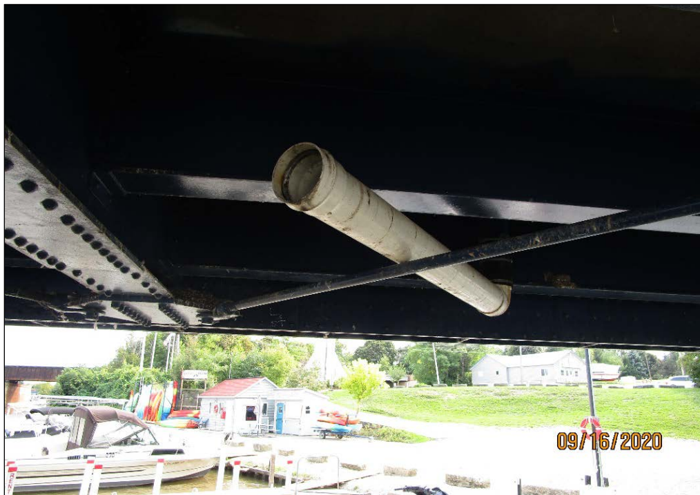
PHOTO 16 – SHORTENED DRAINPIPE ON THE NORTHEAST CORNER
