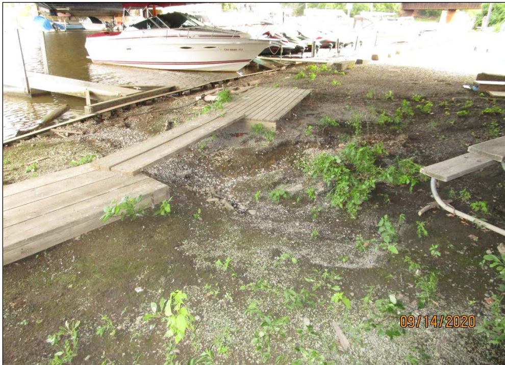
PHOTO 71 – EROSION IN FRONT OF REAR ABUTMENT
