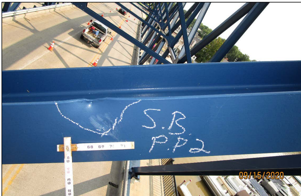
PHOTO 55 – IMPACT DAMAGE TO FLANGE, PANEL POINT 2
