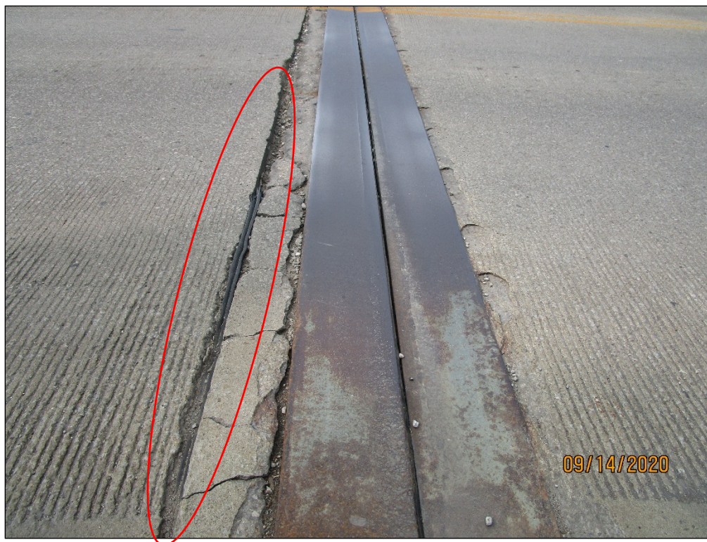
PHOTO 64 – REAR APPROACH SLAB WITH FAILED COMPRESSION SEAL AND SPALLS
