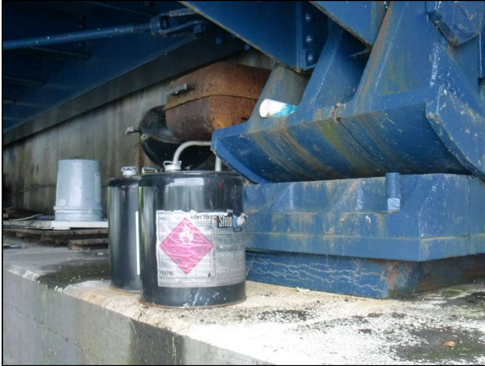
Photo 58 – Flammable Material & Charcoal Grills Stored on Rear Abutment Seat
