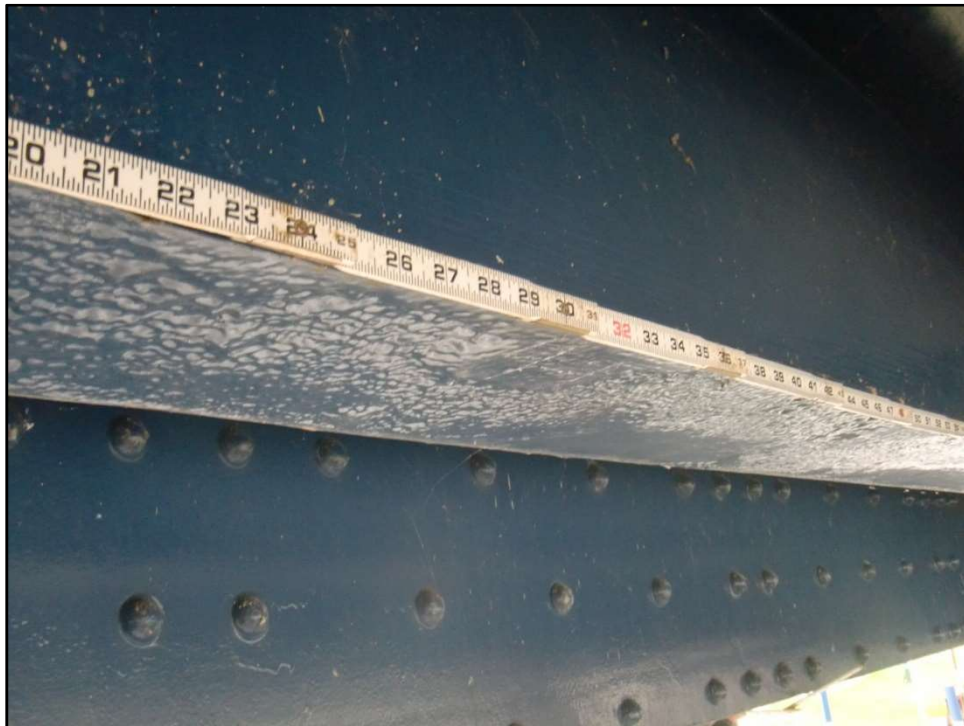
Photo 19 – Bottom Flange Pitting, Stringer 1, Panel 5
