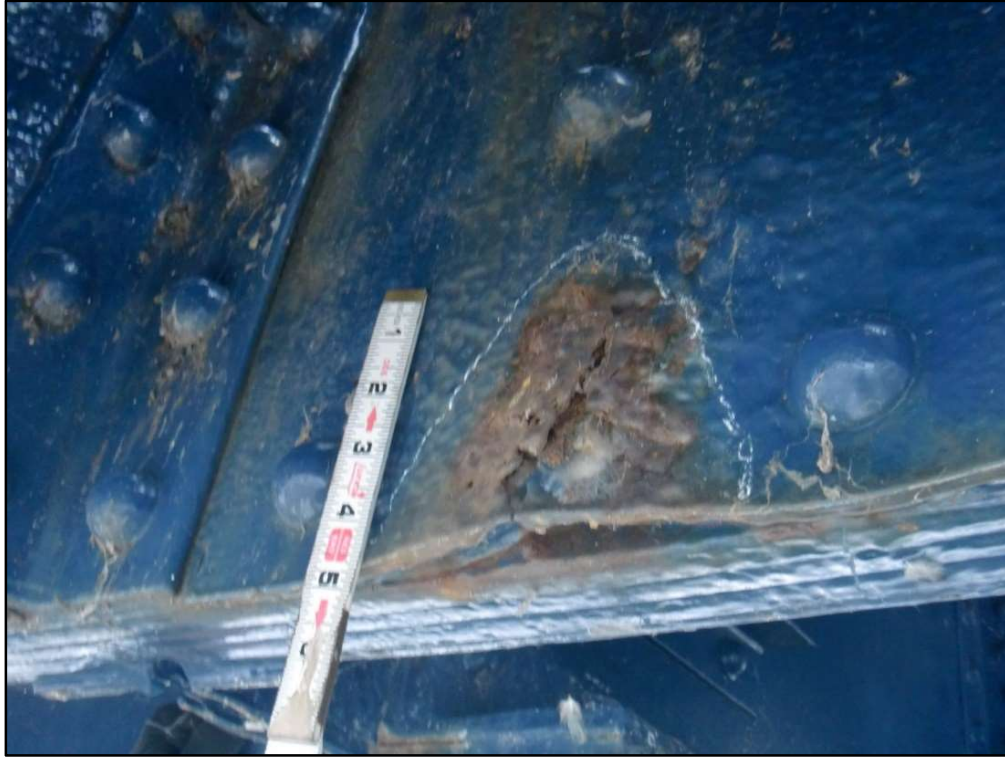
Photo 35 – Lower Chord Web Plate Perforation, L 2 L 3 North
