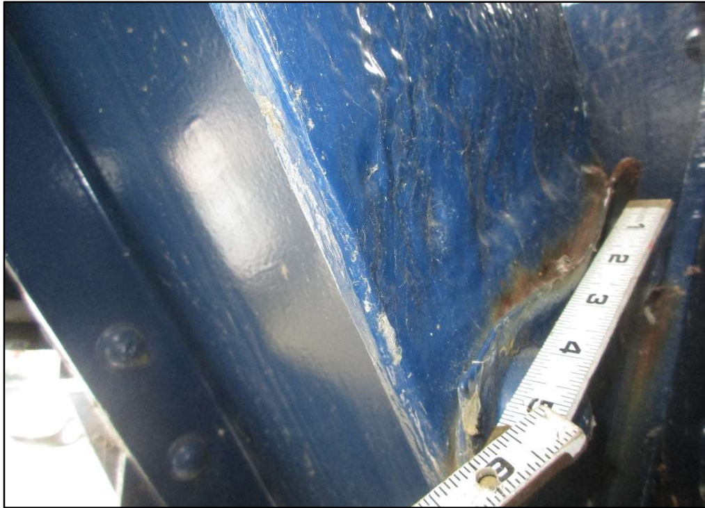
Photo 28 – Section Loss to Flanges with Pack Rust Behind Fill Plate, L 3 U 4 South at L 3 S
