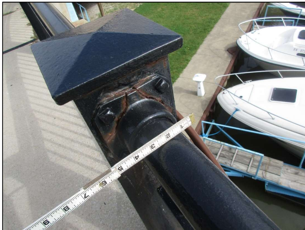
Photo 11 – Typical Cracked Railing Bracket, South Rail
