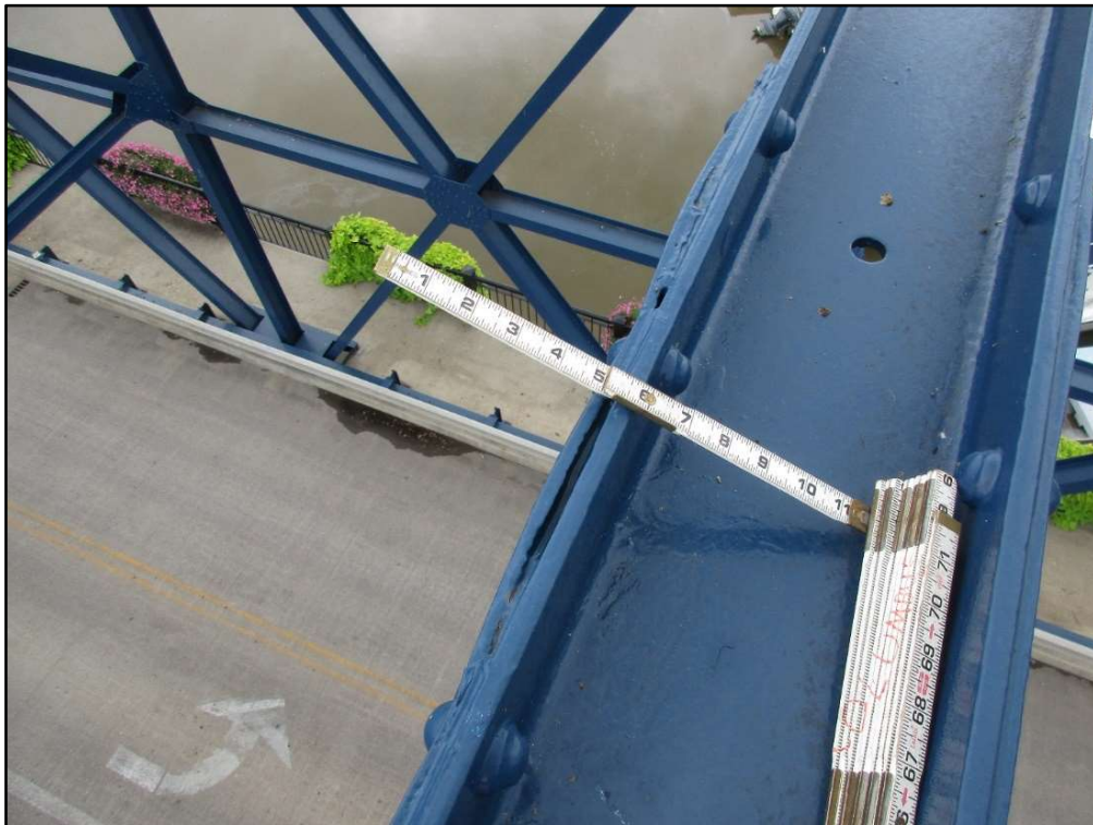
Photo 41 – Typical Pack Rust Behind Sway Bracing Gusset
