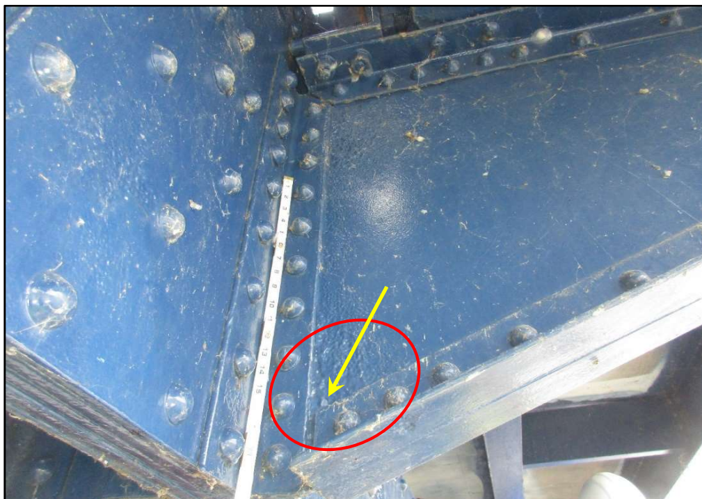
Photo 26 – Web Pitting (Circled) with Perforation (at Arrow), Floorbeam Sidewalk Cantilever End, L 5 North
