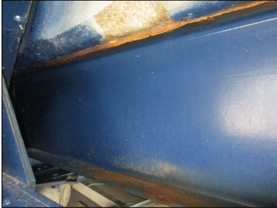
Photo 18 – Top Flange Active Corrosion, Stringer 1, Panel 9
