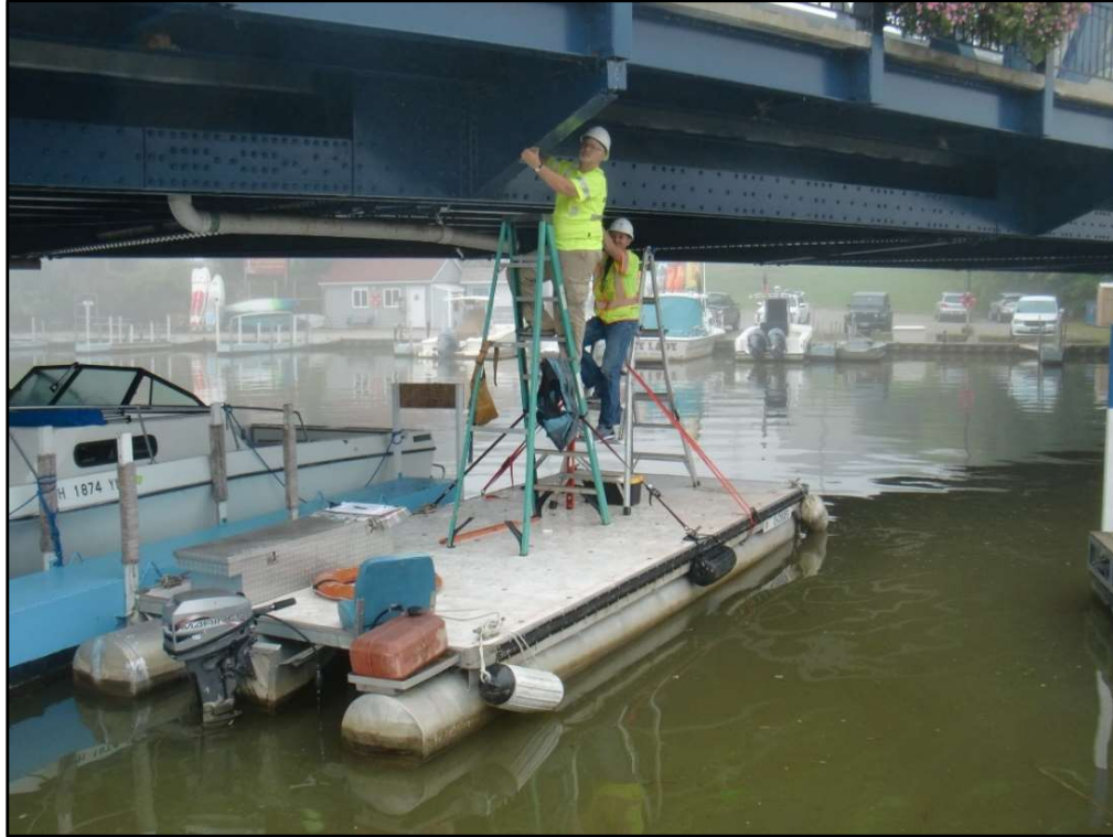
Photo 3 – Lower Chord & Floor System Inspection with a Pontoon Boat & Step Ladders
