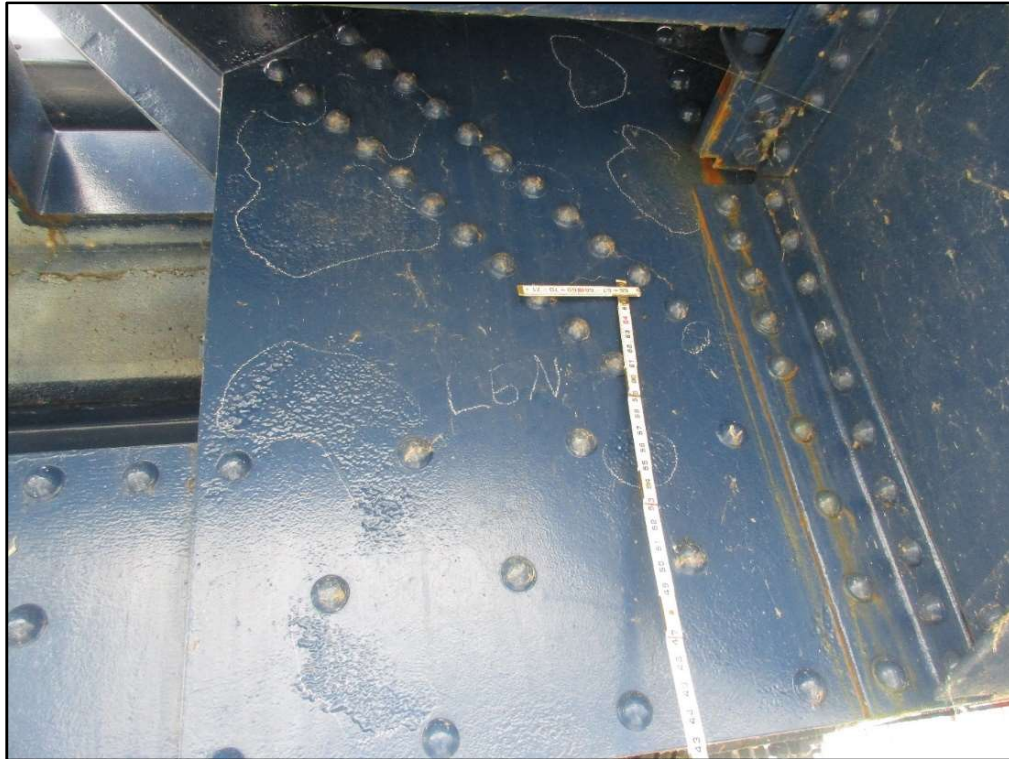
Photo 36 – Typical Scattered Minor Pitting, L6 North Exterior Gusset Plate
