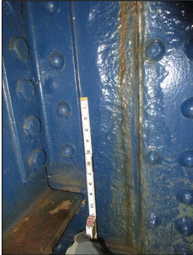
Photo 23 – Pitting to Web, Floorbeam 1 at L 1 South
