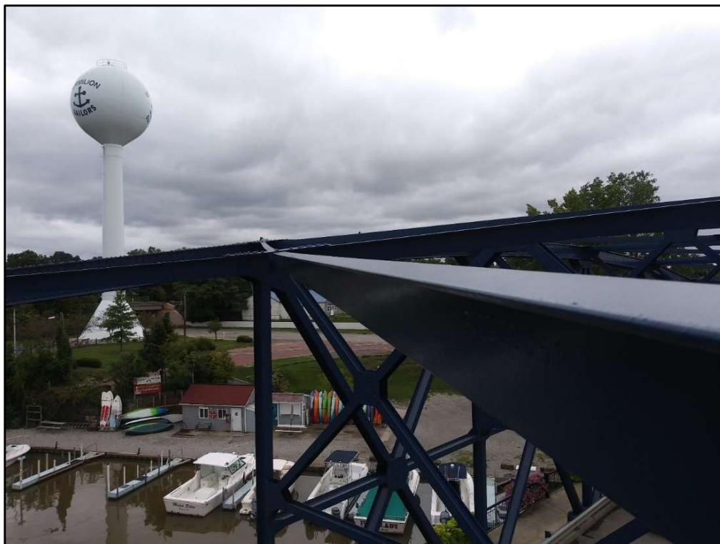
Photo 40 – Typical Upper Lateral Bracing Sag
