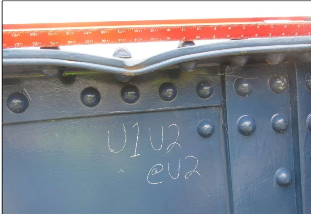
Photo 31 – Dented Top Flange Plate and Angle, U 1 U 2 North
