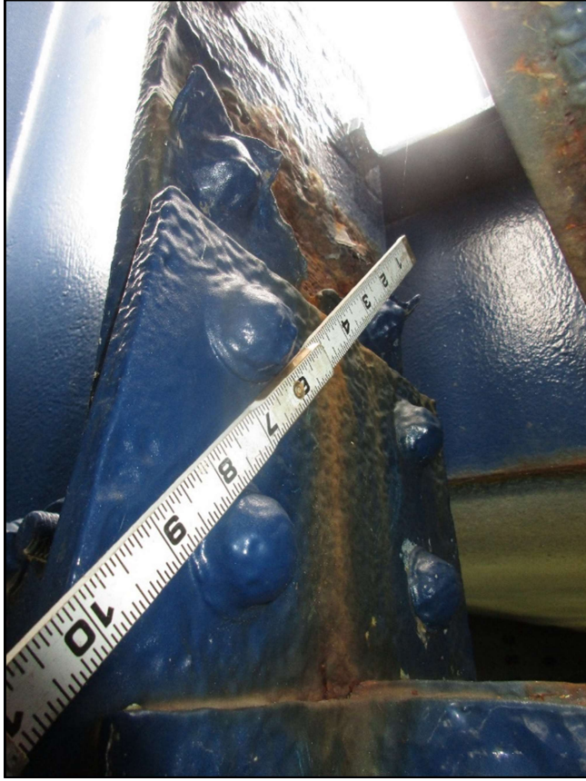
Photo 44 – Common Local Protective Coating System Failure & Reactivating Pack Rust Failure, Bearing Gusset Plates
