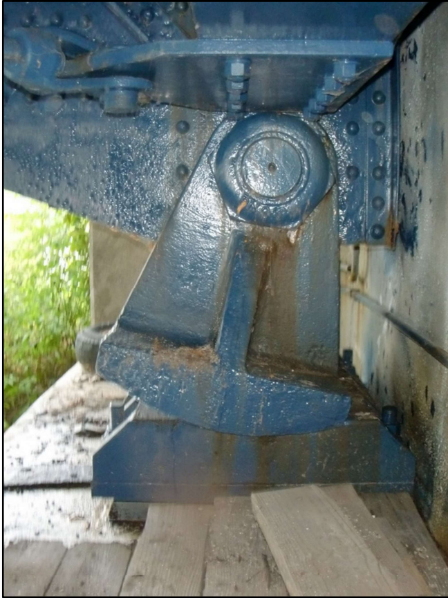
Photo 43 – Expanded Rocker Bearing, L 0 South at 75° F
