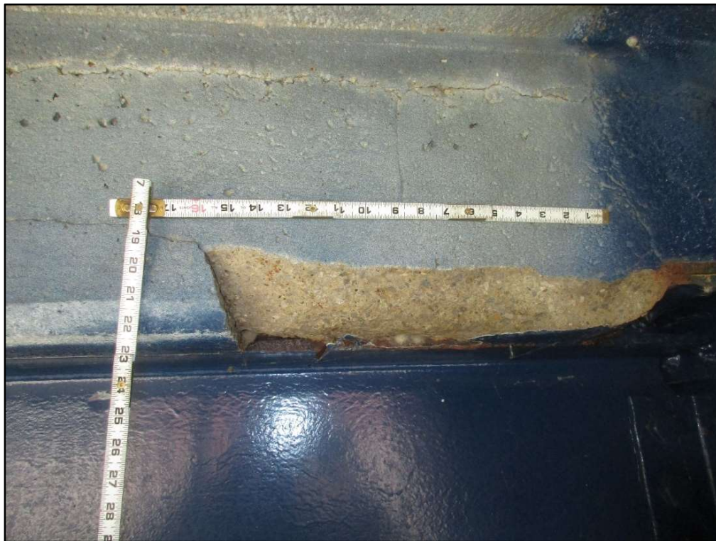
Photo 6 – Typical Corner Spall and Delamination, Edge of Roadway Deck
