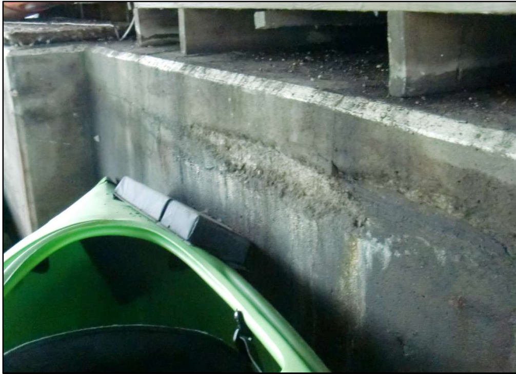
Photo 46 – Scaling Below New Abutment Seat, Rear Abutment
