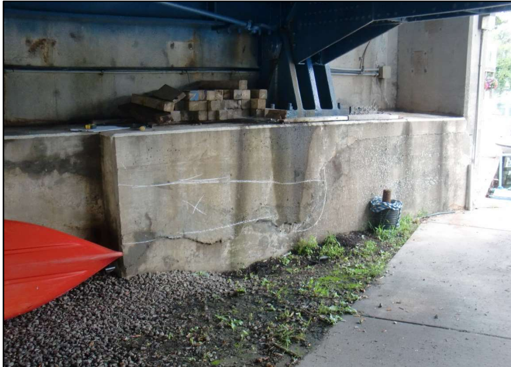
Photo 47 – Delamination Below New Abutment Seat, Forward Abutment
