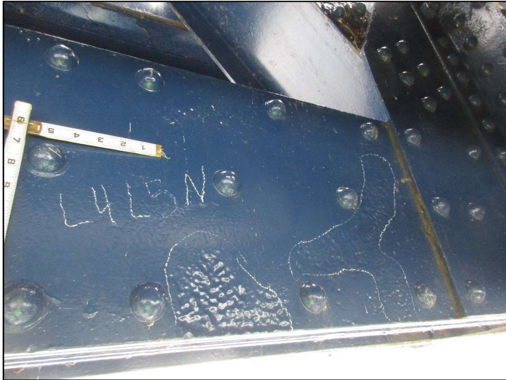
Photo 33 – Typical Lower Chord Pitting
