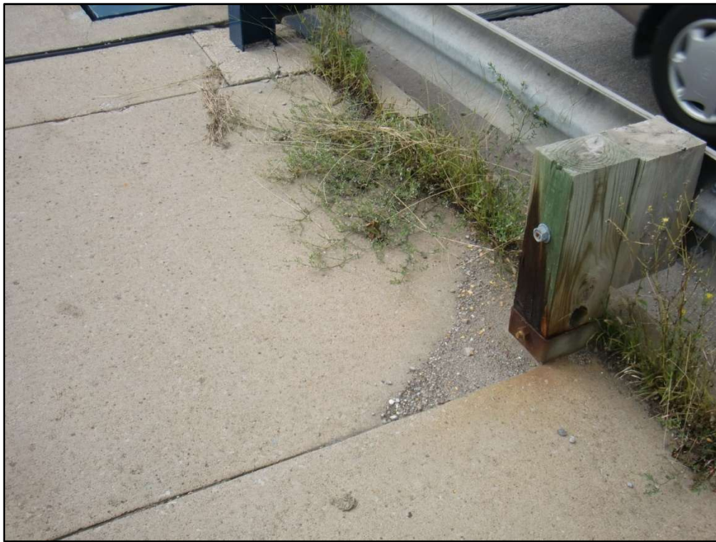
Photo 54 – Typical Approach Sidewalk Settlement (Northwest Approach Sidewalk shown)
