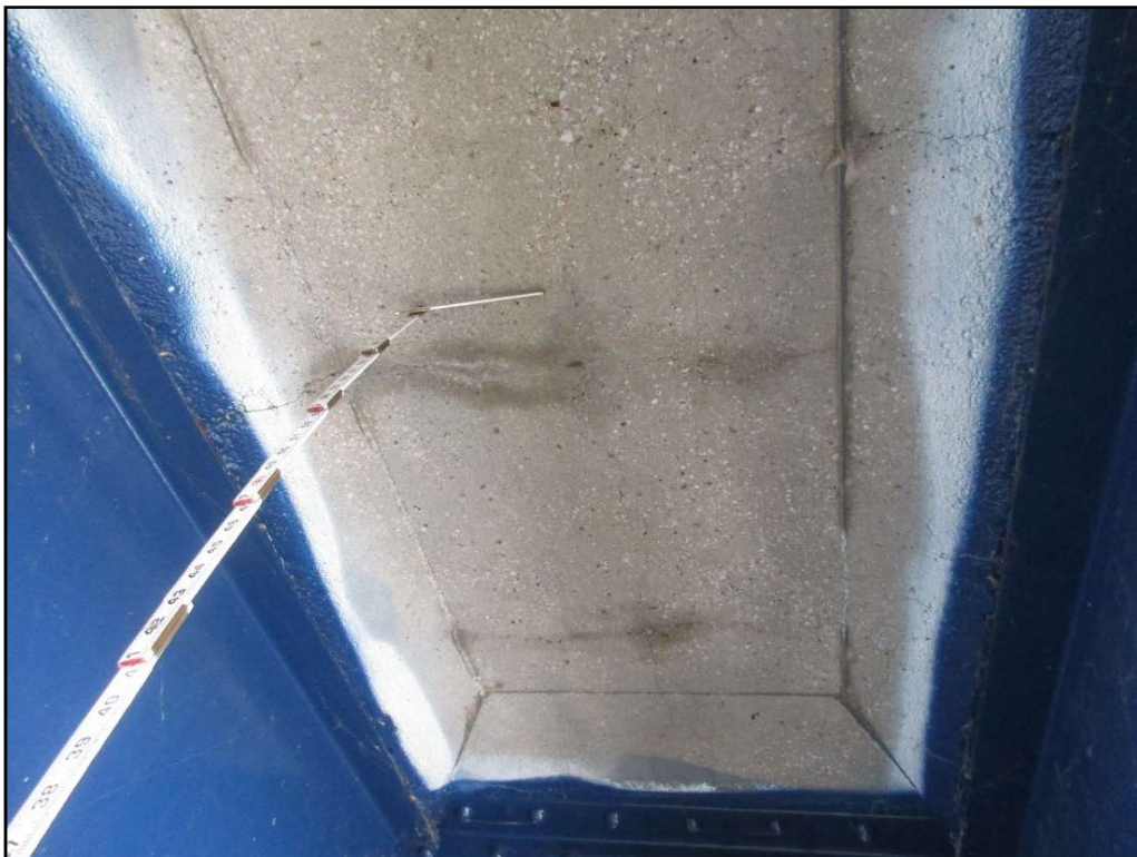
Photo 5 – Typical Transverse Crack in Underside of Deck with Efflorescence
