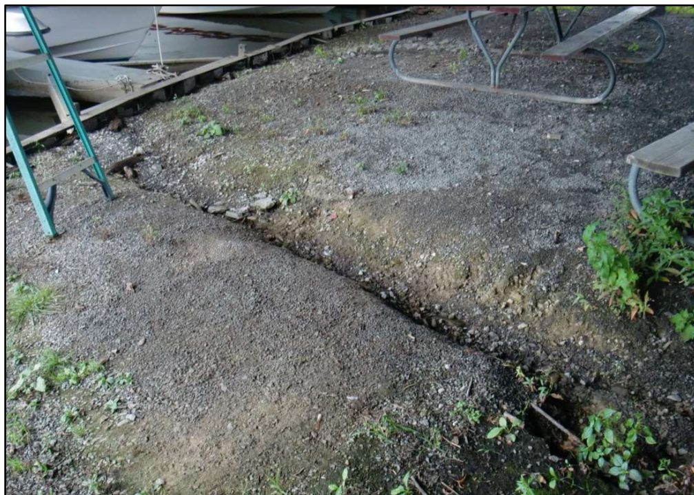
Photo 48 – Erosion Gully, Rear Abutment
