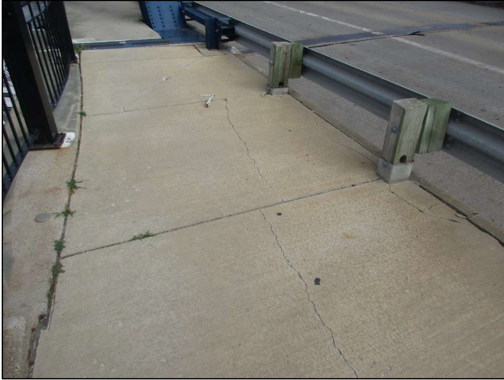
Photo 55 – Settlement & Vegetation, Southeast Approach Sidewalk
