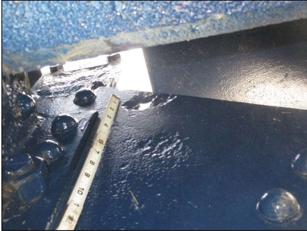
Photo 38 – Perforation at Top of Interior Gusset Plate, L4 South
