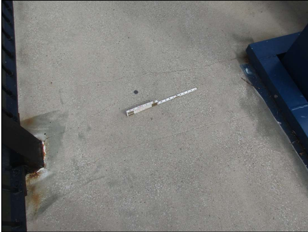
Photo 9 – Typical Transverse Cracking in Sidewalk
