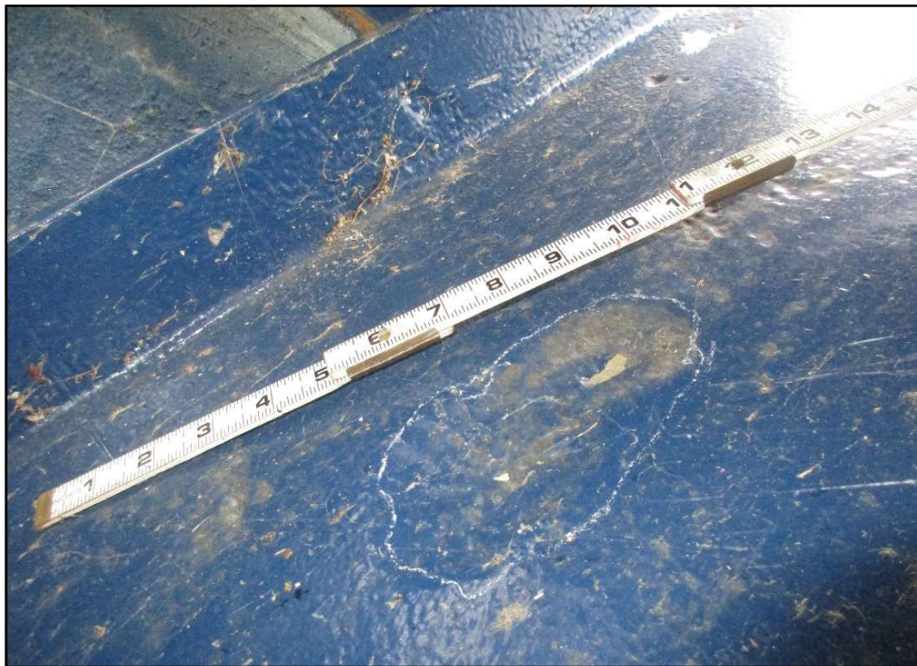
Photo 29 – Web Pitting with Perforation, U 5 L 6 North, Near L 6 North
