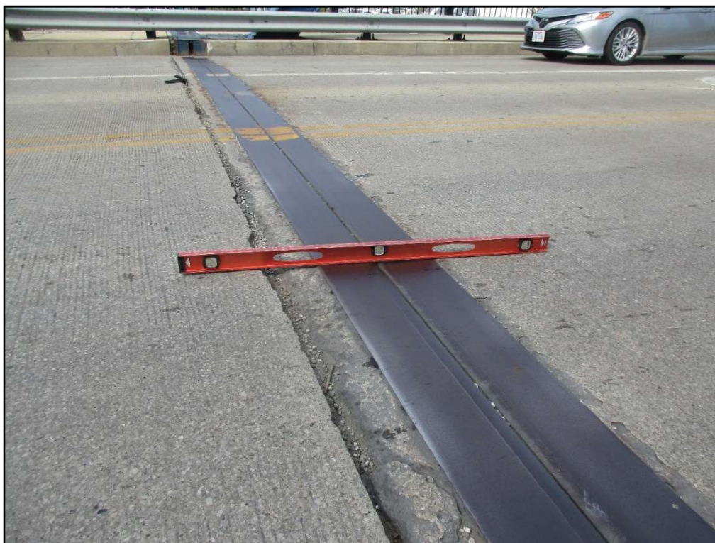
Photo 53 – Uneven Approach-to-Floor Transition, Rear Approach
