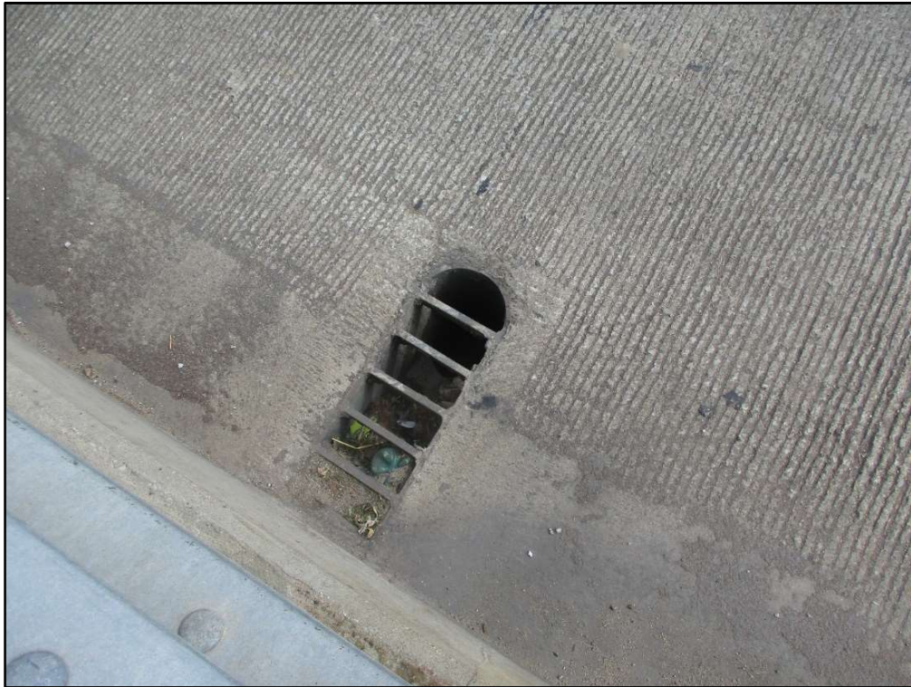
Photo 14 – Partly Clogged Scupper Inlet, North Curb
