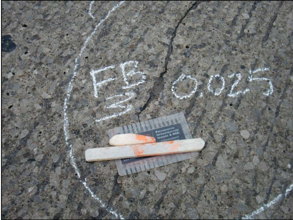
Photo 4 – 0.025" Wide Transverse Crack in Deck, Near Floorbeam 3
