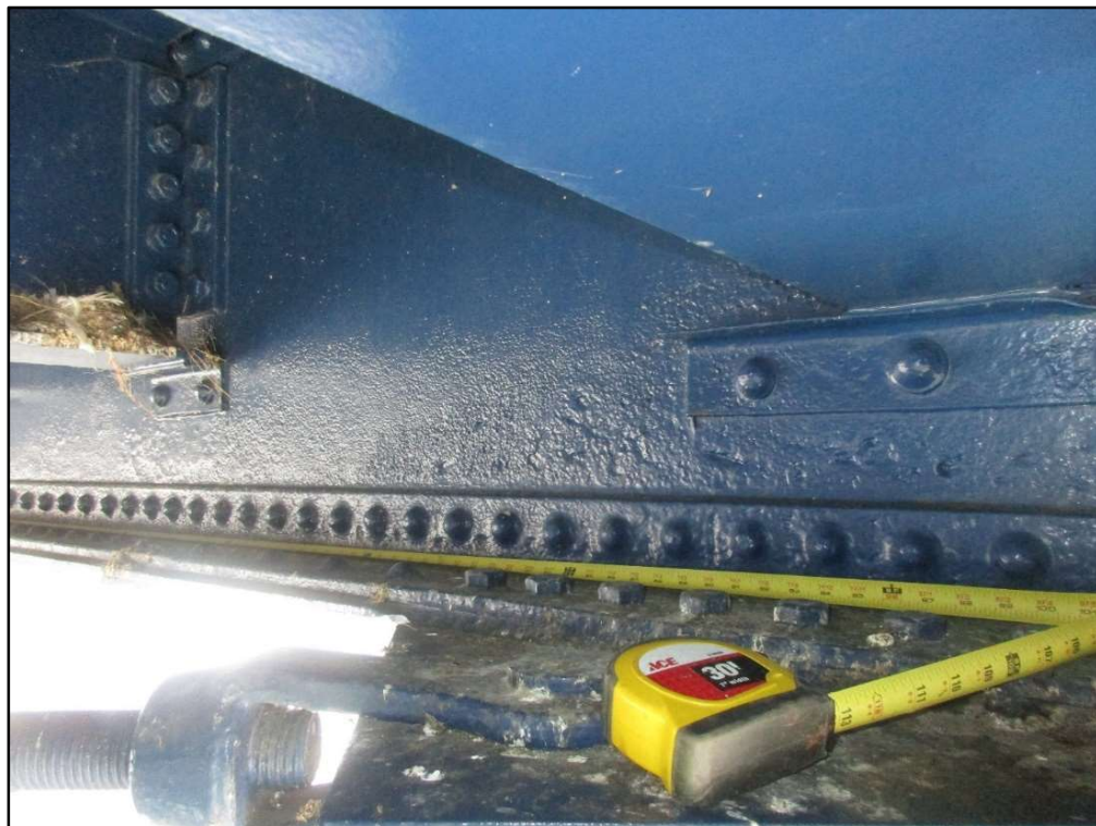
Photo 24 – Typical Pitting to Floorbeam End & Bottom Flange Angle, Near Truss Connection
