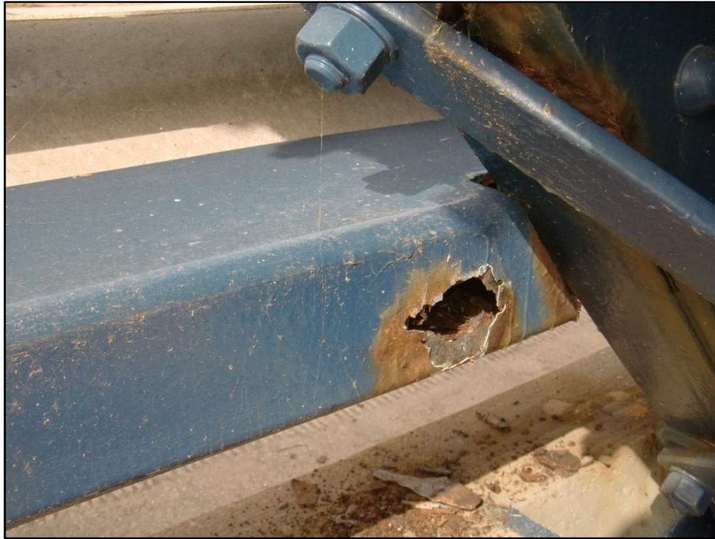
Photo 10 – Active Corrosion with Perforation, Railing Tubular Steel Backup, near L 9 South
