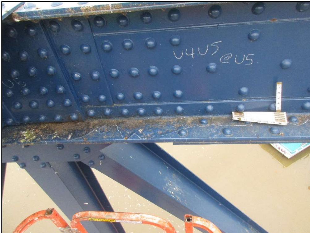
Photo 30 – Pitting to Bottom Flange Angle, U4U5 South
