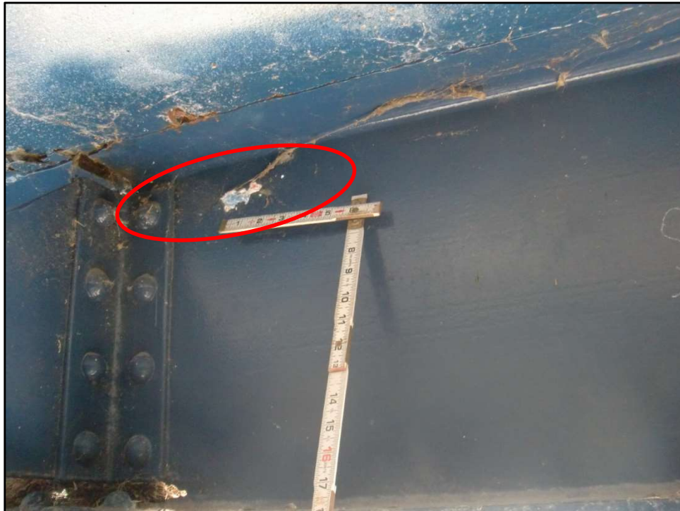
Photo 21 – Typical Web Perforations (Circled), Exterior Sidewalk Stinger
