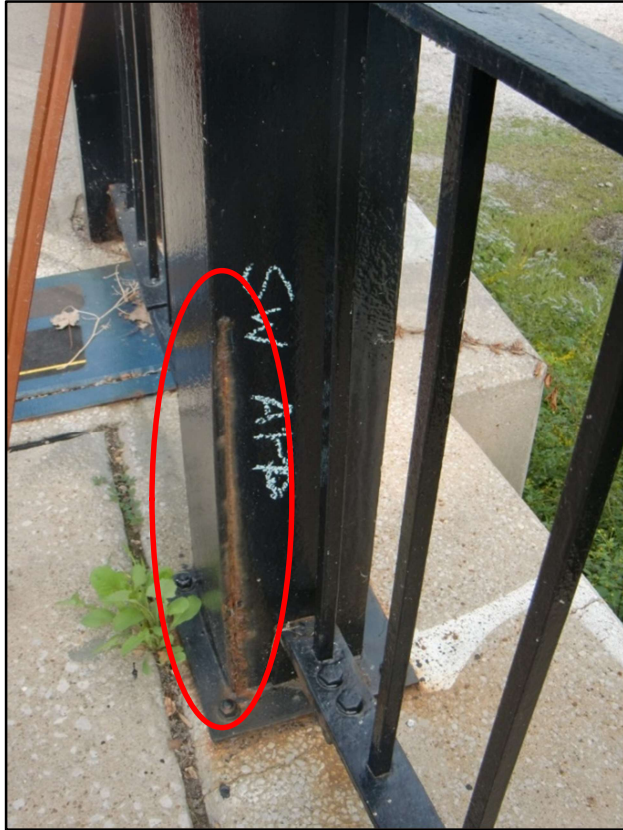
Photo 12 – Vertical Crack in Railing Post (Circled), Southwest Approach
