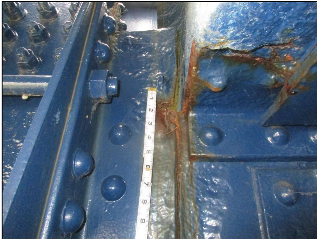
Photo 22 – Pitting with Edge Hole in Connection Angle, Floorbeam 1 at L1 South
