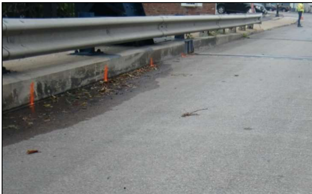
Photo 16 – Minor Ponding & Debris Along Edge of Deck, Southwest Curb
