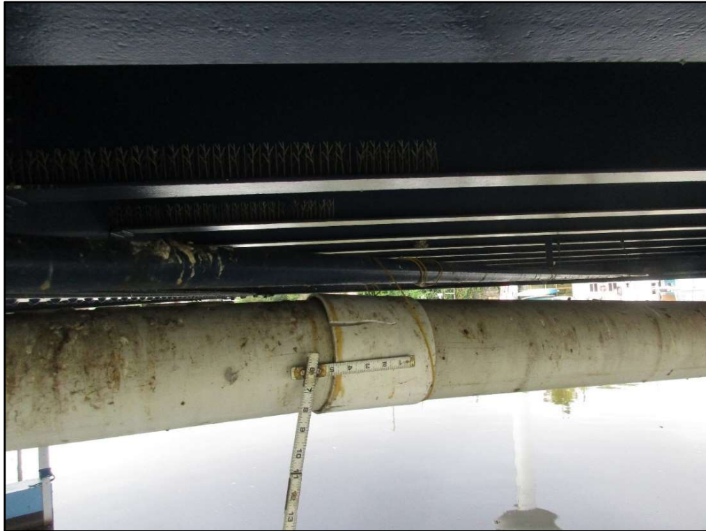
Photo 15 – Cracked Drain Pipe Coupling, Northeast Corner
