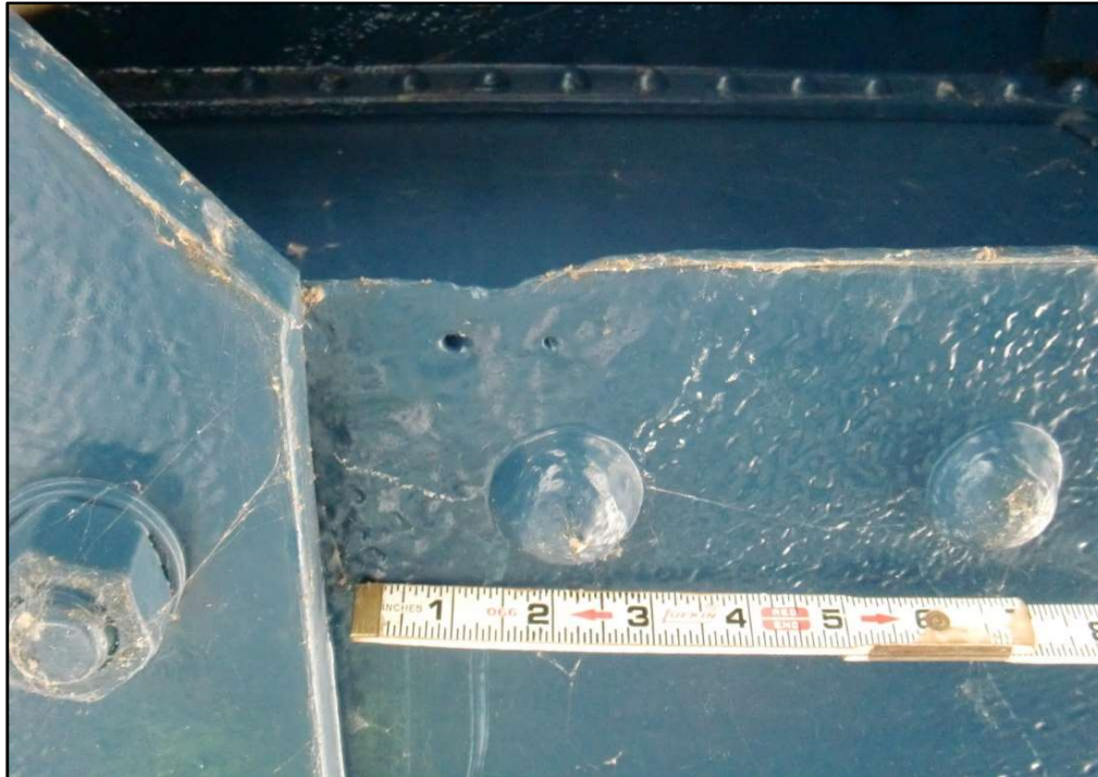
Photo 25 – Pitting with Pinholes to Bottom Flange, Floorbeam 5 at North Lower Lateral Brace Connection Plate
