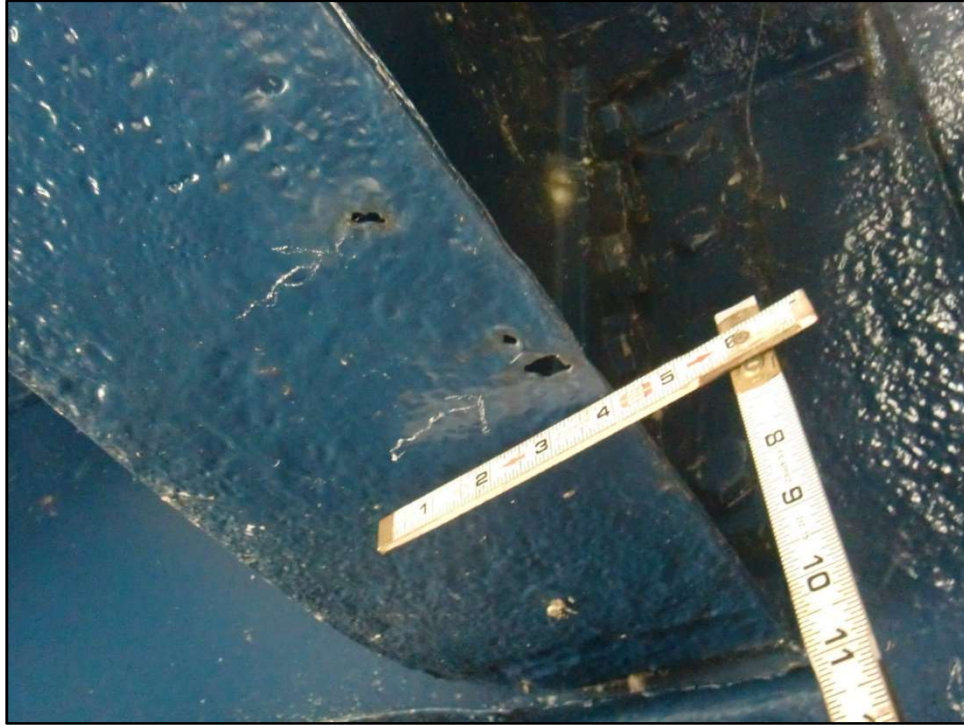
Photo 20 – Bottom Flange Pitting with Perforations, Stringer 1, Panel 7
