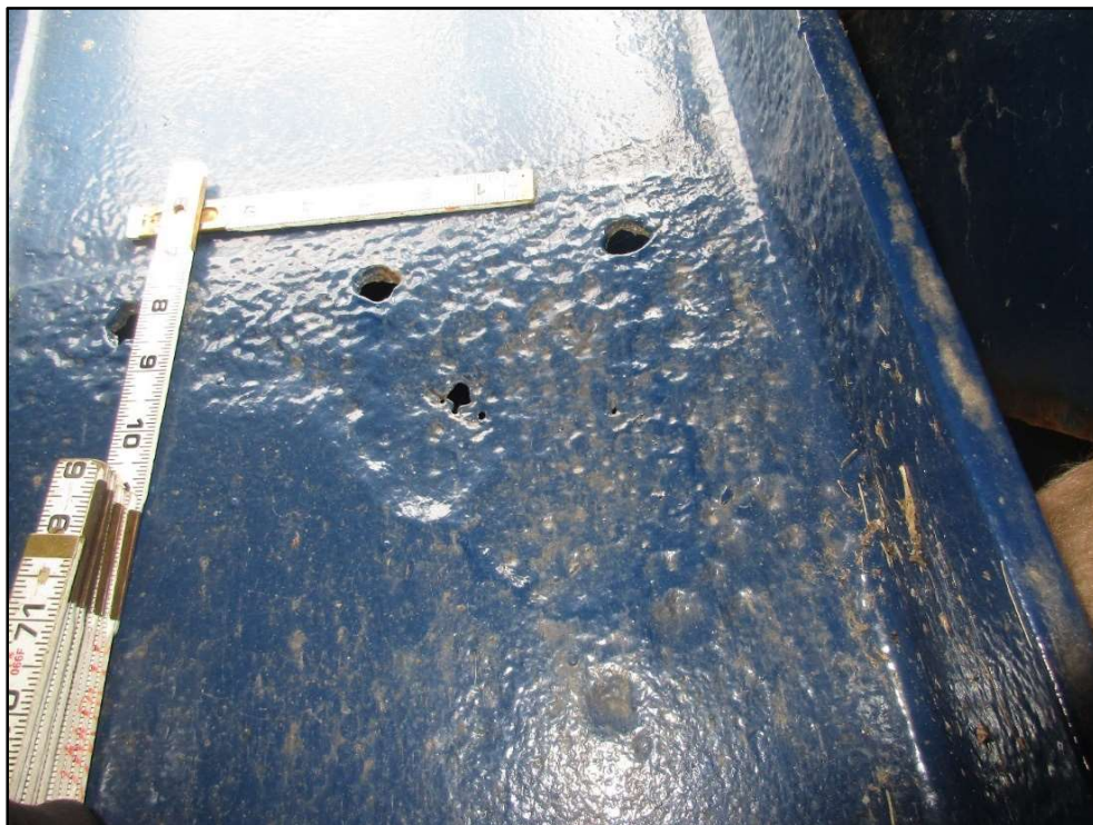
Photo 27 – Web Pitting & Perforations, L 6 U 6 North
