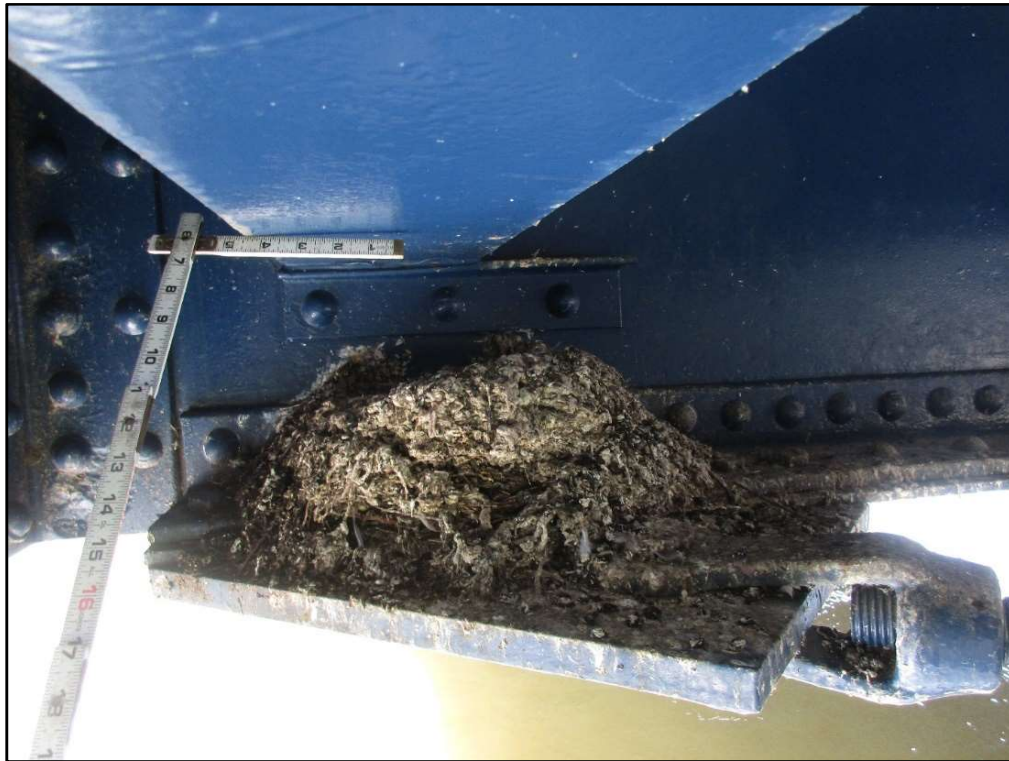
Photo 45 – Typical Pigeon Manure Pile, Lower Lateral Bracing Gusset Plate
