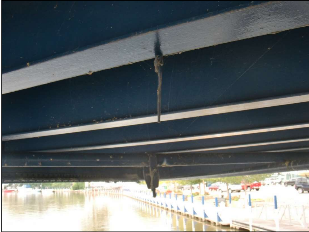
Photo 39 – Broken Lower Lateral Bracing Rod Hanger, Panel 7
