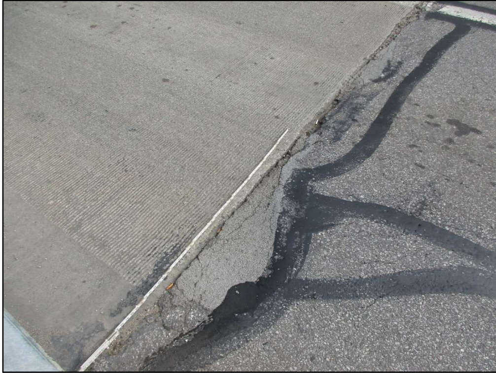
Photo 50 – Deteriorating Approach Wearing Surface Patch, West Approach
