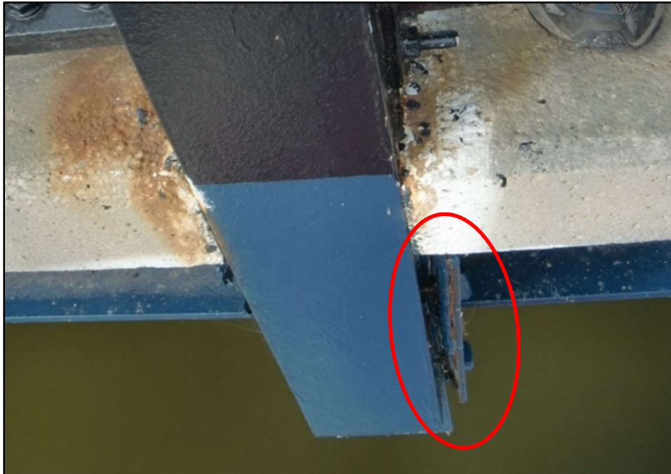
Photo 13 – Advanced Section Loss to Abandoned Railing Post Connection Assembly (Circled)
