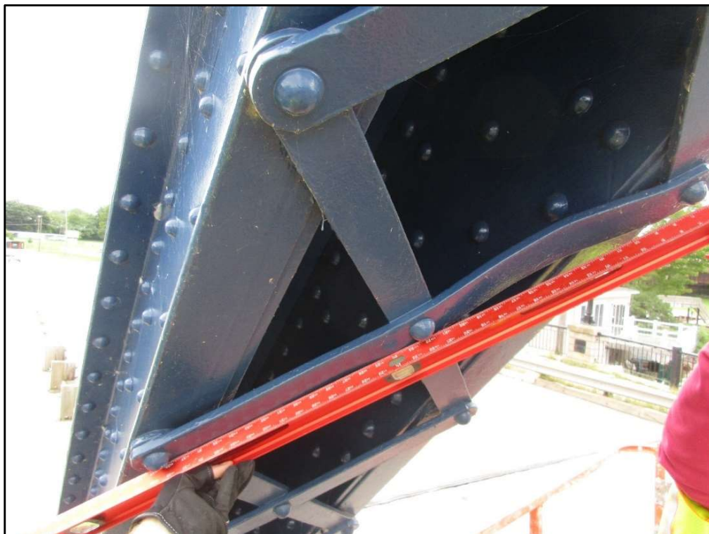
Photo 32 – Typical Bent Lacing Bar, U 8 L 9 North
