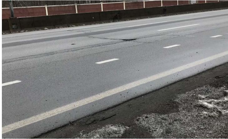
Photograph 3: IR-77 Pavement (Concrete)
