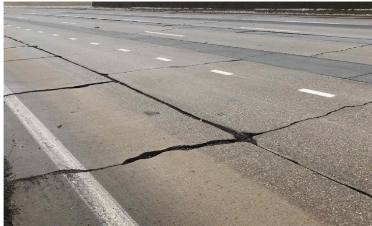
Photograph 5: Ramp P Concrete Pavement
