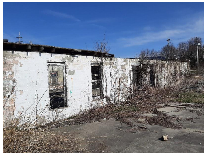
Rear of building
