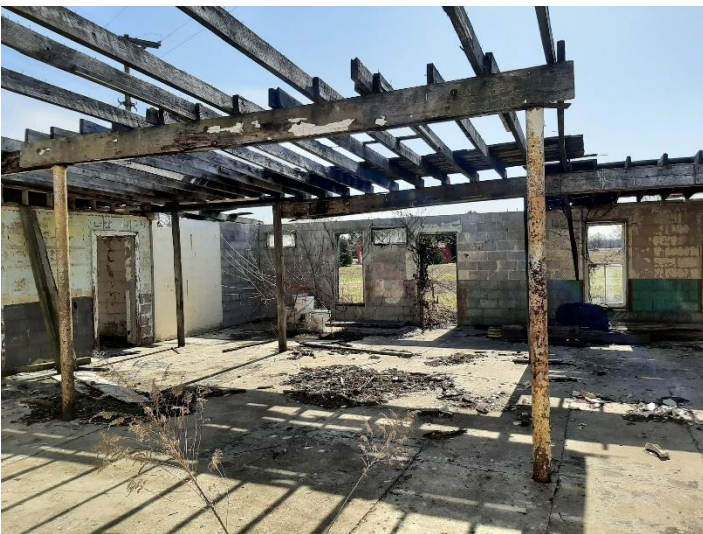
Interior of building
