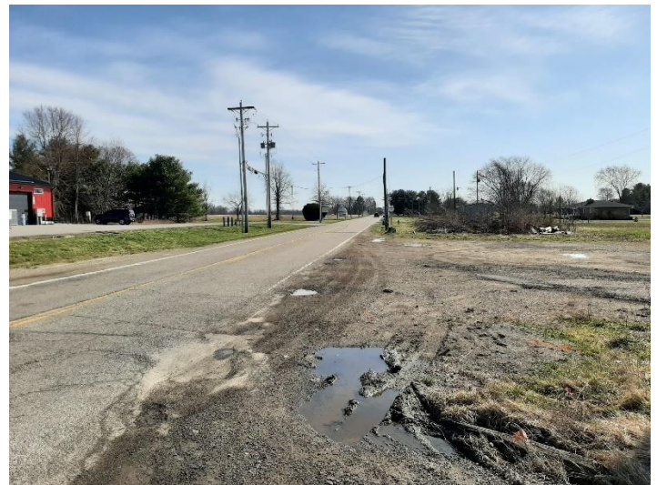
State Route 256 looking east
