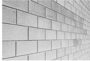
Concrete blocks are concrete masonry units, or CMUs, but we often refer to them as concrete blocks or cinder blocks. Learn more about [concrete masonry units](#). A wall typically requires  $1\frac{1}{8}$  blocks per square foot.
