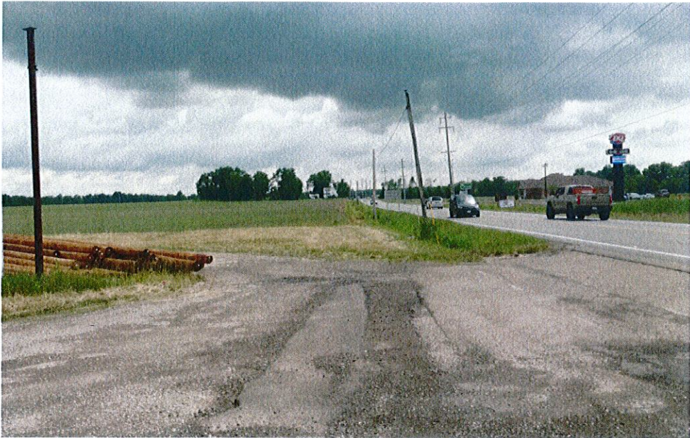
View looking south along Lancaster-Newark Road at SH-1 and T-1
