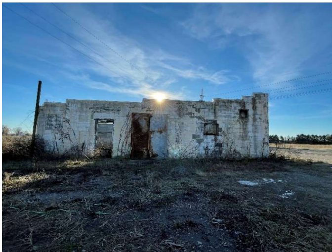
SIDE (Facing South-West from SR-256)
