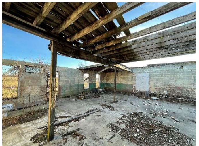
INSIDE (Facing South at Rear and Side)
