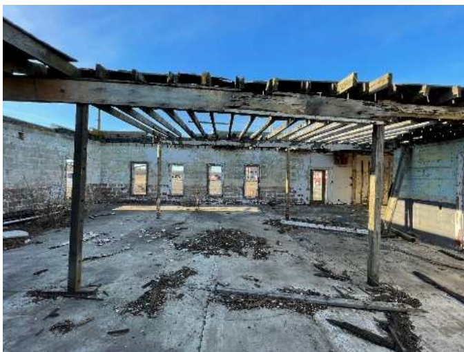
INSIDE (Facing North-West at Front)
