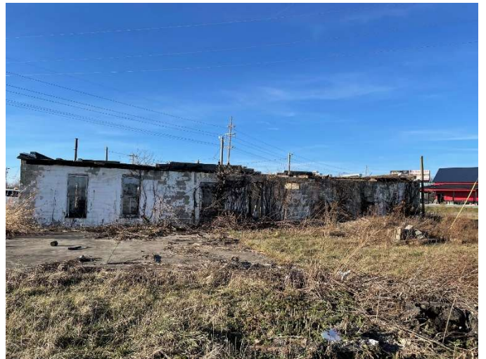
REAR (Facing North-West from Field)
