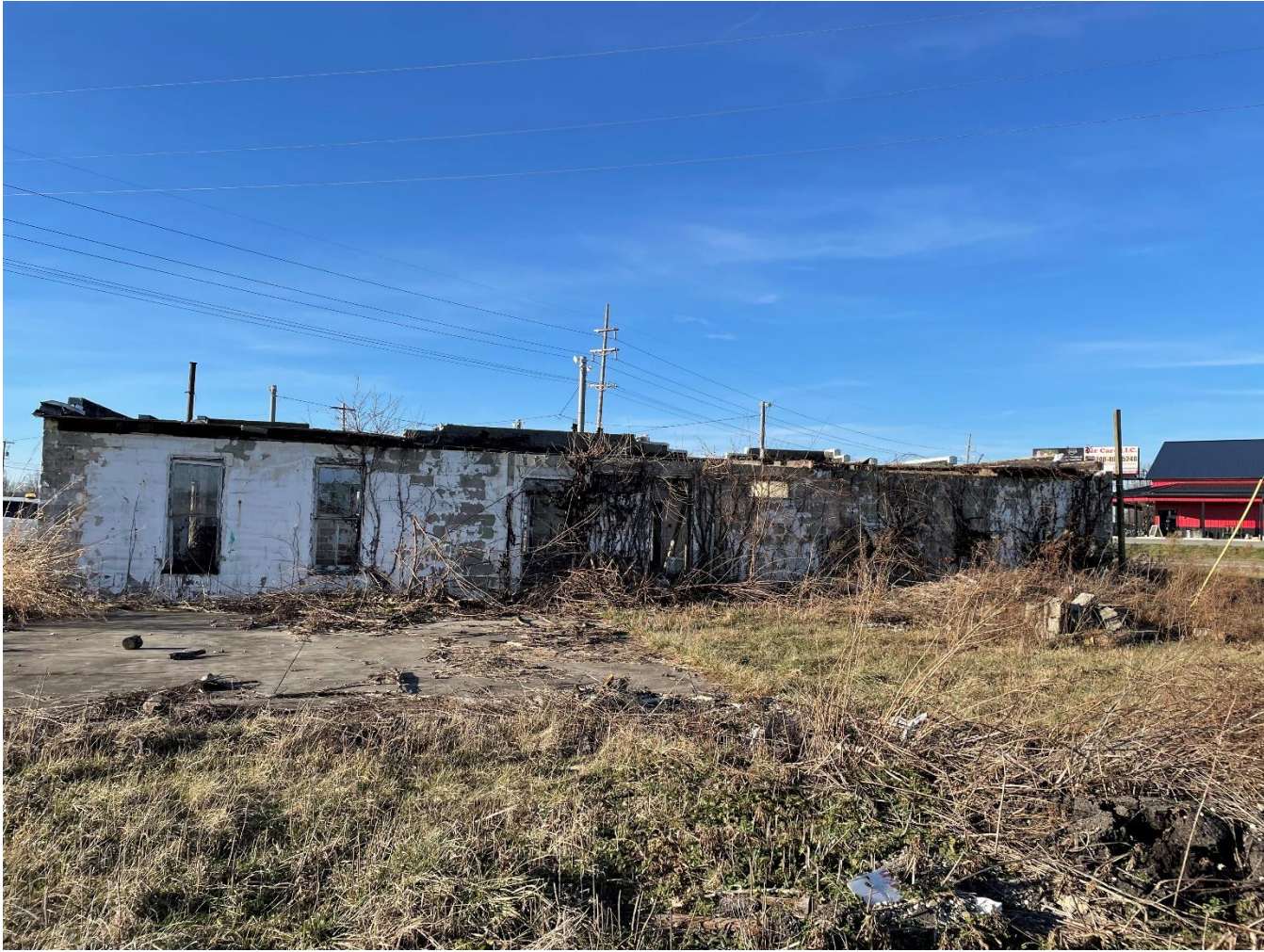
REAR (Facing North-West from Field)
