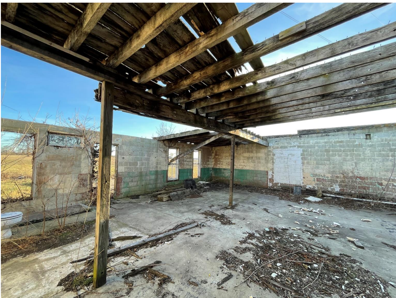
INSIDE (Facing South at Rear and Side)
