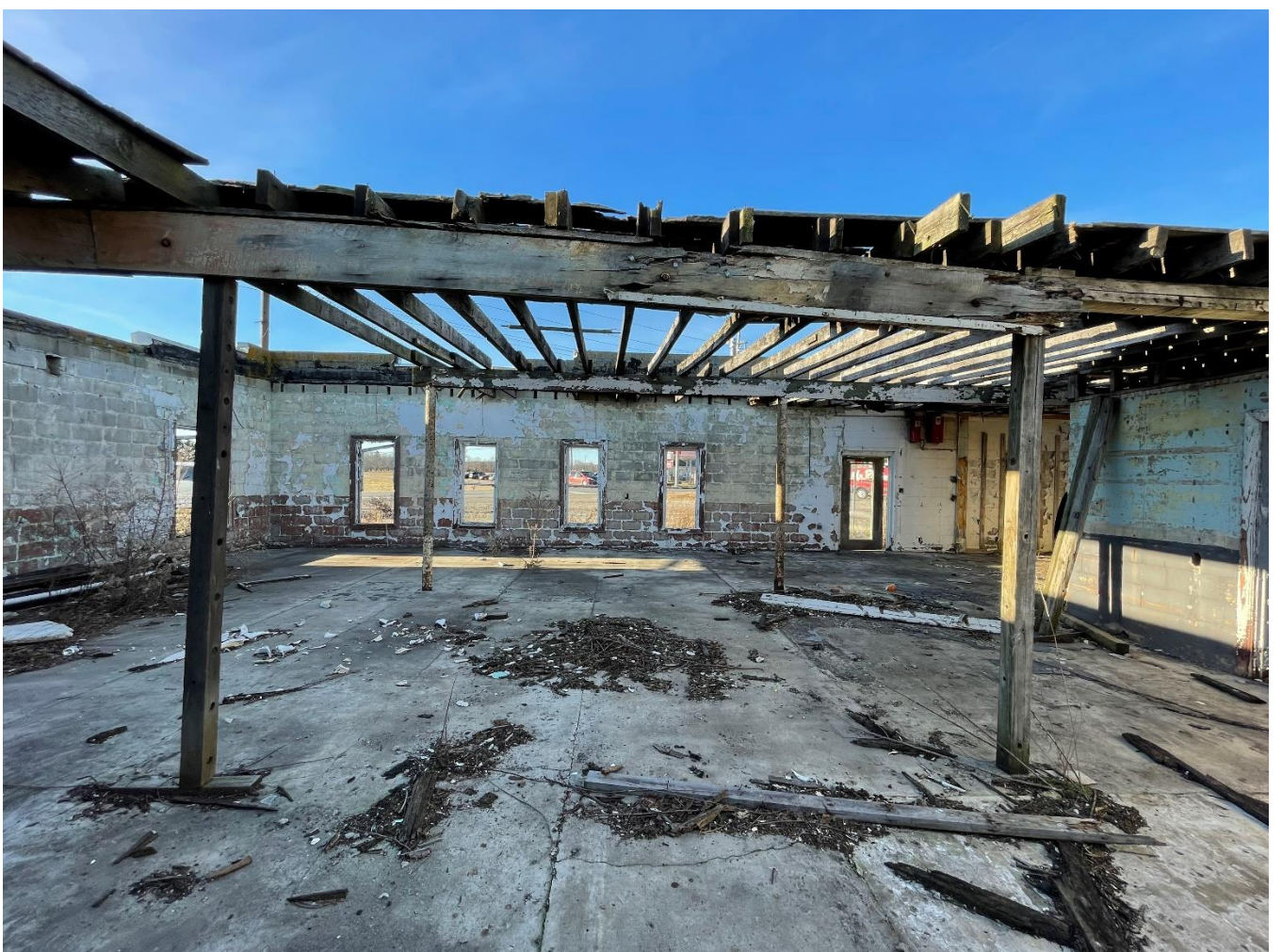
INSIDE (Facing North-West at Front)
