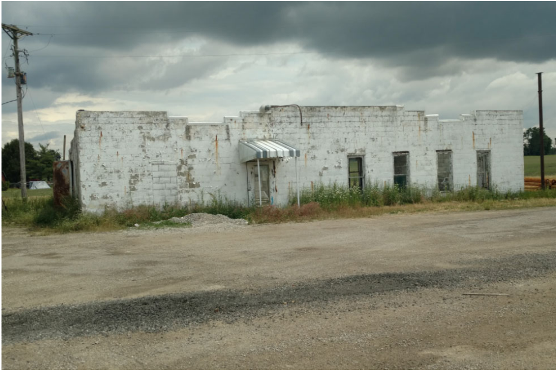
View looking southeast at dilapidated structure
