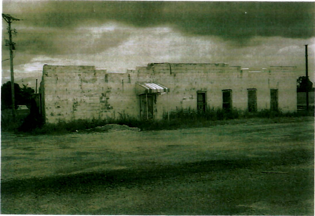
View looking southeast at dilapidated structure
