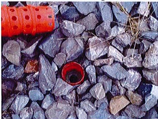
below-riser inlet showing restrictive orifice plate
