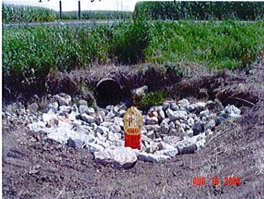
below-riser inlet showing restrictive orifice plate
