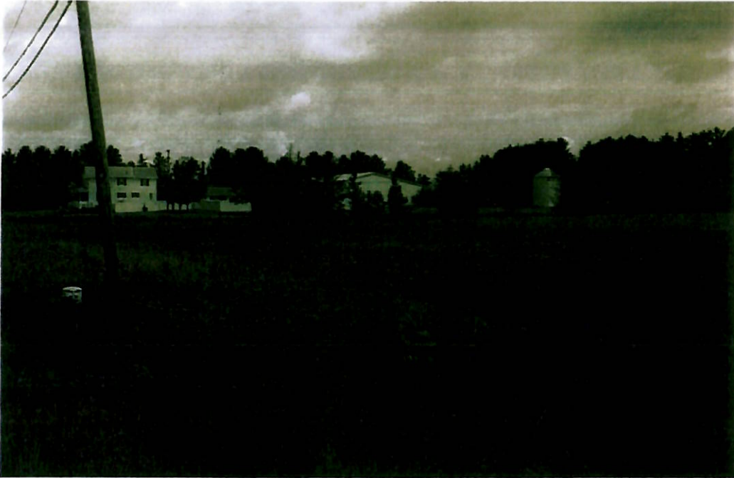
View looking east along the proposed acquisition SH1 and Baltimore-Somerset Road
