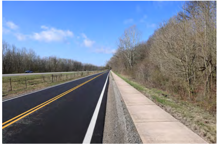
Example of a good sidewalk project location along Marne Rd. S-27 on project list.
