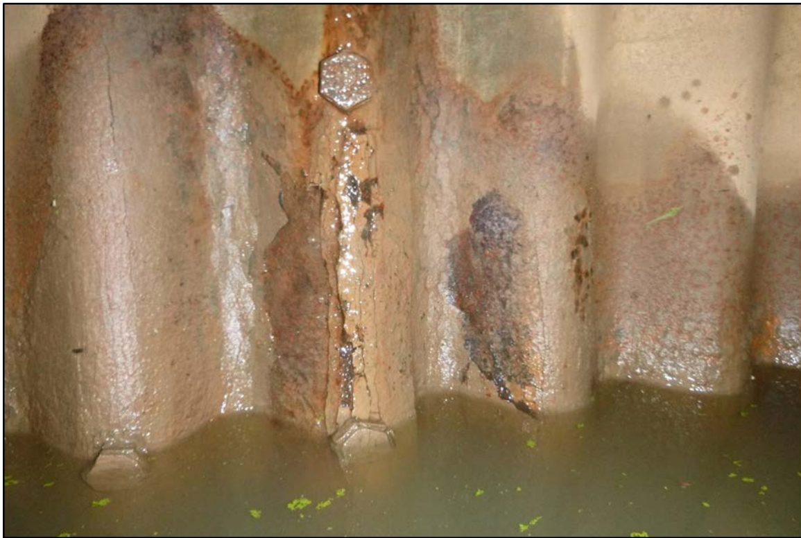
Photograph No. 10: View of the Typical Corrosion on the Vertical Joints of the Structure, Looking West.
