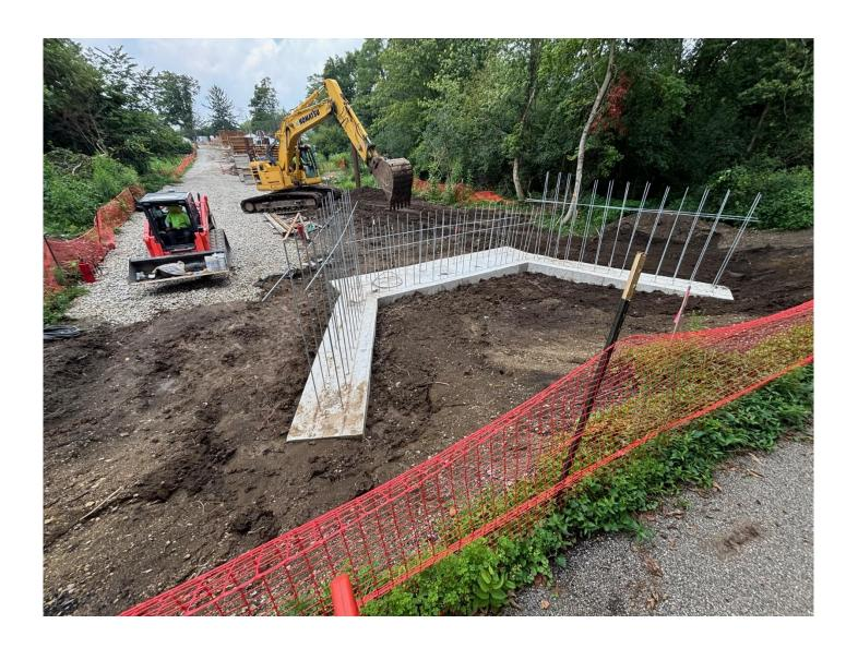
Blackswamp working on installing galvanized reinforcing in the piers.
