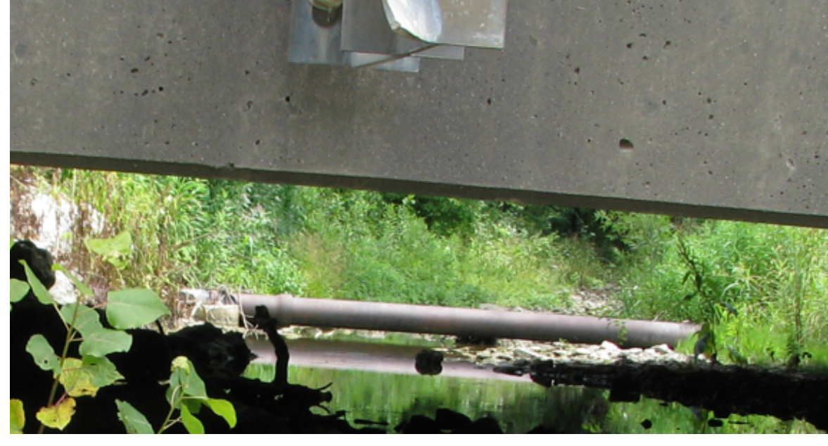
2008 inspection photo showing aerial crossing
