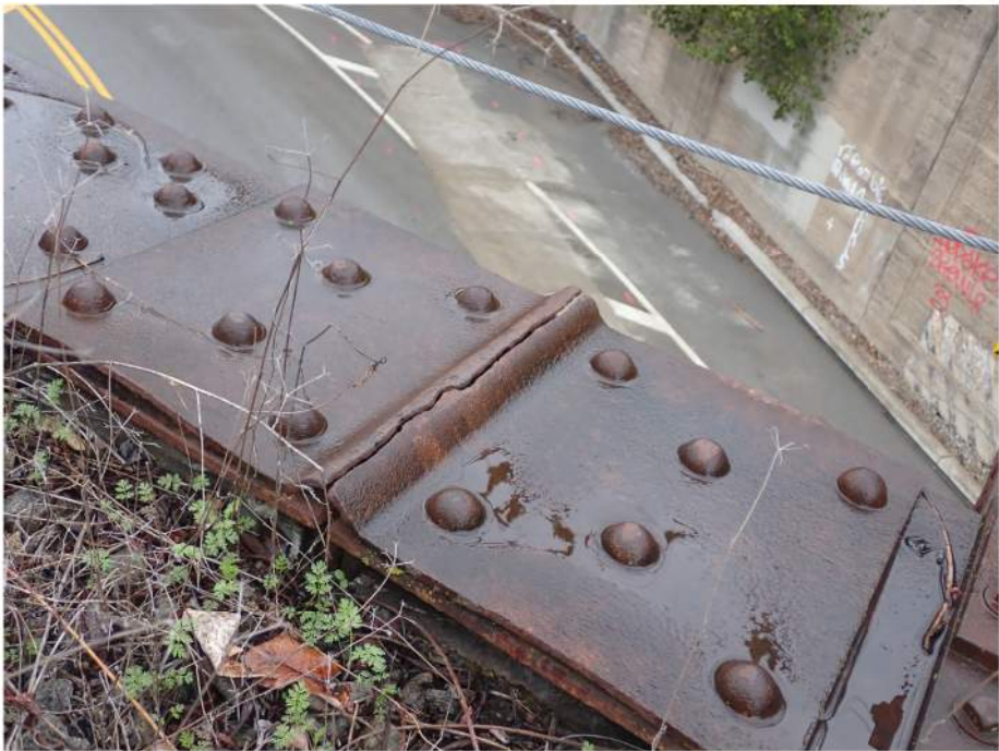
BROKEN TOP FLANGE SPLICE PLATE FOR EACH GIRDER
