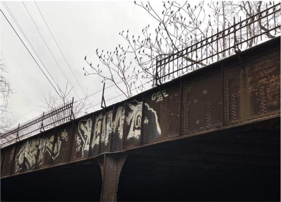
MISSING FENCE SECTIONS ALONG THE NORTH GIRDER
