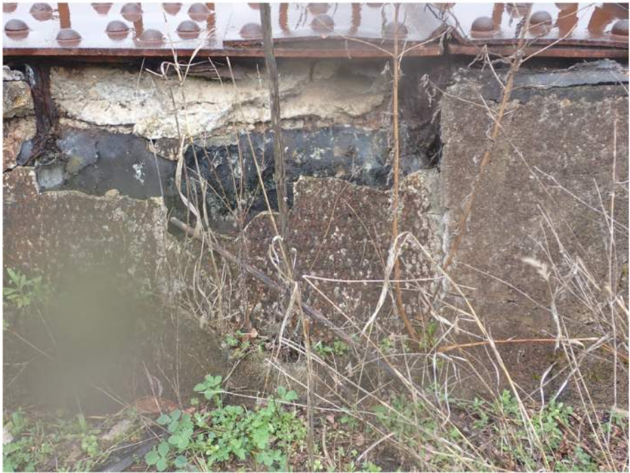
SPALLED CONCRETE AT INSIDE FACE OF TPG
