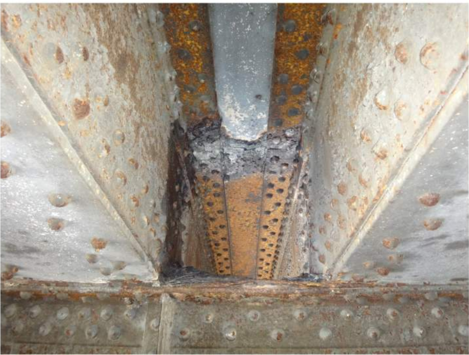
WATER LEAKING THROUGH DECK JOINT
