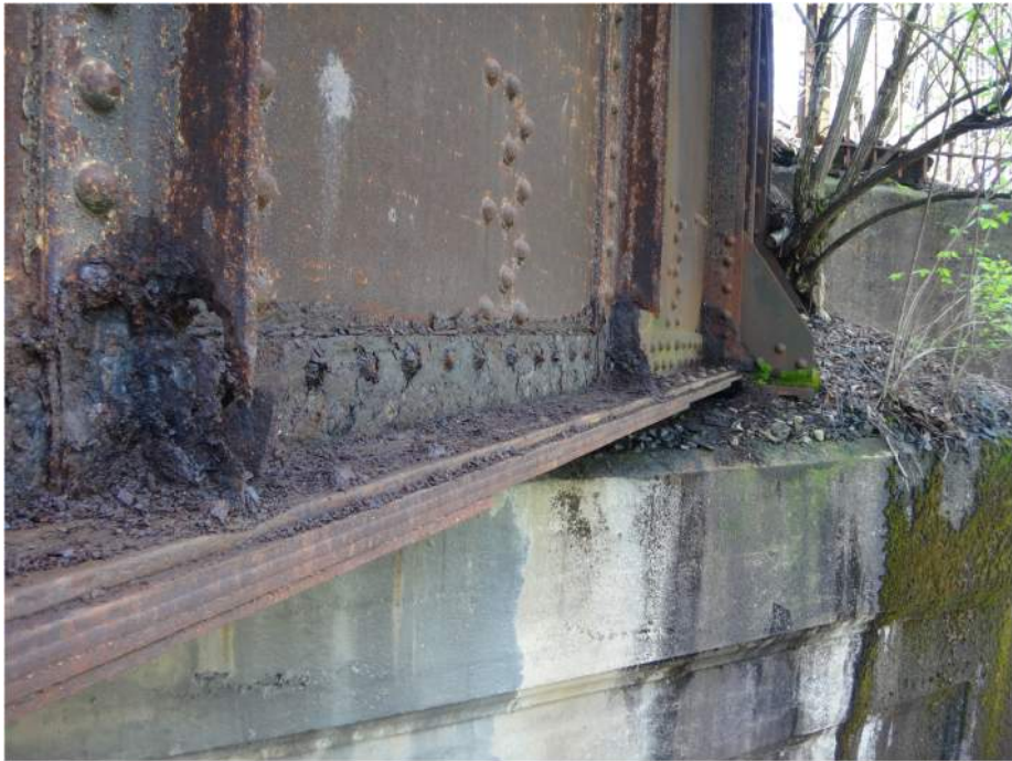
STEEL DELAMINATION AT BOTTOM FLANGE ANGLE, STEEL DETERIORATION STIFFENER ANGLE, AND LEAKING BALLAST AND INVASIVE FLORA
