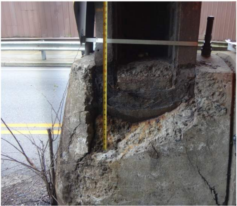
SPALLED CONCRETE AT PIER WALL, VEGETATION AROUND THE PIER WALL, AND STEEL PIER
