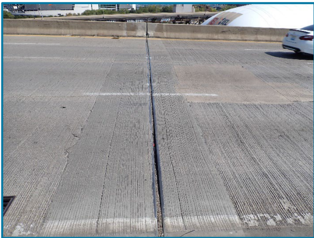
Photo 13 – Typical expansion joint at Pier 8A (looking east).
