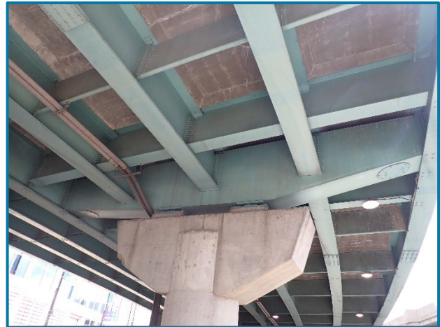
Photo 131 – Pier 2 (FWW) south elevation (looking north).
