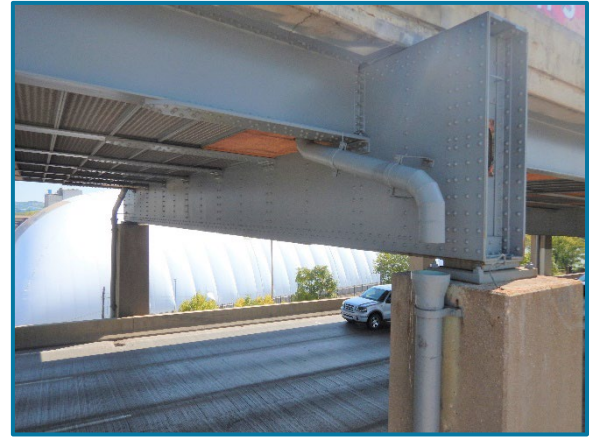
Photo 90 – Pier Cap 6A north elevation (looking southeast).
