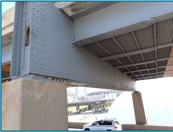
Photo 84 – Pier Cap 5A south elevation (looking northeast).
