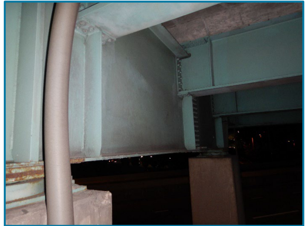
Photo 128 – Pier 29B south face at the west end (looking east).
