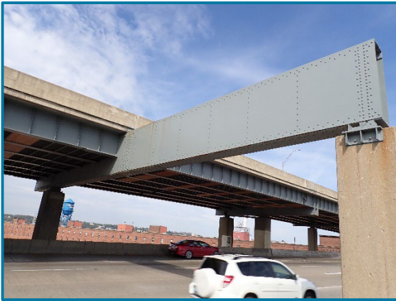
Photo 115 – Pier Cap 11A south elevation (looking northwest).
