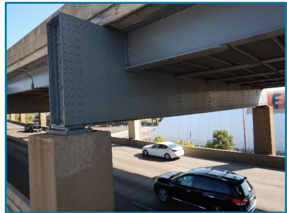
Photo 75 – Pier Cap 3A north elevation (looking southwest).
