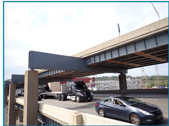
Photo 111 – Pier Cap 10A north elevation (looking southwest).
