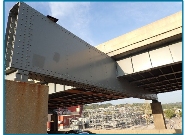
Photo 104 – Pier Cap 9A north elevation (looking southwest).
