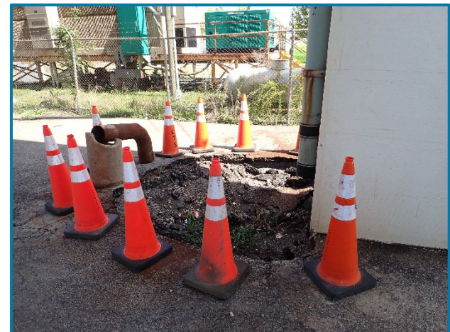
Photo 23 – Erosion at the base of Column 2 on the north side of Pier 4A (looking east).
